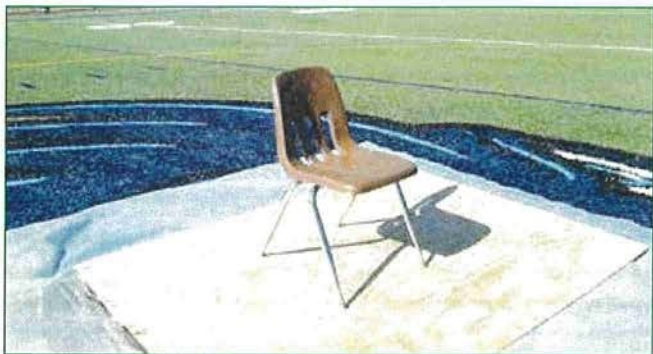
Spread Static Loads with Polyethylene Sheets and Plywood
