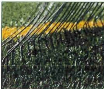
Work infill in with a rake
