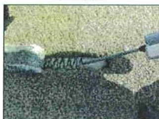
Apply adhesive with 1/4" bead width
