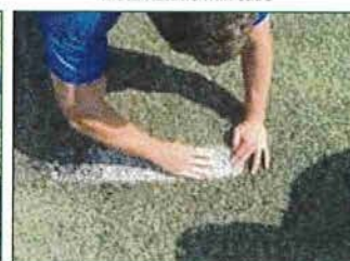
Reaffix turf, hold, and replace infill
