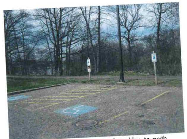
No connection from handicapped parking to path
