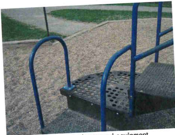
No ADA safety mat to playground equipment
