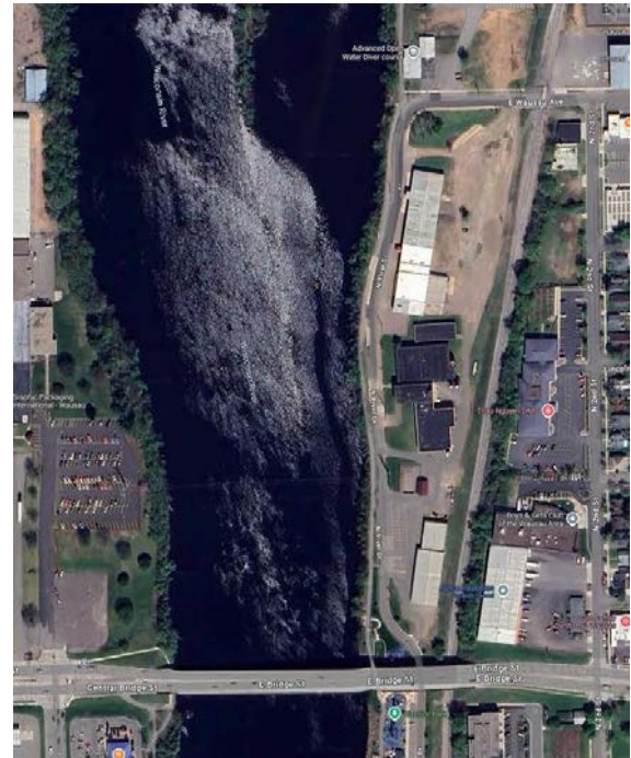
WATER PLANT DEMOLITION STRATEGIC REDEVELOPMENT LOCATION
