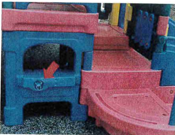
Play structure wheel is missing
