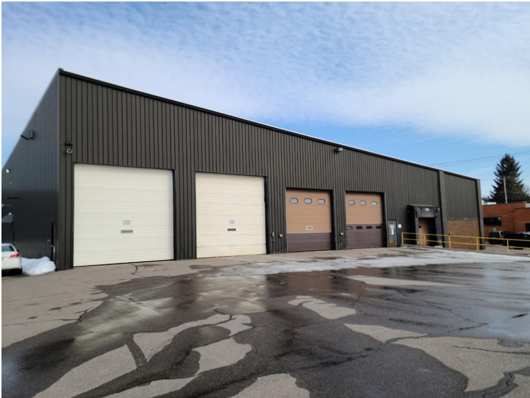
West side of the building and parking area
