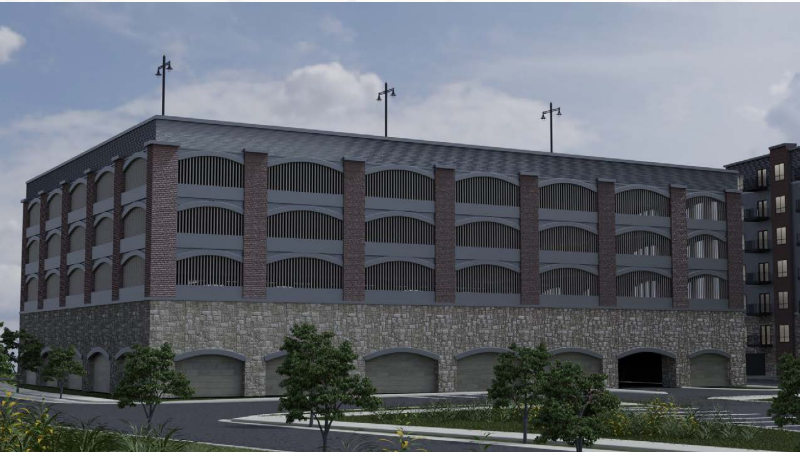
Parking Ramp Structure
