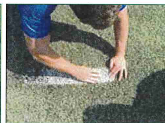
Reaffix turf, hold, and replace infill
