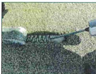
Apply adhesive with 1/4" bead width
