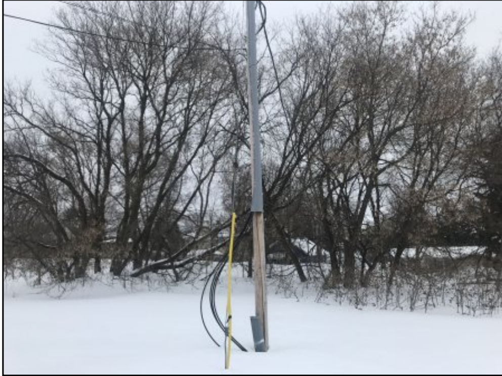
Overhead electric pole southeast of building
