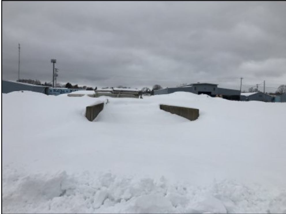
Concrete retaining wall from the previous building structure.
