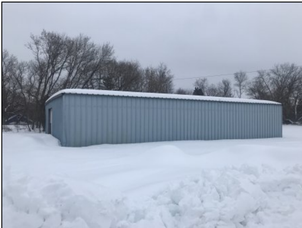
West side of remaining building
