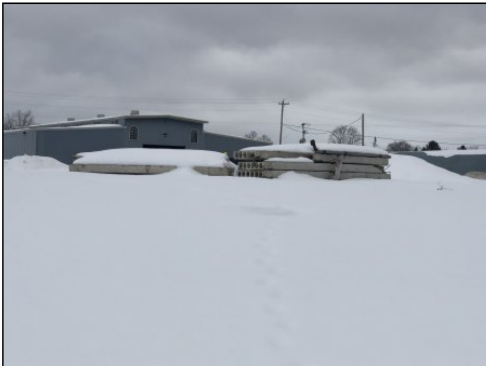
View of concrete debris located on the property.
