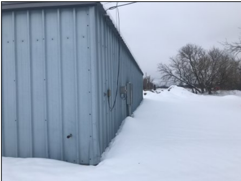
View north along each side of building
