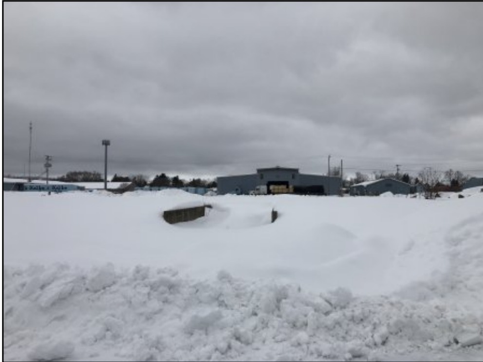
View of concrete retaining wall from previous building structure.
