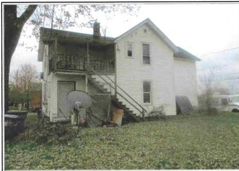
REAR OF SUBJECT PROPERTY
