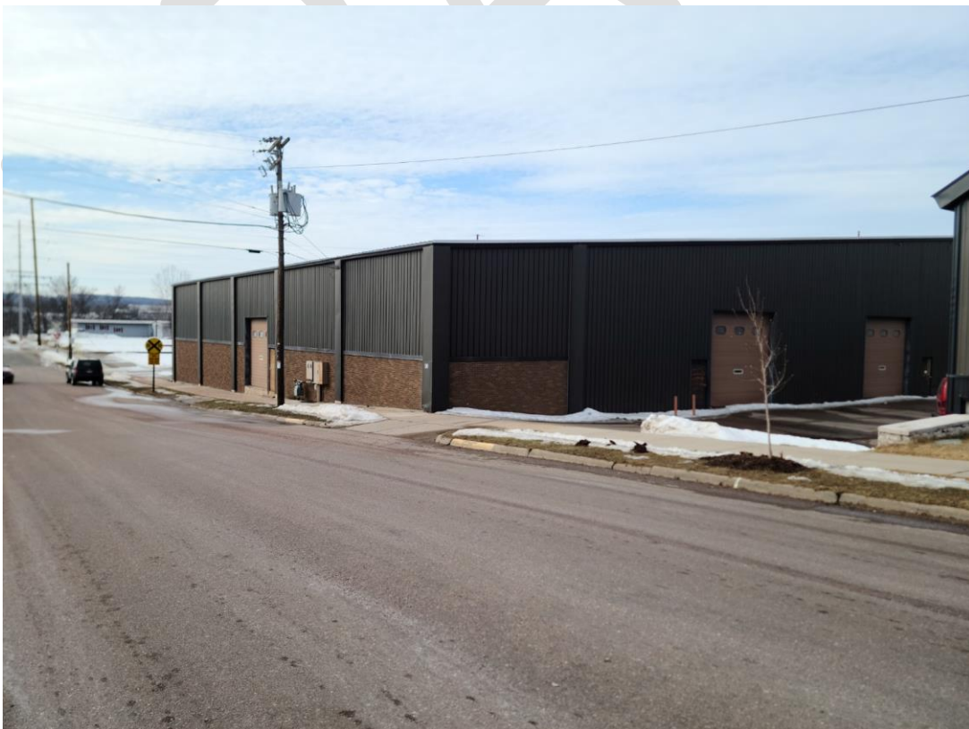
Southeast of the building looking across East Wausau Ave.
