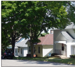
An older residential street.
