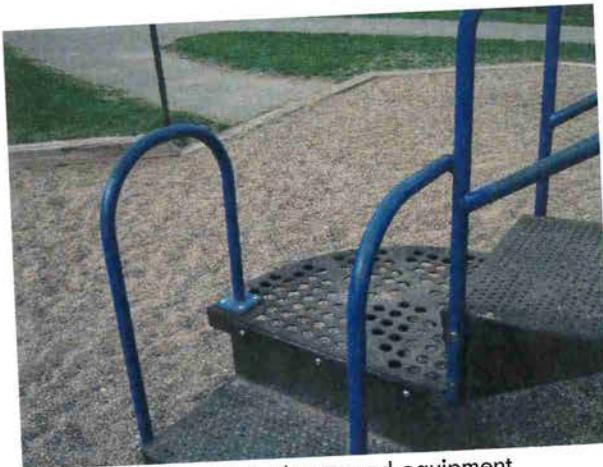
No ADA safety mat to playground equipment
