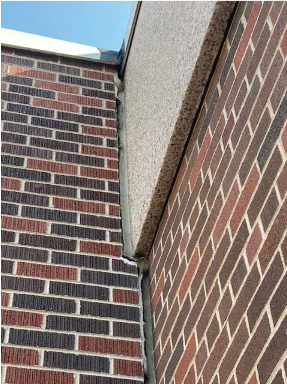
Building Control Joint Separation - Exterior
