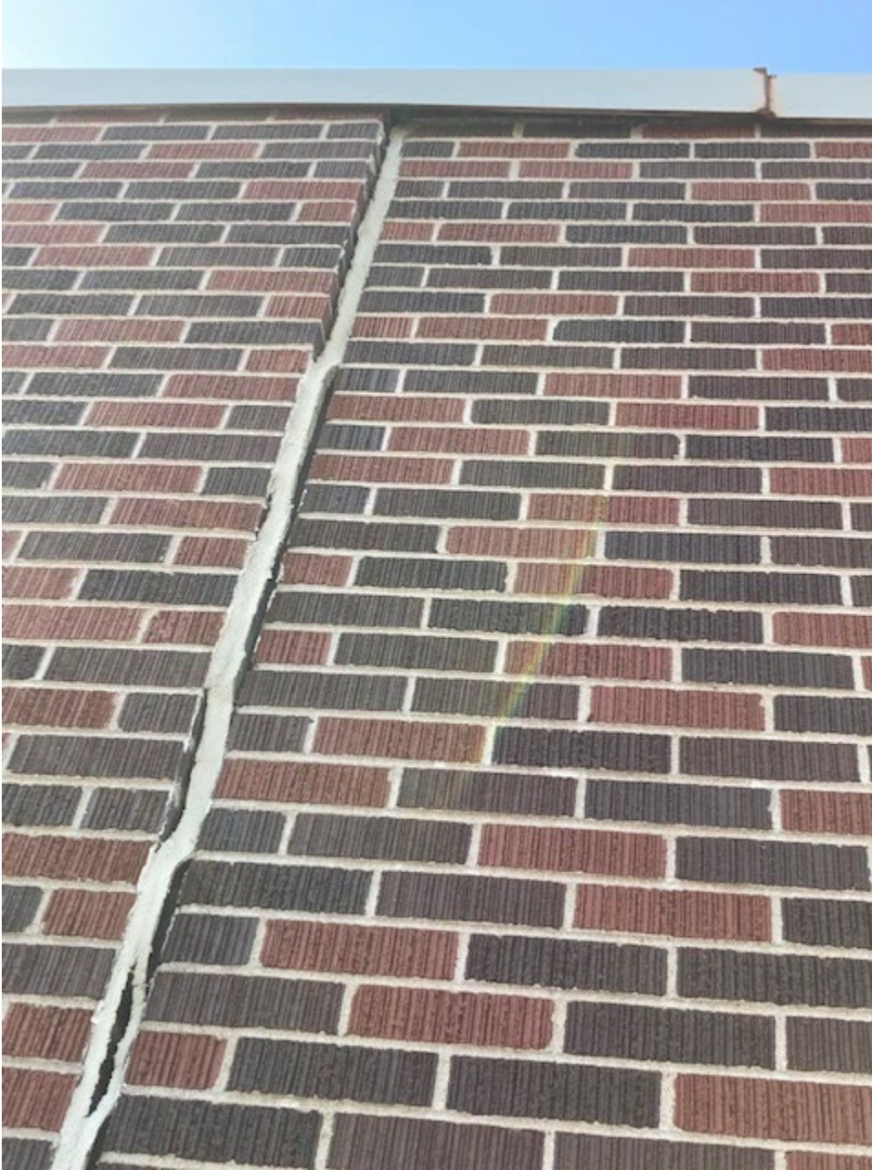
Building Control Joint Separation - Exterior
