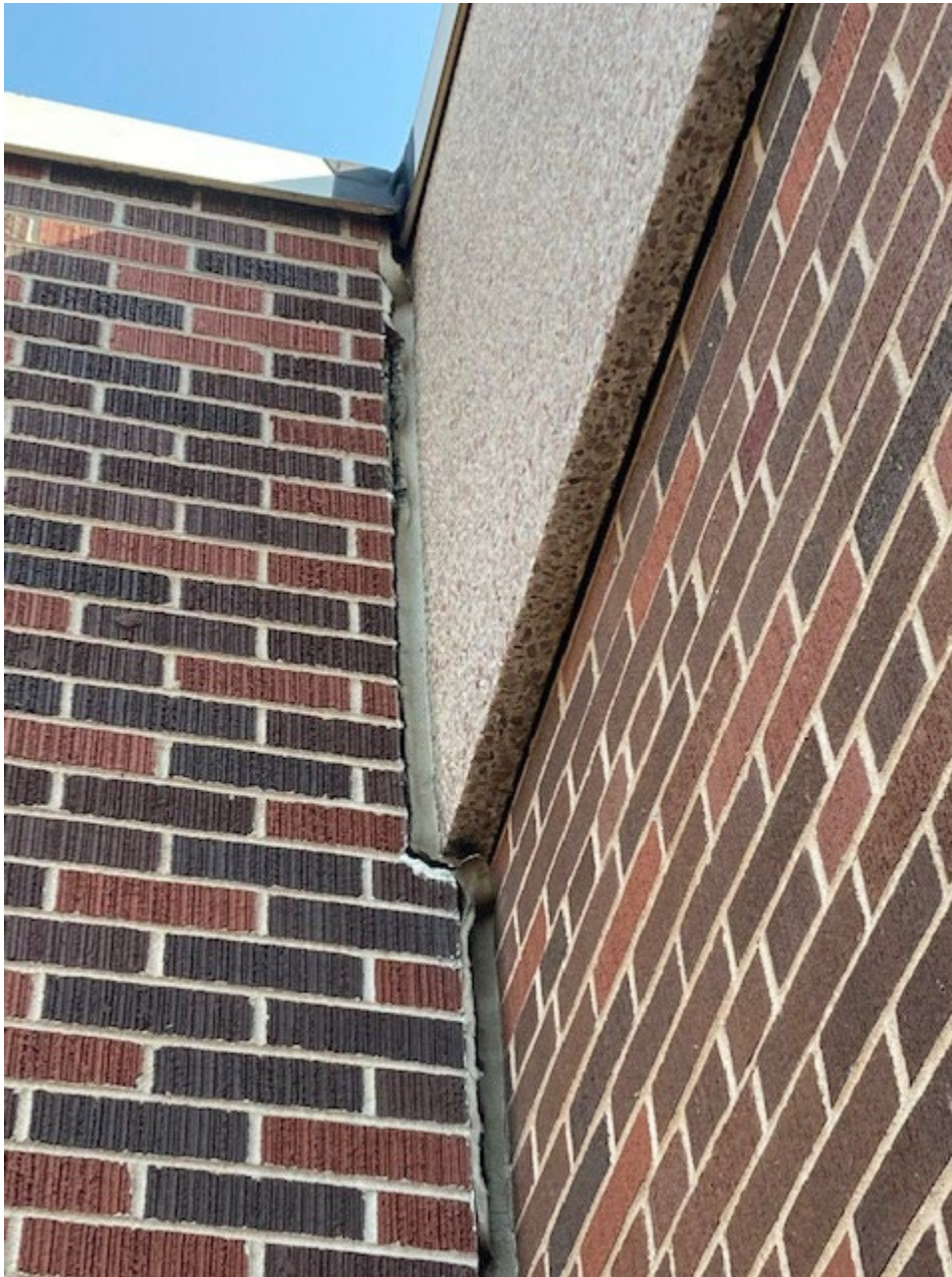
Building Control Joint Separation - Exterior
