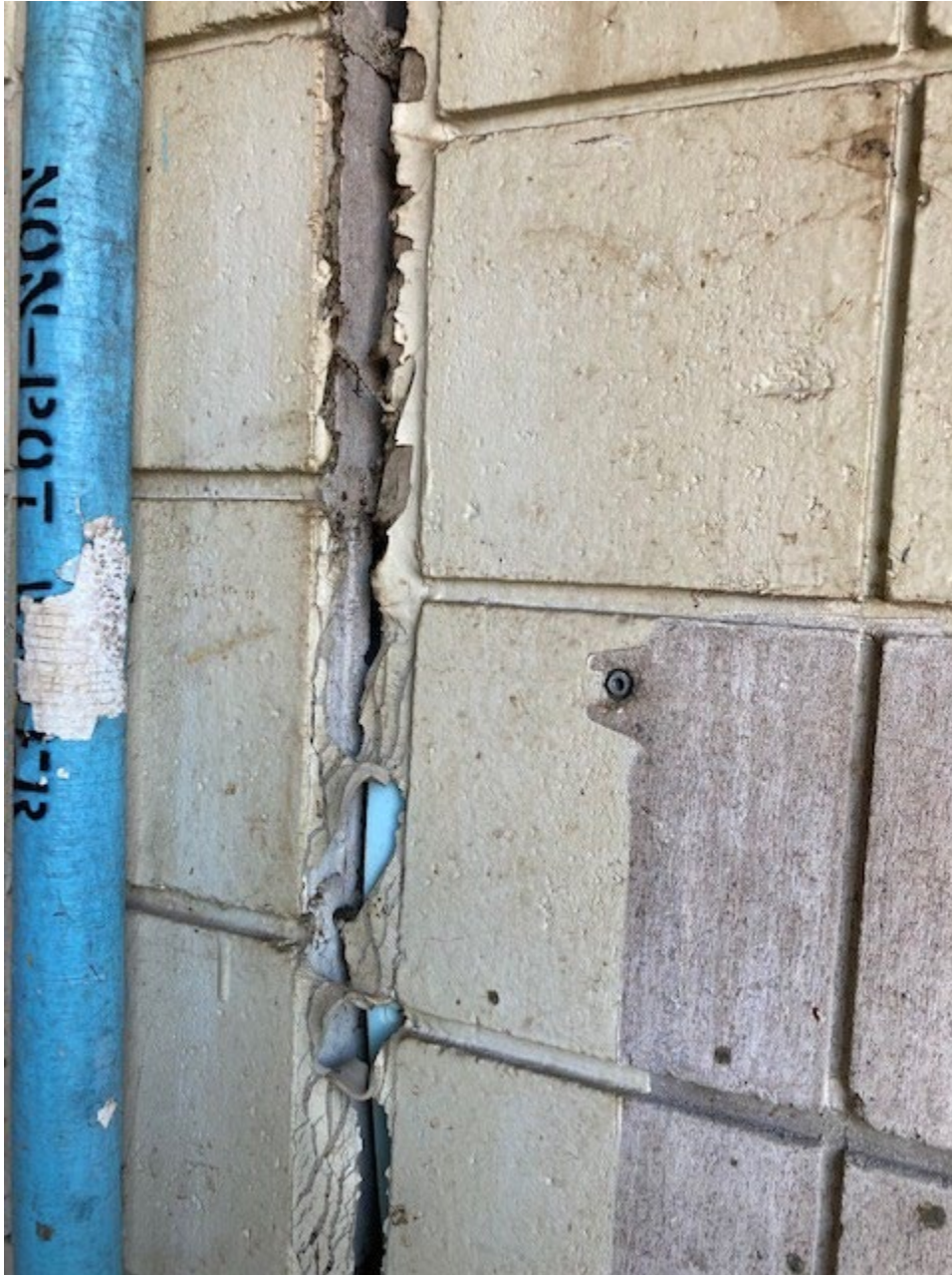
Building Control Joint Separation - Interior
