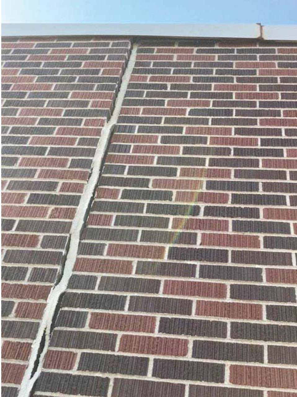
Building Control Joint Separation - Exterior
