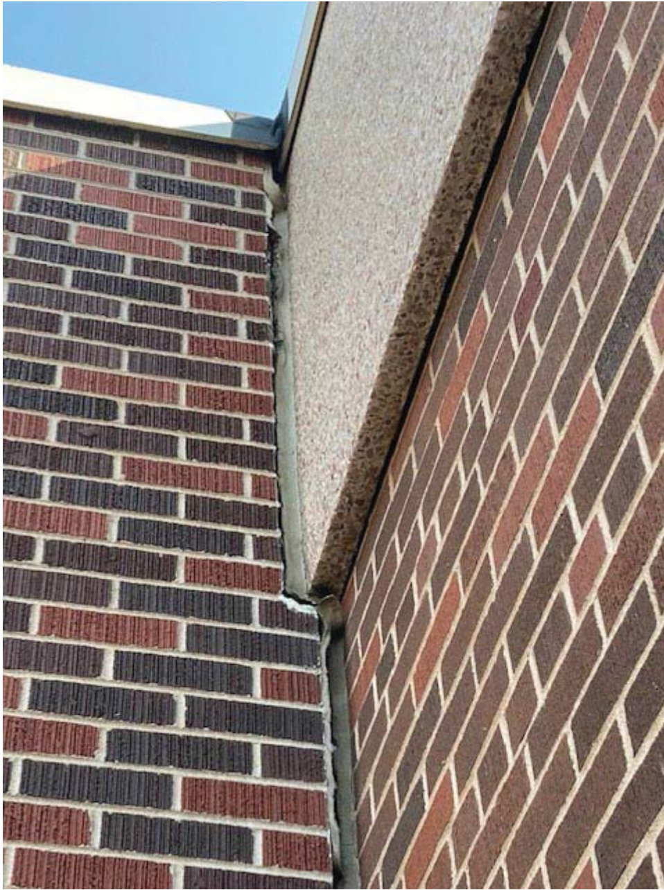
Building Control Joint Separation - Exterior
