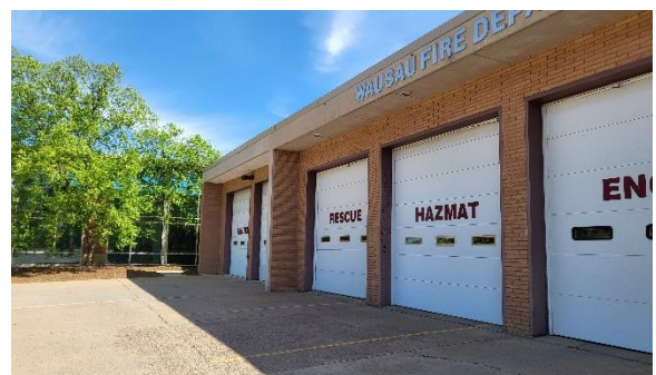
Figure 2-3: Front of Wausau Fire Station No. 01
