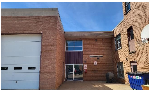
Figure 2-6: Rear entry to Wausau Fire Station No. 01
