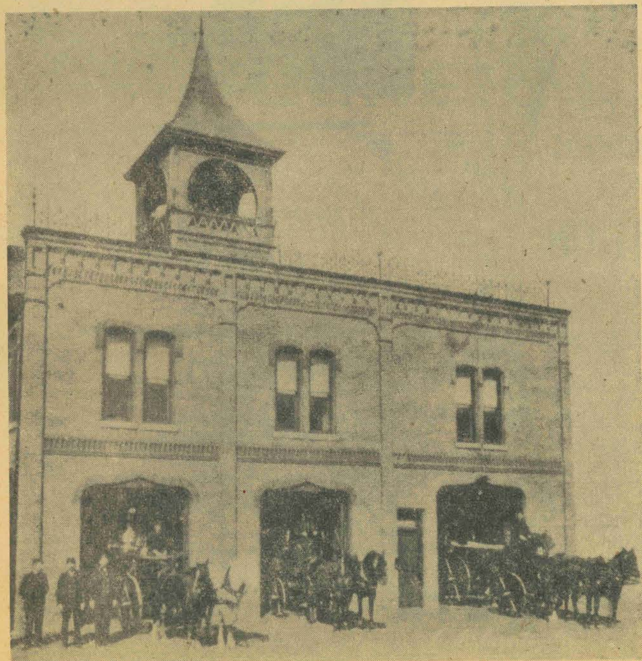
TIME DID LITTLE TO CHANGE FIRE STATION—Take away the horse-drawn fire wagons and the fire station above would look like a modern building. The station, recently abandoned, at
