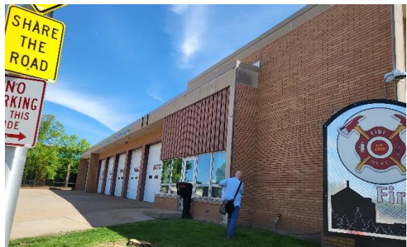
Figure 2-2: Front of Wausau Fire Station No. 01
