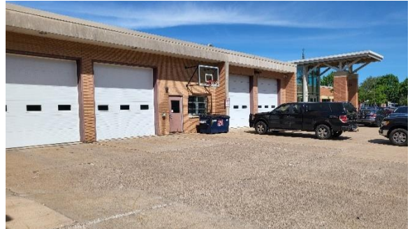
Figure 2-4: Rear of Wausau Fire Station No. 01
