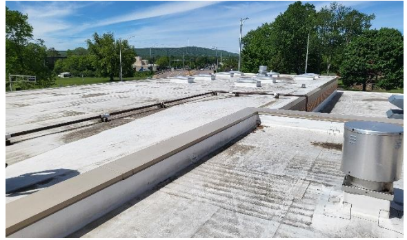
Figure 2-8: Roof of Wausau Fire Station No. 01
