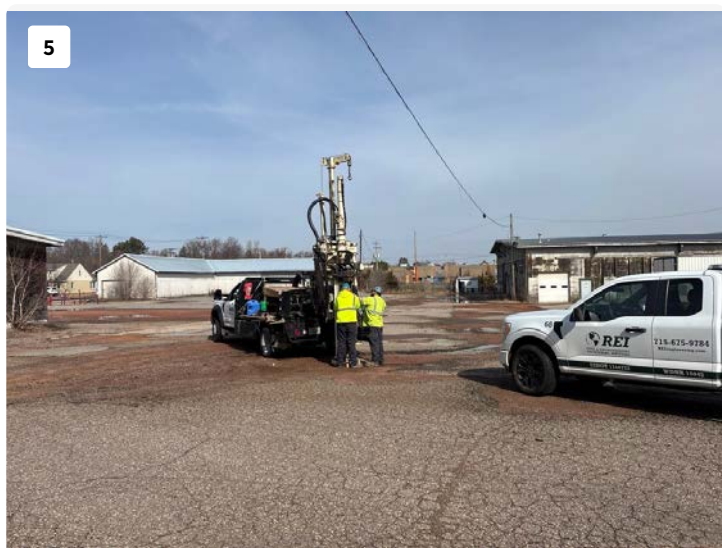
Geoprobe boring GP-5
