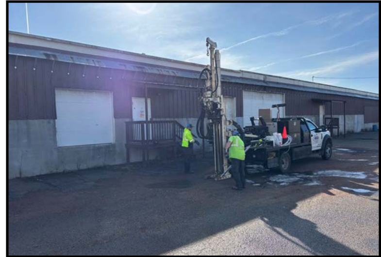
Soil boring GP-6 (03/10/2025)
