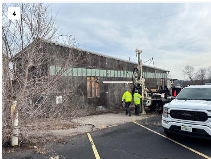
Geoprobe boring GP-4
