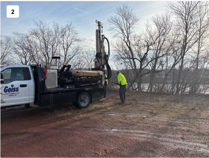
Geoprobe boring GP-2
