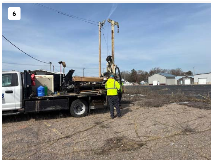
Geoprobe boring GP-6
