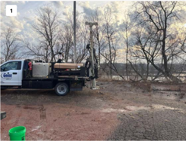
Geoprobe boring GP-1
