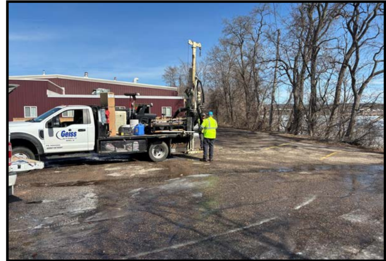
Soil boring GP-10 (03/10/2025)
