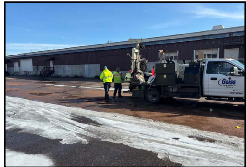
Soil boring GP-8 (03/10/2025)
