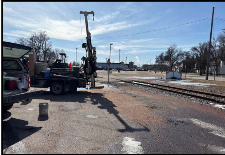
Soil boring GP-9 (03/10/2025)
