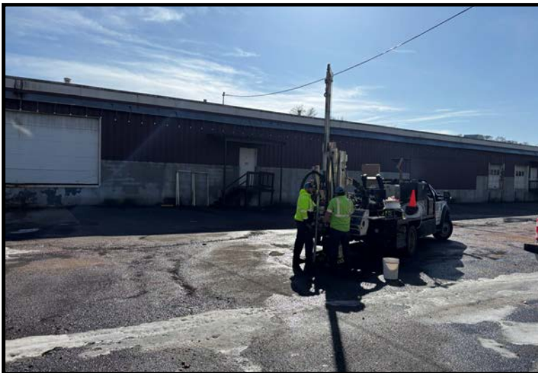
Soil boring GP-7 (03/10/2025)
