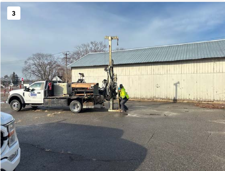
Geoprobe boring GP-3
