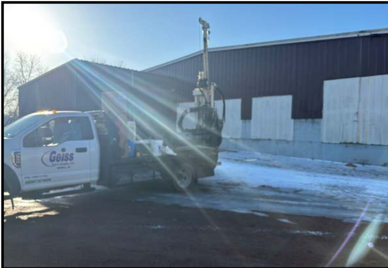
Soil boring GP-3 (03/10/2025)
