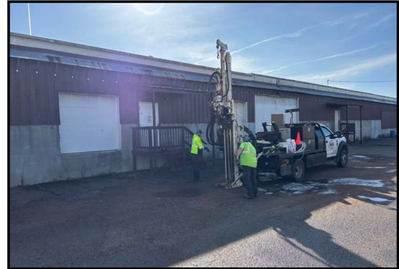
Soil boring GP-6 (03/10/2025)
