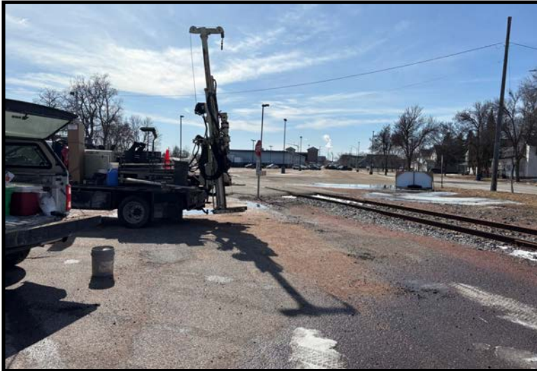
Soil boring GP-9 (03/10/2025)
