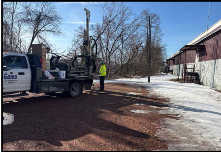
Soil boring GP-5 (03/10/2025)
