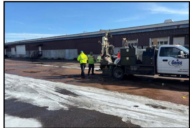
Soil boring GP-8 (03/10/2025)
