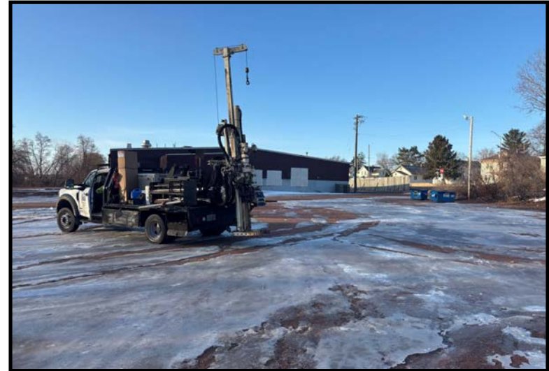
Soil boring GP-2 (03/10/2025)
