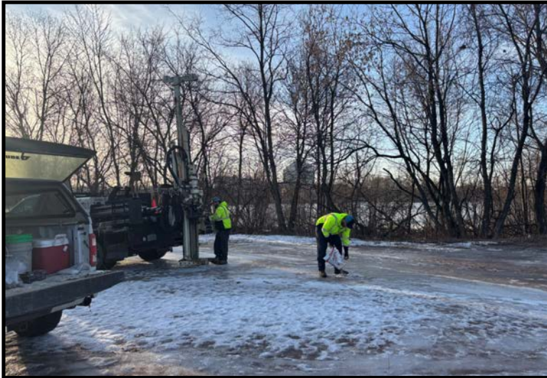
Soil boring GP-1 (03/10/2025)
