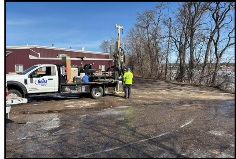
Soil boring GP-10 (03/10/2025)
