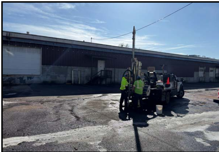
Soil boring GP-7 (03/10/2025)
