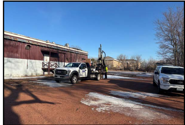
Soil boring GP-4 (03/10/2025)
