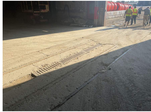
B. PREVIOUSLY REMOVED RAILROAD TRACKS THROUGH SITE
