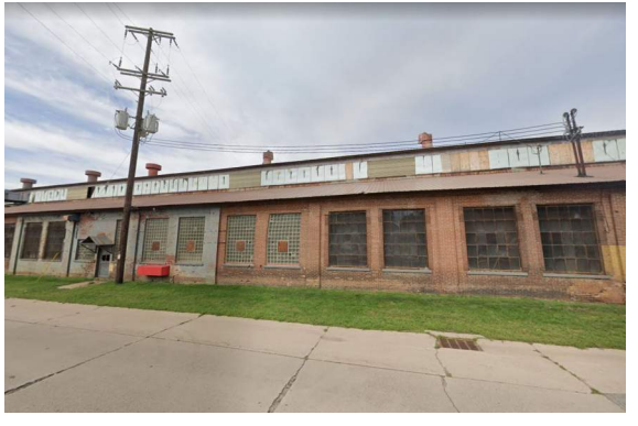
A. MAIN UTILITY LINE ENTRY TO SITE
