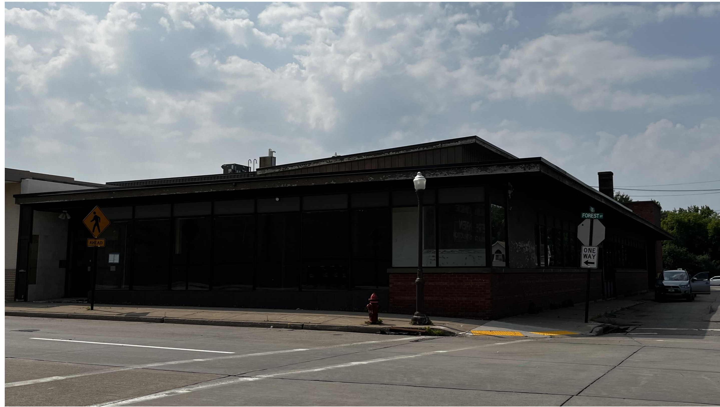
EXISTING VIEW FROM FOREST STREET
