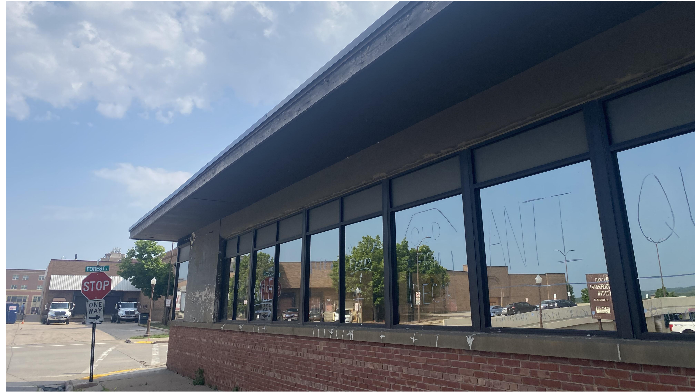
EXISTING VIEW FROM SECOND STREET
