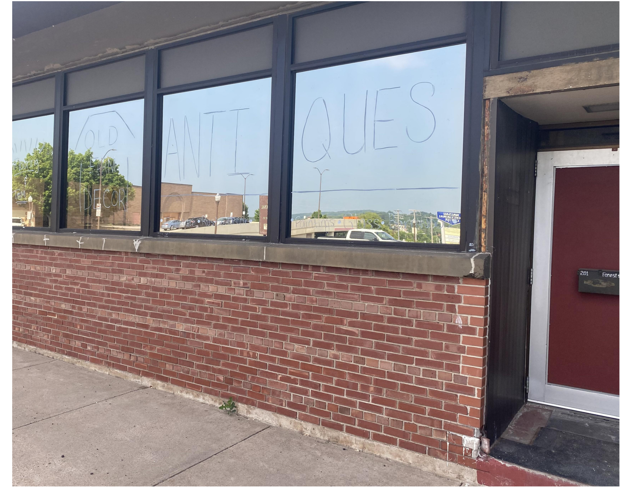
EXISTING VIEW FROM SECOND STREET
