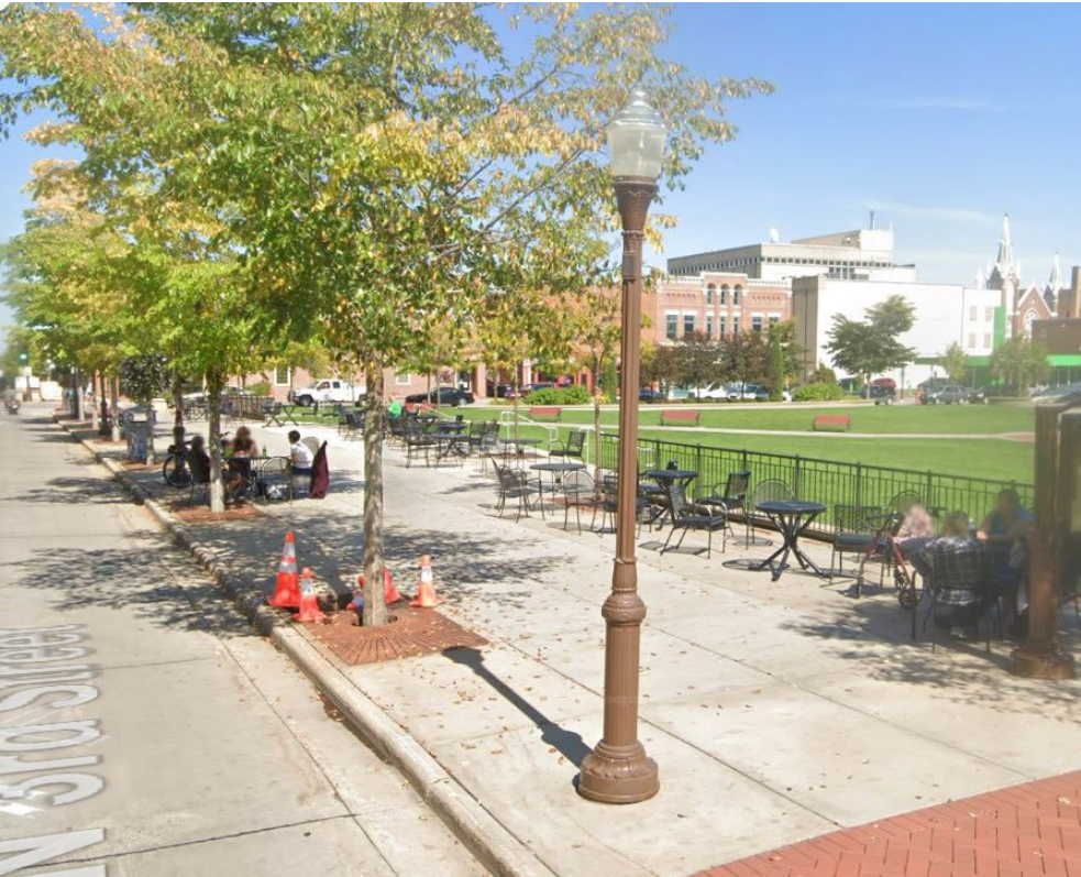
Existing Street Light Standard - converted to LED
