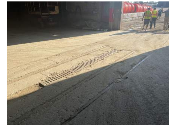
B. PREVIOUSLY REMOVED RAILROAD TRACKS THROUGH SITE
