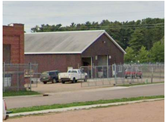
7. WAUSAU MOTORSPORTS BUILDING 5,500 SF
