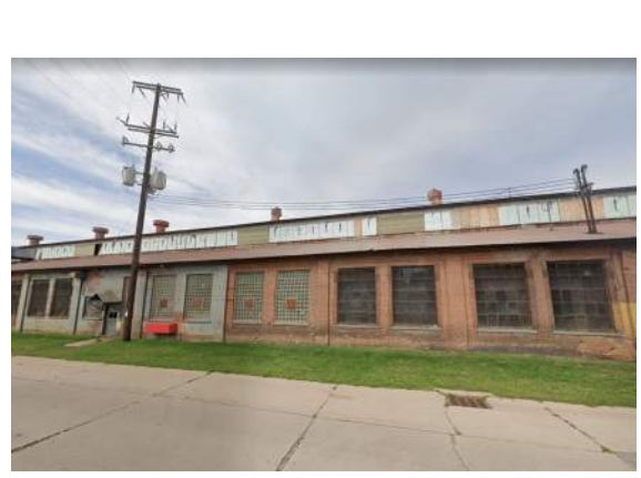
A. MAIN UTILITY LINE ENTRY TO SITE
