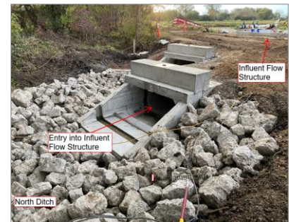
2020 construction – influent flow structure diverts upstream flows to basins.
