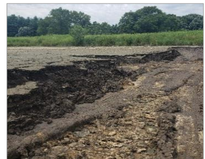
Curtis Pond dredging supported by NR 528 and NR 347-compliant sediment sampling and sediment disposal plan.
