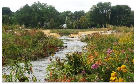
Natural channel replaced highly erodible stormwater ditch to protect downstream wetlands and Lake Wingra.
