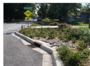
Rain garden and bump-out at bike path crossing.
