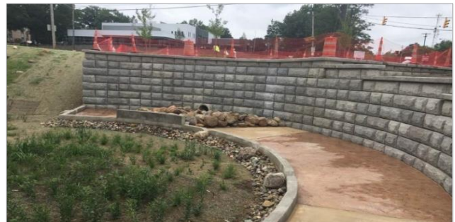
Fairhill/MLK: 19,700-square-foot bioretention basin serving 59-acre watershed with pretreatment, energy dissipation, and level spreading header.
