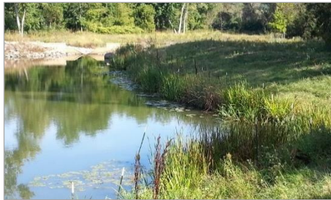
Secret Pond with irregular wetland edge and littoral shelf enhances nutrient removal.
