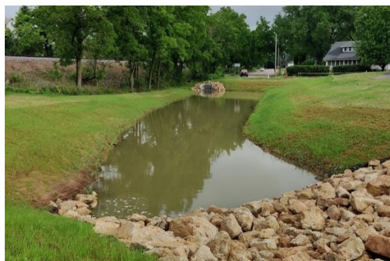
spillway/berm were restored with a turf reinforcement mat system. Native plant plugs were spaced one plug every 1-linear foot at 1-foot vertical above the normal water level of both detention basin cells in nonriprap areas.
