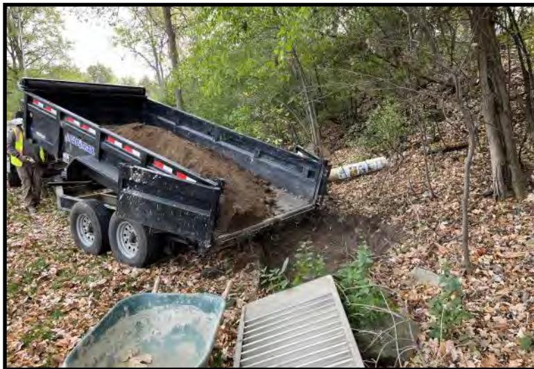
Backfilling soil excavation (10/12/2023)
