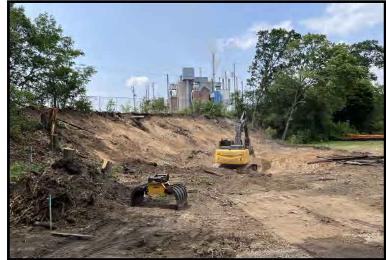
Ongoing soil excavation (7/18/2023)
