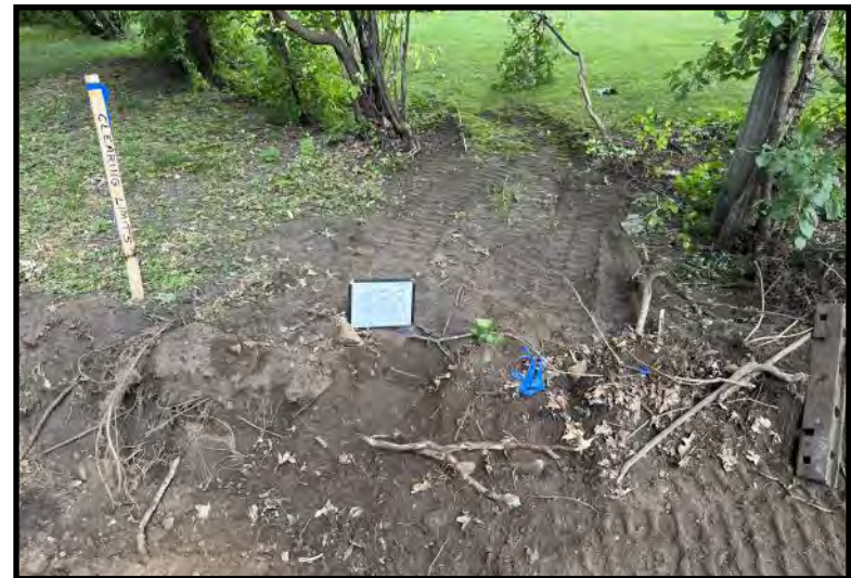
Excavation Sidewall Sample: S38 (7/19/2023)
