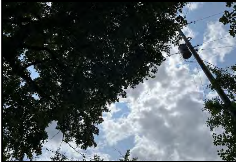
Site Preparations - Tree Contacting Overhead Utility Lines (7/6/2023)
