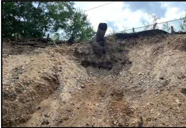
Excavation at culvert discharge (7/18/2023)
