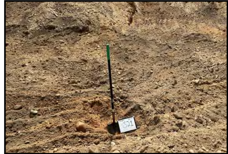
Excavation Base Soil Sample: S21 (7/18/2023)
