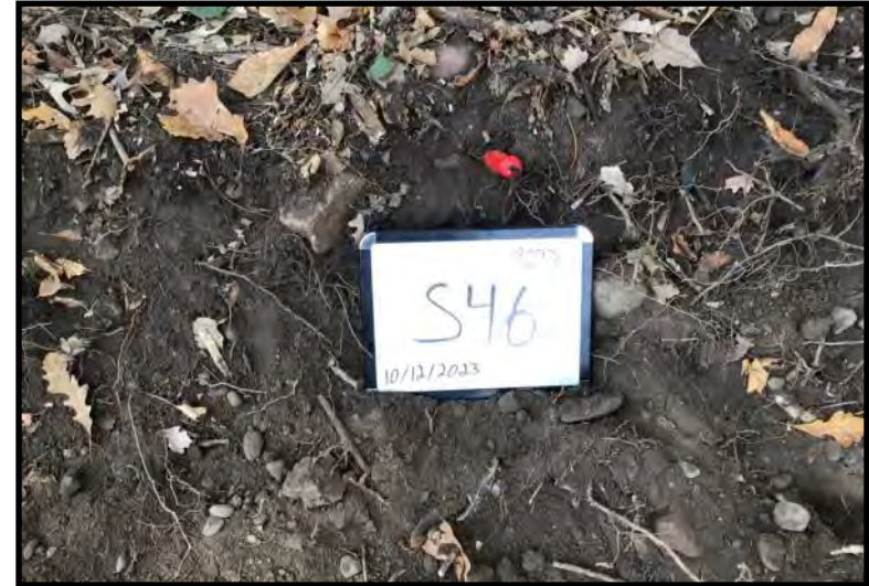
Excavation Sidewall Soil Sample: S46 (10/12/2023)
