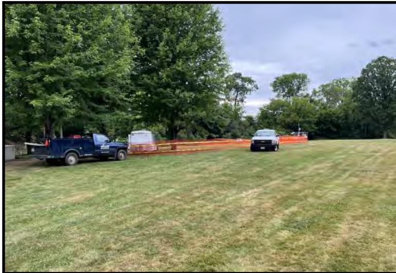
Site Preparations - Safety Fence Installation (7/5/2023)
