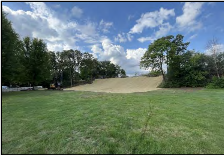
Site restoration: Seeded and erosion control mat installed (8/2/2023)
