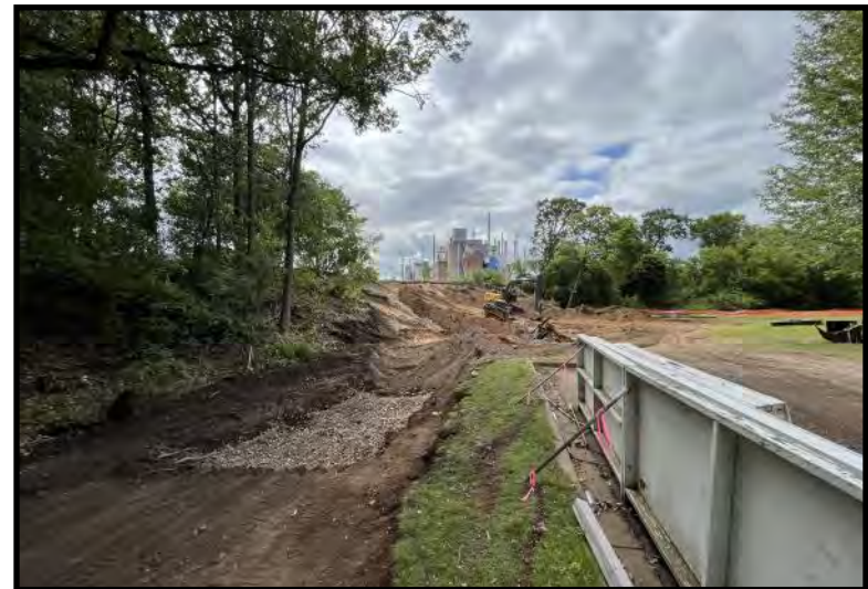
Ongoing soil excavation and backfilling (7/20/2023)
