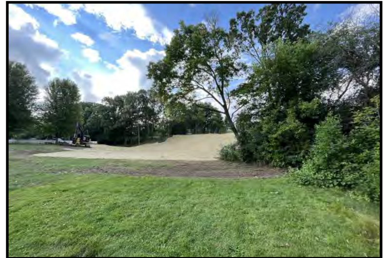
Site restoration: Seeded and erosion control mat installed (8/2/2023)
