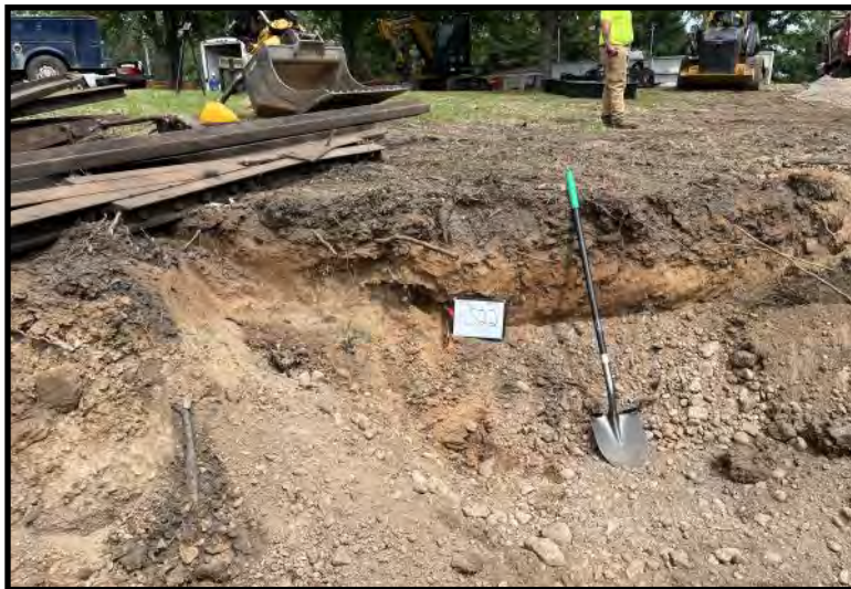
Excavation Sidewall & Base Soil Sample: S22 (7/18/2023)
