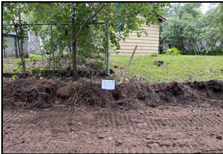
Excavation Sidewall Sample: S37 (7/19/2023)
