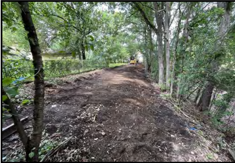
Ongoing soil excavation and backfilling (7/20/2023)
