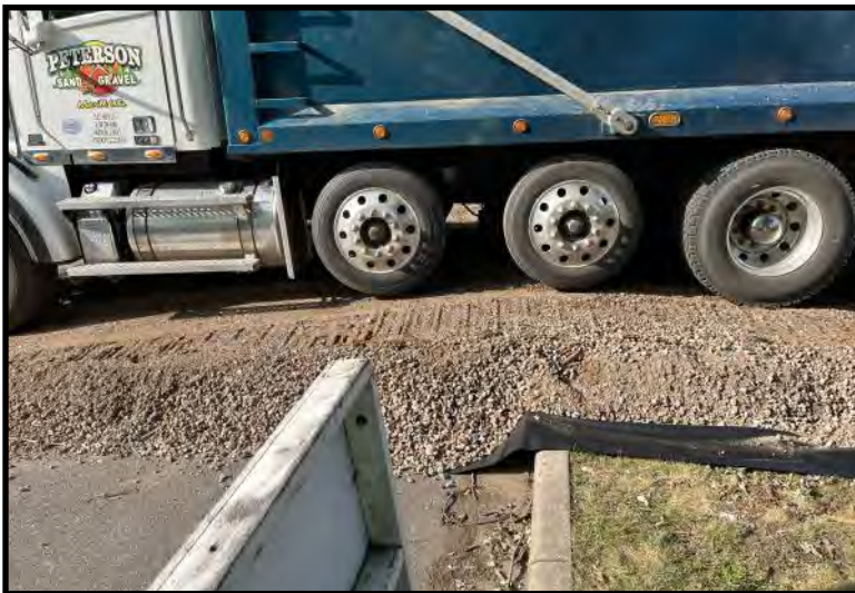
Gravel installed for protection of concrete curb (7/17/2023)
