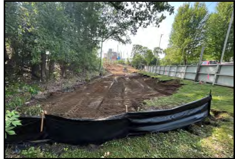
Ongoing backfilling of excavation (7/21/2023)
