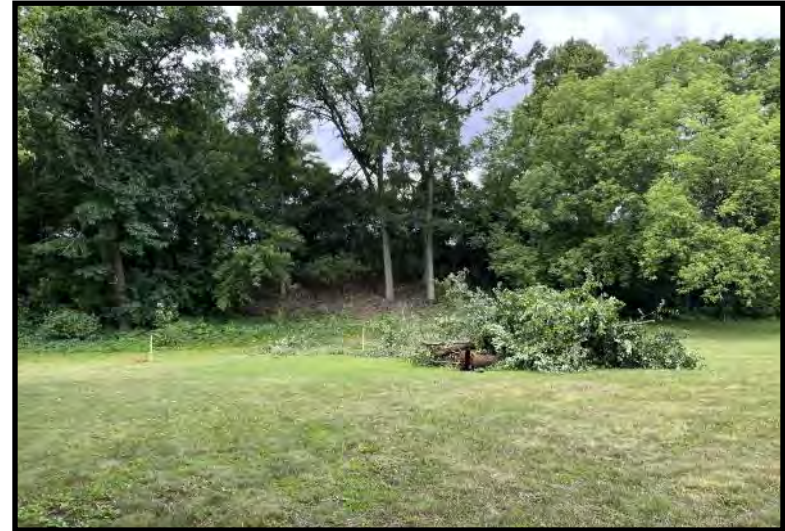
Site Preparations - Start of Vegetation Removal (7/5/2023)
