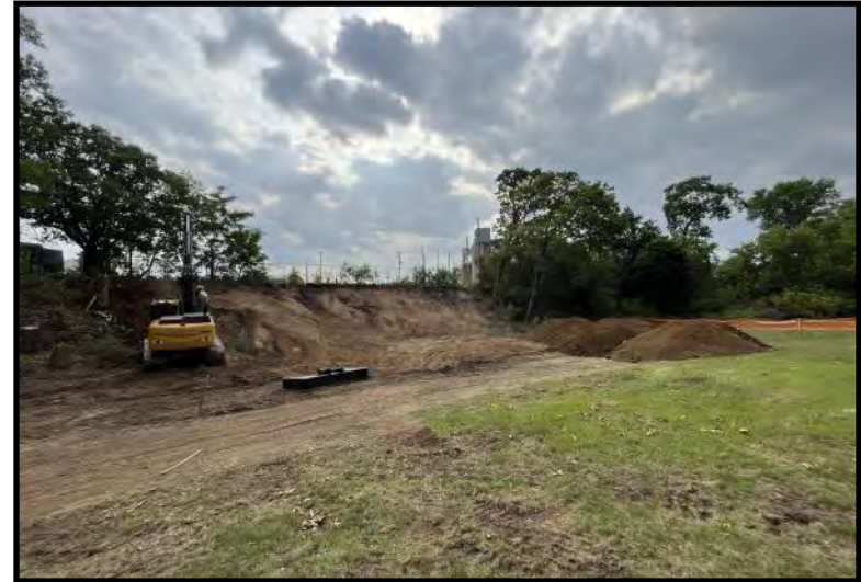
Ongoing soil excavation (7/18/2023)
