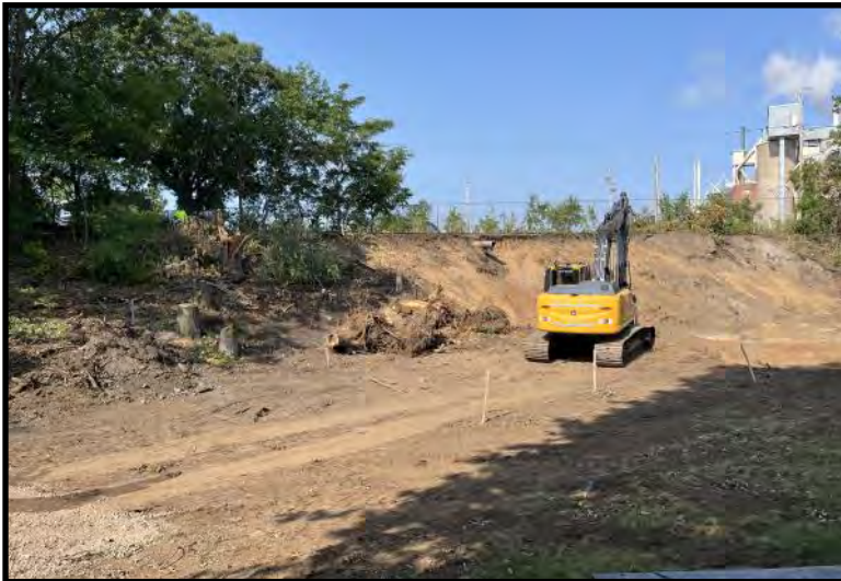
Ongoing Soil Excavation (7/18/2023)
