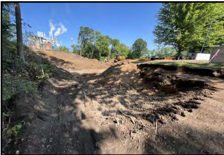
Ongoing soil excavation and backfilling (7/21/2023)
