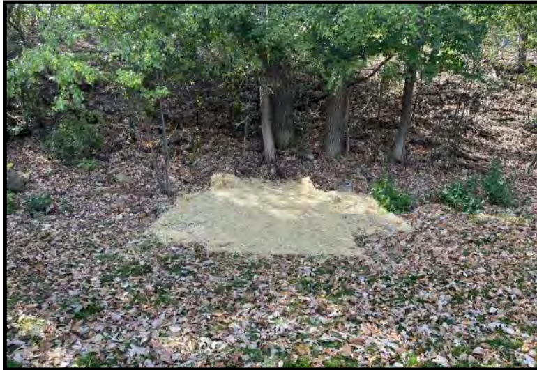
Excavation backfilled, seeded, and erosion control mat installed (10/12/2023)
