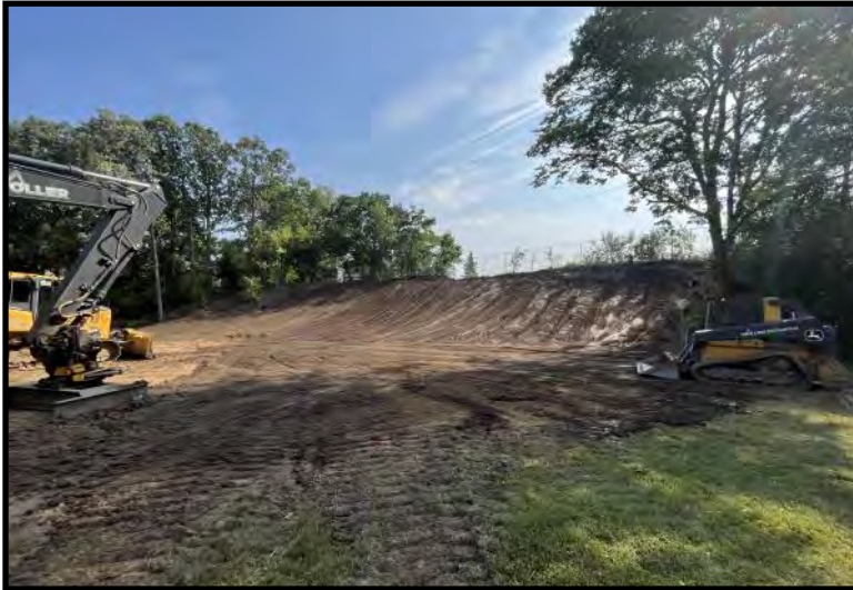
Ongoing backfilling of excavation (7/25/2023)
