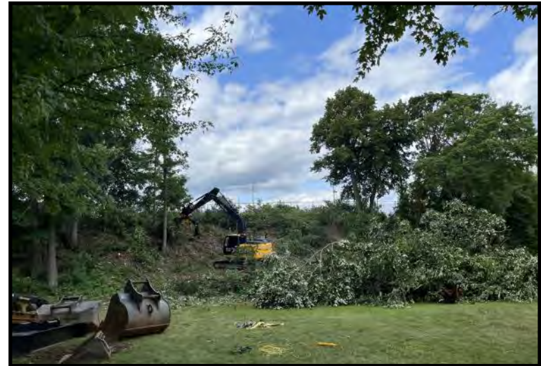
Site Preparations - Vegetation Removal (7/6/2023)
