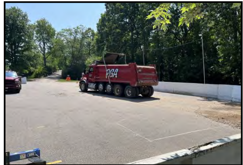
Last truck load departing excavation area (7/21/2023)
