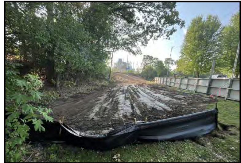
Ongoing backfilling of excavation (7/25/2023)
