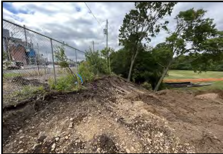
Ongoing soil excavation and backfilling (7/20/2023)
