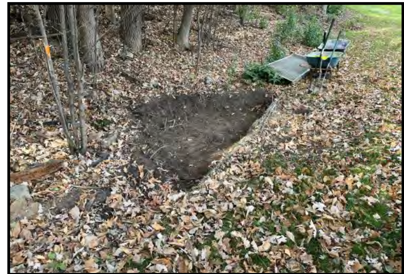
Limited soil excavation completed in area of soil sample S33 (10/12/2023)
