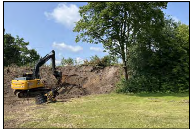
Start of soil excavation (7/17/2023)
