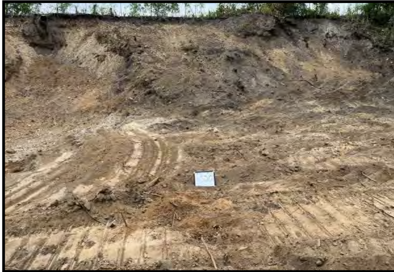
Excavation Base Soil Sample: S20 (7/18/2023)
