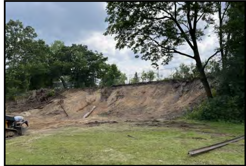
Culvert removed from the site (7/18/2023)
