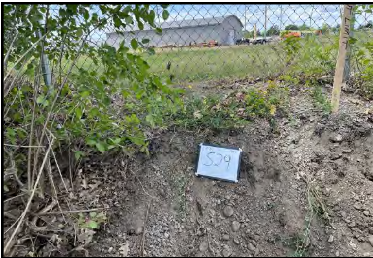
Excavation Sidewall Soil Sample: S29 (7/19/2023)
