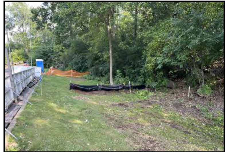
Site Preparations - Silt Fence Installation (7/13/2023)
