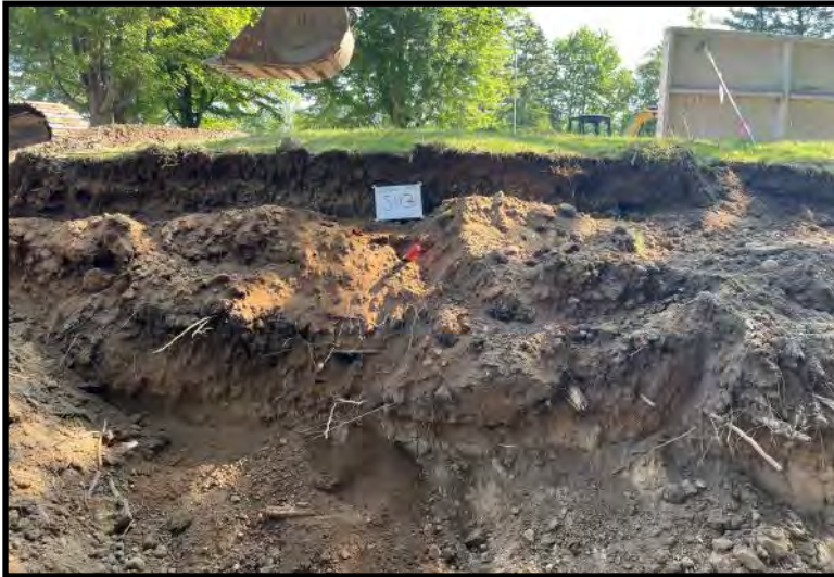
Excavation Sidewall & Base Soil Sample: S43 (7/21/2023)
