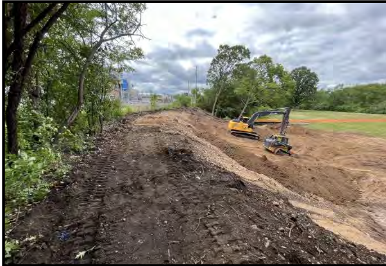
Ongoing soil excavation and backfilling (7/20/2023)
