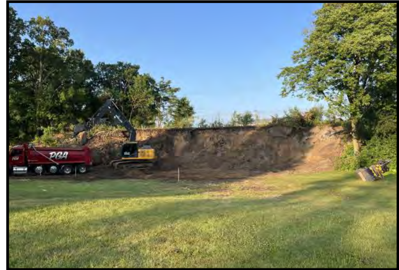
Ongoing Soil Excavation (7/18/2023)
