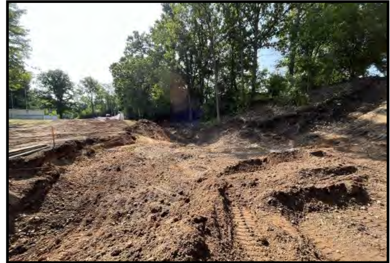
Ongoing soil excavation and backfilling (7/21/2023)
