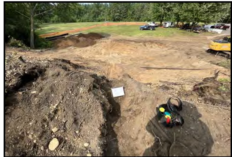
Excavation Base Soil Sample: S27 (7/18/2023)
