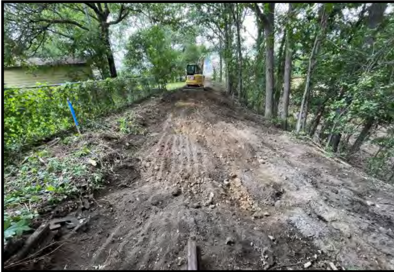
Excavation along removed railroad tracks (7/19/2023)
