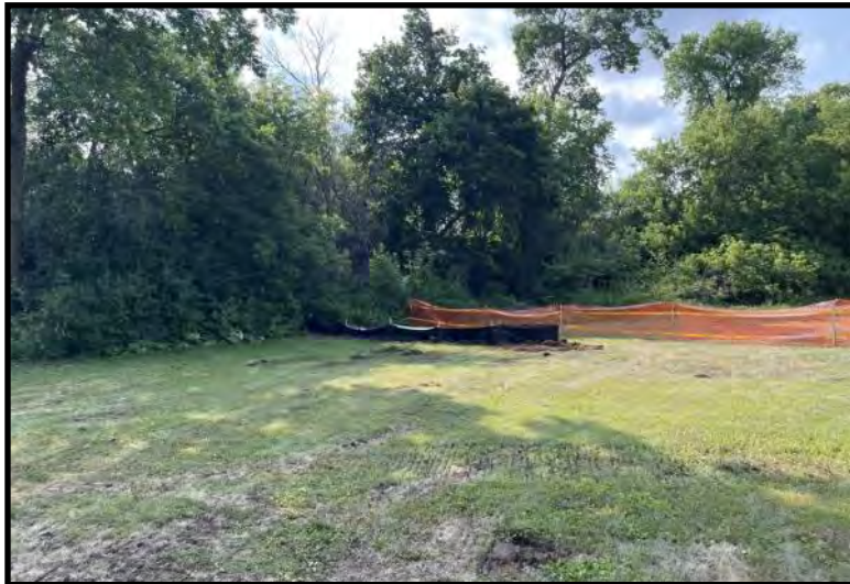
Site Preparations - Silt Fence Installation (7/13/2023)
