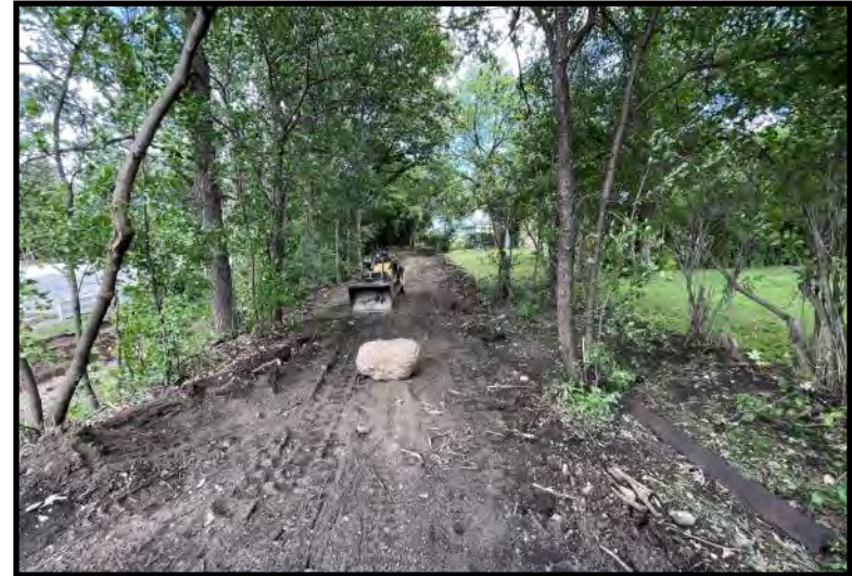
Ongoing soil excavation and backfilling (7/20/2023)
