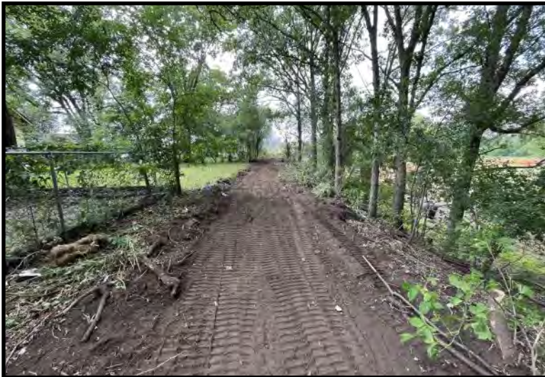
Former Railroad track after removal (7/18/2023)
