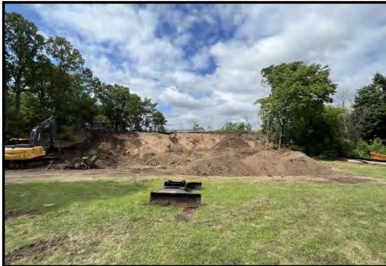
Ongoing soil excavation and backfilling (7/20/2023)
