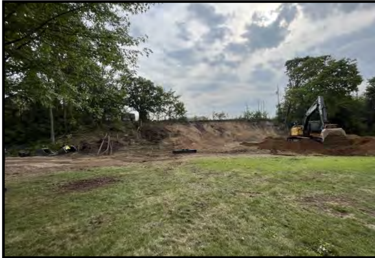
Installation of borrow material on completed northern portion of excavation (7/18/2023)
