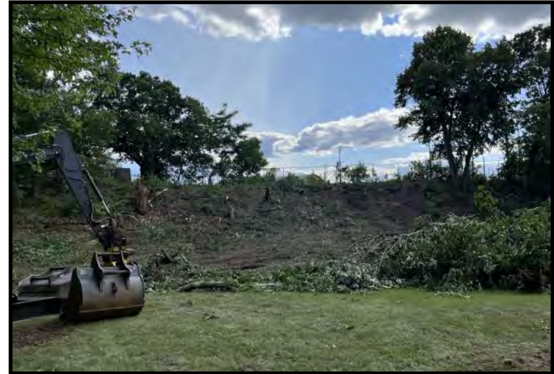
Site Preparations - Vegetation Removal (7/6/2023)
