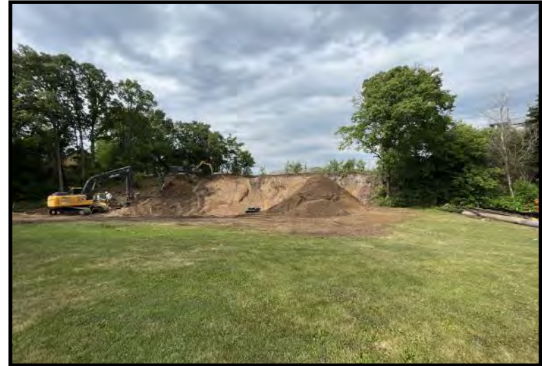
Ongoing soil excavation (7/19/2023)
