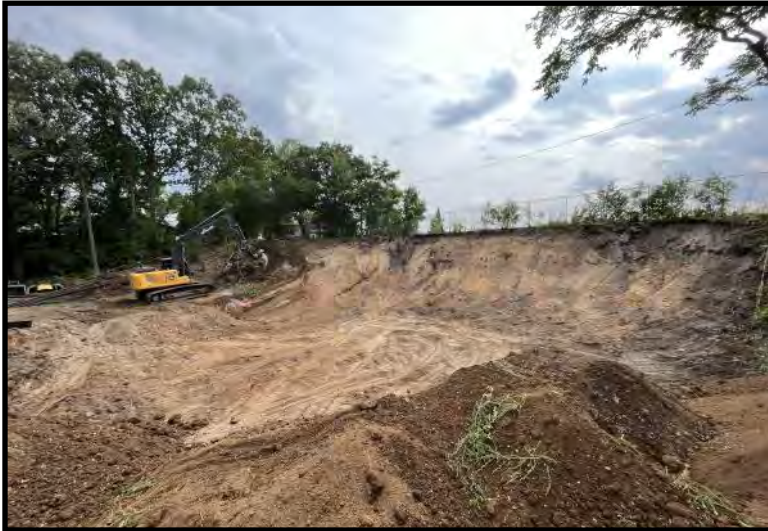
Ongoing soil excavation (7/18/2023)
