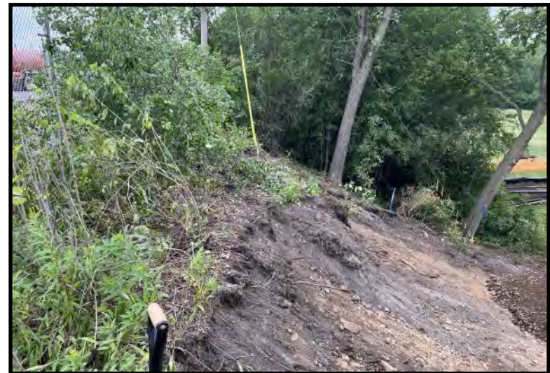
Excavation limited due to guide wire for utility pole (7/19/2023)
