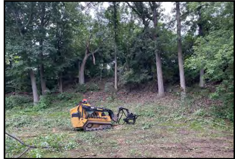
Site Preparations - Vegetation Removal (7/5/2023)
