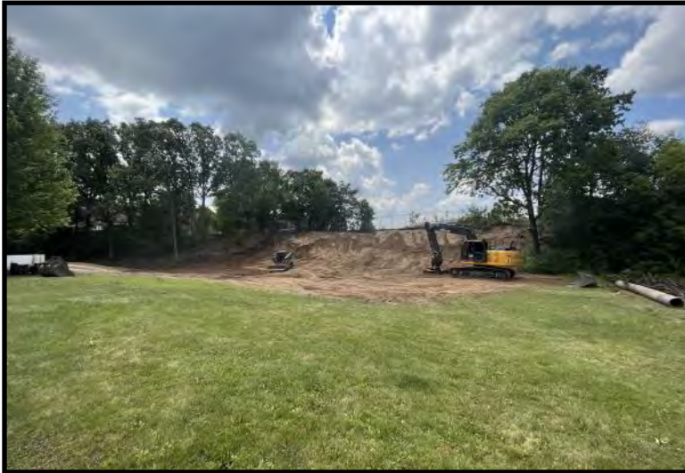
Ongoing backfilling of excavation (7/21/2023)
