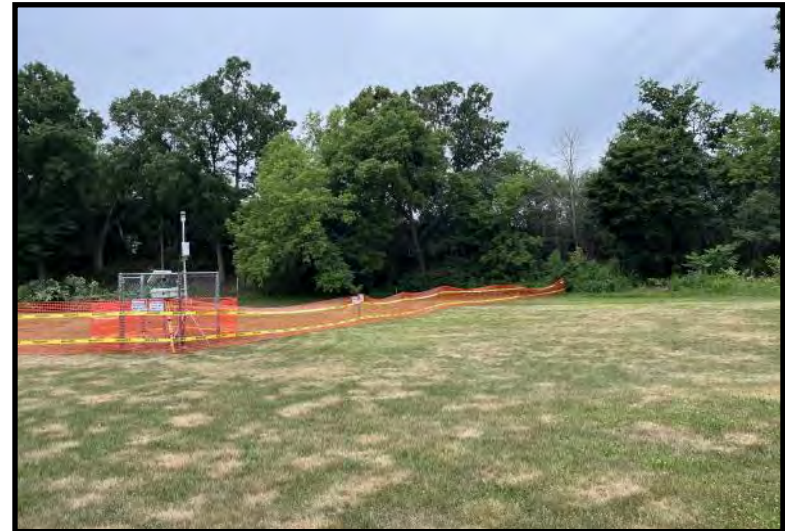
Site Preparations - Safety Fence Installation (7/5/2023)
