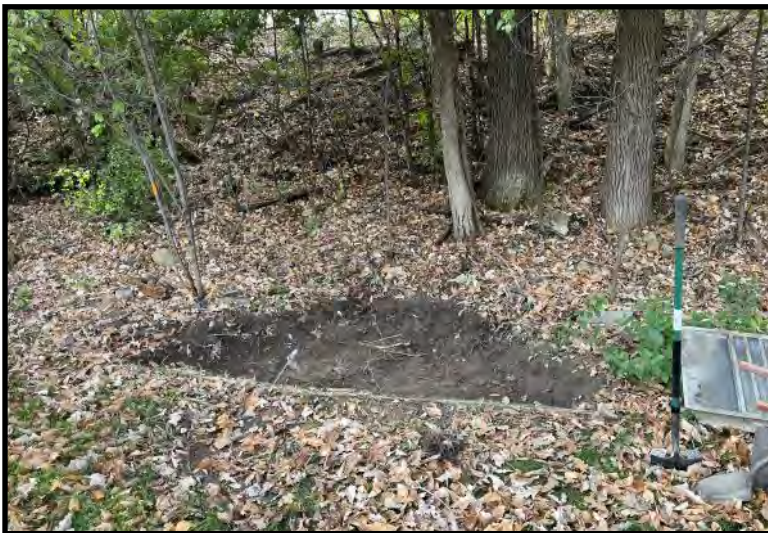
Limited soil excavation completed in area of soil sample S33 (10/12/2023)
