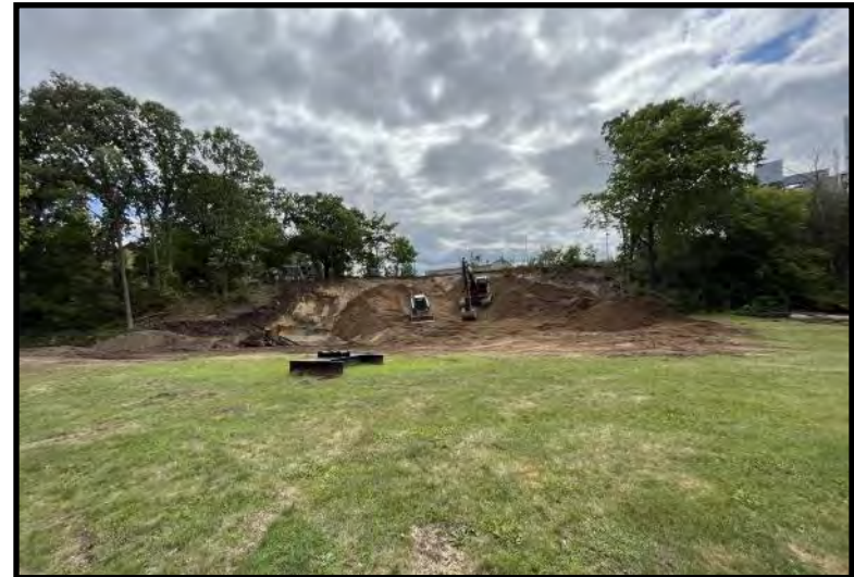
Ongoing soil excavation and backfilling (7/20/2023)
