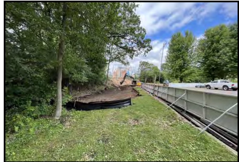
Ongoing soil excavation and backfilling (7/20/2023)
