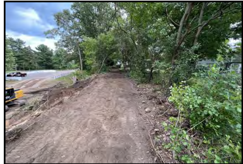
Former Railroad track after removal (7/18/2023)
