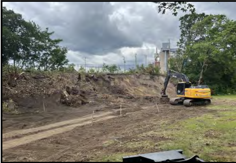
Ongoing Soil Excavation (7/17/2023)
