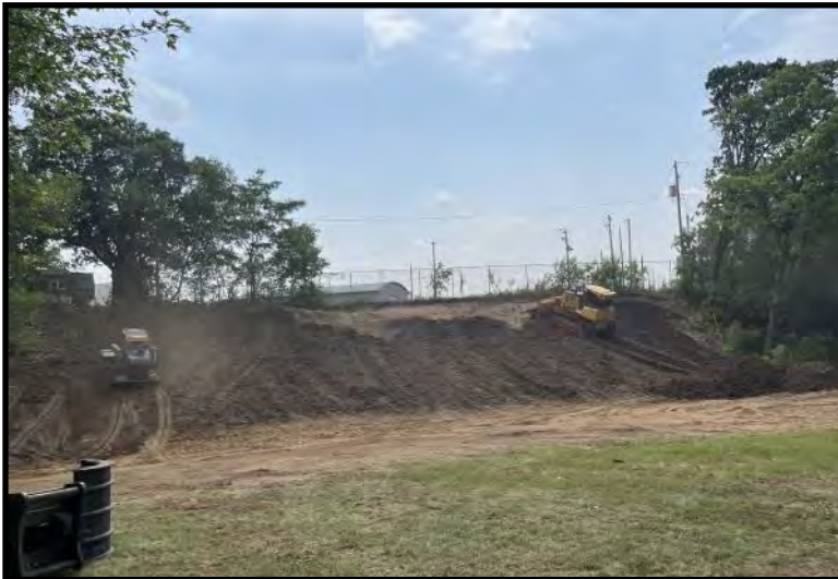
Ongoing backfilling of excavation (7/25/2023)
