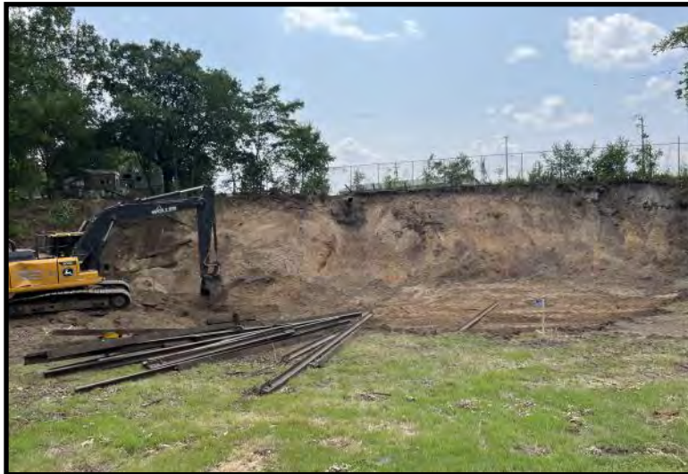
Removed railroad track (7/18/2023)
