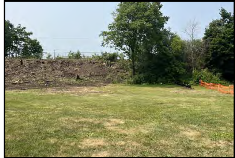
Site Preparations - Vegetation Removal (7/14/2023)
