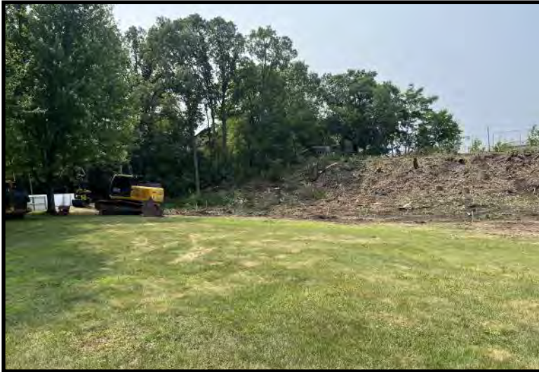
Site Preparations - Vegetation Removal (7/14/2023)
