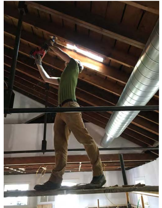
Nick Carnahan cutting skylights in GCA office roof.
