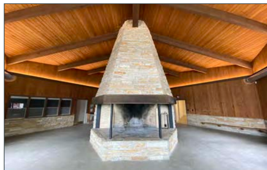
Regrading existing fireplace
