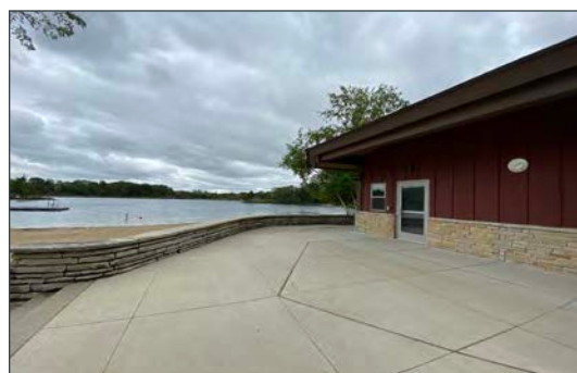
Exterior work repaired a damaged roof edge and patio area
