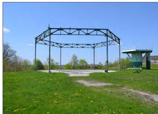
Remaining support structures for radar antennas
