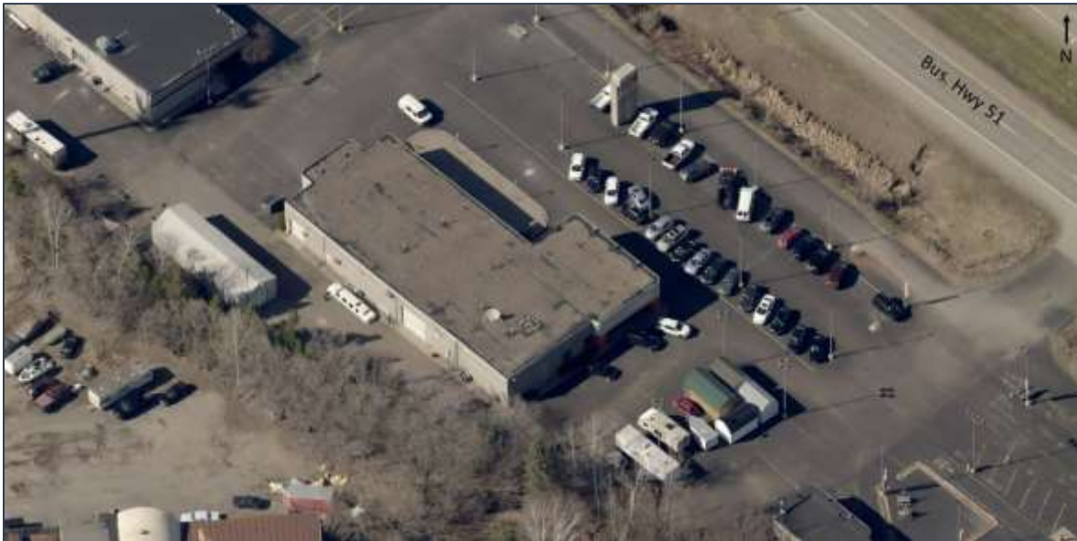
Image 1. Aerial view of subject property
