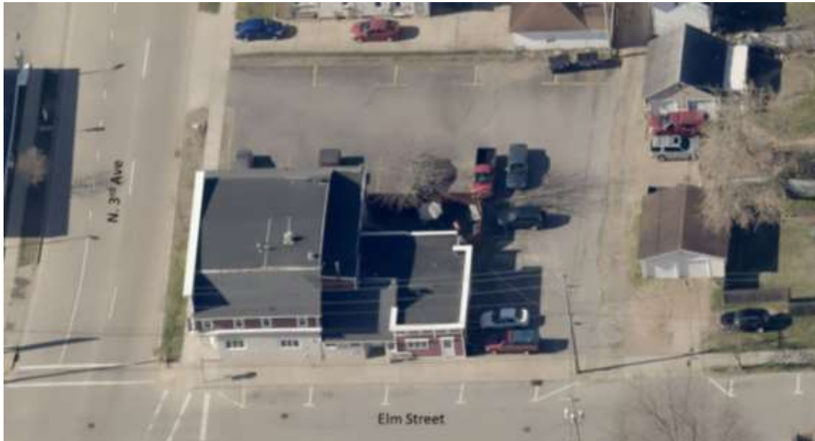
Image 1. Aerial view of subject property
