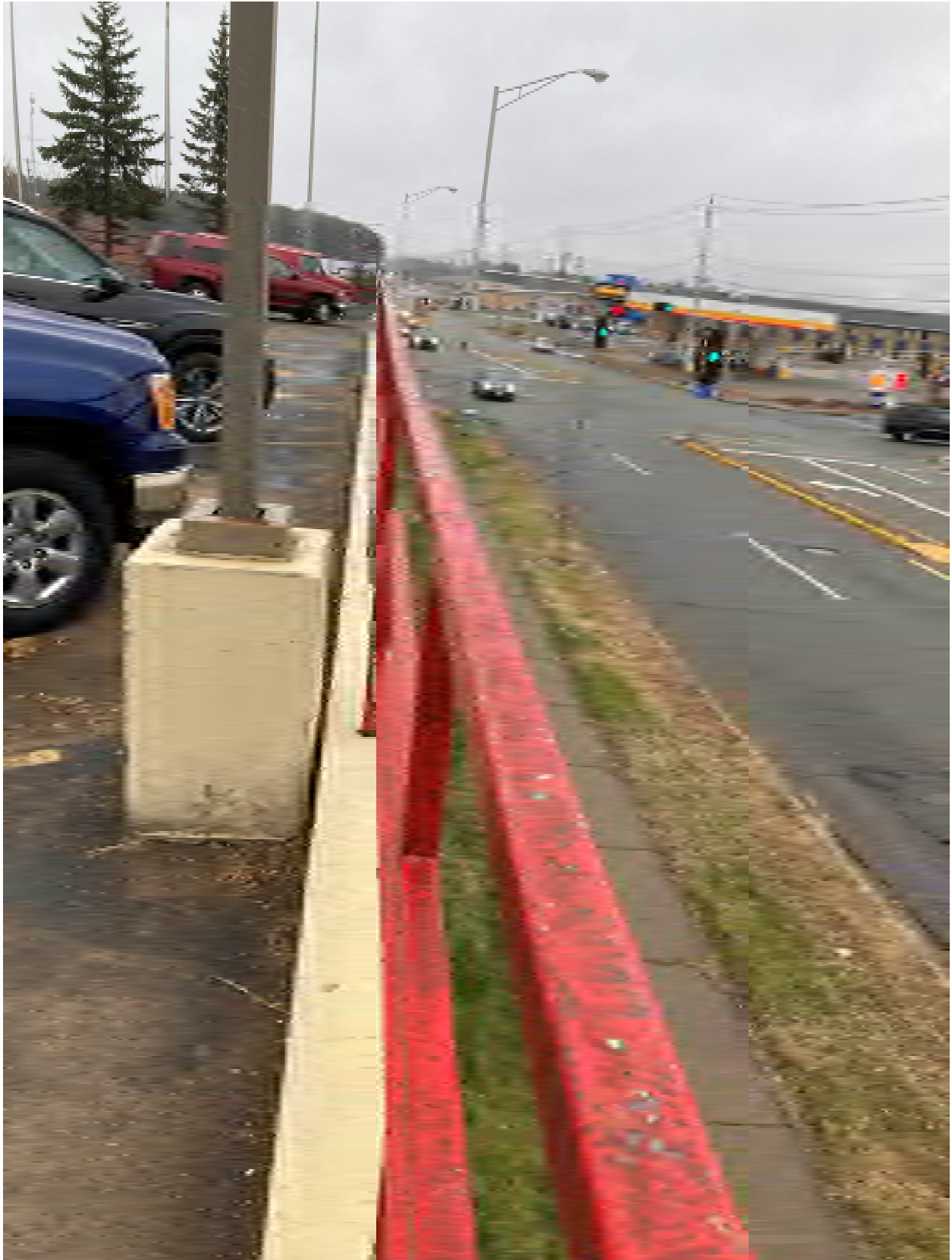
View looking South along existing West Property Line showing previous development with parking lined up to existing railing at property line.
