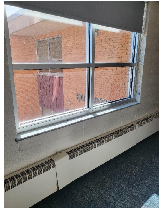
Figure 3-12: Women's Locker Room
