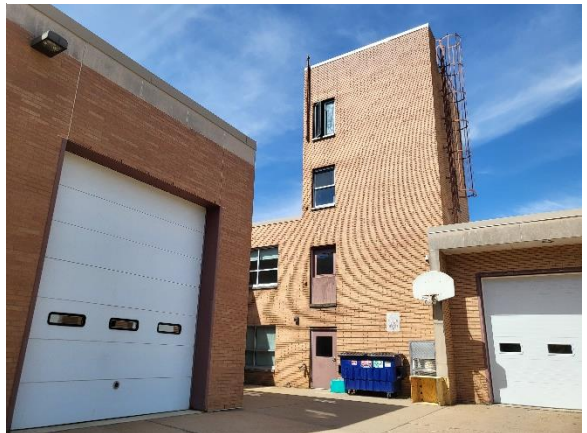
Figure 2-5: Training tower & Maintenance Garage
