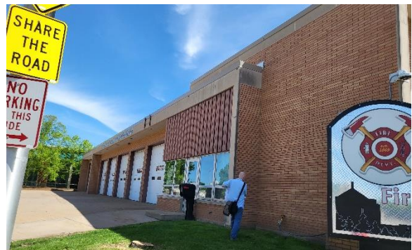
Figure 2-2: Front of Wausau Fire Station No. 01
