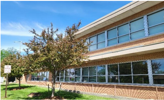
Figure 2-7: South of Wausau Fire Station No. 01
