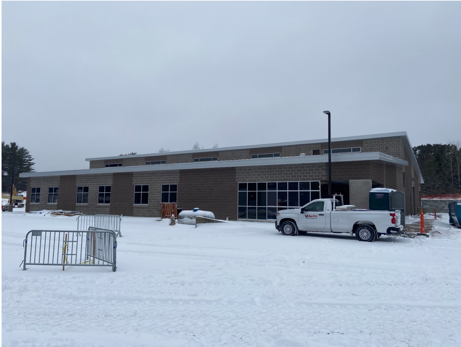
Admin. Bldg. – Soffit and Fascia Installation
