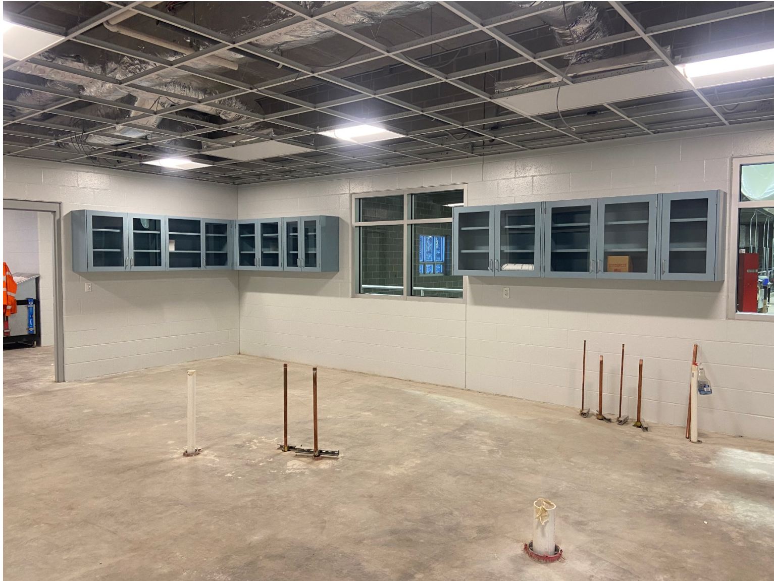
Process Bldg. – Laboratory Cabinet Installation
