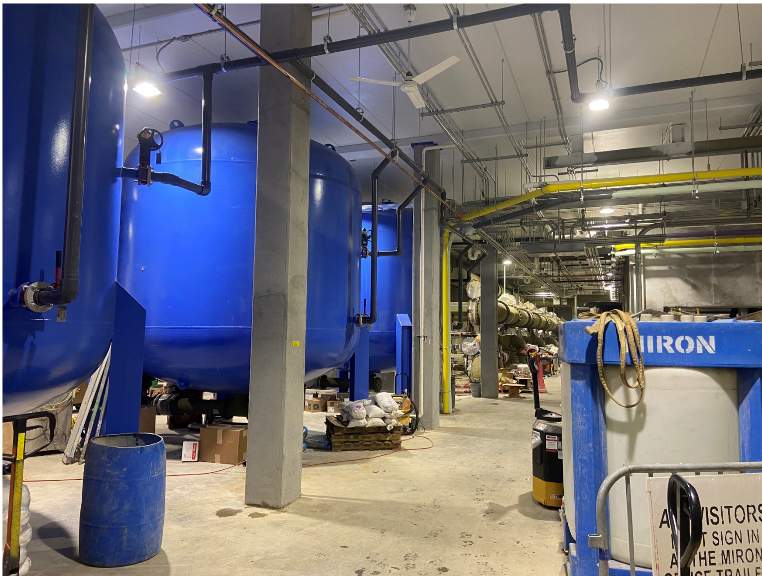
Process Bldg. – Anion Exchange Tanks Where Media Installation into the Tanks Have Begun
