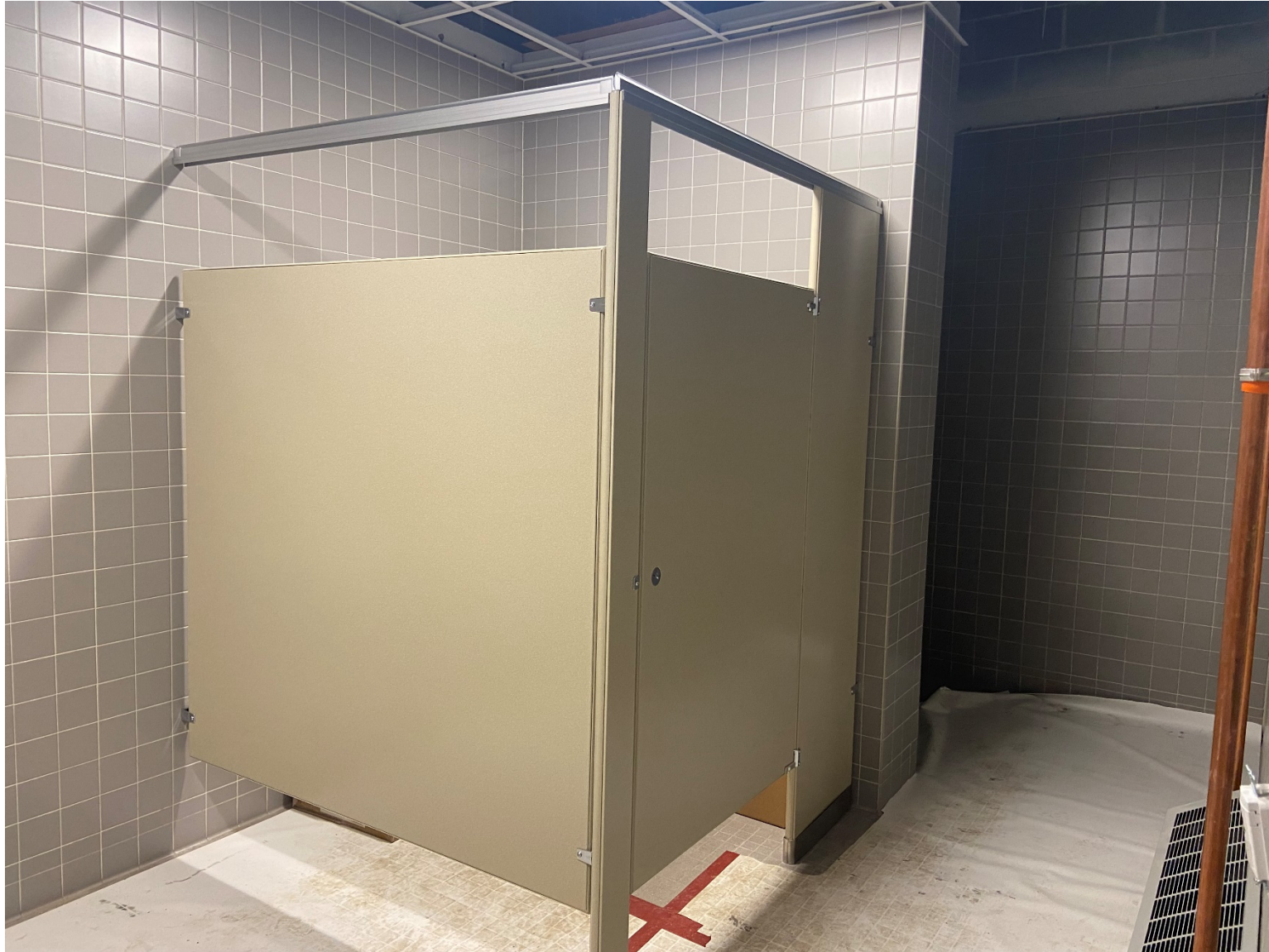
Process Bldg. – Grade Level Bathroom Tile and Toilet Partition Installation
