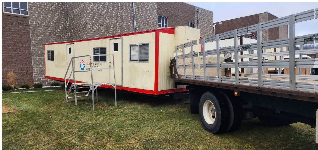
Job Trailers beginning to be removed from site
