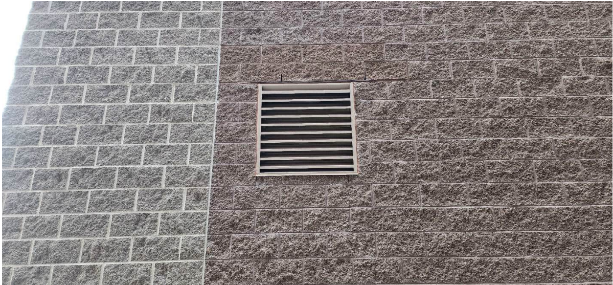
Existing louvre reinstalled and caulked on the northside of Structure 100 (Process Building).
