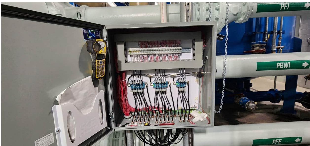
Econ completed the trimming of excess spare wiring in Structure 120 PFAS Vessel Air Valve Control Panels
