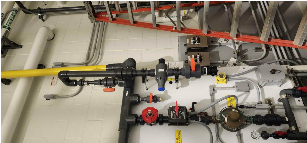
August Winters completed new sodium hydroxide (NaOH) solution chemical pump connection in Structure 100 (Process Building) Brine Room.
