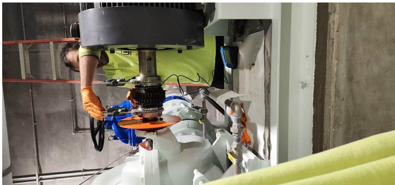
William Reed onsite to complete Structure 100 FW Pump 0911 motor and pump alignment prior to pump start up
