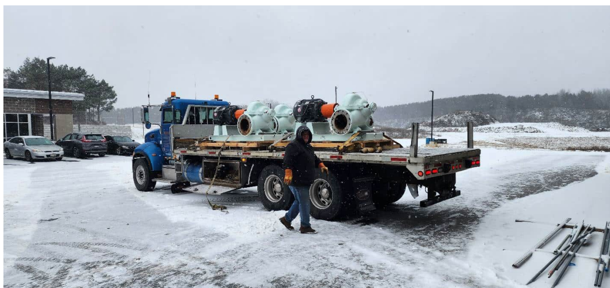
Old smaller Structure 100 (Process Building) Filtered Water Pumps being removed from site
