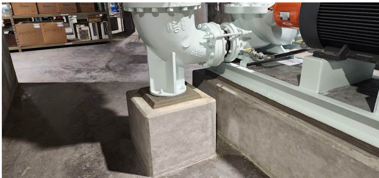
Ellis completed the grouting of the Structure 100 (Process Building) Filtered Water Pump 0911 and discharge pipe elbow.
