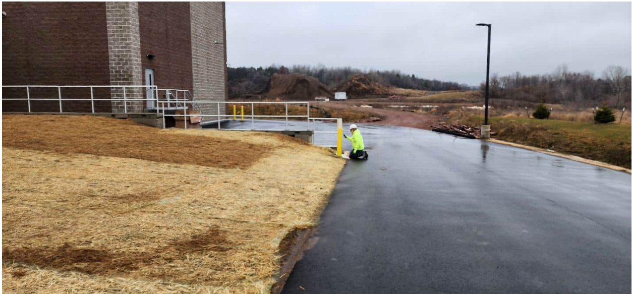
Howard Grote personnel painting new pipe bollard on east side of Structure 100 placed for protecting landscape wall and drain
