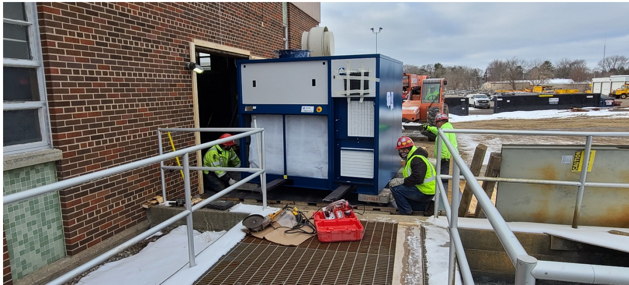
First new blower, being brought into Structure 400 (Activated Sludge Building). Existing north doorway removed to allow for blower entry.
