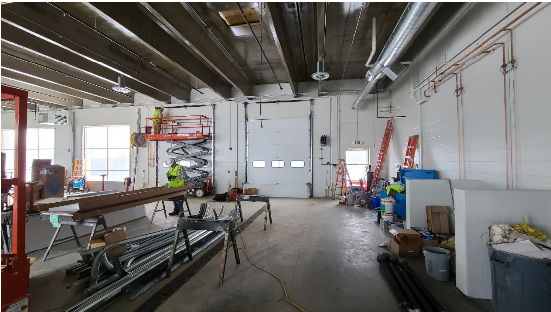
Garage area of Structure 120 (Administration Building): garage doors being installed, lighting and all other mechanical, electrical and plumbing work ongoing.
