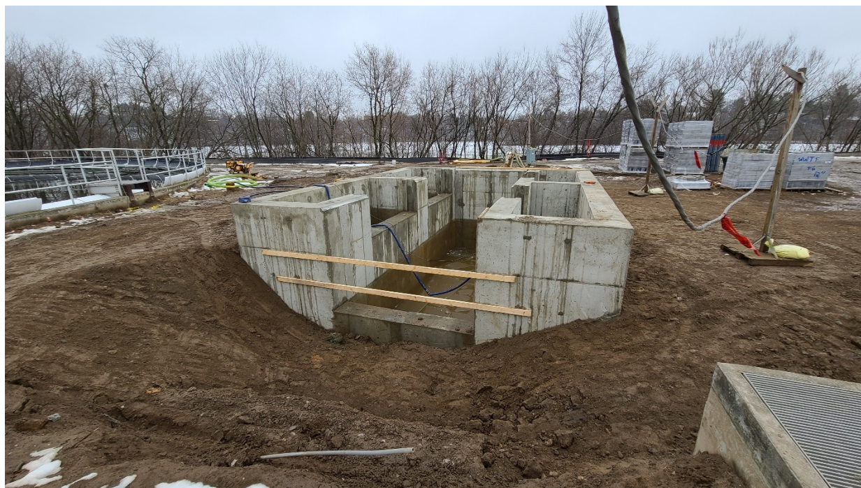
Structure 500 (Secondary Splitter): looking at the west side future connection point to the aeration basin effluent channel.
