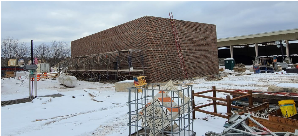
Miron has completed face brick of Structure 610 (Chemical Building)
