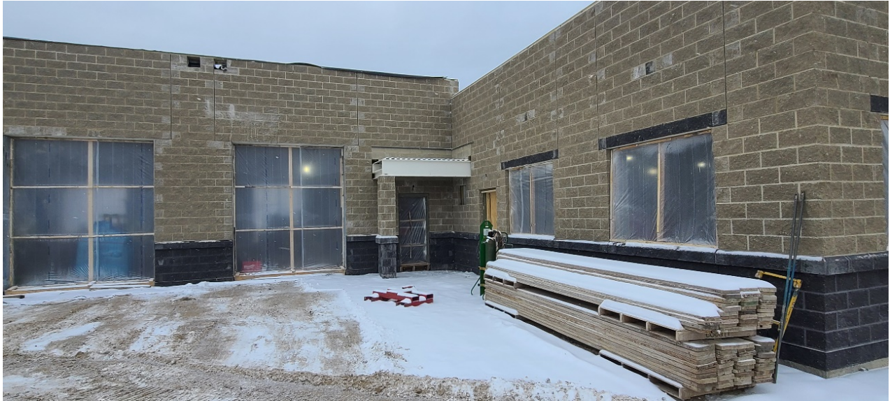
Exterior of Structure 120 (Administration Building) looking at the entryway between the garage and administration areas.
