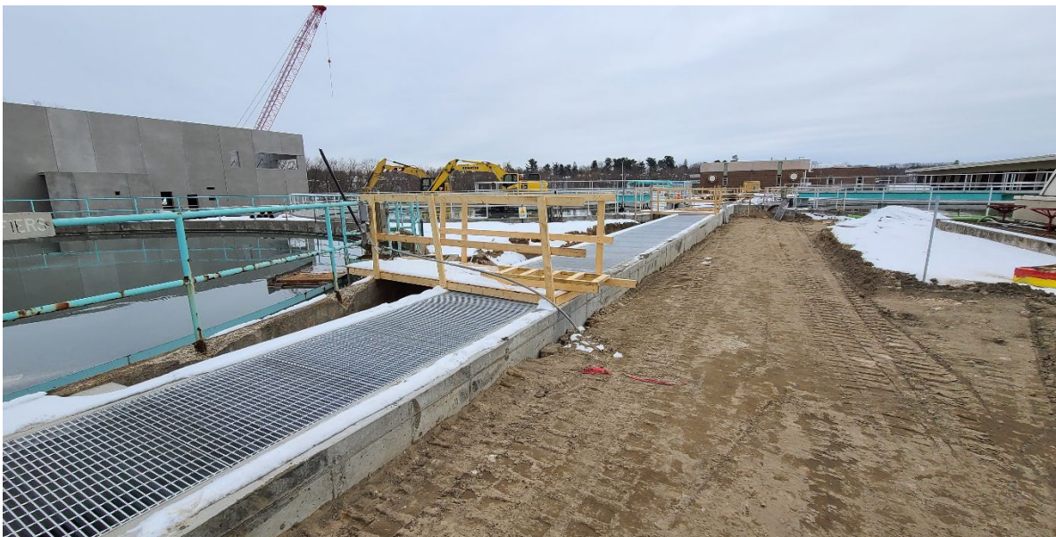
Structure 350 (Primary Effluent Channel) grating installation and backfill west side of channel.
