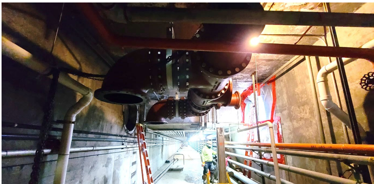
August Winters installation of new 20" RAS piping at south end of Tunnel 900.
