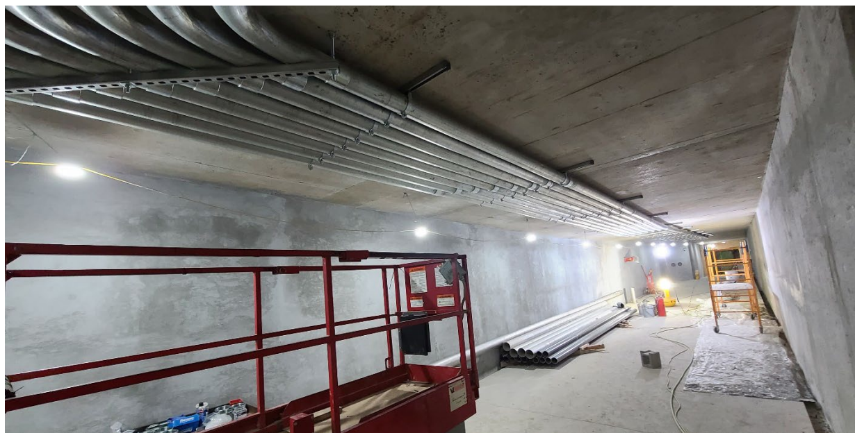
Van Ert Electric running 4-inch conduit along the ceiling of Tunnel 910.
