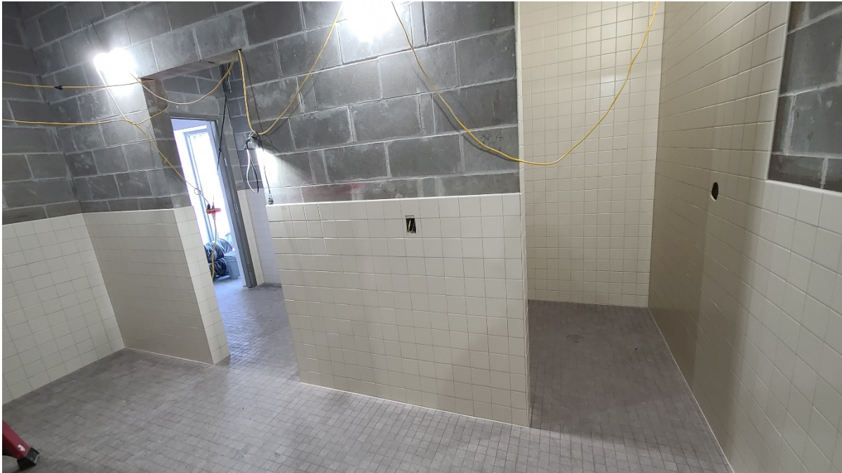
Tile work in Women's Locker Room of Structure 120 (Administration Building)
