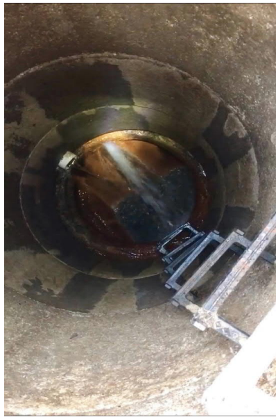
Joints, Steps, Service Connections in Manholes
