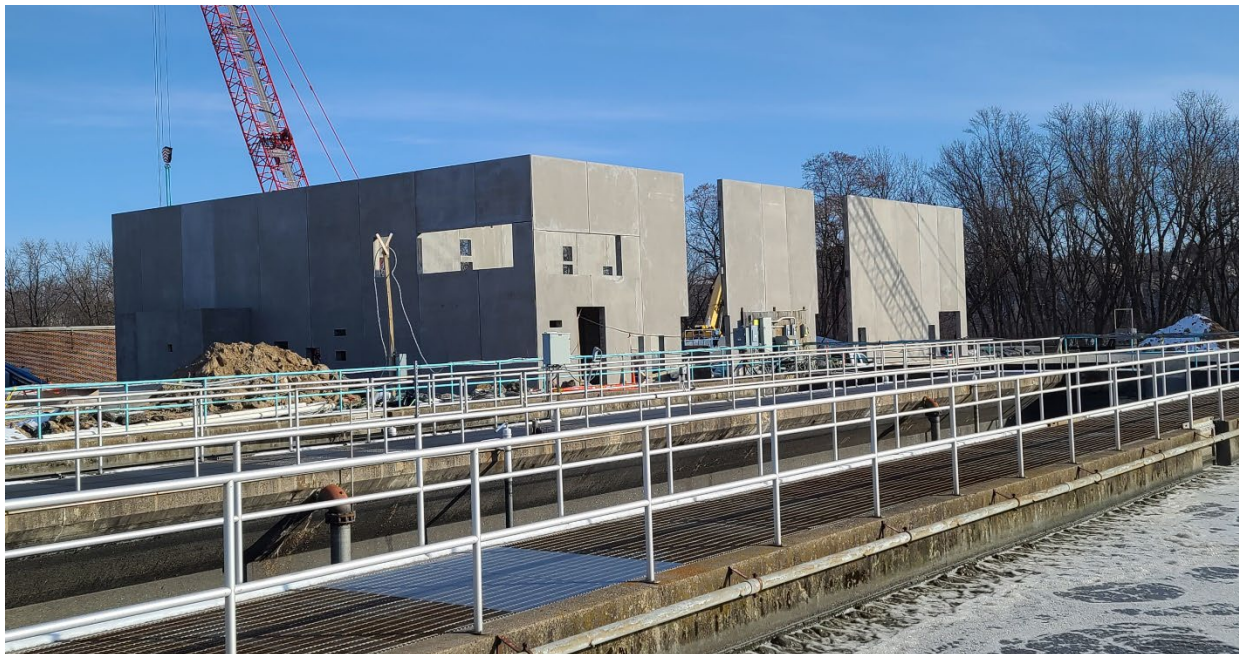
Structure 770 (Solids Building) precast walls were set by end of January.
