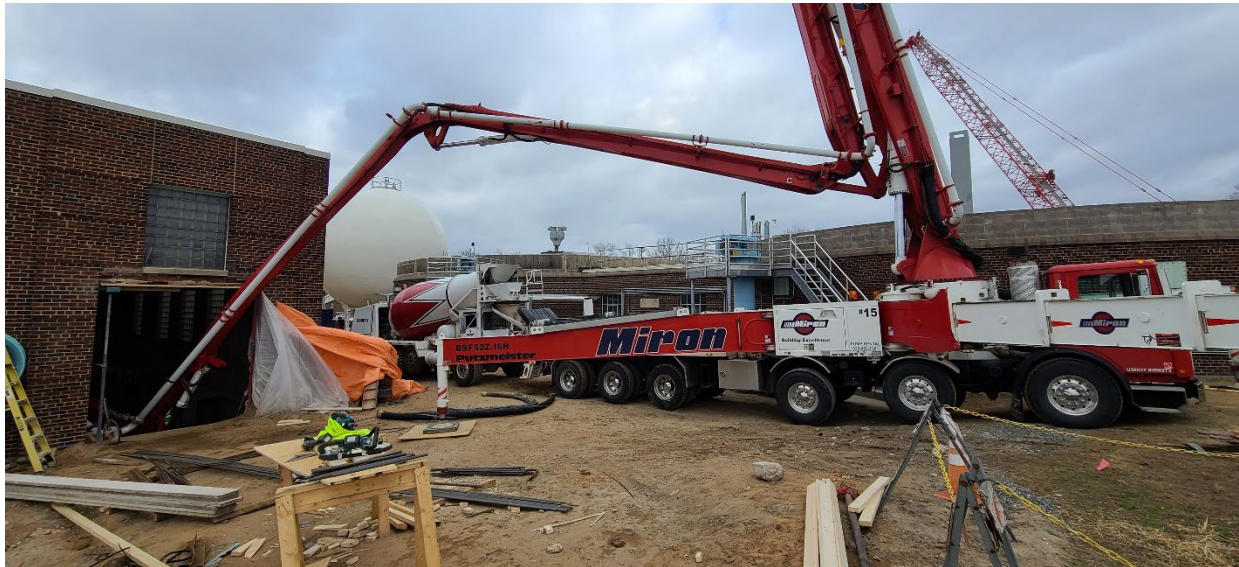
Structure 100 (Main Building): Pumper truck pumping concrete for support walls for generator room.
