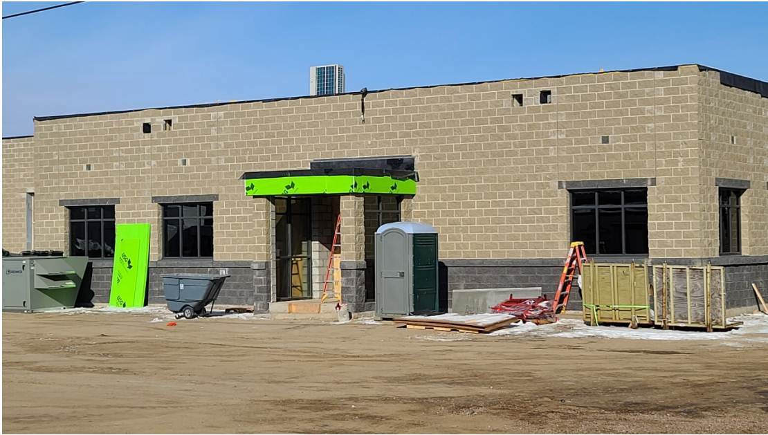
Structure 120 (Administration Building): Vestibule No. 1 roof work and windows in place
