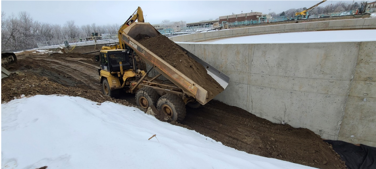
Precision backfilling around Structure 540 (Secondary Clarifier 4).
