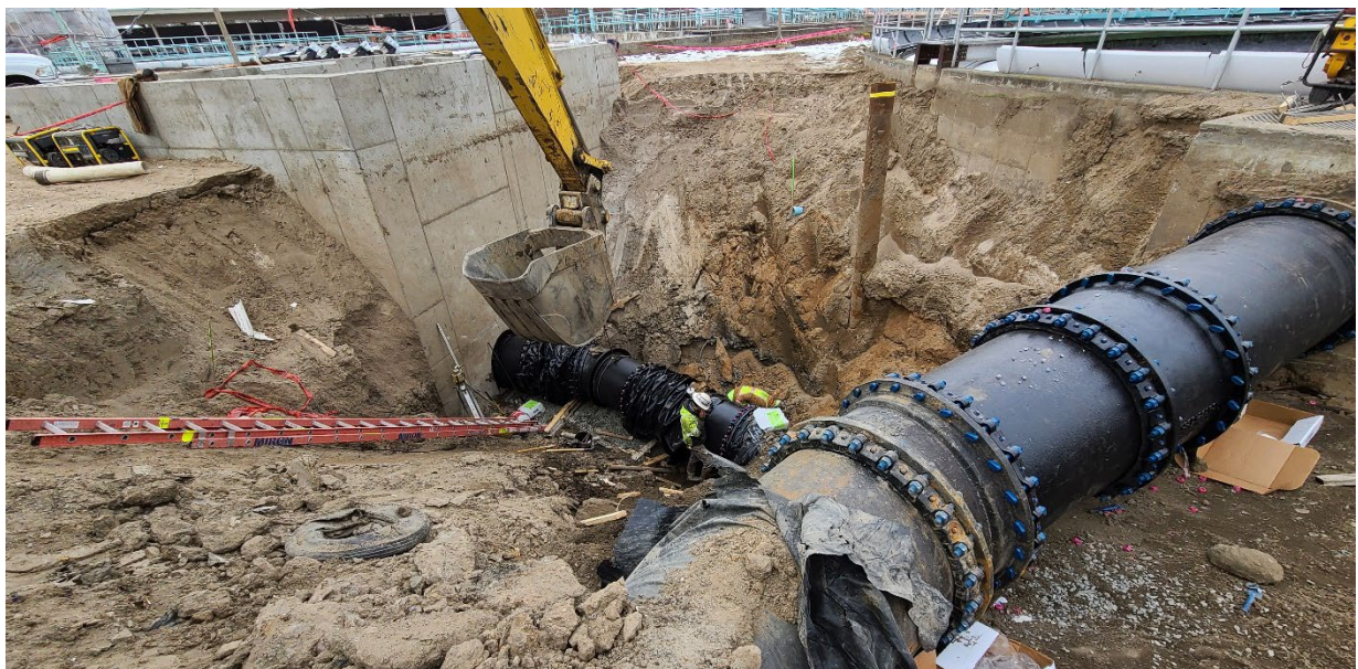
Integrity Grading and Excavating installing the 36-inch Mixed Liquor line into Structure 500 (Secondary Splitter); in the foreground is the new 36-inch Secondary Effluent line from Structure 530 (Secondary Clarifier 3).
