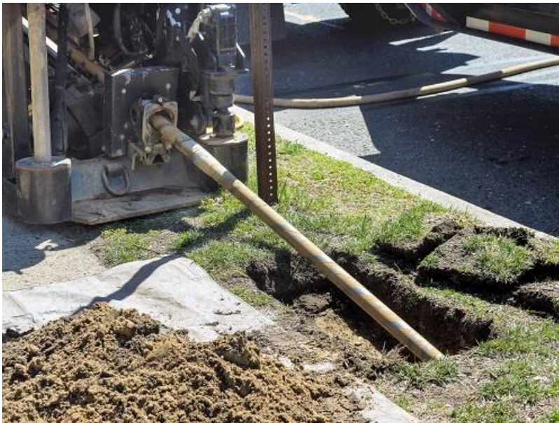
Figure 7-5: Surface Launched HDD Set-Up
