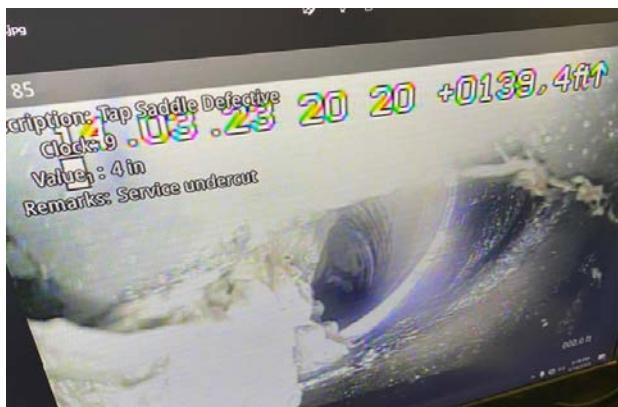
Lateral Opening BEFORE
