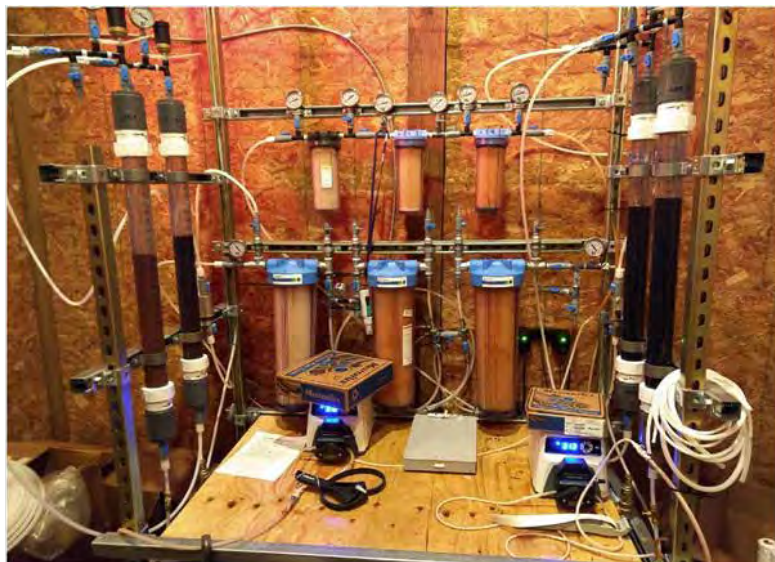
Wood constructed and operated a column study onsite.
