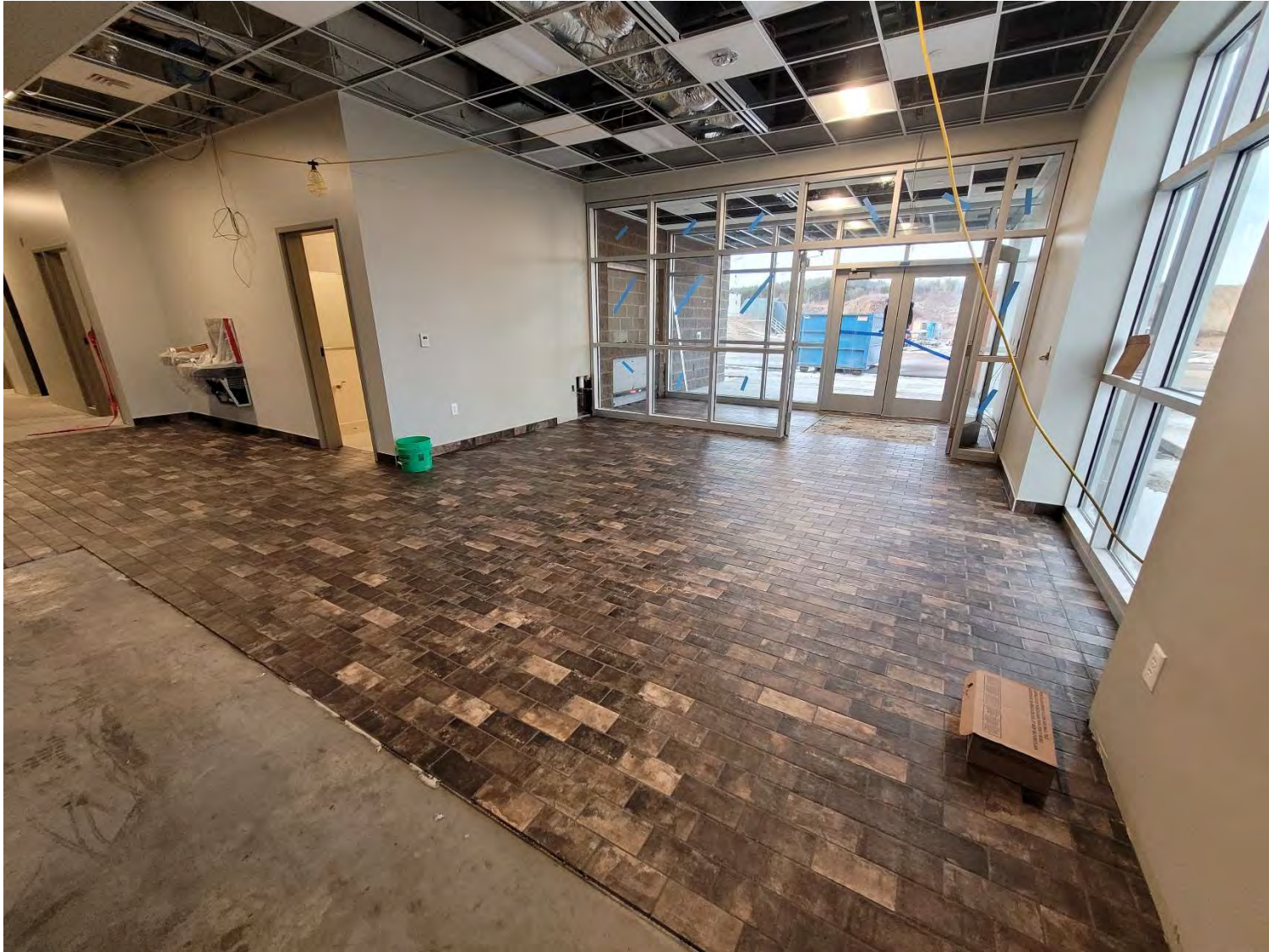
Admin. Bldg. – waiting area tile flooring
