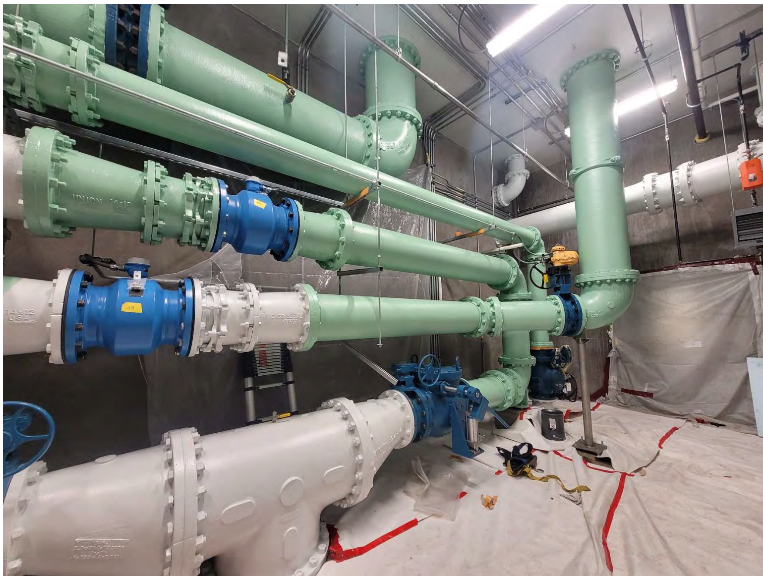
Treatment Facility – piping and fittings in process of final coating
