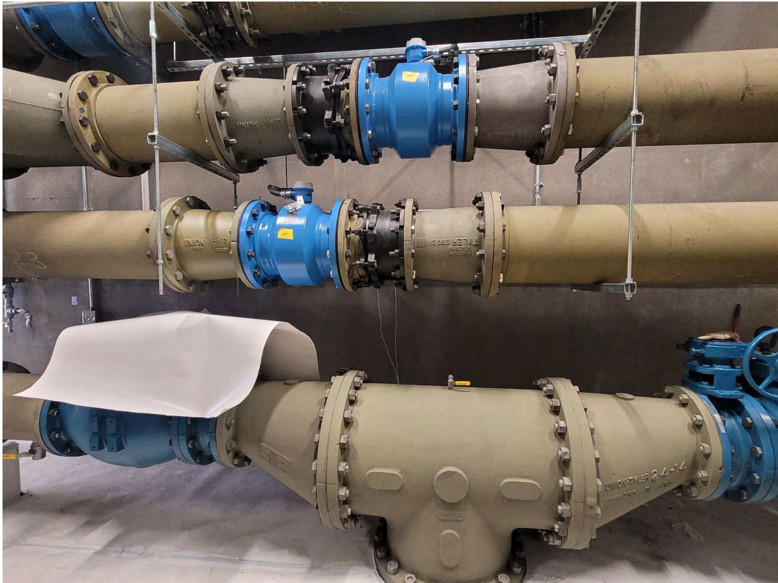
Treatment Facility – Fittings with new prime coat
