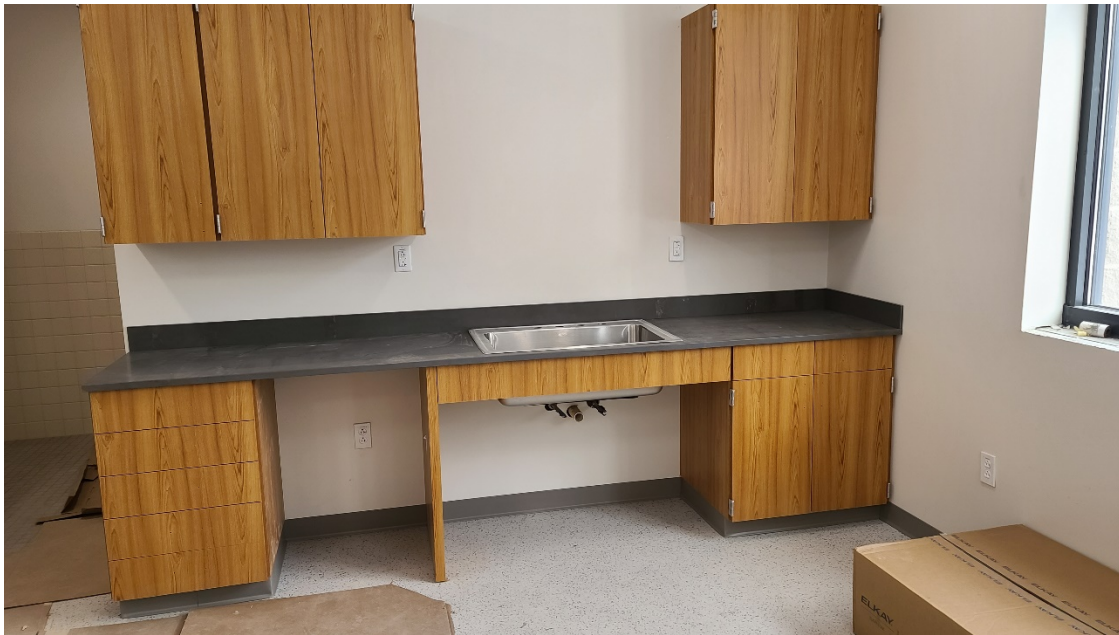
Casework placed in the new breakroom of Structure 120 (Administration Building).
