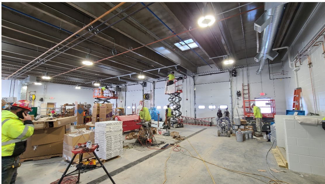
Garage doors, lights and skylights have been installed in Structure 120 (Administration Building).
