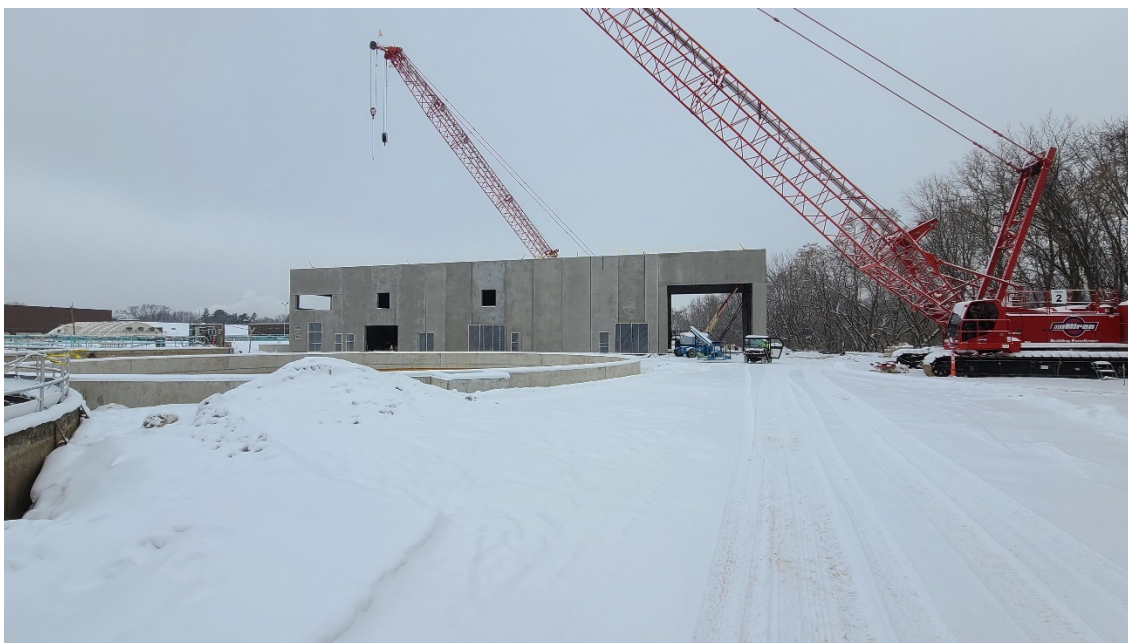
Last of the wall and roof precast work placed for the exterior of Structure 770 (Solids Building).
