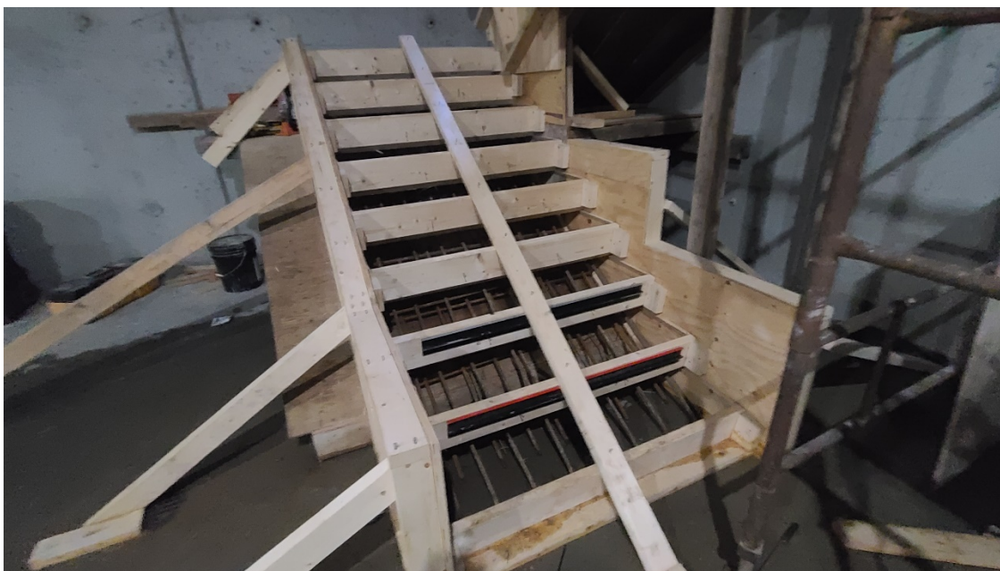
Formwork for northeast corner lower level stairway in Structure 770 (Solis Building).
