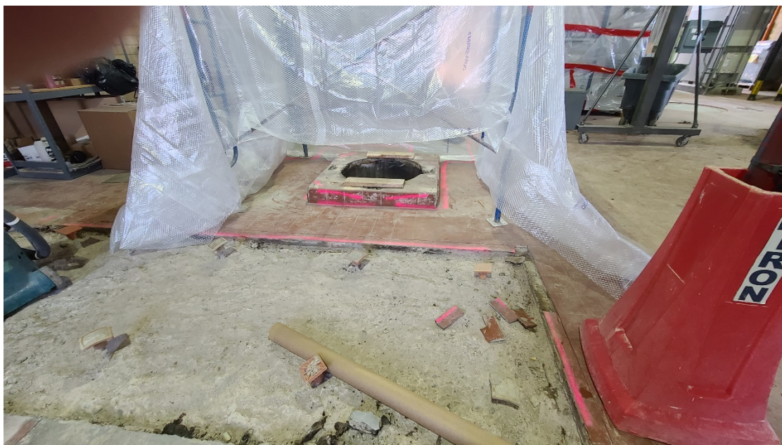
At Structure 400 (ML Channel), Miron preparing to demo existing blower pipe penetration.
