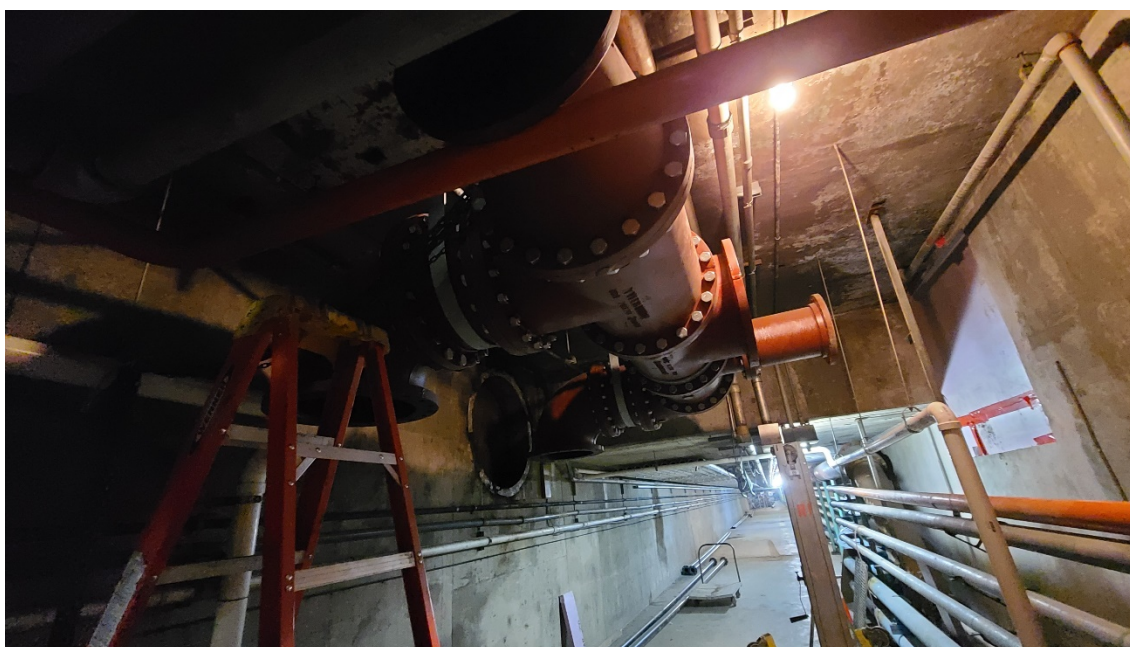
August Winters & Sons placed 16-inch ductile iron return activated sludge piping at south end of Tunnel 900.
