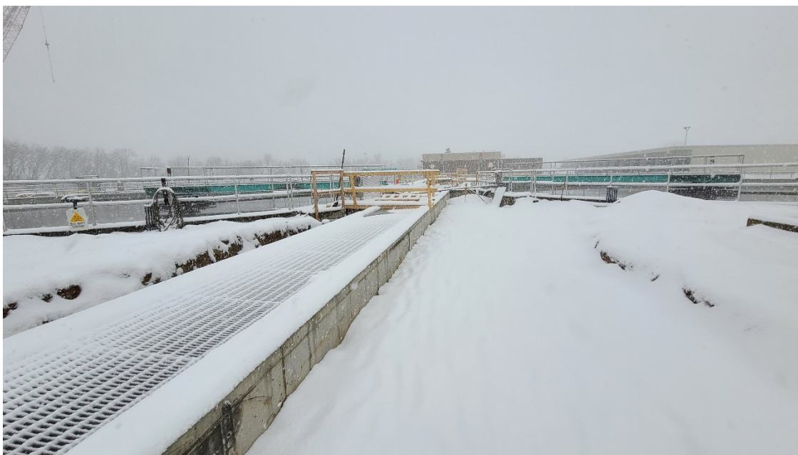
Miron placed the aluminum grating along the top of Structure 350 (Primary Effluent Channel 350).
