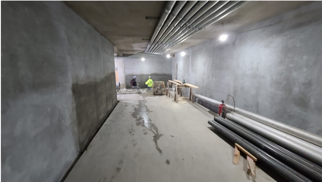
In Tunnel 910, Miron continued with concrete rub on tunnel walls. Van Ert installing 4-inch conduit along ceiling for electrical feeds to Structure 770 (Solids Building).
