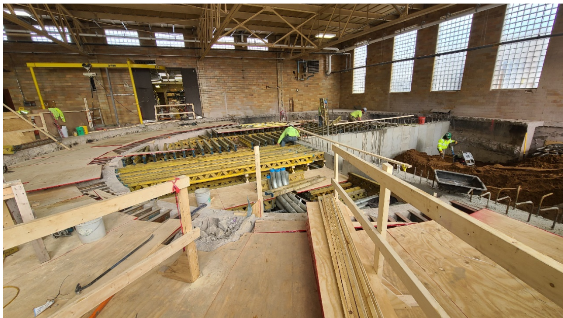
Miron forming for slab on grade pour at Structure 100 (Main Building).
