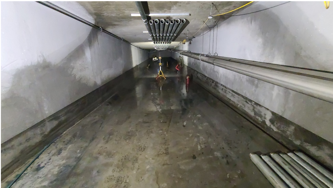
Lines on wall showing sludge depth down new Tunnel 910 heading to Structure 770 (Solids Building).
