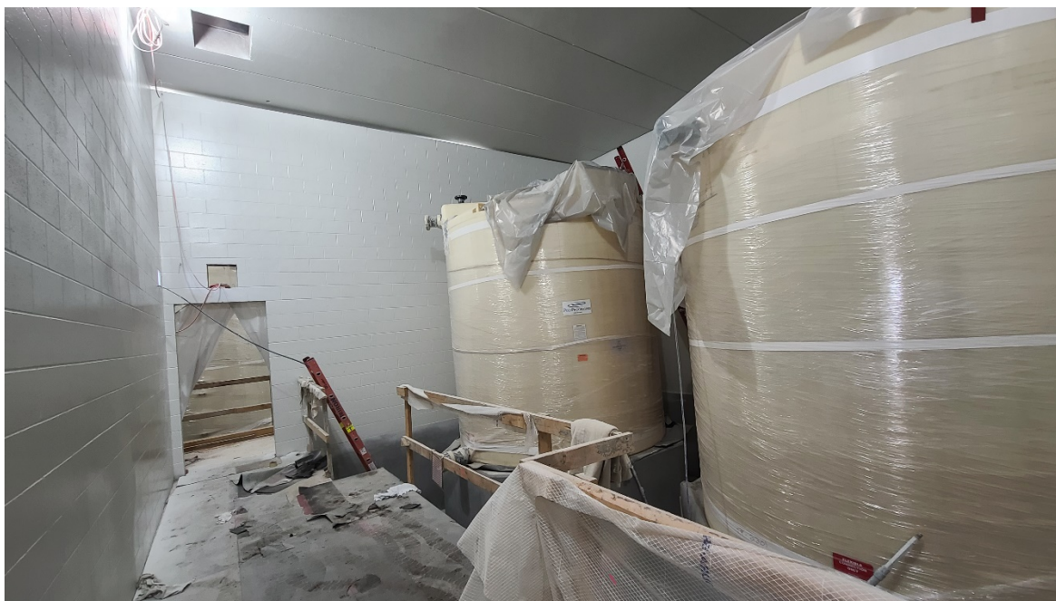
Painters completed chemical tank room coating on interior of Structure 610 (Chemical Building).
