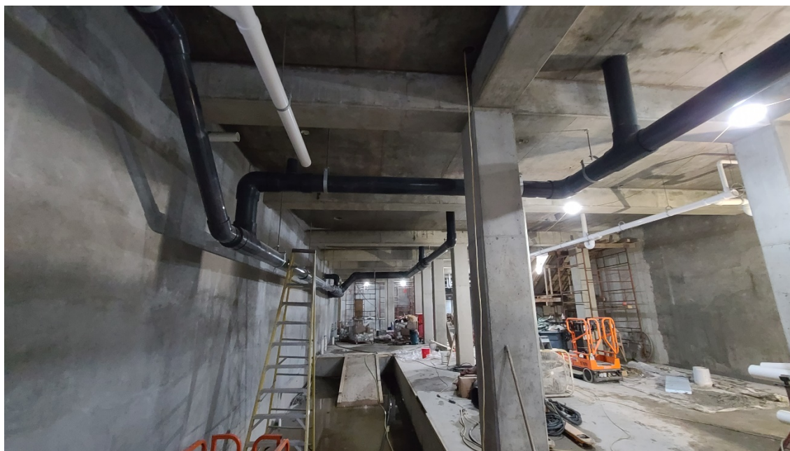
Floor drain and mechanical piping placed in lower level of Structure 770 ( Solids Building).
