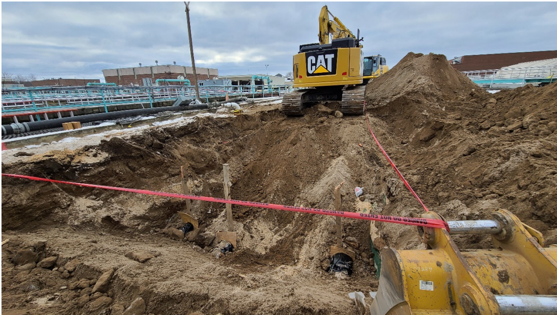
Site work, installing piping runs.
