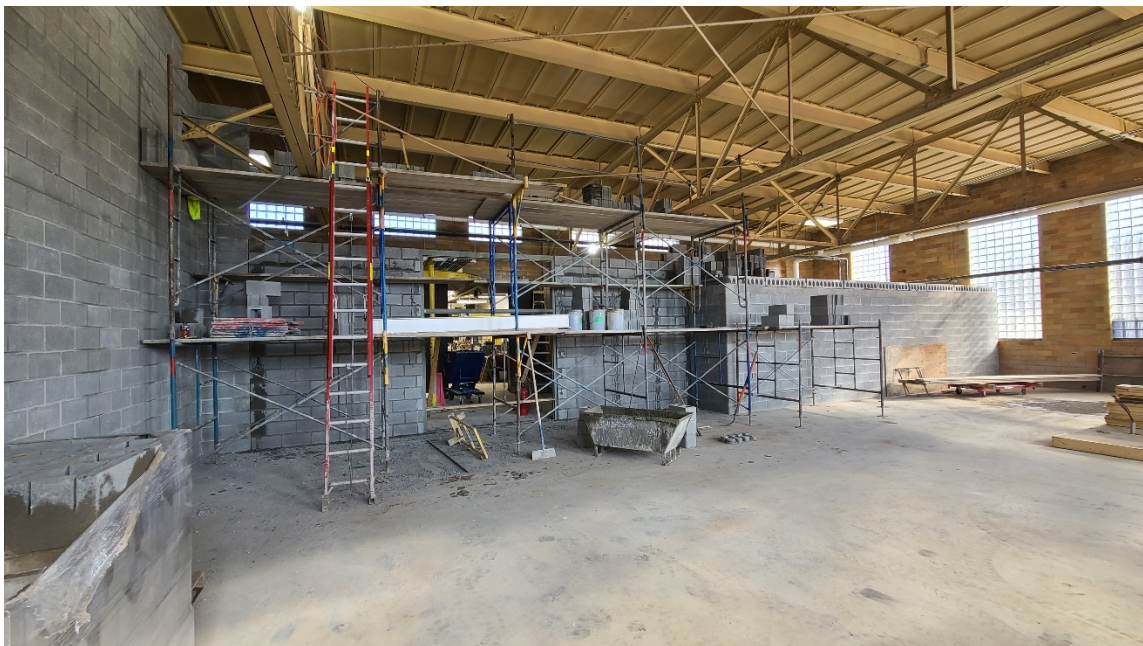
Structure 100 (Main Building) concrete masonry unit walls and precast plank for new electrical room and gas compressor room.
