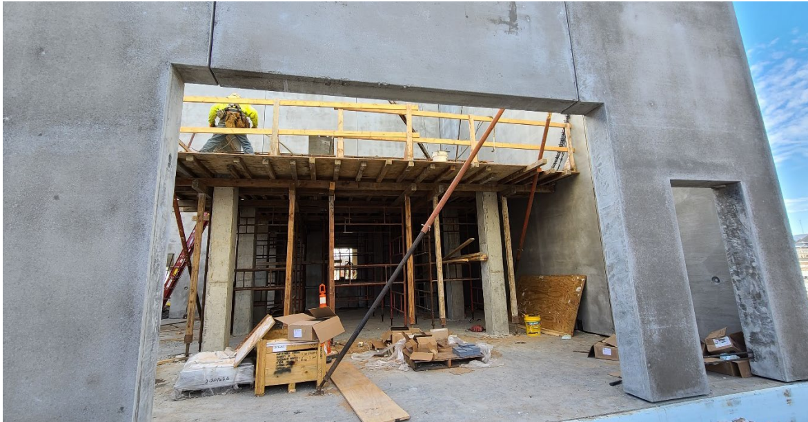
Structural slab for sludge screening room placed in Structure 770 (Solids Building).
