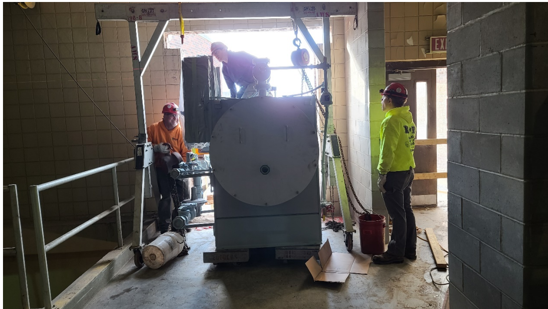
August Winters & Sons bringing in a new biogas boiler through new south access door at Structure 700 (Digester Building).
