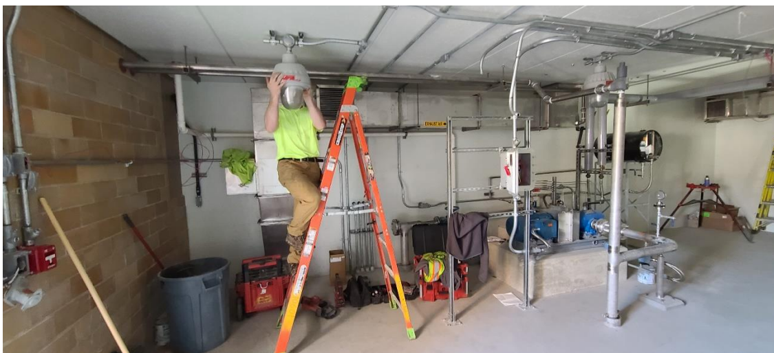
Wiring for control and power to new digester gas compressor and installation of lights at Structure 100 (Main Building).
