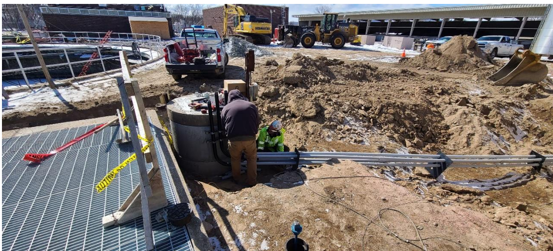
Completion of conduit work to Structure 415 (Basin Drain Pump Station) for power, controls and disconnects.
