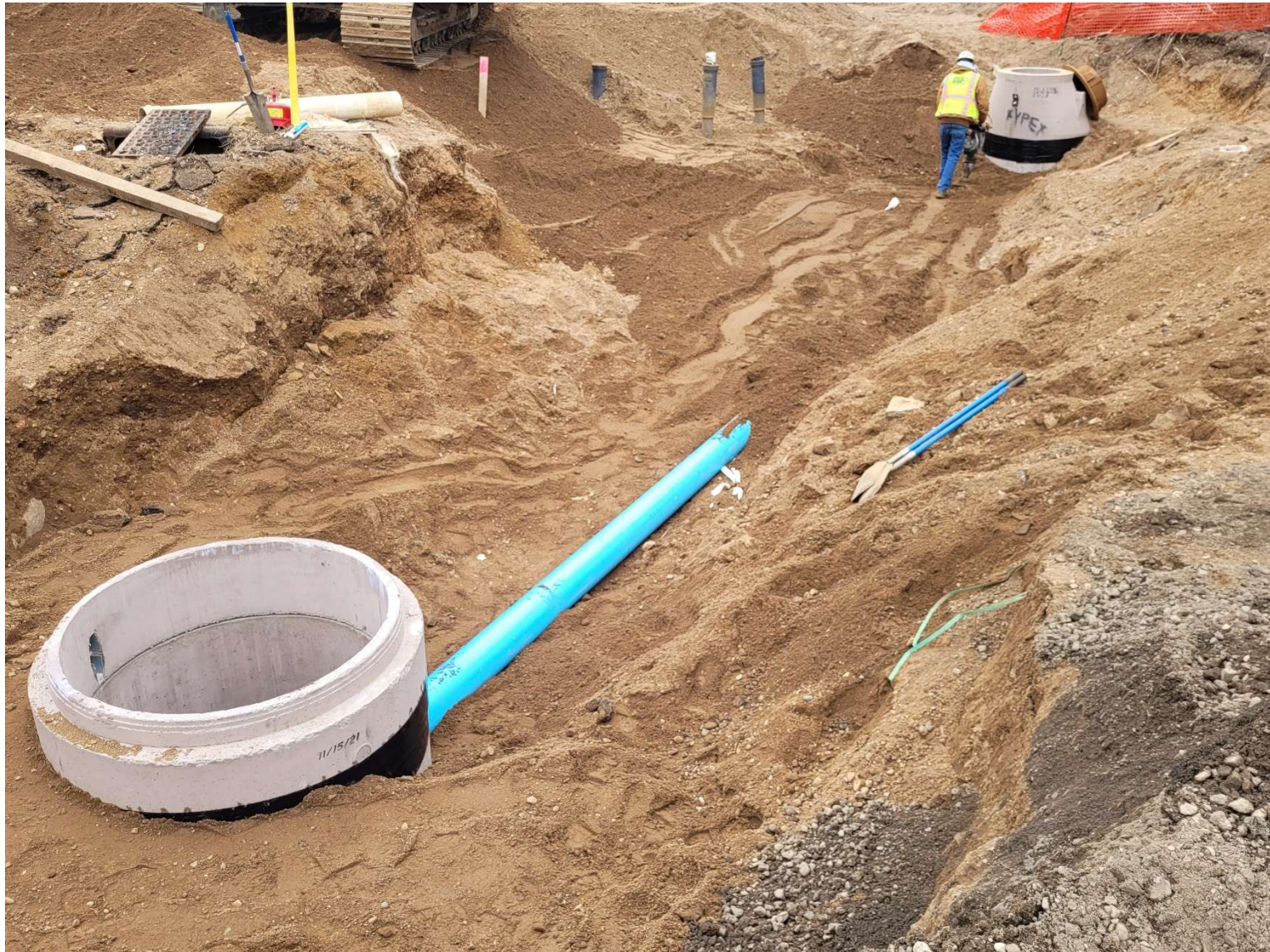
Manhole and Sanitary Sewer Installation – Bugbee Ave.
