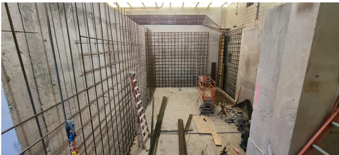
Rebar being placed for new secondary effluent treatment basins of Structure 600 (Effluent Building).
