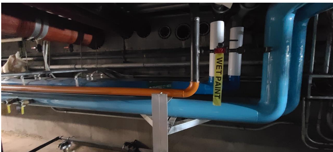
Painting of process pipe and gas lines continued in the 900 Tunnel
