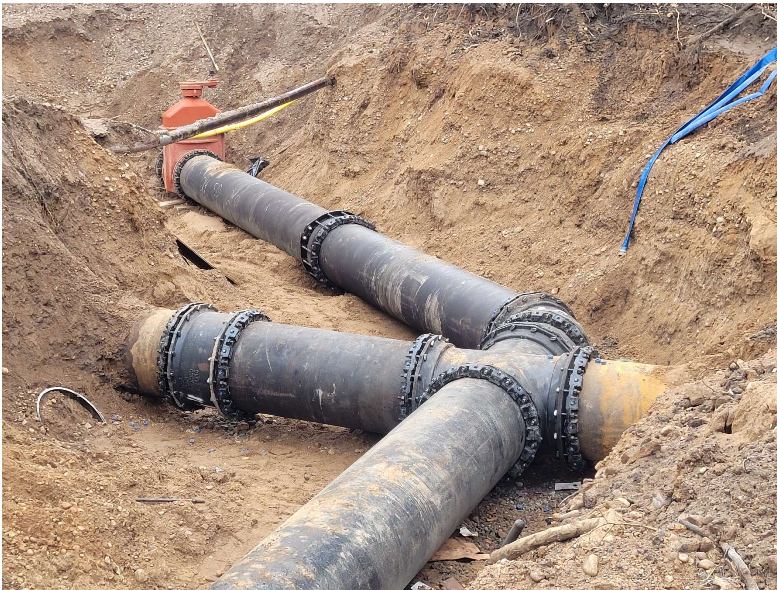
Water Main Connection to New Facility. Lighter Color Pipe is Existing Water Main to be Reused
