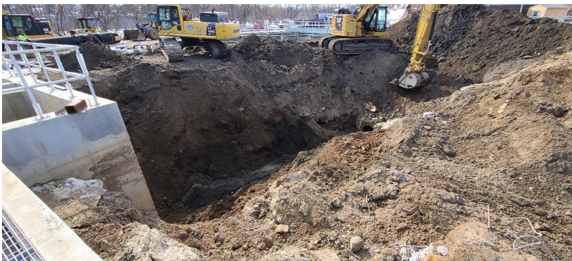
Integrity Grading and Excavating working on the mixed liquor (ML) line to Structure 510 (Secondary Clarifier 1).
