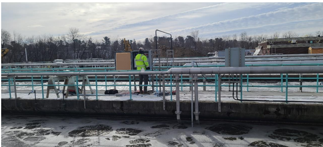
Van Ert Electric working on new dissolved oxygen probe cleaning system for Aeration Basin 1 of Structure 410 (Activated Sludge Basins).
