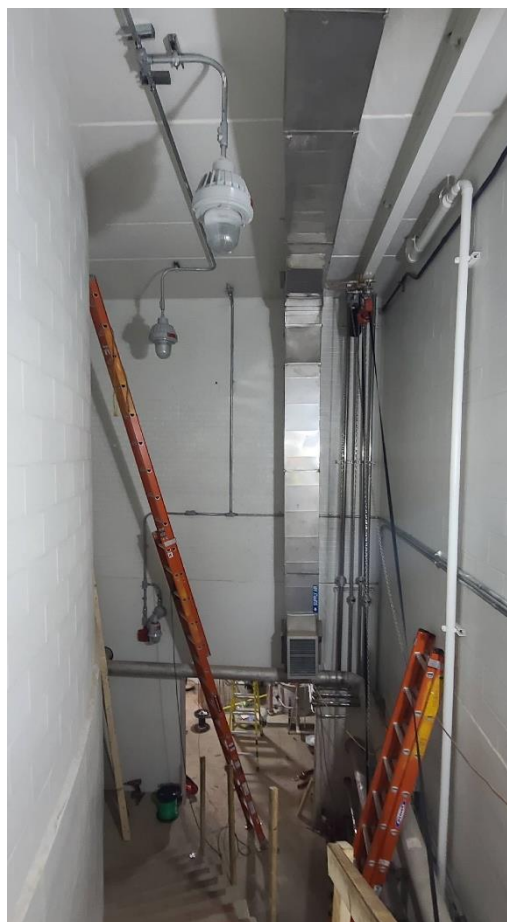
New interior lighting place in gas handling room of Structure 700 (Digester Building).
