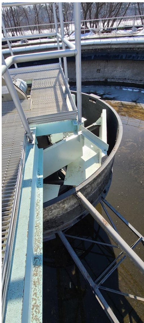
New baffles placed in Structure 520 (Secondary Clarifier 2).
