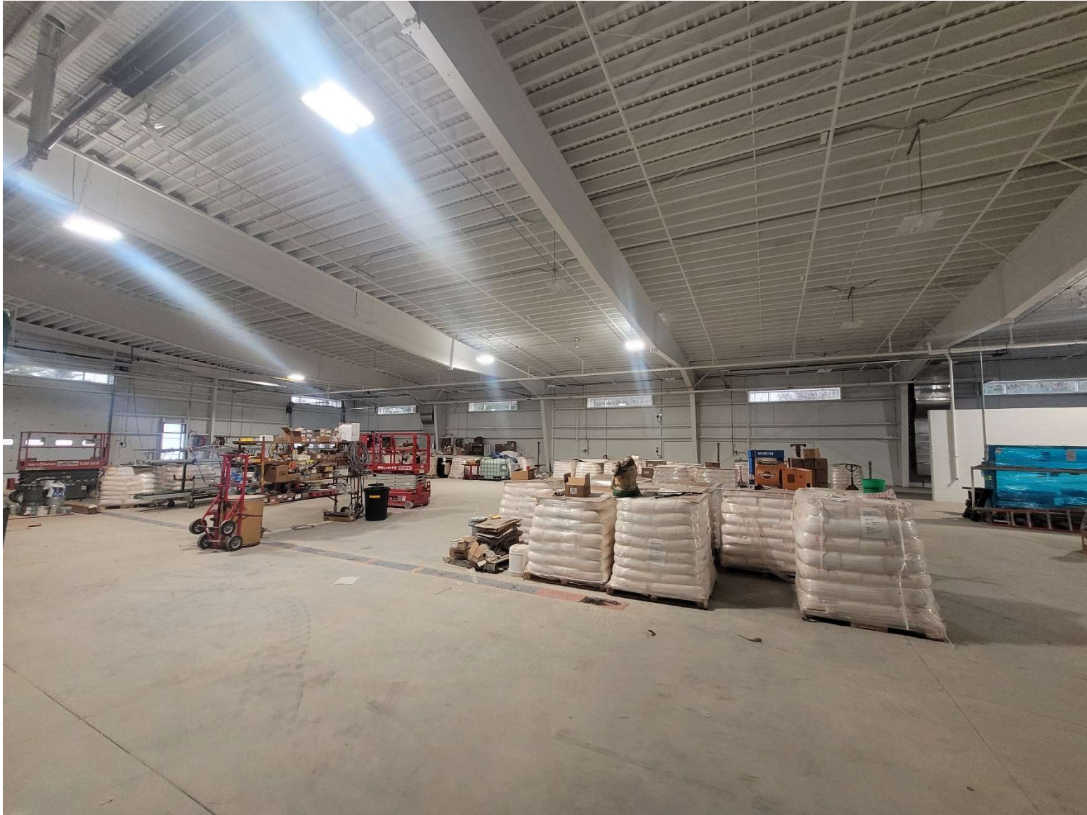
Admin. Bldg. – Vehicle Storage Garage
