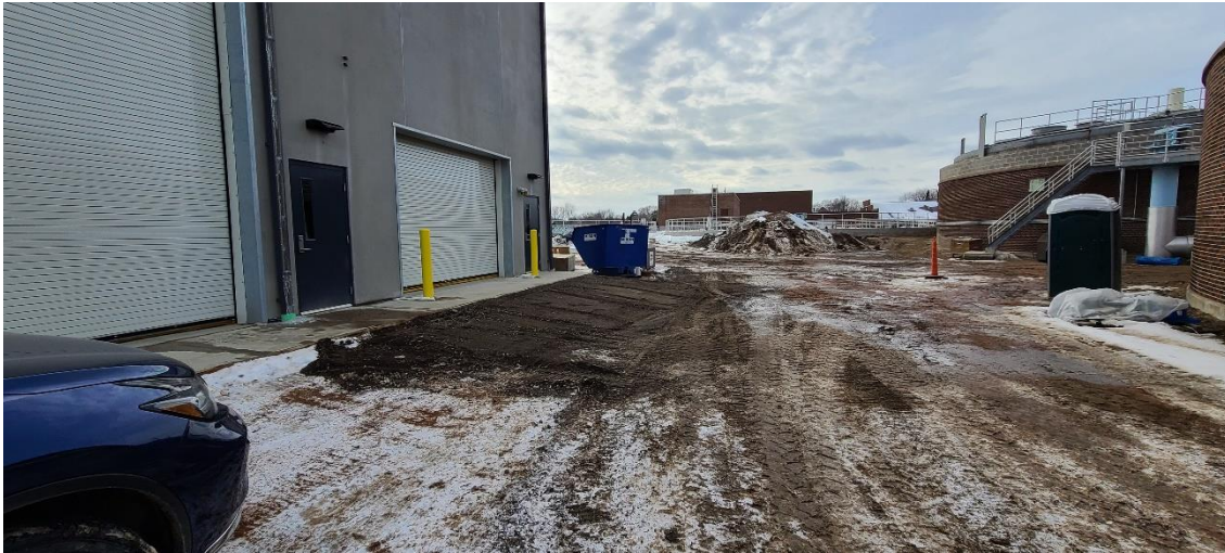
Precision Grading and Excavating placing material for an access ramp to be used for sludge screenings dumpster collection.
