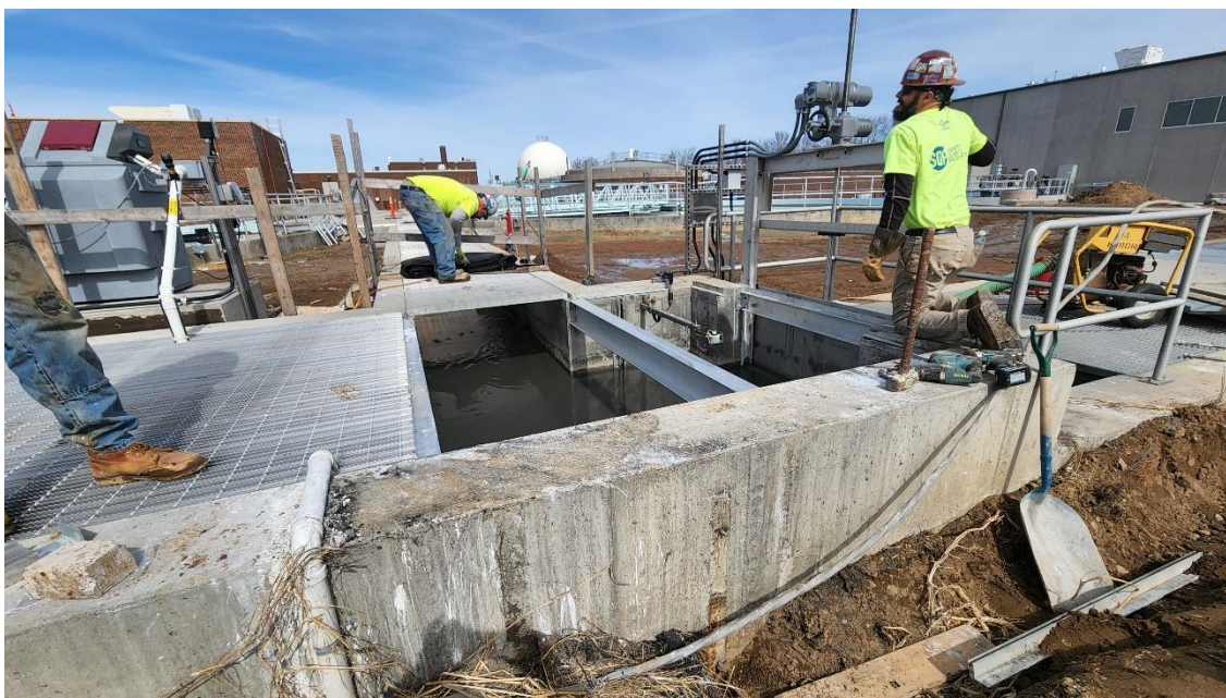
Wet weather gate placed and grating being placed on Structure 404 (Junction Structure).
