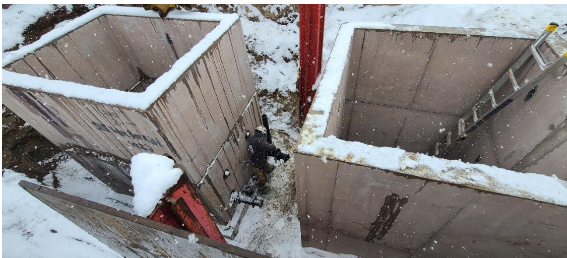
Structure 515 (Secondary Scum Manhole 1)
