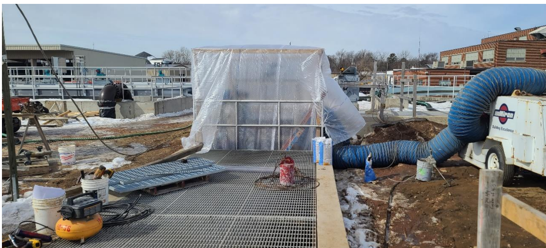
Keeping grout warm so it will set up properly for north influent gate placement at Structure 410 (Activated Sludge Basins).
