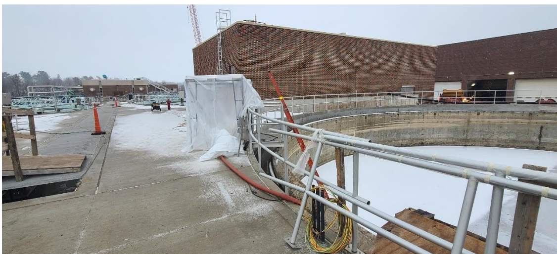
Omni sand blasting and painting set up for Structure 310 (Primary Clarifier 1) scum manhole
