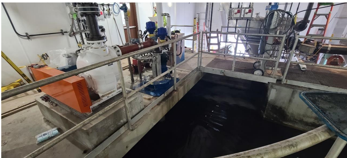
Primary effluent flowing through new grit equipment at Structure 200 (Grit Building).
