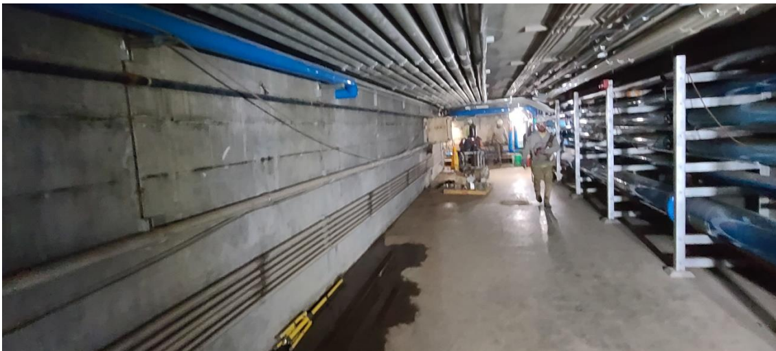
North end of the 900 Tunnel with all old piping demolished.
