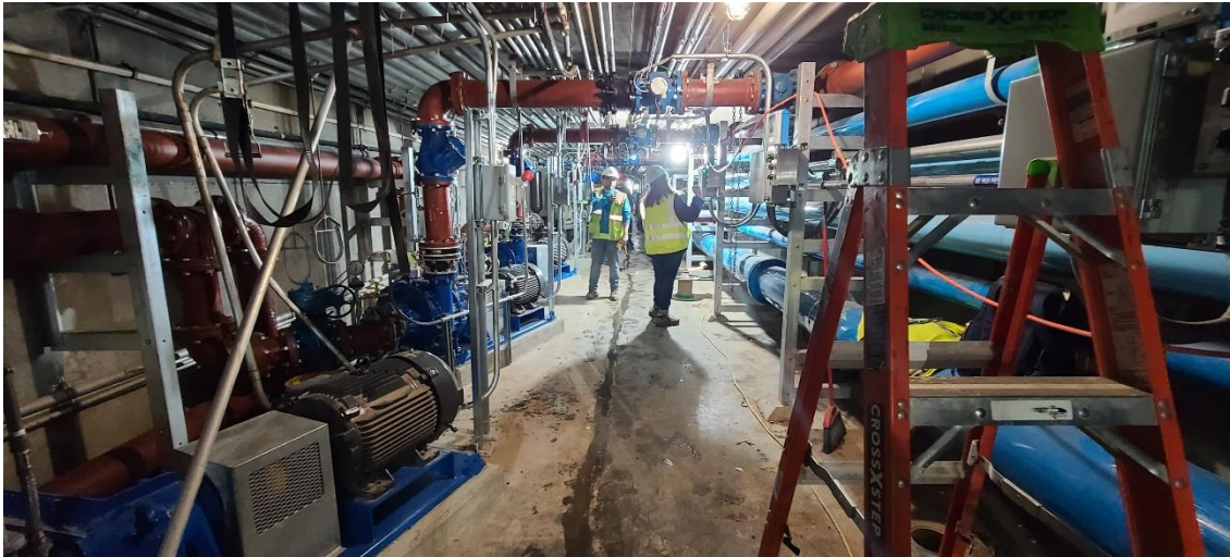
Vender checkout and startup of the primary sludge pumps
