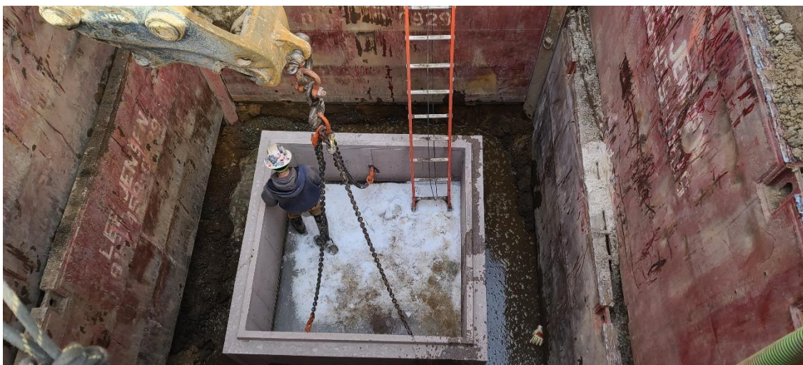
Placement of the first section of Structure 515 (Scum Manhole 1).
