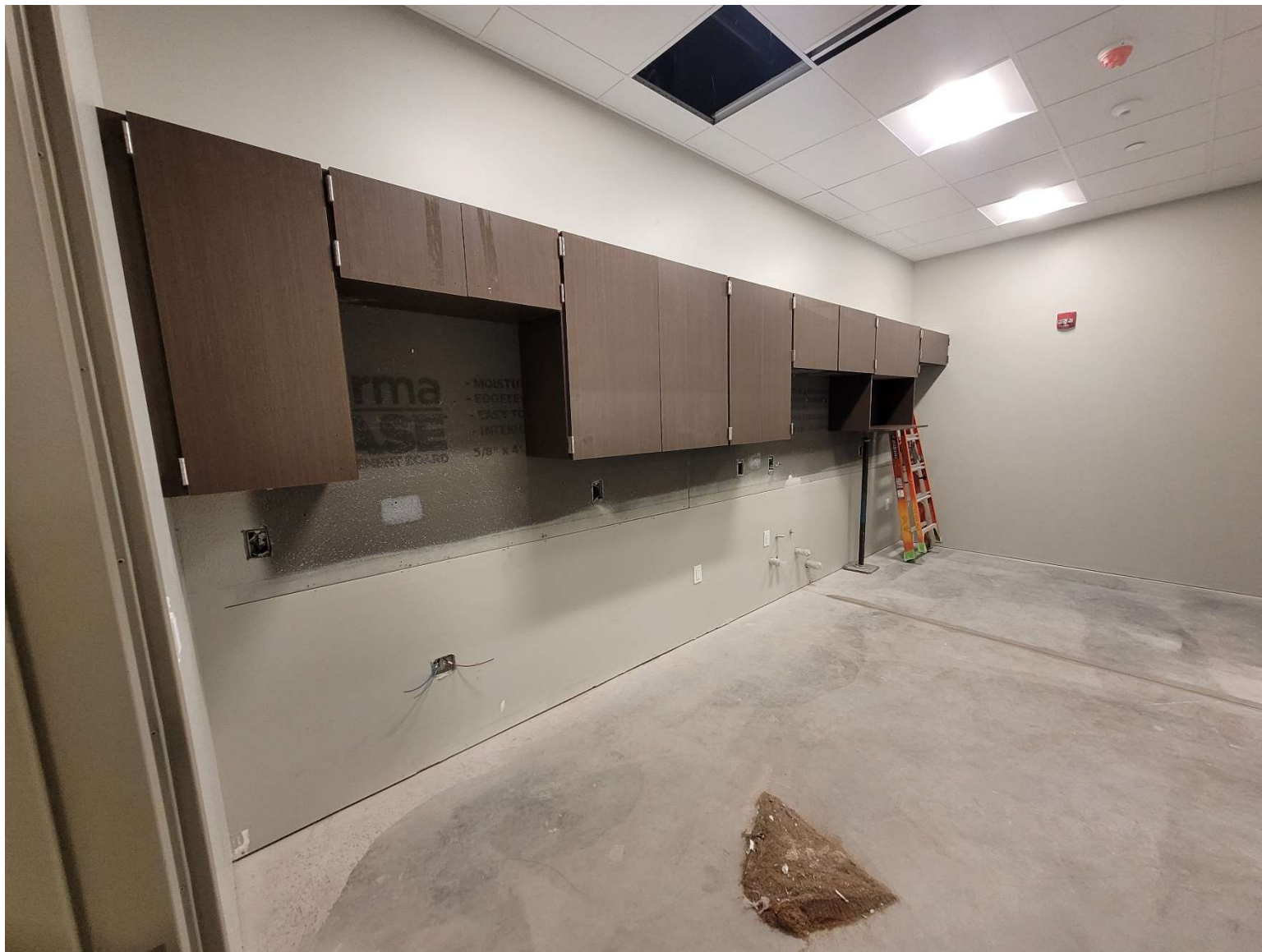
Admin. Bldg. – Kitchen Area in Break Room
