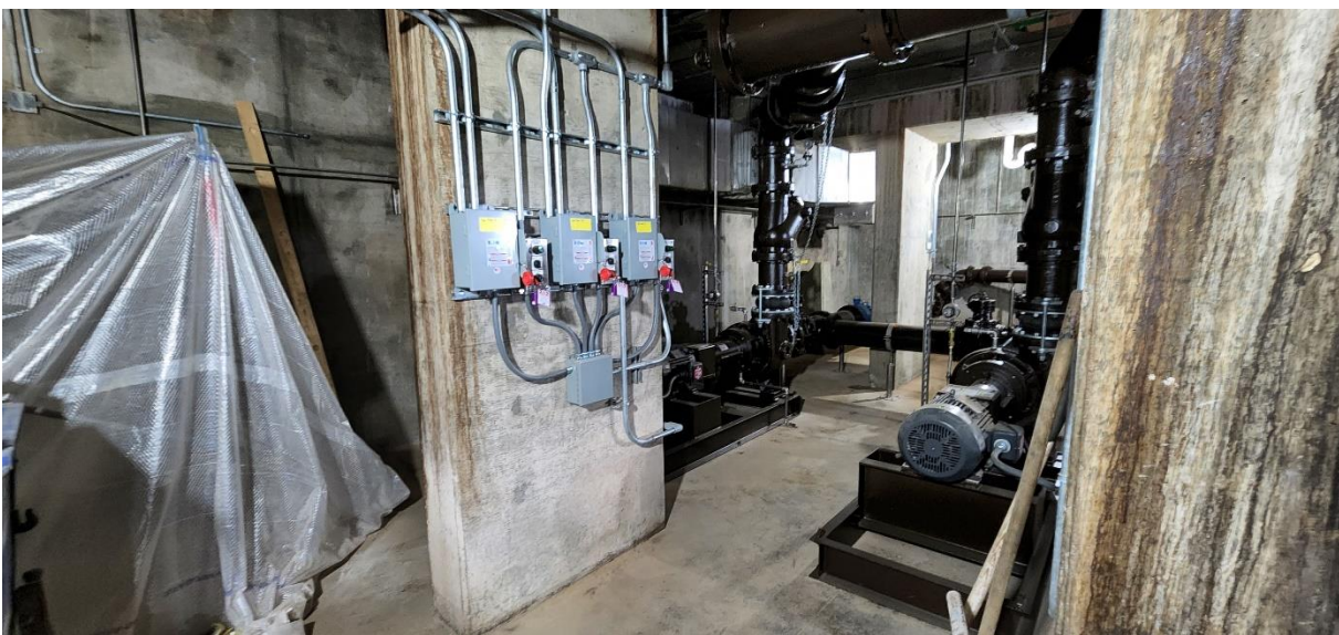
New return activated sludge (RAS) pump disconnects installed at Structure 400 (Activated Sludge Building).
