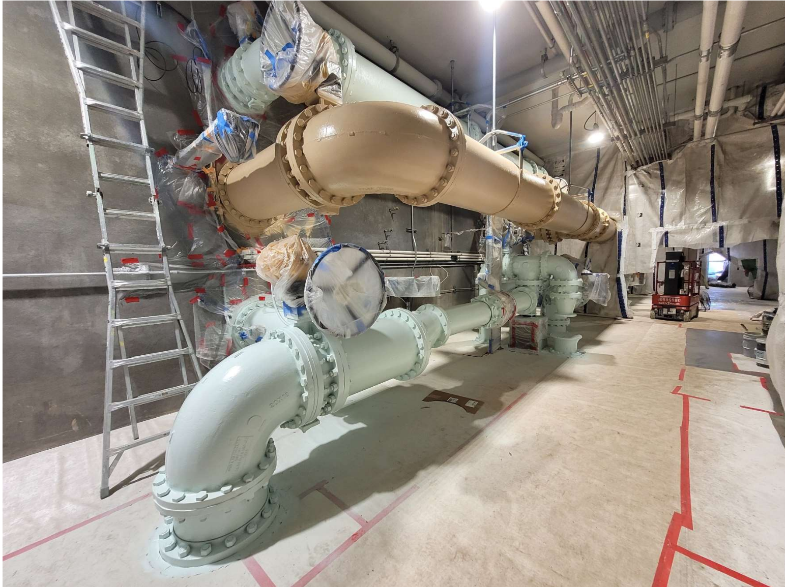
Grade-Level Pipe Coating
