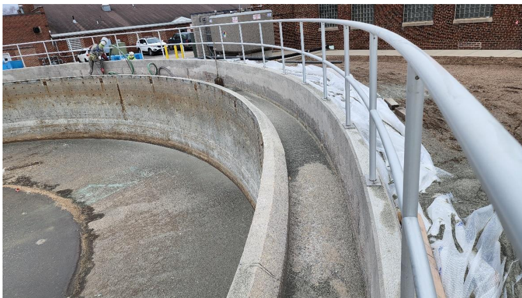
Sand blasting Structure 310 (Primary Clarifier 1) trough to prepare for coating.
