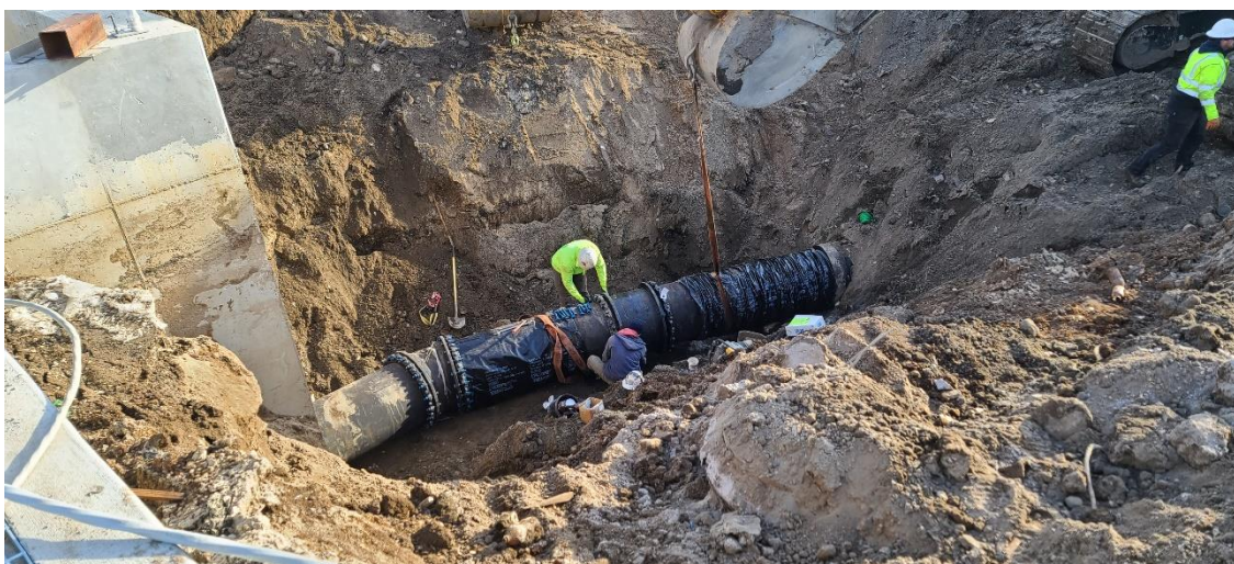
Final fitting being bolted up for mixed liquor (ML) lines to Structure 510 (Secondary Clarifier 1).
