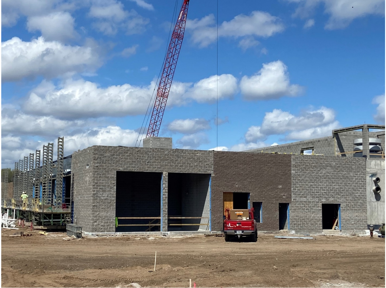
Exterior split face block along the south wall of the drinking water treatment facility
