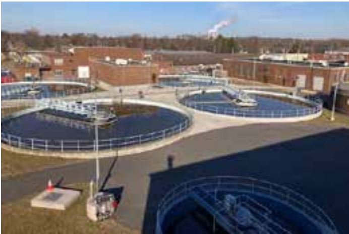
Primaries and primary sludge thickener
