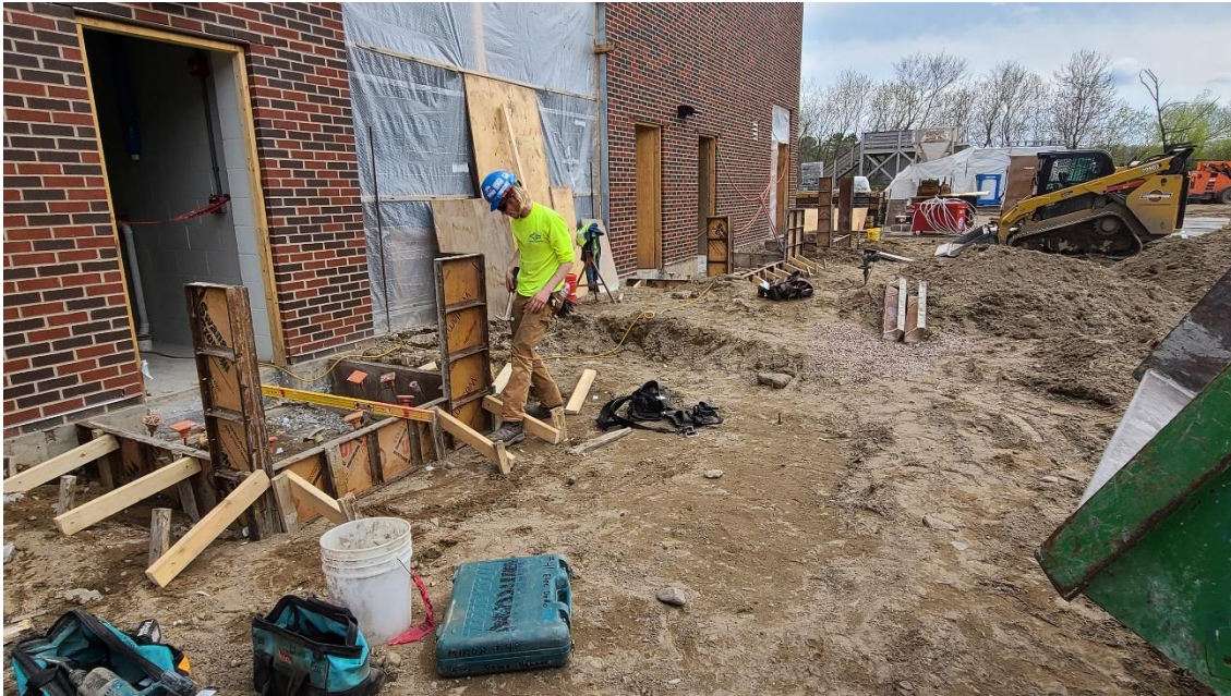
Doorway stoops being formed at the west side of Structure 610 (Chemical Building).
