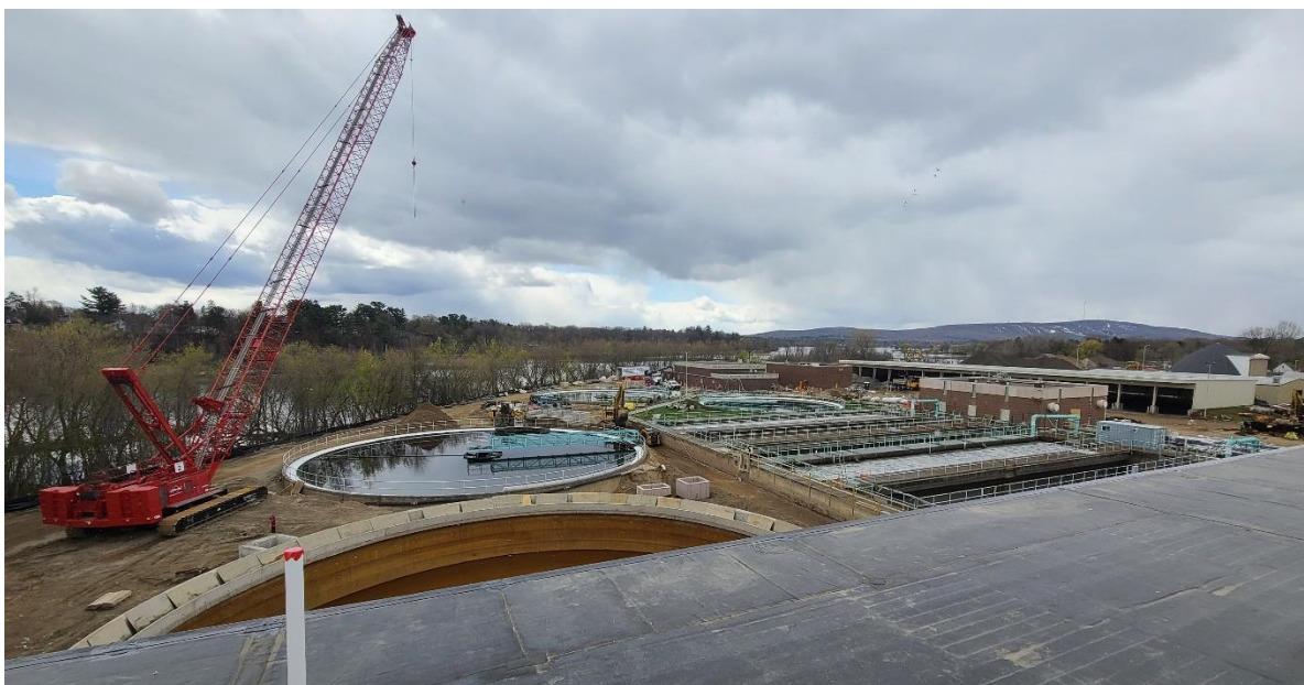
View from the top...of Structure 770 (Solids Building) that is; looking south.
