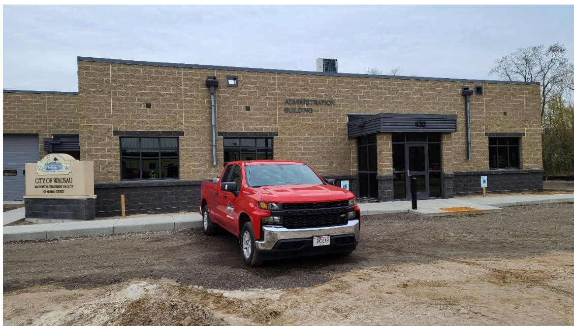
New sign, lettering, numbering, sidewalk have been placed for Structure 120 (Administration Building).
