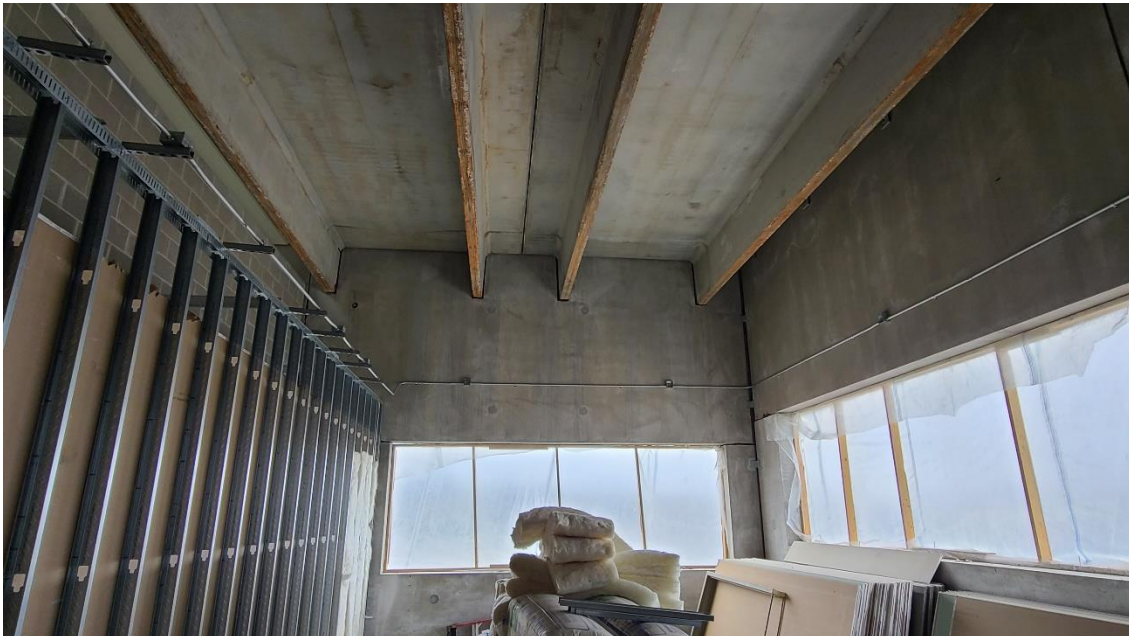
Work ongoing in new control room of Structure 770 (Solids Building).
