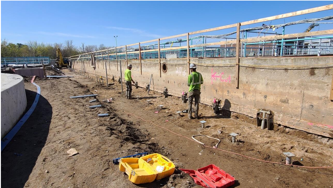
Helical piers placed for the Structure 420 (Mixed Liquor Channel) footings.
