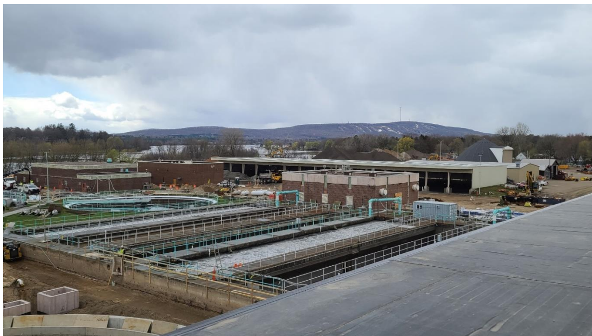
Another rooftop view, looking southwest from Structure 770 (Solids Building).
