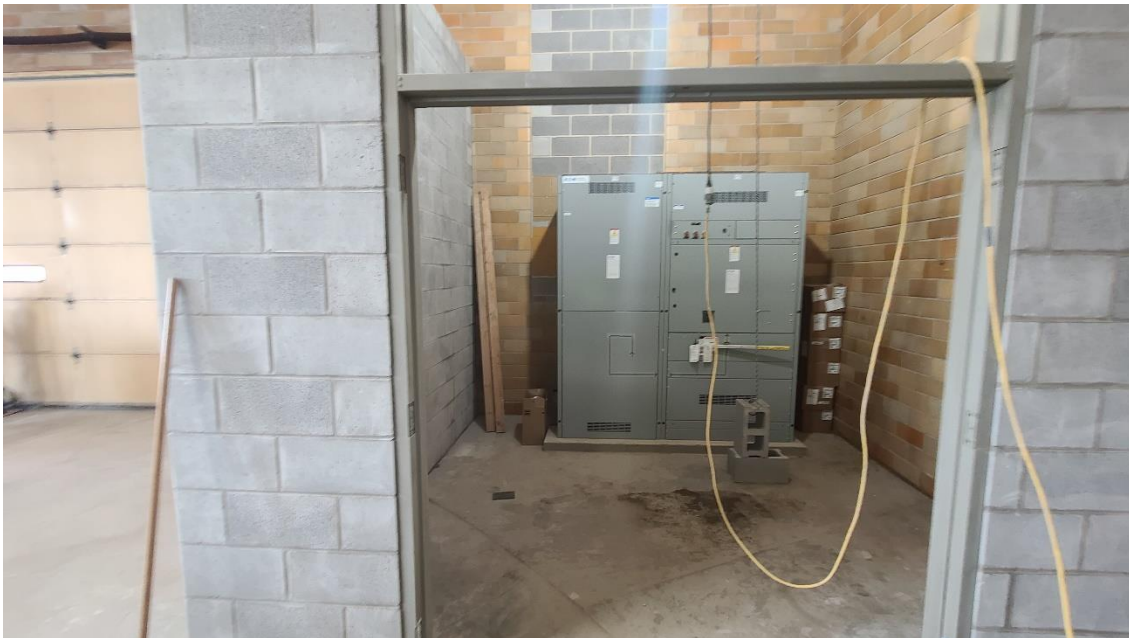
Structure 100 (Main Building): masons completed block walls of northwest electrical service room with window infill and door frame set.
