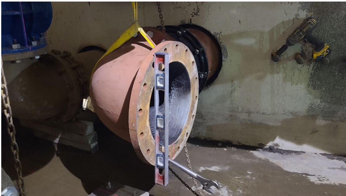
New 16-inch pipe and elbow being placed at the location of the leak site in the lower level of Structure 700 (Digester Building).
