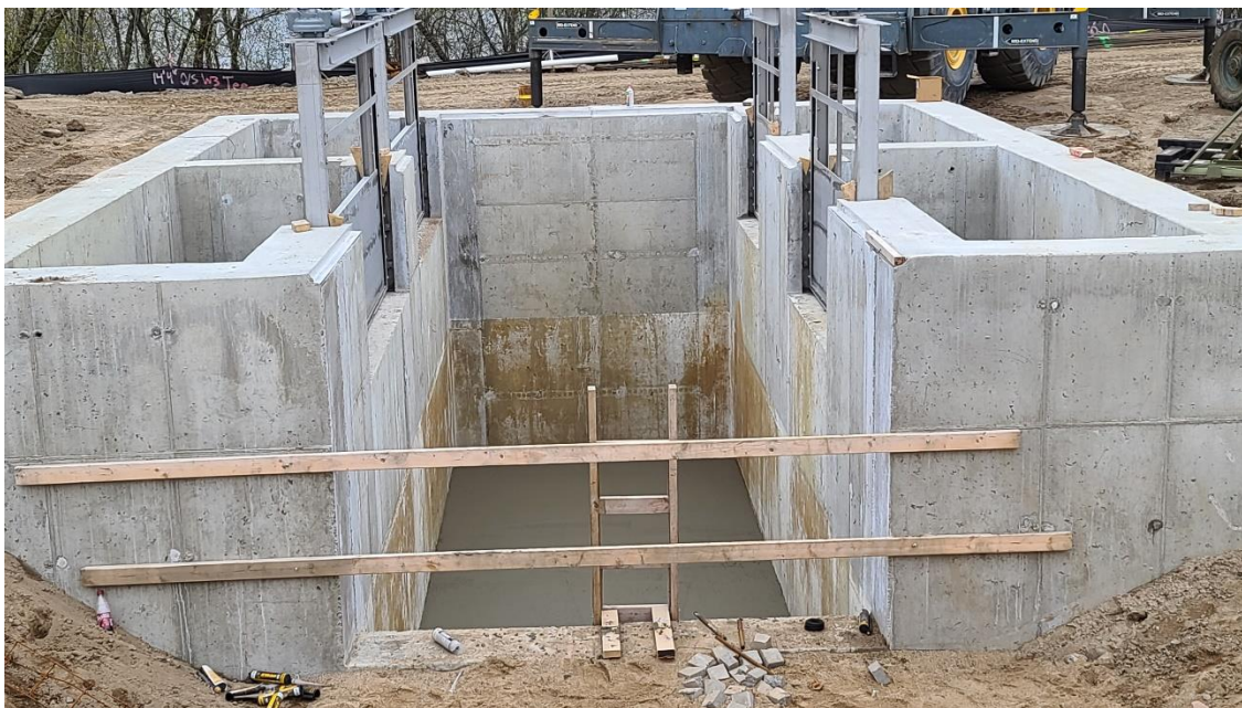
Structure 500 (Secondary Splitter) last slab pour and gates installed but not yet grouted in place.
