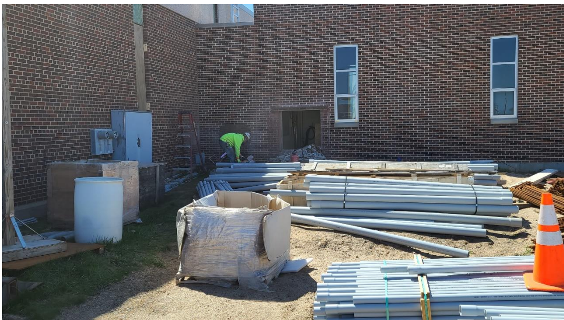
Saw cutting opening and demo of walls on the north side of Structure 400 (Activated Sludge Building).
