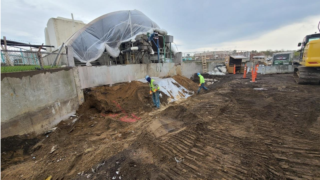
Structure 200 (Grit Building) roof demolition, existing west slab and footings removed and preparations made for raw wastewater piping and new footings and slab.
