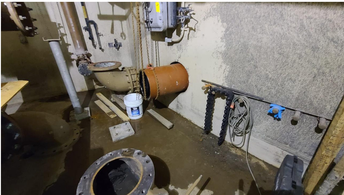
New 16-inch pipe connecting to Structure 740 (Digester 4); the site of the Valentine's Day sludge leak.
