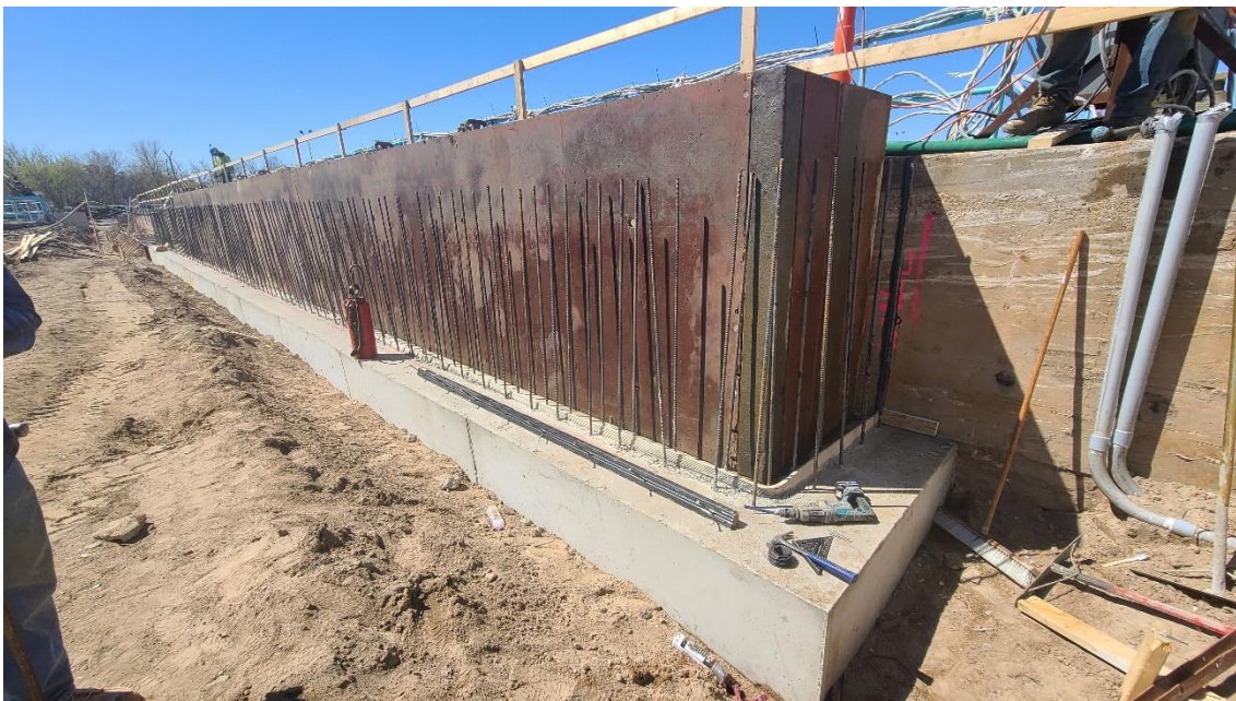
North footings of Structure 420 (Mixed Liquor Channel) complete with foundation wall being formed and rebar placed.
