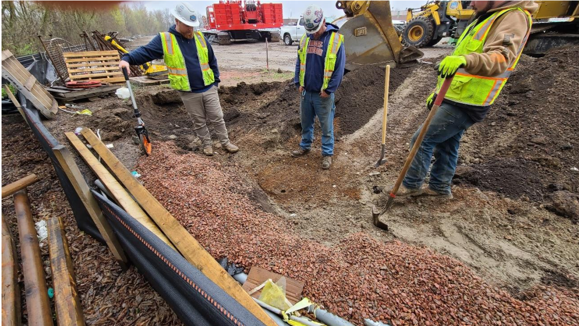
Buried storm manhole discovered east of Structure 540 (Secondary Clarifier 4) before Wisconsin River outfall.
