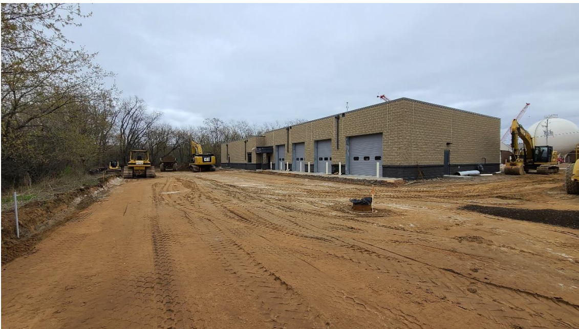
Precision Grading working on the grading north side parking area of Structure 120 (Administration Building).
