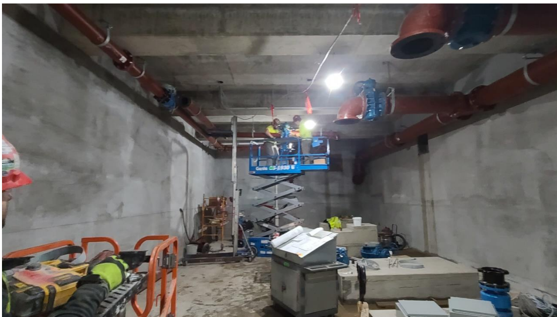
Lower level overhead ductile iron piping for the waste activated sludge and return activated pumps being installed within Structure 770 (Solids Building).
