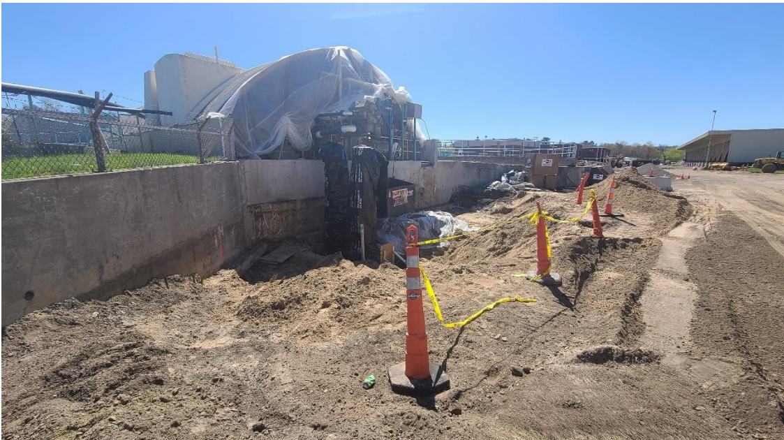
New raw wastewater piping installed to Structure 200 (Grit Building) and helical piers to be placed for new footings/foundation.
