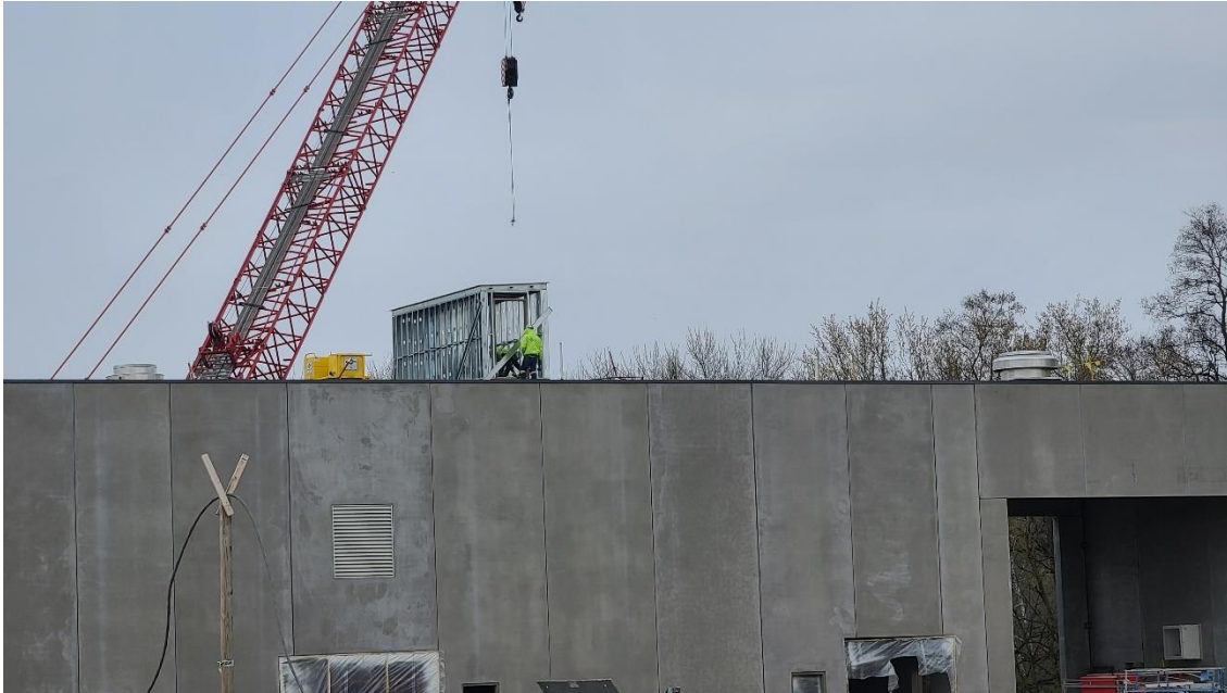
Structure 770 (Solids Building) roof access dog house steel stud framework being completed.
