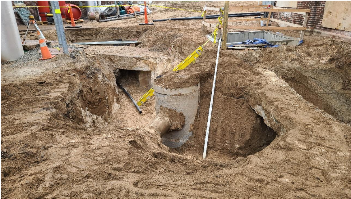
Integrity Grading & Excavating's installation of biogas piping requires working around a maze of piping, conduit, electrical vaults and storm manholes.
