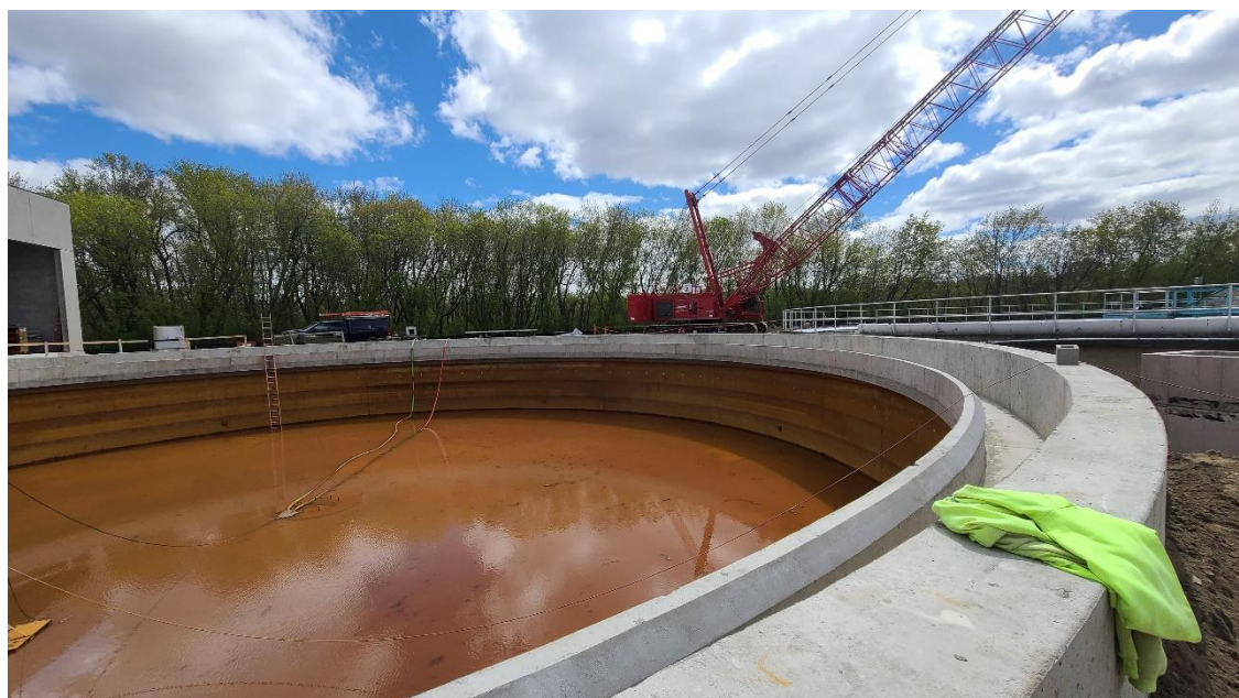
Structure 540 (Secondary Clarifier 4) launders complete, being pumped down to allow for installation of new interior equipment.
