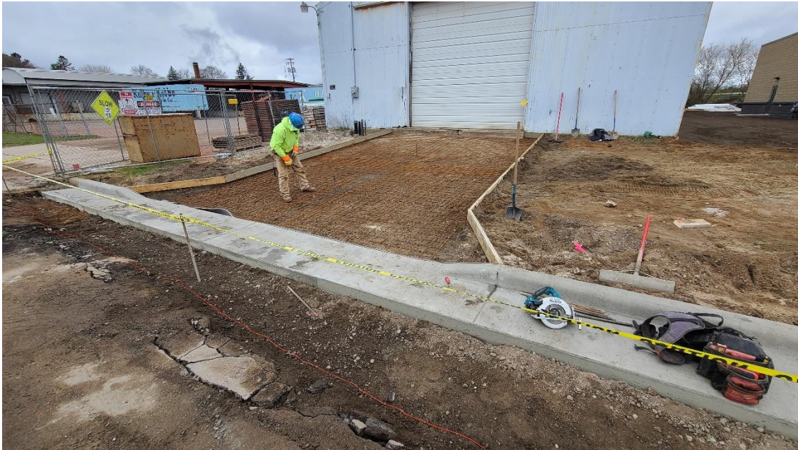
Concrete formwork for the driveway entrance to Structure 115 (Equipment Storage Building) adjacent to Structure 120 (Administration Building).
