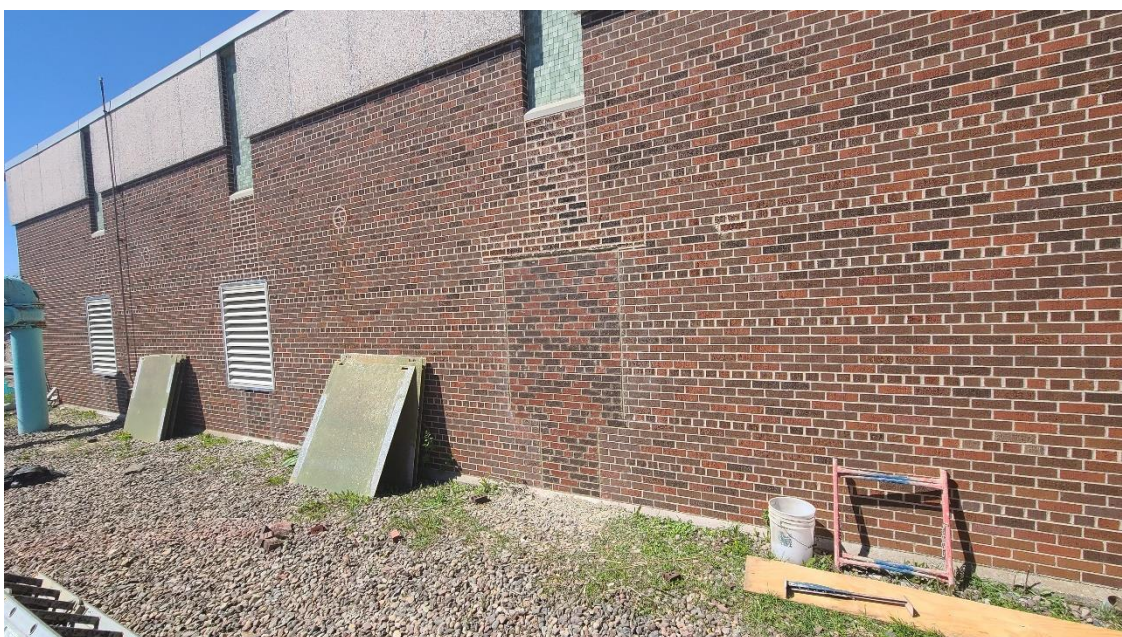
New exterior brick infill of former blower vent opening, on exterior east wall of Structure 400 (Activated Sludge Building).
