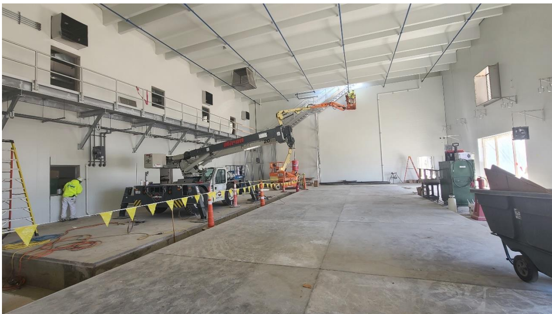
Dryer room pad complete, walkway construction nearly complete at Structure 770 (Solids Building).
