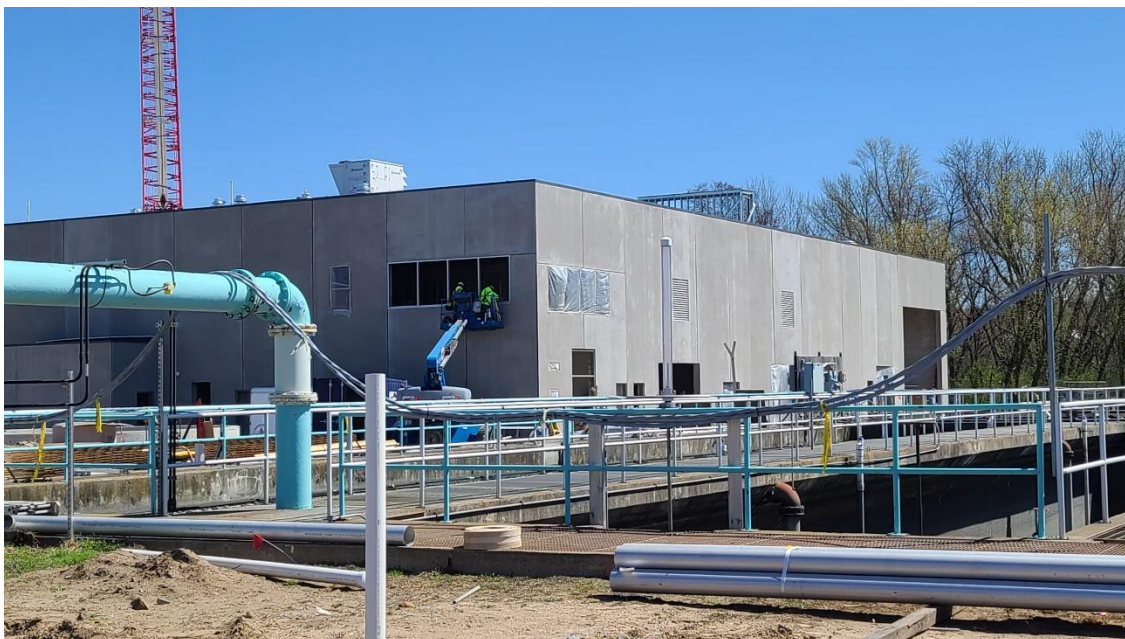
Windows and door frames being installed in Structure 770 (Solids Building).
