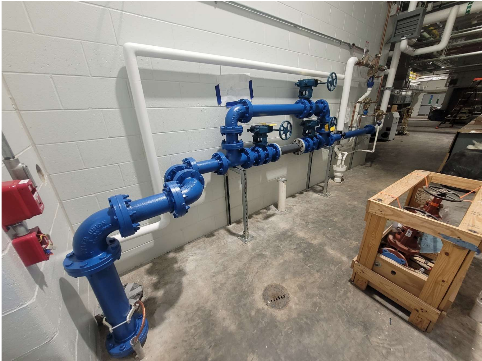
Completed Pipe Coatings
