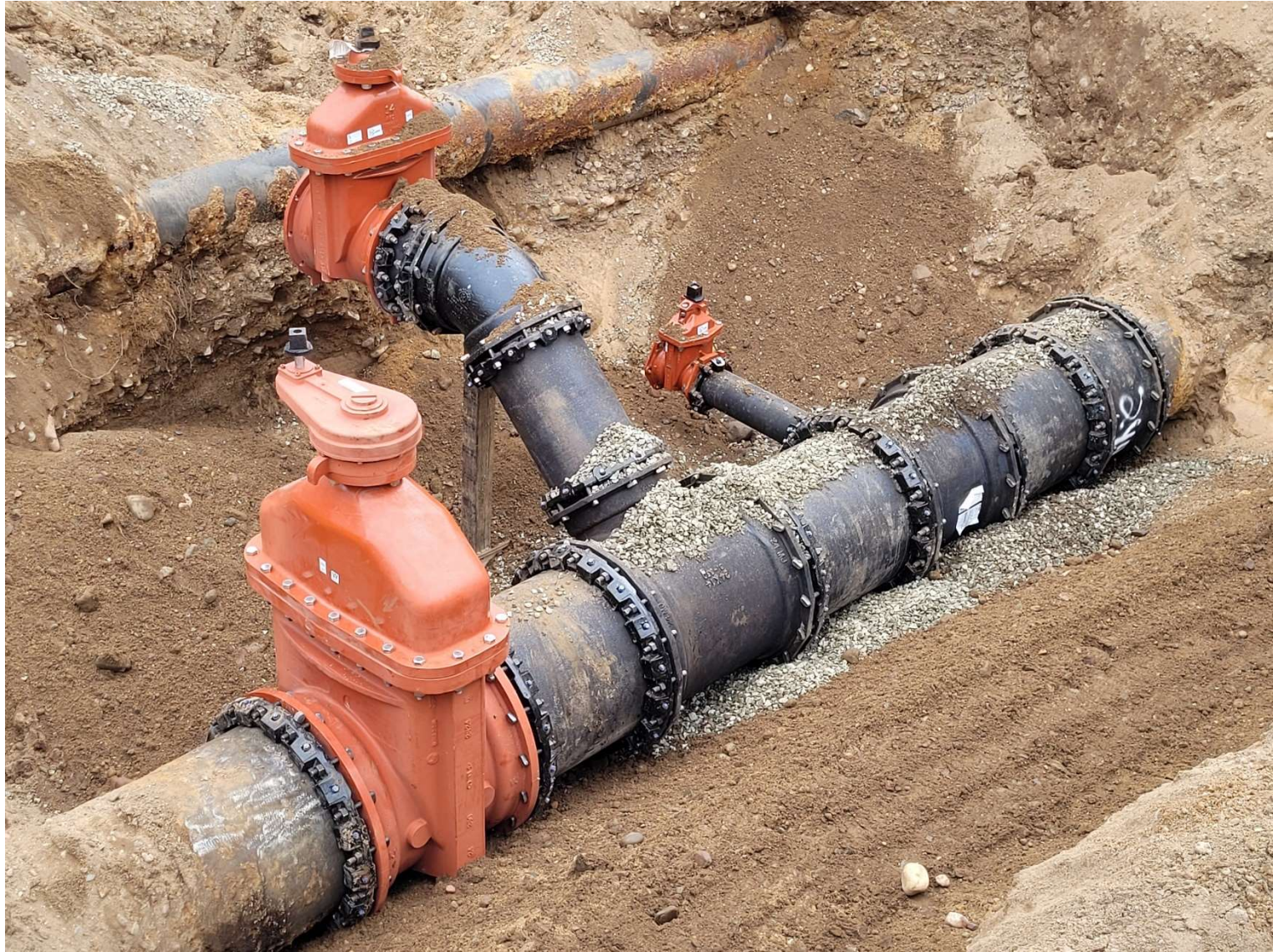
Water Main Connections at Schofield Park
