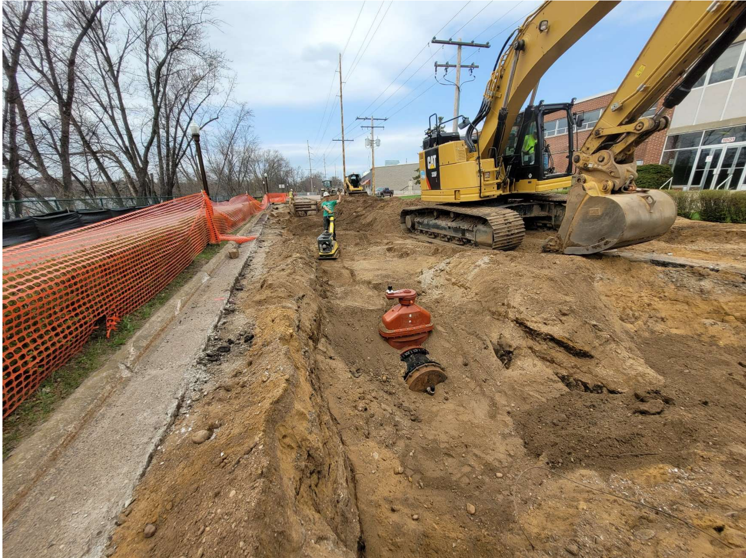
Water Main Installation at the Existing DWTF Site
