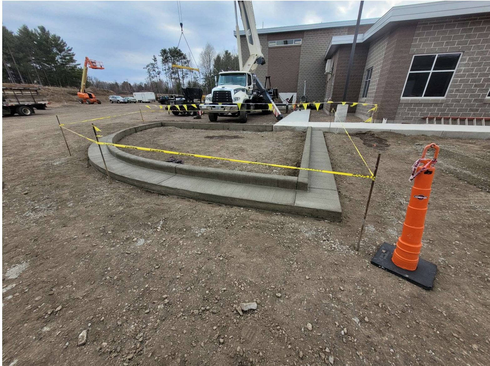
Curb and Gutter at the Administration Building
