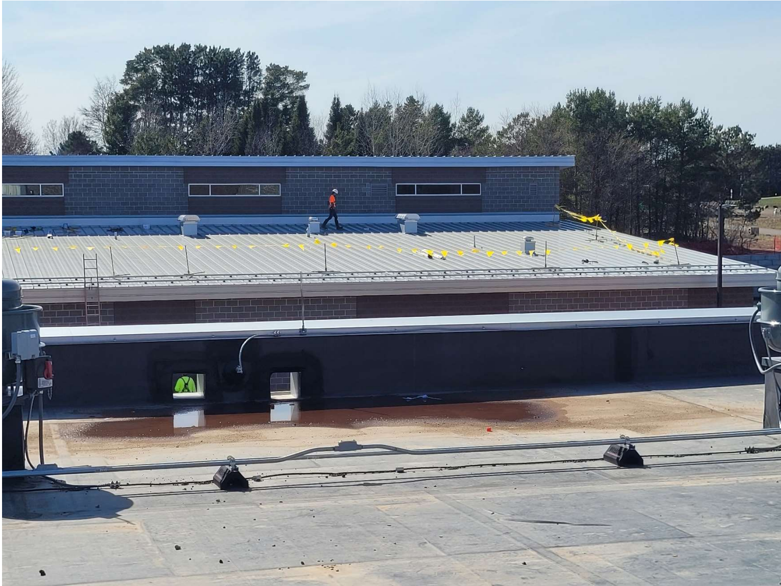
Administration Building Roofing
