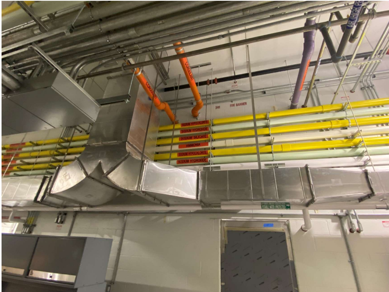
Interior Mechanical Work and Chemical Feed Lines
