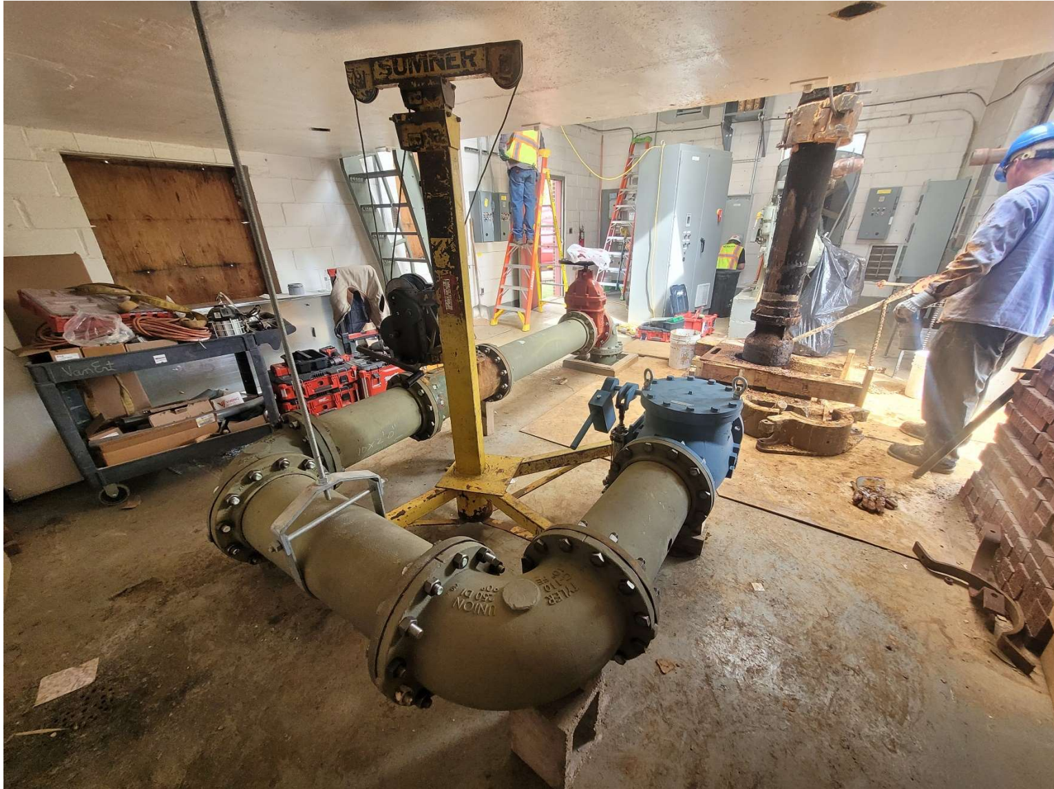
Well 6 Piping and Electrical Modifications
