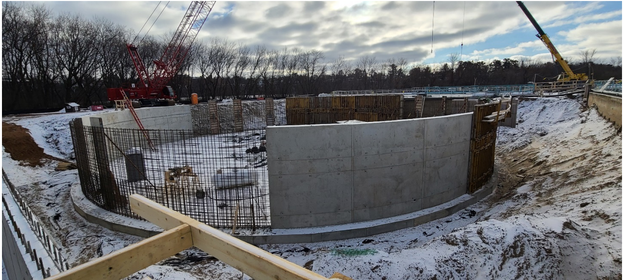
Walls of Structure 540 (Secondary Clarifier 4) being poured and formed in approximate 60 foot sections.
