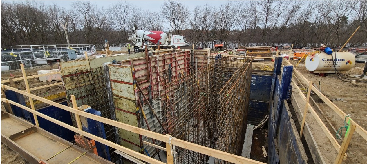
Miron and Wisconsin Rebar forming the Structure 500 (Secondary Splitter) tank walls.
