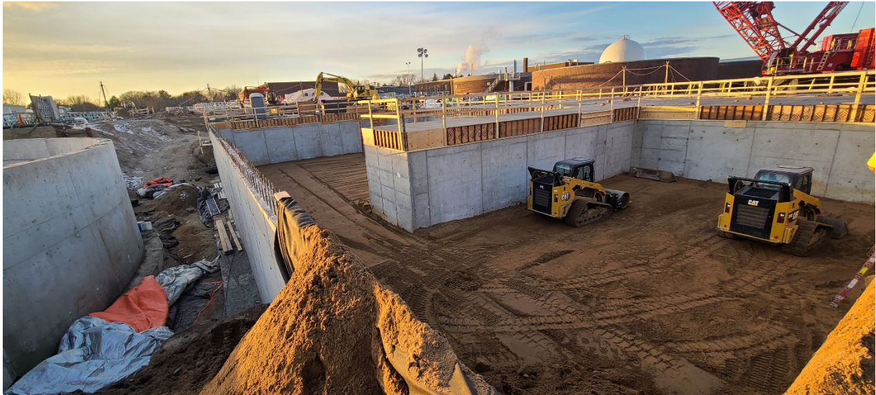
Structural backfill of the area below the southern portion of Structure 770 (Solids Building) slab on grade.
