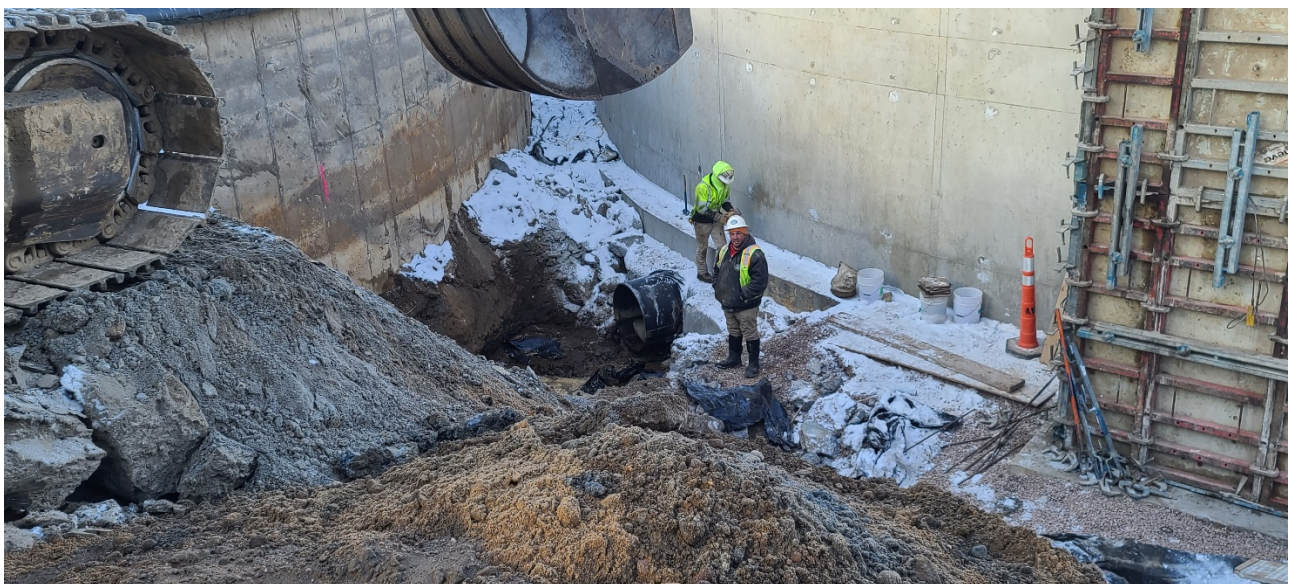
Integrity connecting the 36-inch Mixed Liquor line to Structure 540 (Secondary Clarifier 4).
