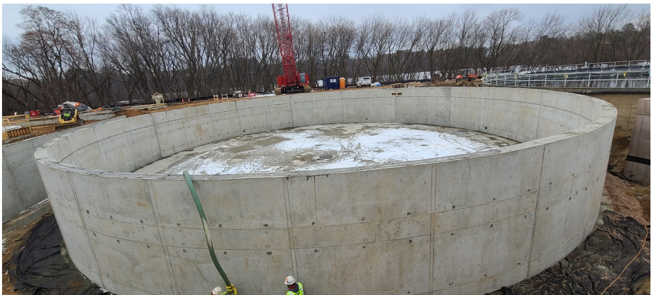
Miron beginning to fill Structure 540 (Secondary Clarifier 4) for a tank leakage test.
