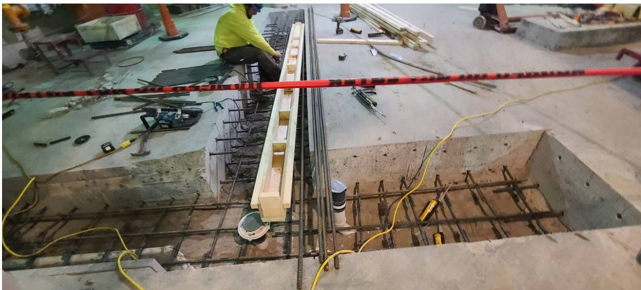
Concrete demolition work in lower level of Structure 700 (Digester Building) to allow for the connection of a trench drain to floor drain system.
