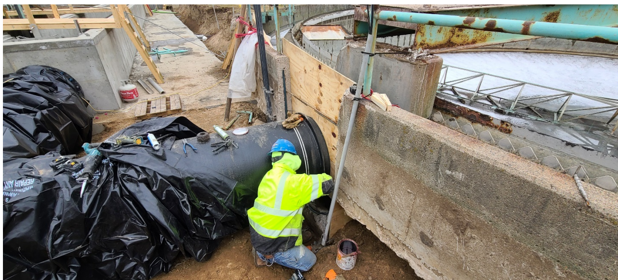
Final connection of Structure 350 (Primary Effluent Channel) to Structure 310 (Primary Clarifier 1).
