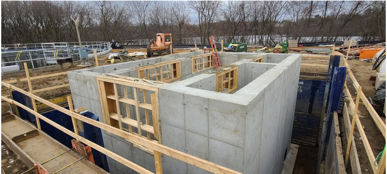
Forms removed from Structure 500 (Secondary Splitter) tank walls.
