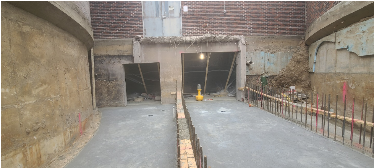
Openings in lower level of Structure 700 (Digester Building) provide access ground level and Tunnel 910.
