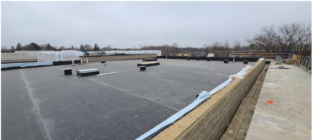
Placement of the membrane roof on top of Structure 120 (Administration Building).
