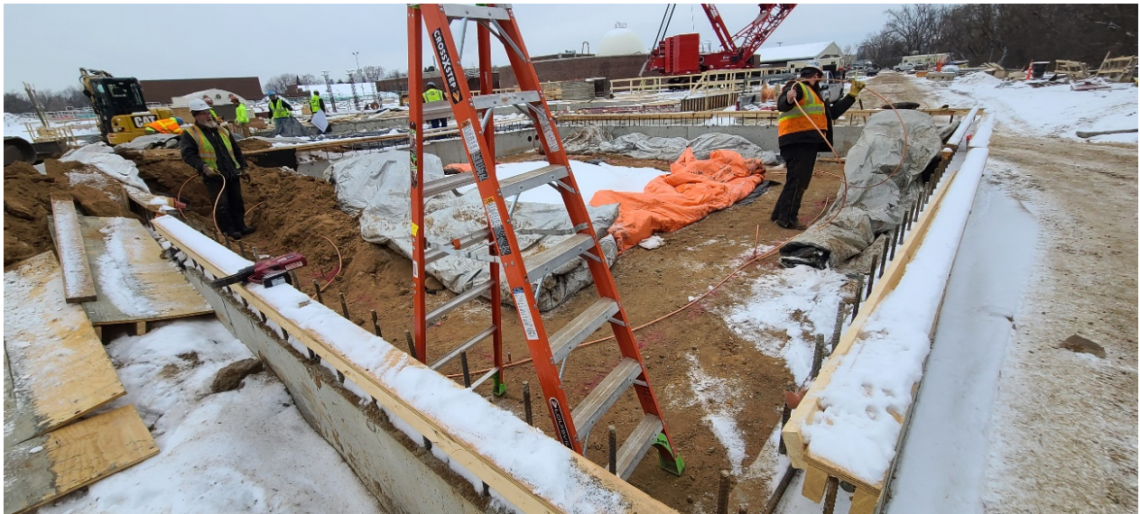
Van Ert Electric placing grounding below the floor slab for the solids collection bins in the southeast corner of Structure 770 (Solids Building).
