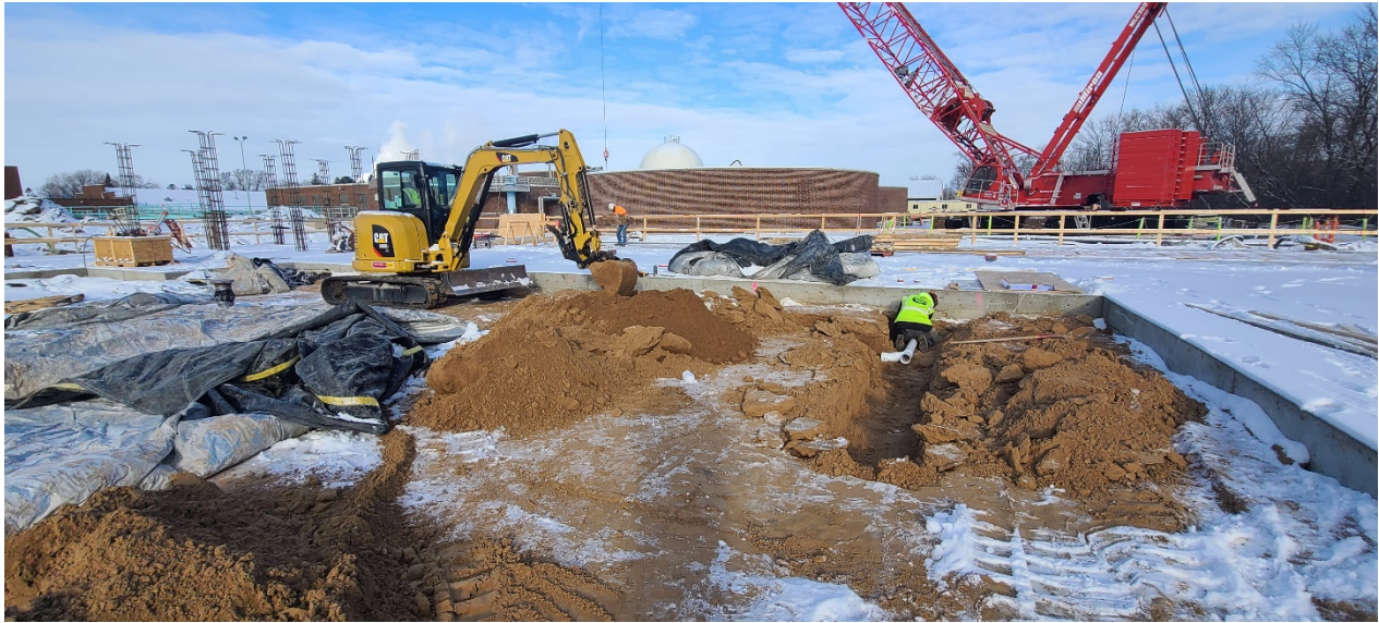
August Winters and Sons placing floor drains below the southern slab for Structure 770 (Solids Building).
