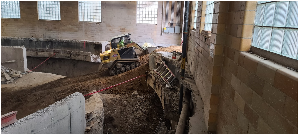
Structure 100 (Main Building): Demolition old clarifier tank in the Gravity Thickener area continues. A hole has been cut in the wall of the structure to allow easy access and removal of debris.
