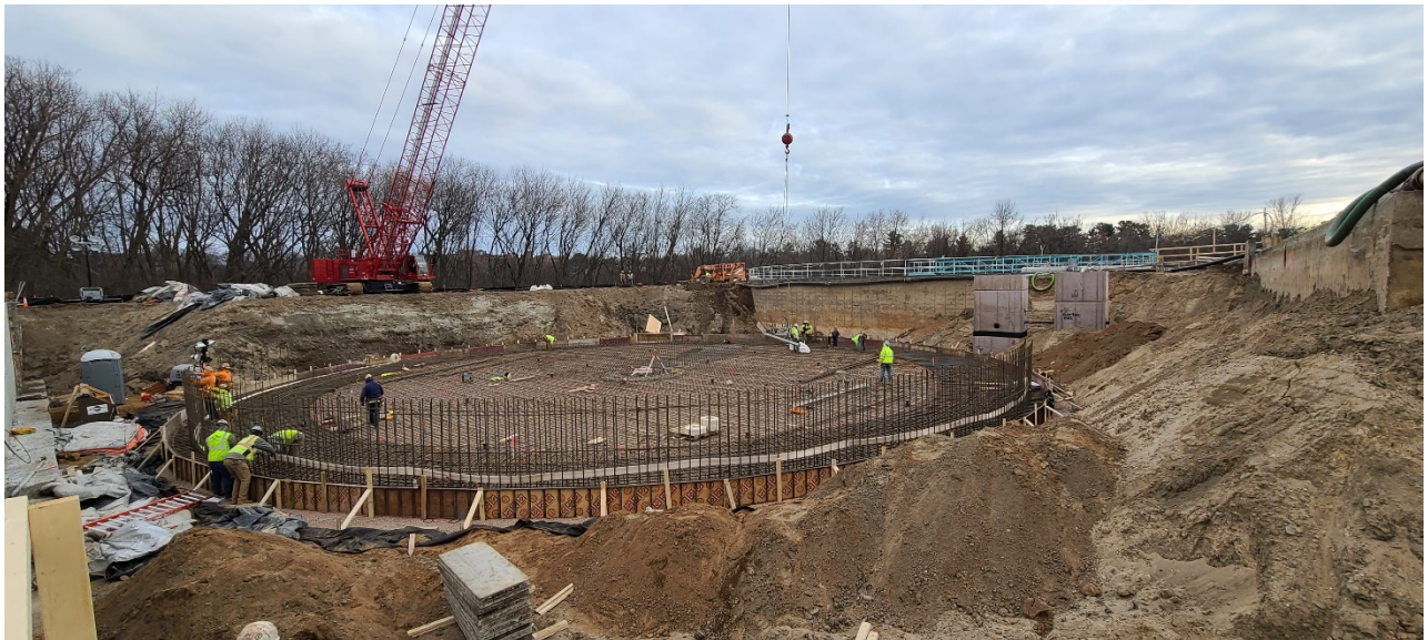
Structure 540 (Secondary Clarifier 4): slab and tank wall rebar and formwork in process.
