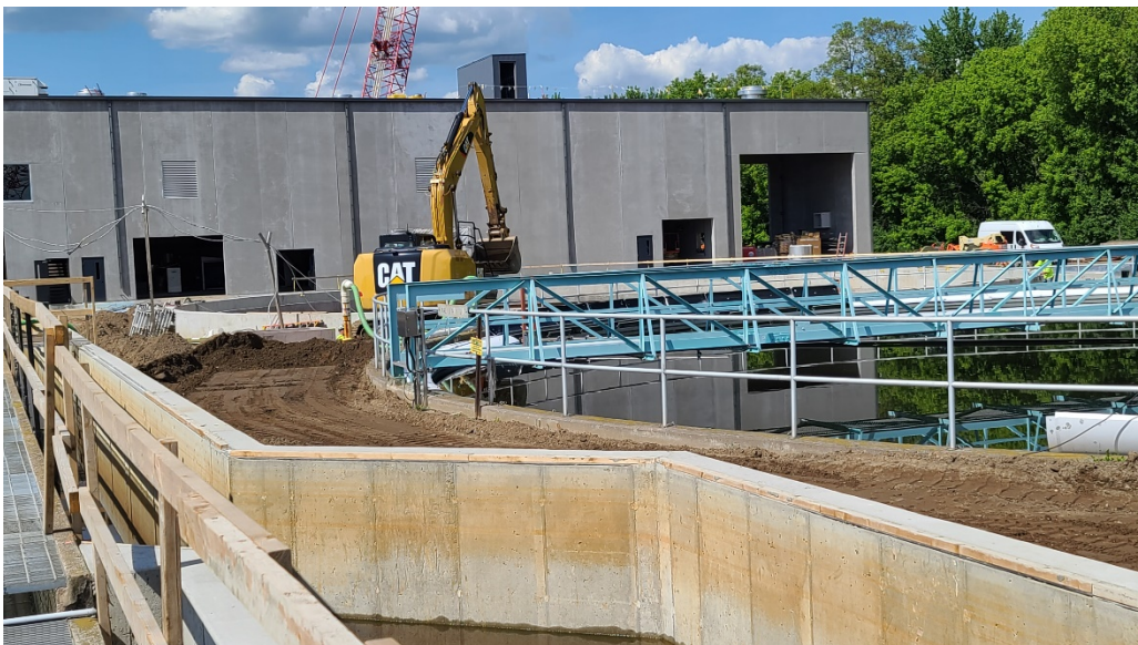
Backfill and grading along the east side of the Structure 420 (Mixed Liquor Channel).
