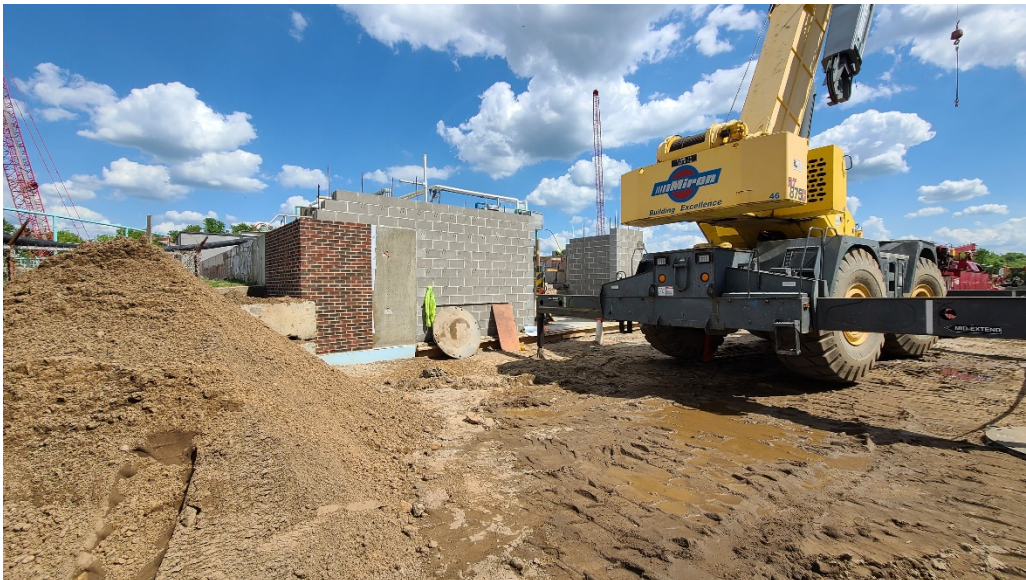
West extension of Structure 200 (Grit Building), new concrete masonry unit wall with the start of brickwork.
