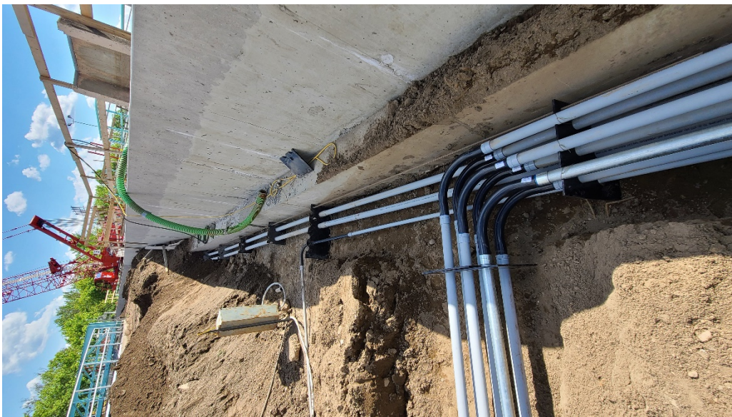
Duct Bank O being placed along the east side of Structure 420 (Mixed Liquor Channel).
