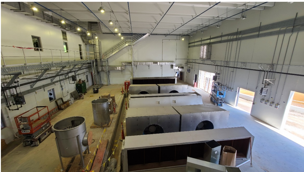
New dryer components set on pad, catwalk to Mechanical Room in the Dryer Room of Structure 770 (Solids Building).
