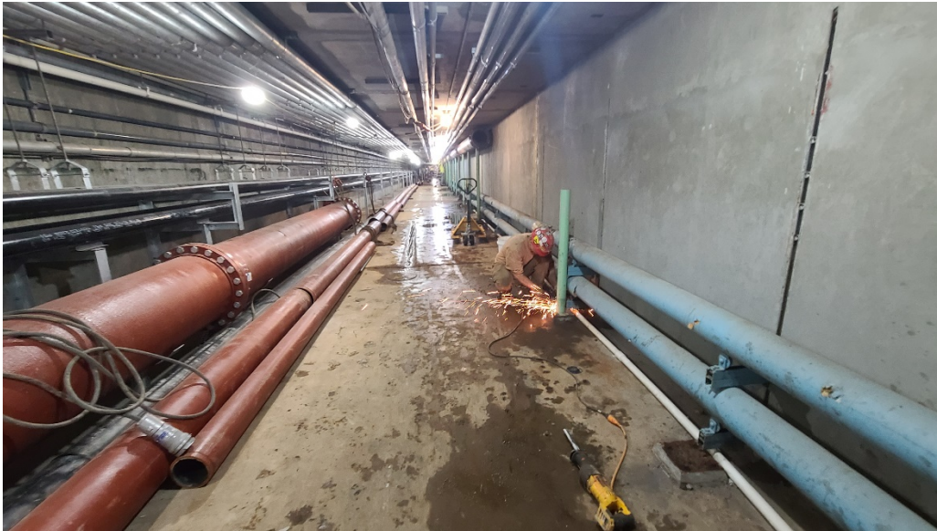
Looking north, new pipe racks and piping being placed along west wall (left side of photo) of Tunnel 900. Demolition of existing piping along the east wall (right side of photo).
