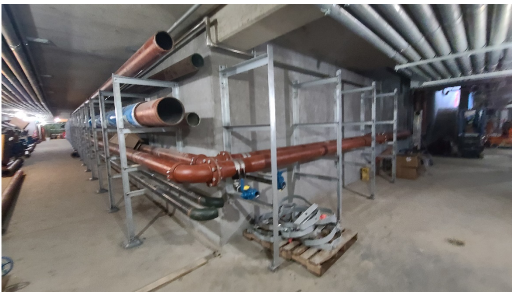
Looking north and east at south end of tunnel, starting piping tie-ins.
