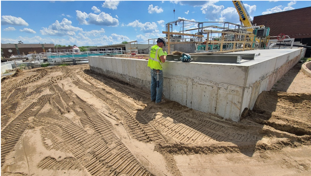
East side of Structure 200 (Grit Building), showing new concrete work around influent gates and new grade floor for electrical room.
