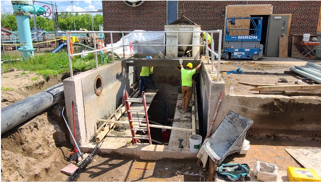
Pouring channel slab foundation walls at Structure 406 (Mixing Tank).
