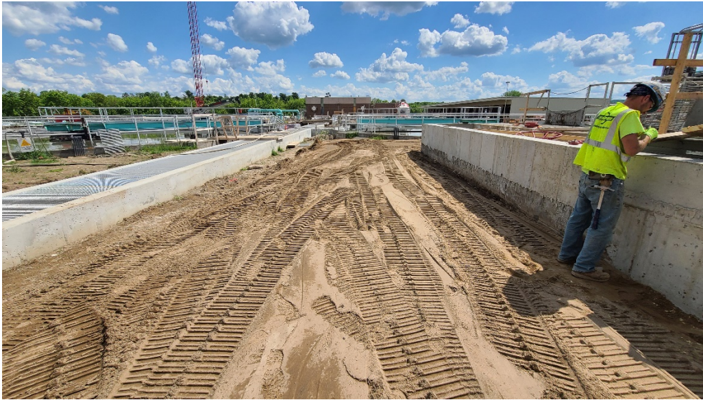
Fill and grade work between Structure 200 (Grit Building) and the west side of the Structure 350 (Primary Effluent Channel).
