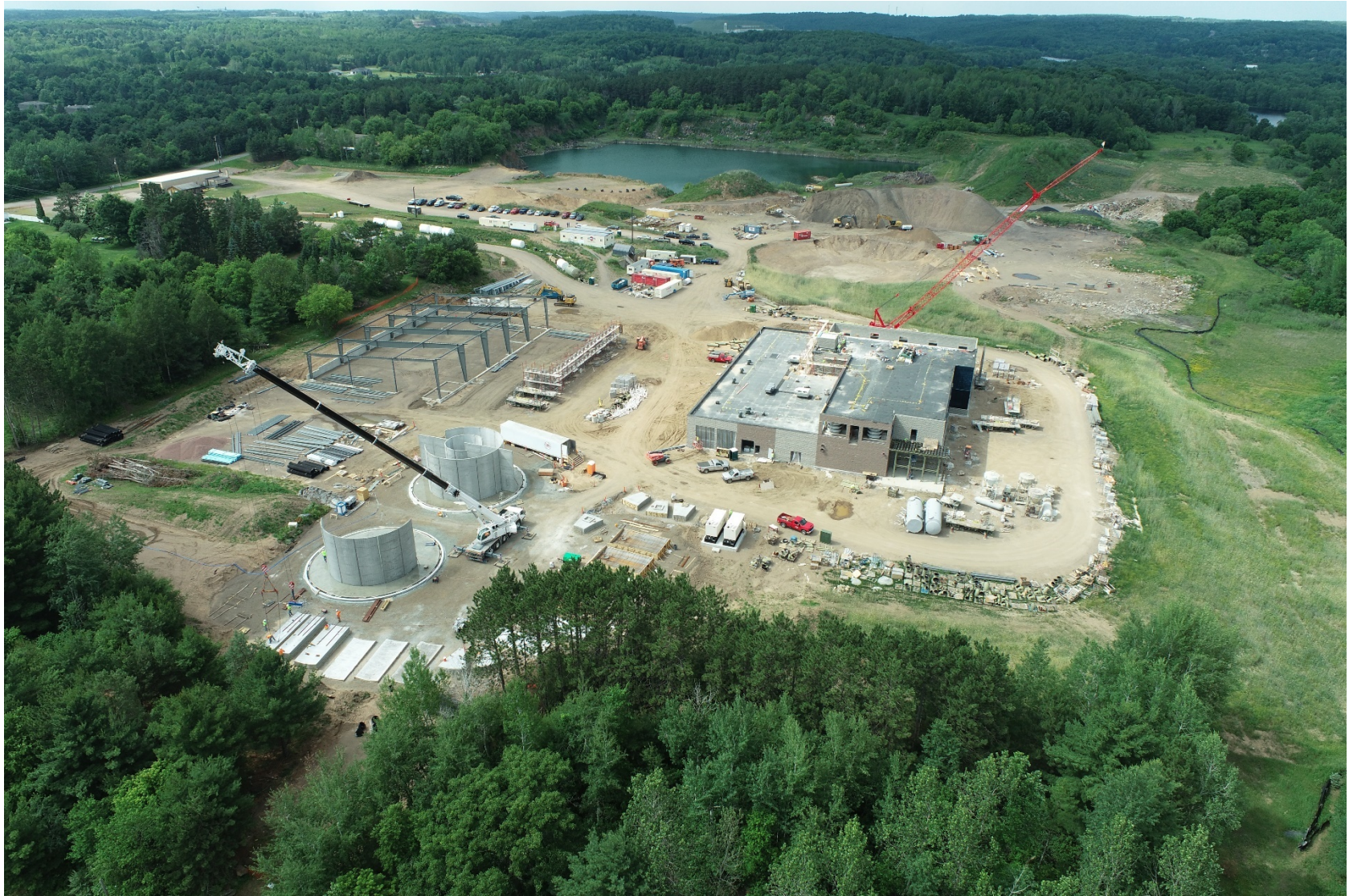
Overall Site Looking North
