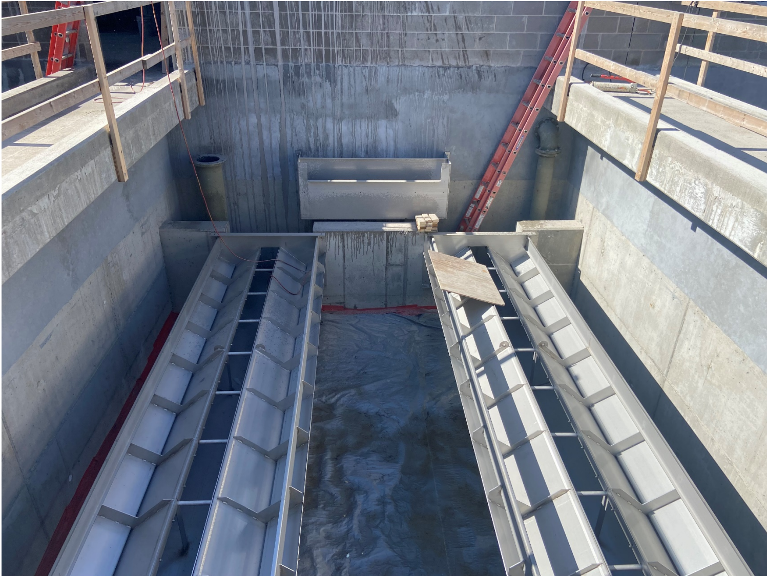
Filter Troughs and Wier Installed
