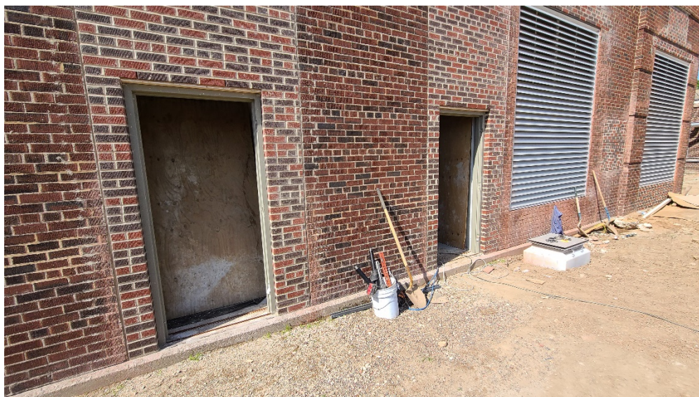
Southside of Structure 100 (Main Building), new door frames and generator louvers.
