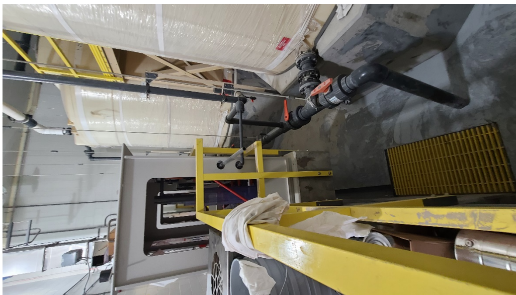
Chemical feed skids set and piping from skids being installed.
