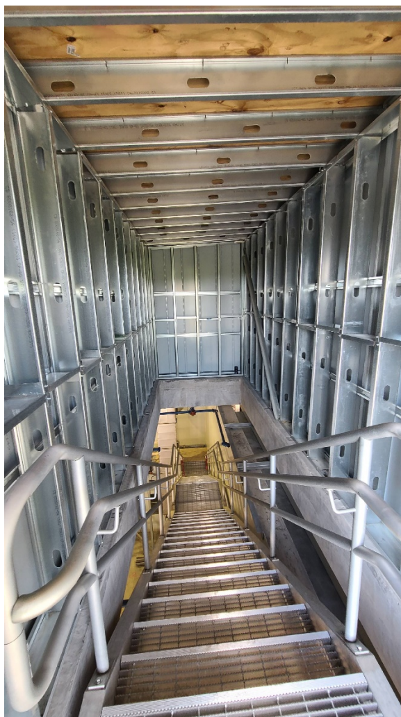
Looking down the stairway from Structure 770 (Solids Building) roof doghouse to the dryer room catwalk.
