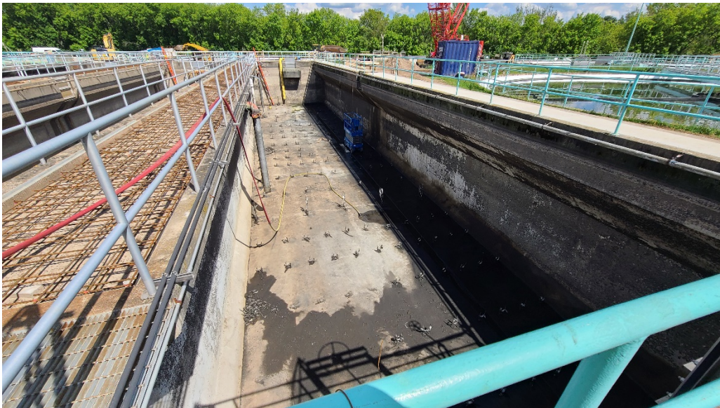
Aeration basin 6, cleaned, aeration header piping demolished and infill walkway (left) filled and being prepped for concrete walkway.
