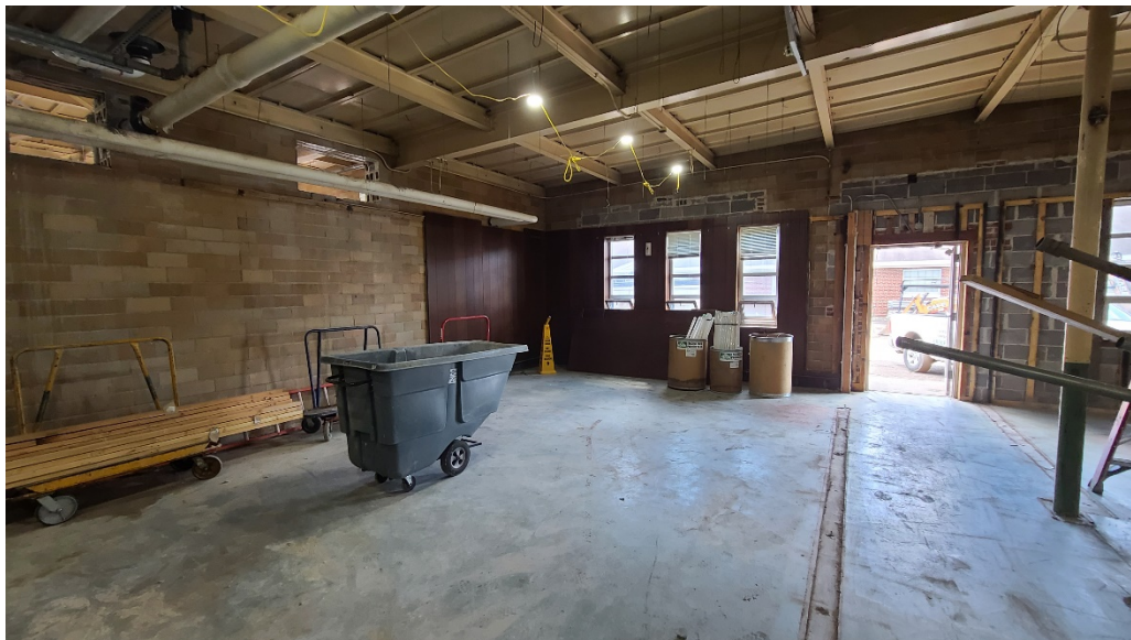
Demolition work within the old offices, lunch room, bathroom area.
