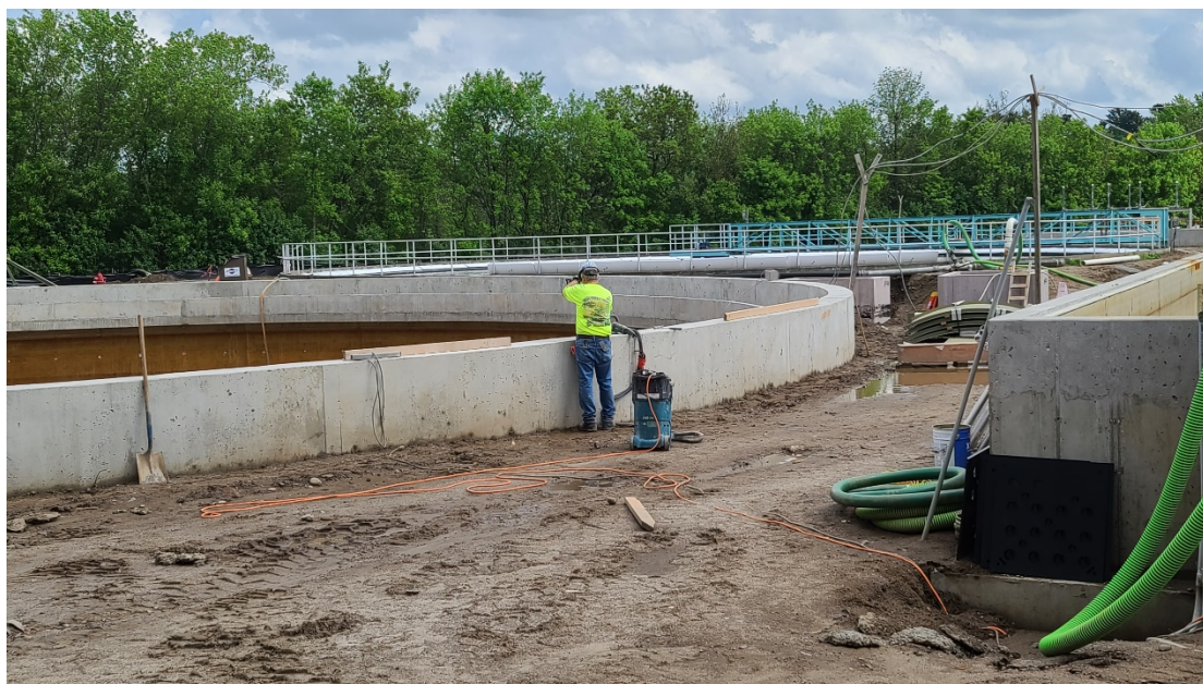
Concrete finish work on Structure 540 (Secondary Clarifier 4) launder.
