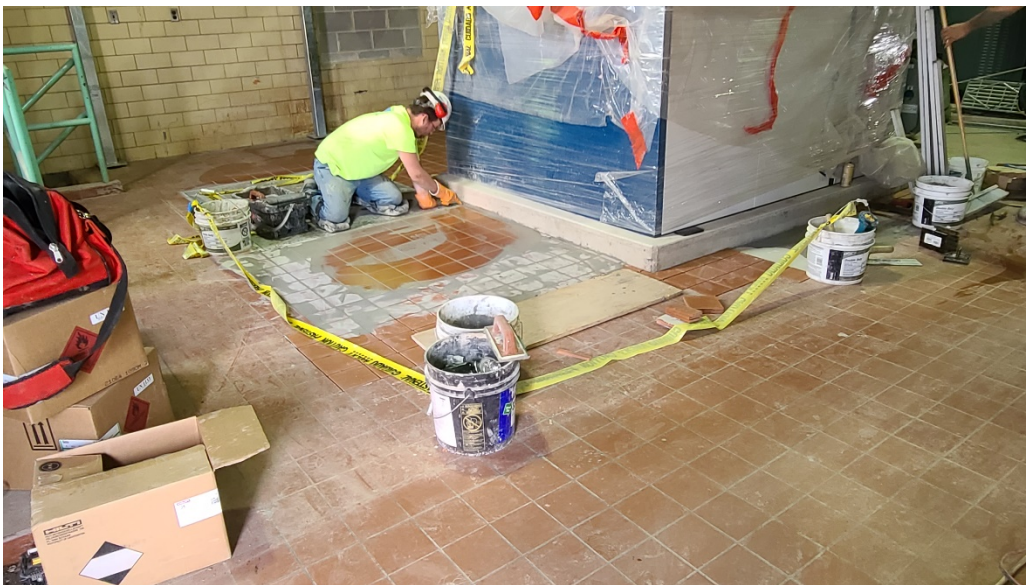
Tile work around new blower and new hatch.
