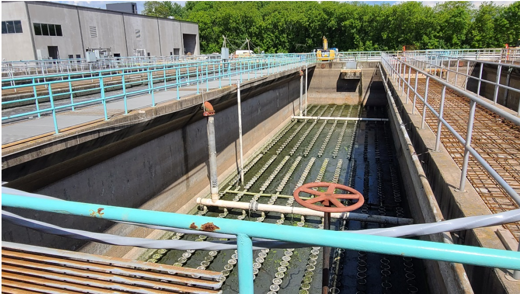
Aeration basin 5, pumped down, waiting to be cleaned for piping demo work.
