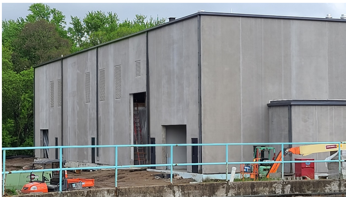
New gutters, roof trim and downspouts on north side of Structure 770 (Solids Building).
