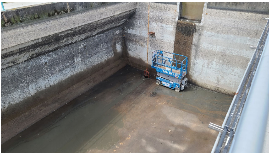
West gate removed from Activated Sludge Basin 6.
