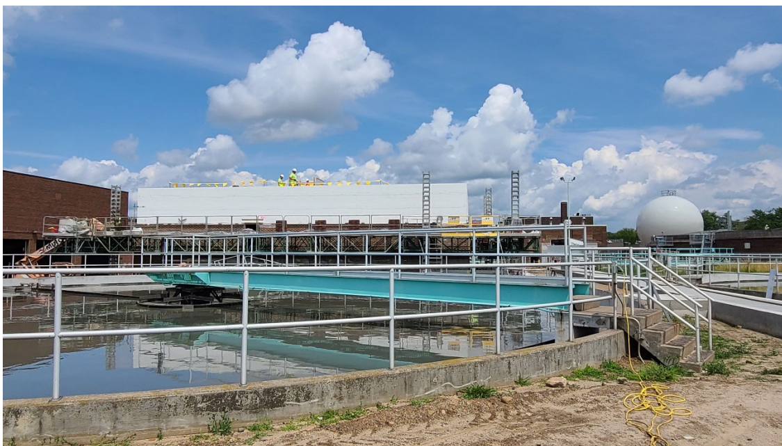
Roof penetrations and HVAC work started Structure 200 (Grit Building)
