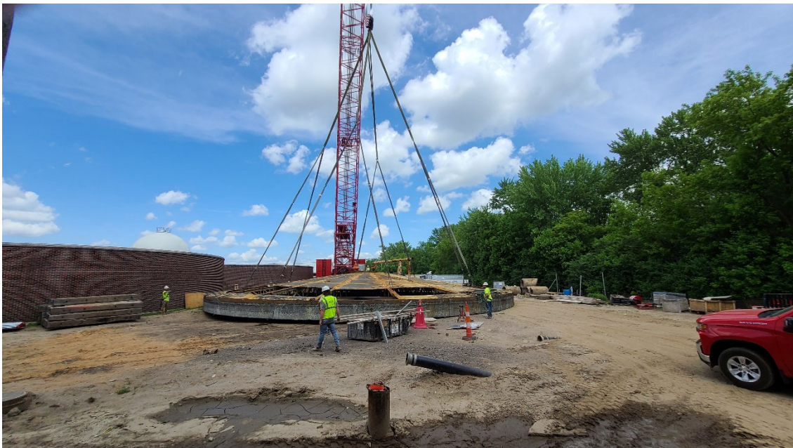
Removal of Structure 720 (Digester 2) roof.
