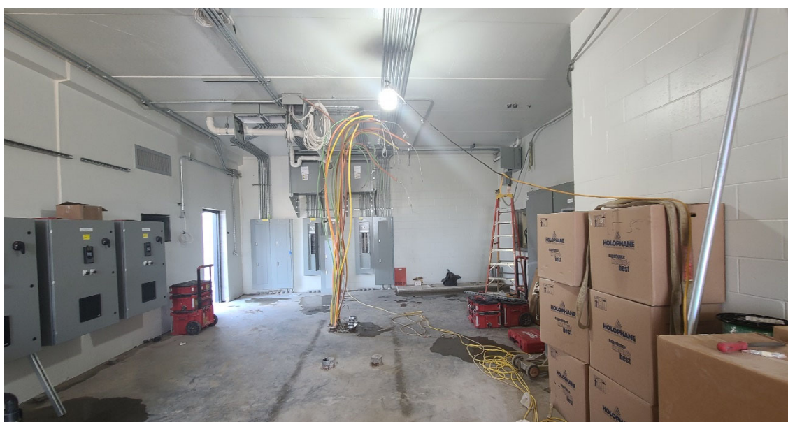
Electrical room of Structure 770 (Solids Building) with switchgear pad layout, new VFDs hung and main feed lines pulled.
