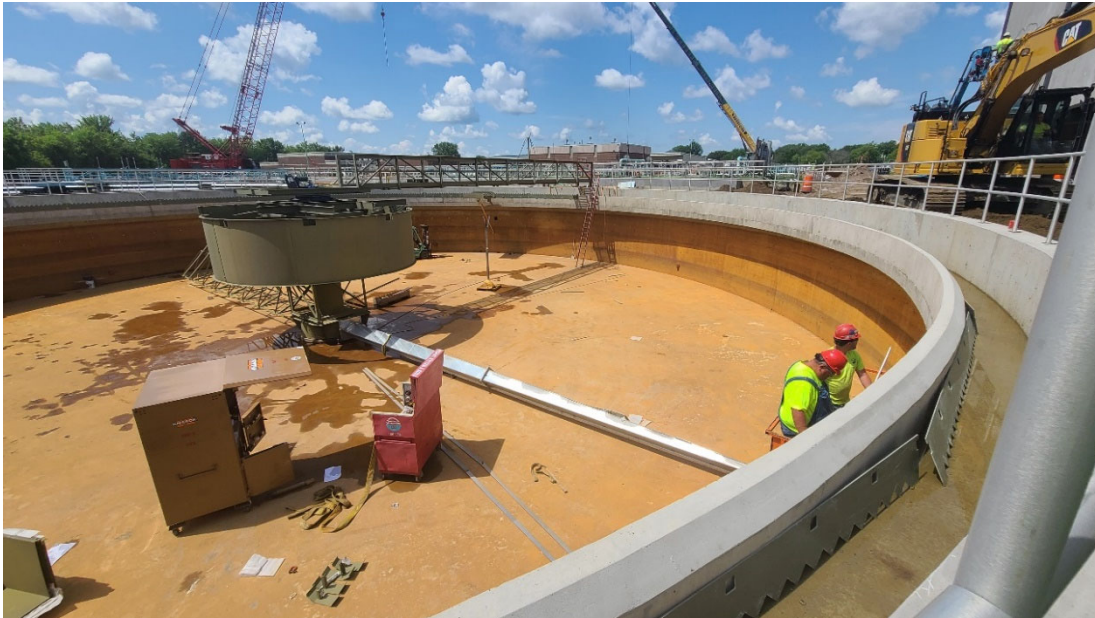
August Winters starting on placement of internals of the clarifier as well as the weir plates for the trough at Structure 540 (Secondary Clarifier 4).
