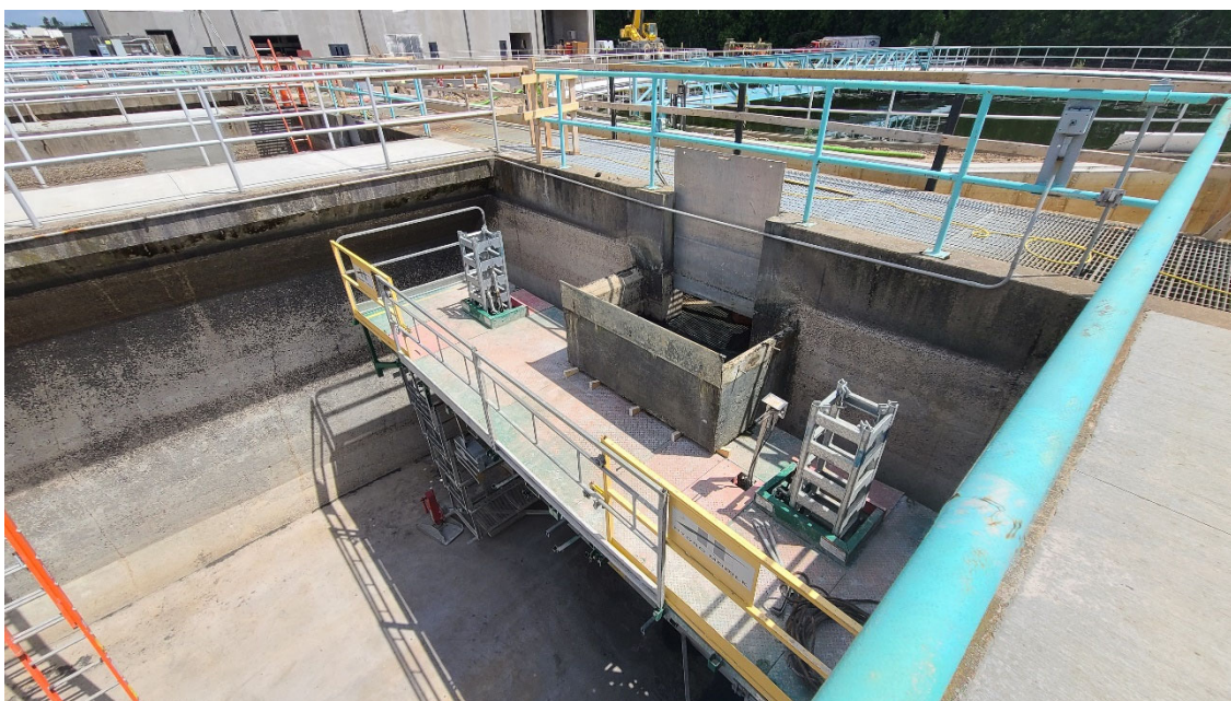
East weir being prepared for removal on Activated Sludge Basin 6.
