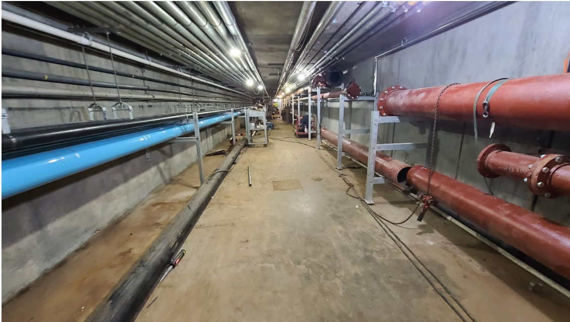
Looking north, new pipe racks and piping being placed along east wall (right) of Tunnel 900.
