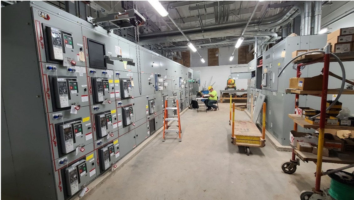
Van Ert Electric getting the new switchgear ready in Structure 100 (Main Building)
