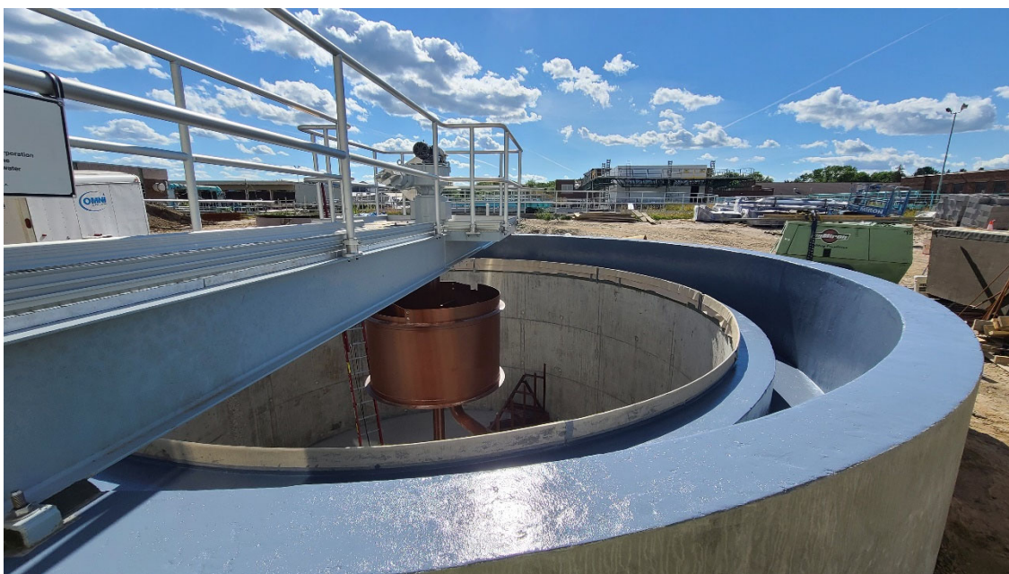
Structure 775 (PSD Thickener) internal mechanical equipment set and equipment access walkway placed.
