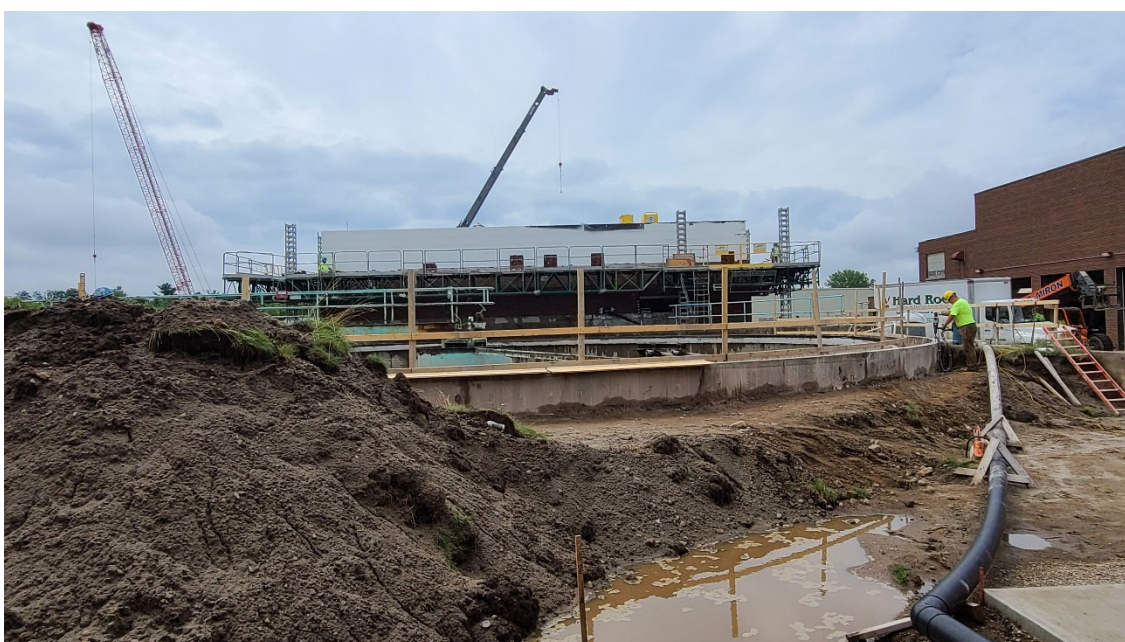
Structure 310 (Primary Clarifier 1) has had hand rail removed and the top foot of the tank removed.
