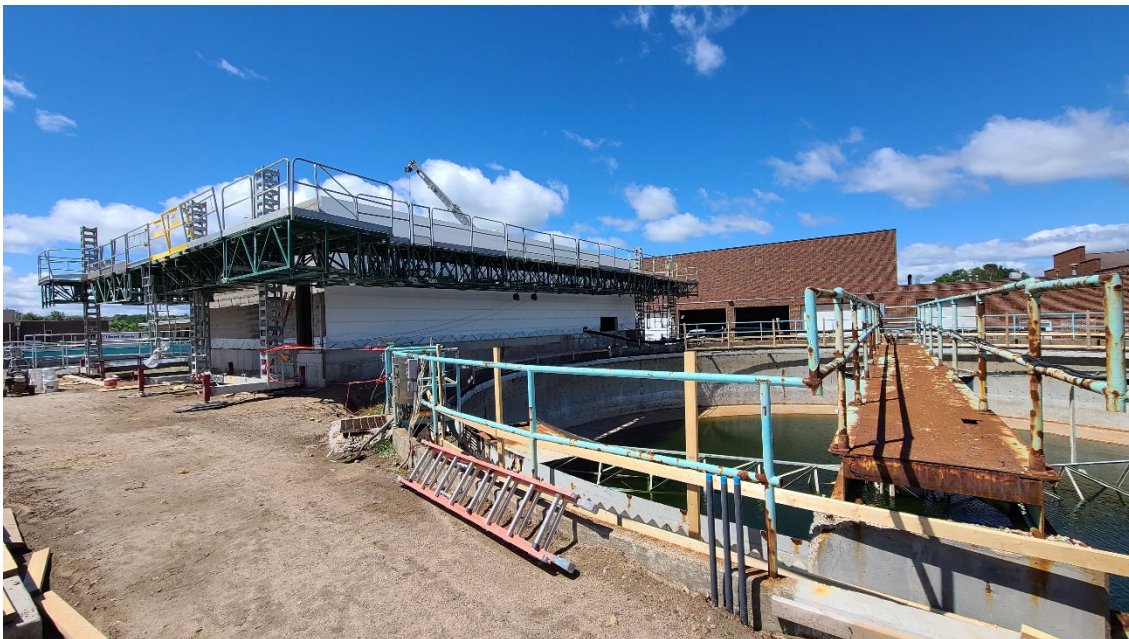
West extension of Structure 200 (Grit Building): new concrete masonry unit (CMU) wall with the start of brick work.
