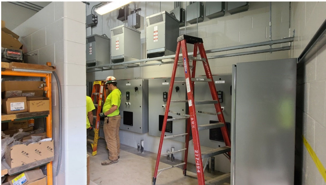
Van Ert Electric installing the new VFDs and harmonic filters in the Structure 610 (Chemical Building) electrical room.
