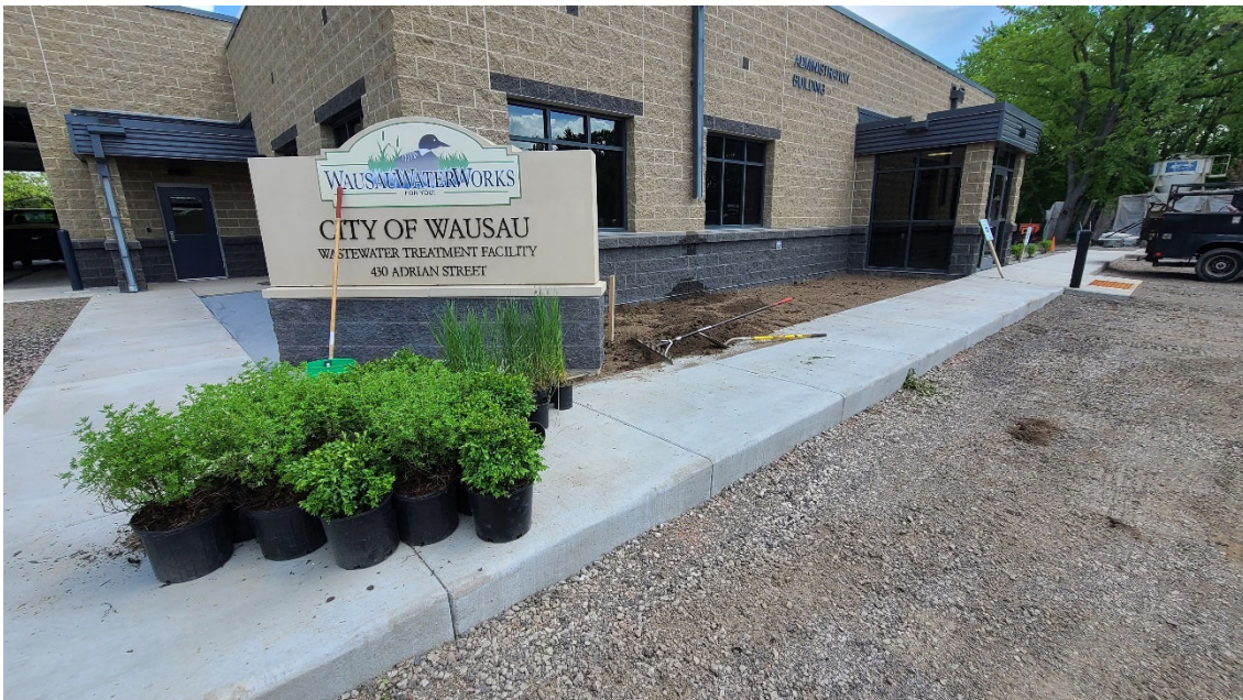
Front walkway and landscaping at Structure 120 (Administration Building).
