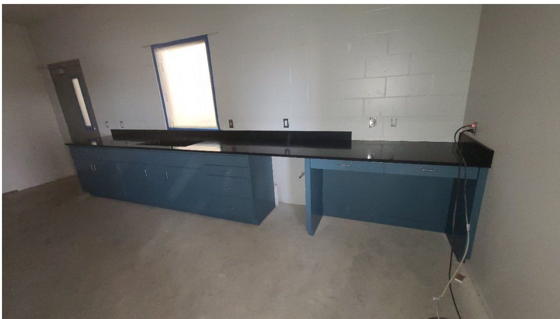
New control room area lab case work set in Structure 770 (Solis Building).
