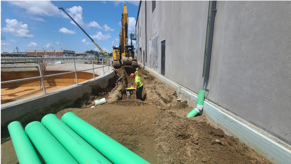
Storm water installation between Structure 540 (Secondary Clarifier 4) and Structure 770 (Solids Building).
