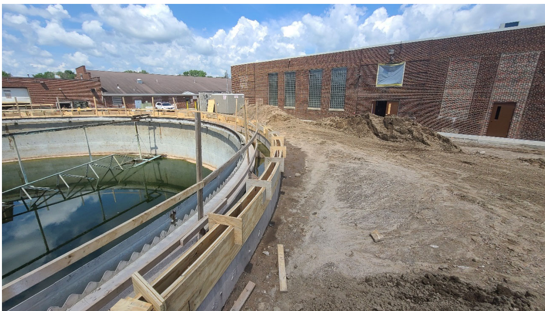
Formwork in place to pour new top for Structure 310 (Primary Clarifier 1).
