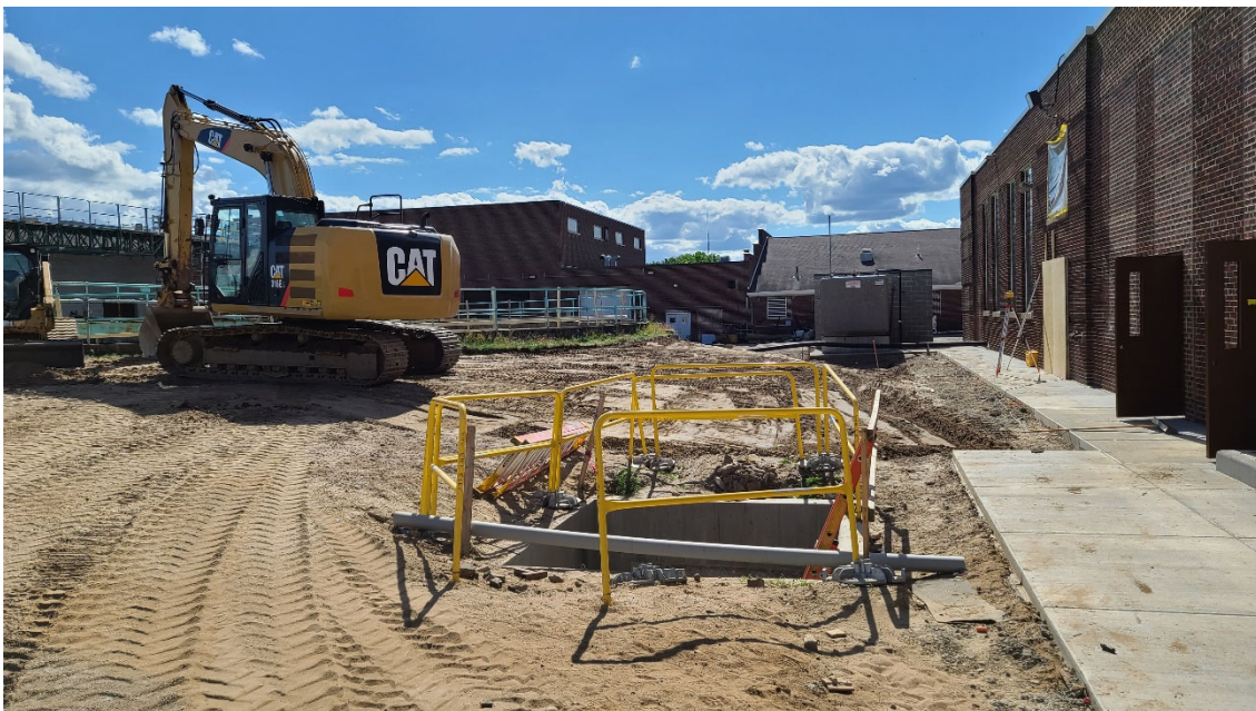
New sidewalk and exterior doors south side of Structure 100 (Main Building and the start of grading between Structure 100, Structure 105 (Standby Fuel Tank) and Structure 310 (Primary Clarifier 1).
