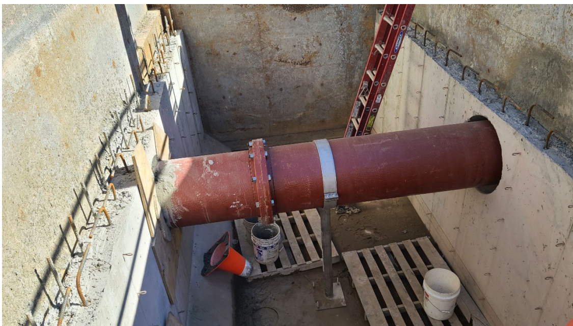
Return activated sludge piping from Tunnel 900 placed below eventual new channel slab.
