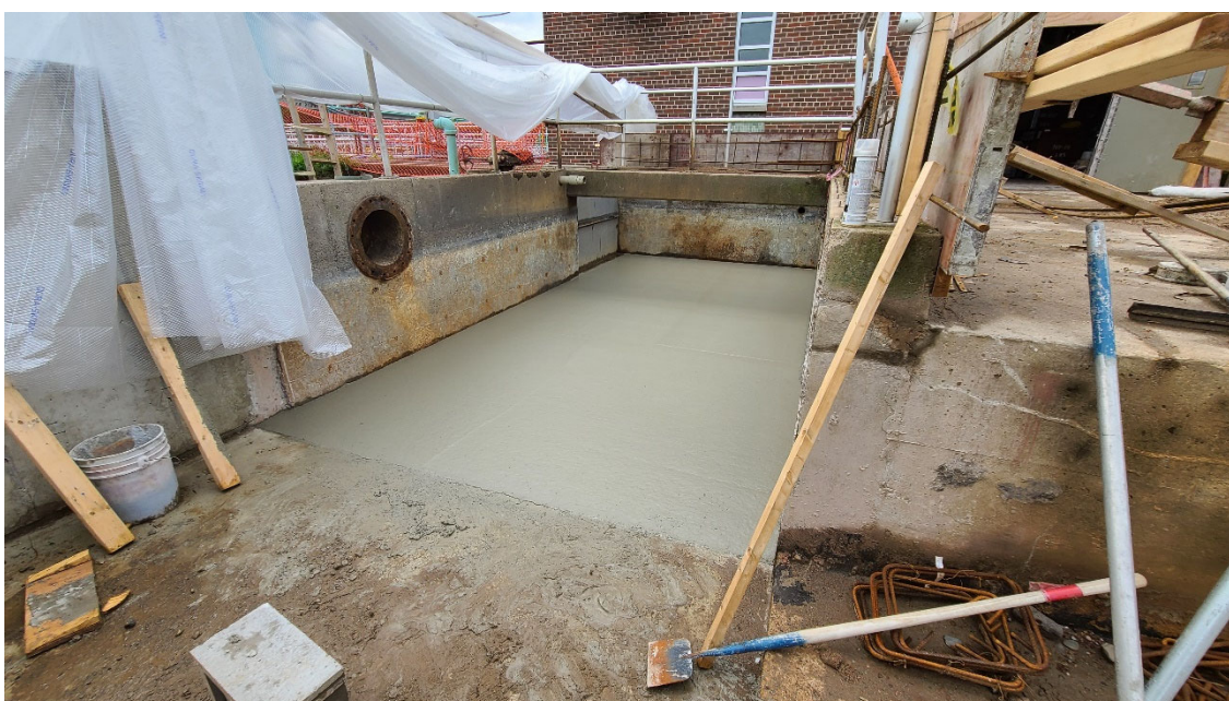
New channel slab placed to eventually tie Structure 405 (Anoxic Selector Tank) to Structure 410 (Activated Sludge Basins).
