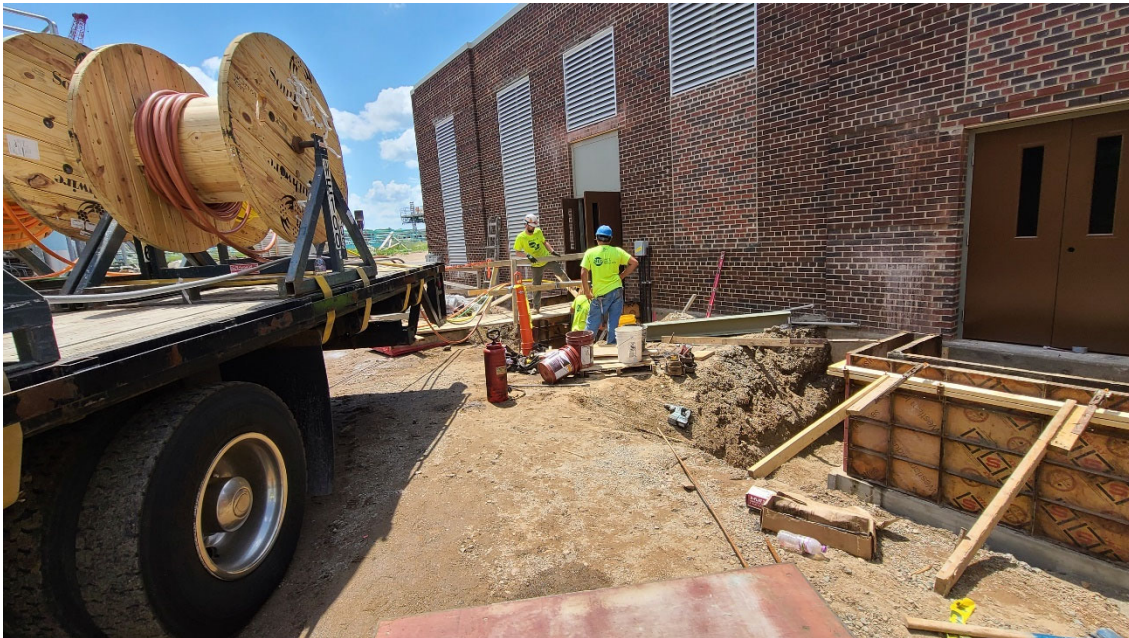
Van Ert Electric pulling main wire into electric manhole 2, stoop work for east doorways also in progress
