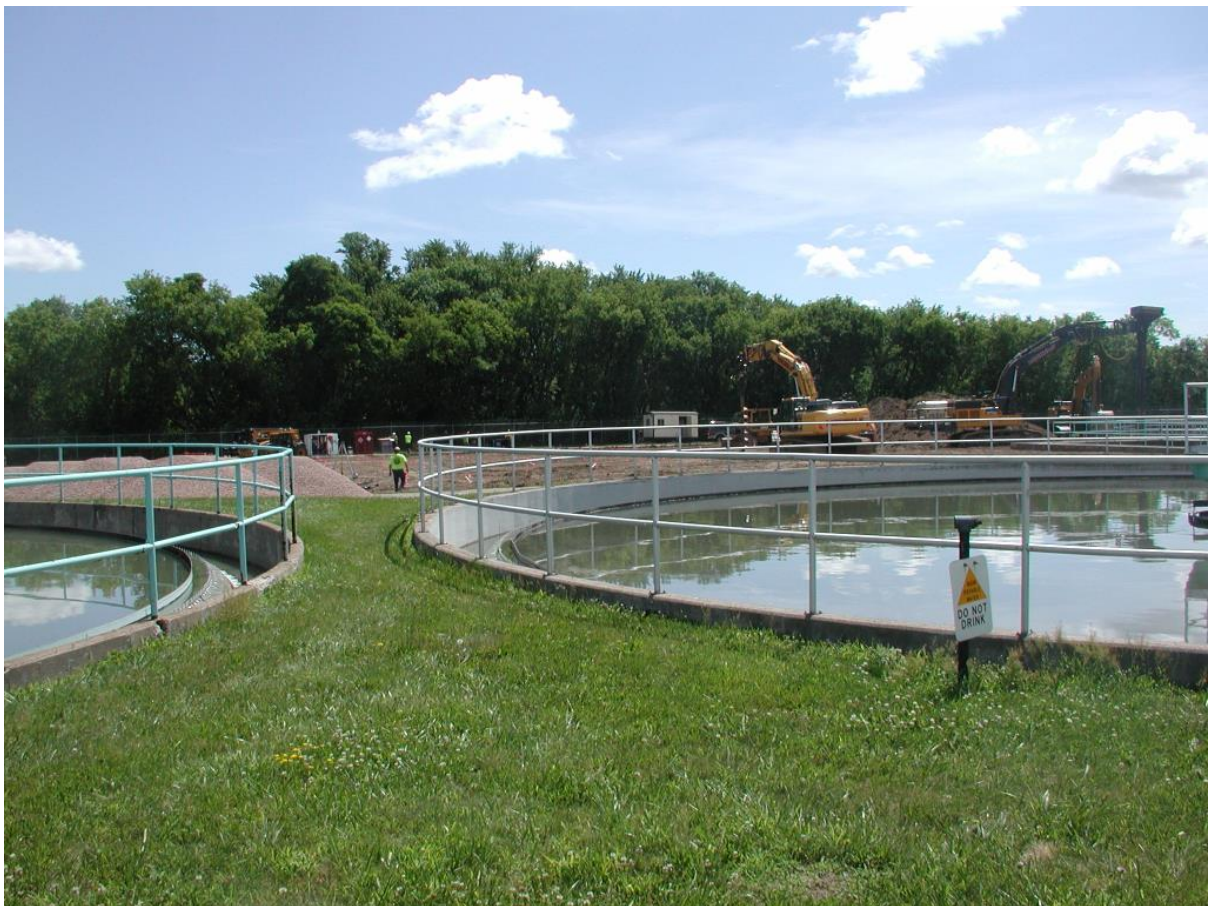
Photo 8: Construction of new sludge handling facility, primary clarifiers in the foreground
