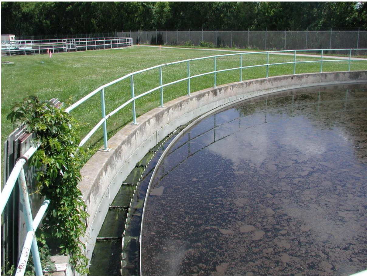
Photo 17: South eastern secondary clarifier
