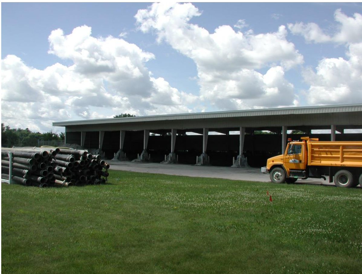
Photo 13: Biosolids storage facility
