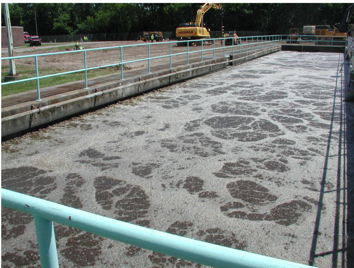
Photo 12: Northernmost aeration basin
