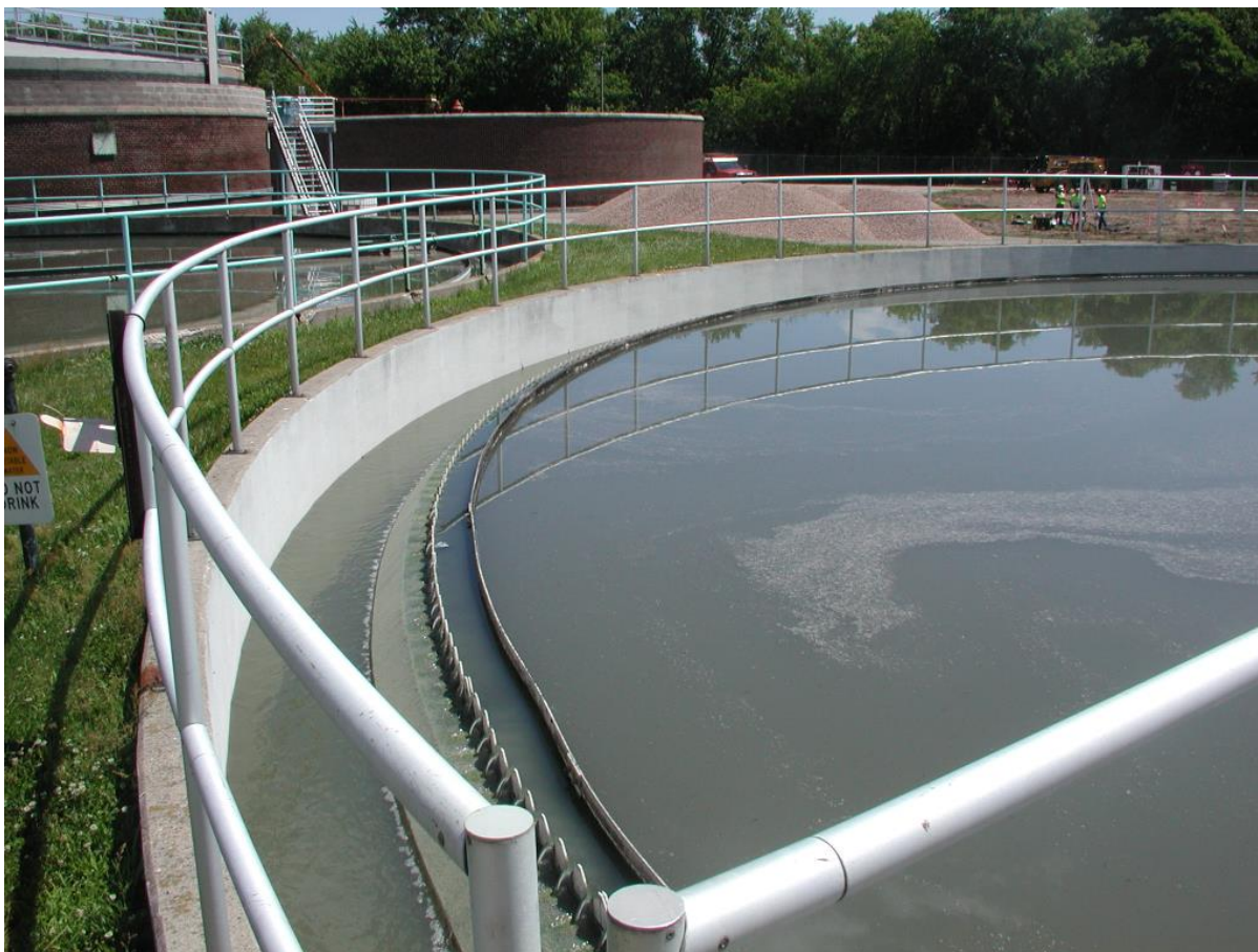
Photo 11: Easternmost clarifiers (South looking North)
