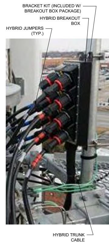
4 TYPICAL MOUNTING DETAILS N.T.S.
