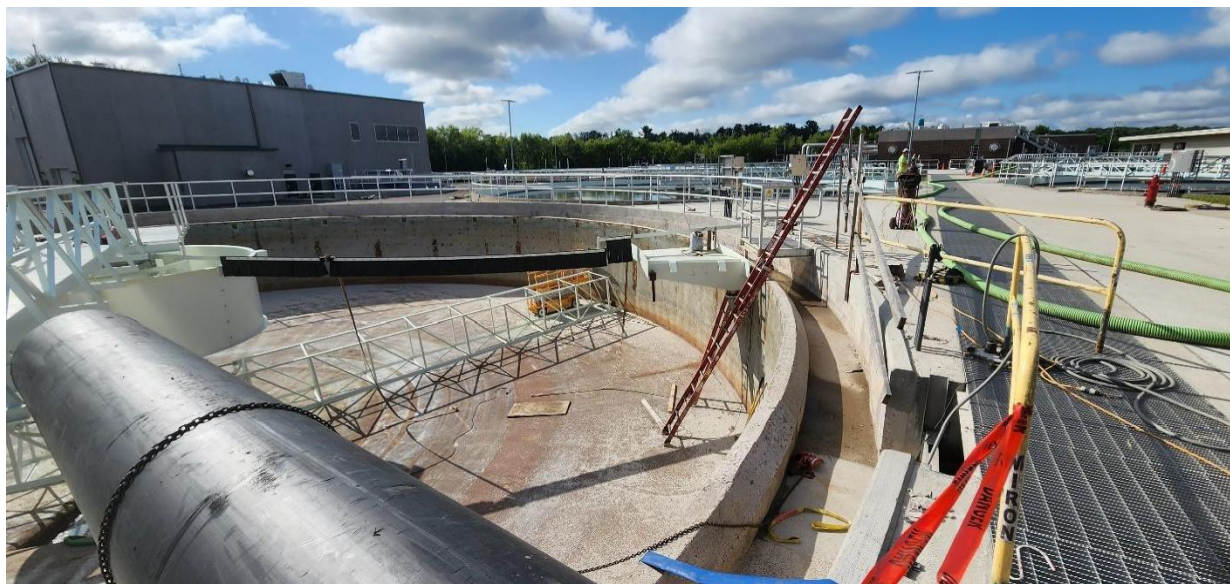
Installation of the new mechanism for Structure 320 (Primary Clarifier 2).
