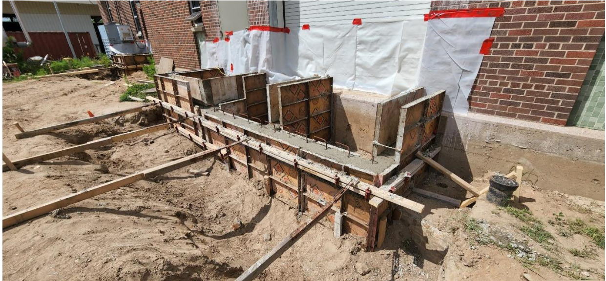
New stoops ready for concrete on south side of Structure 400 (Activated Sludge Building).
