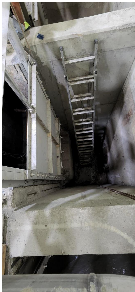
New Structure 320 (Primary Clarifier 2) influent gate installed.
