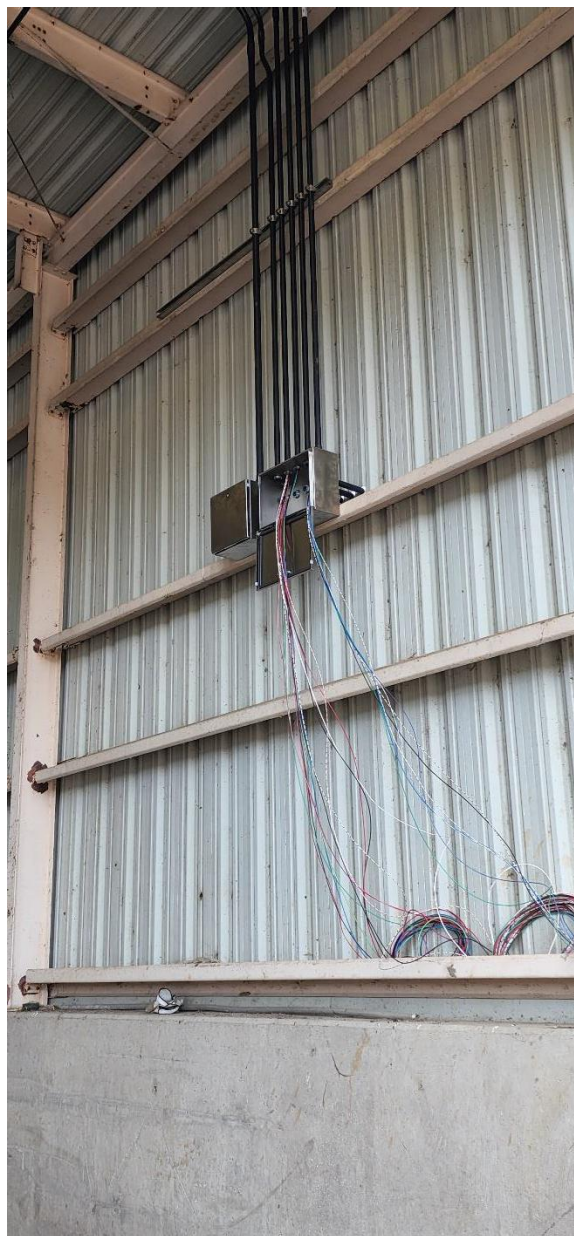
Start of conduit and junction boxes for control panel installation in the north bay Structure 760 (Biosolids Storage Building).
