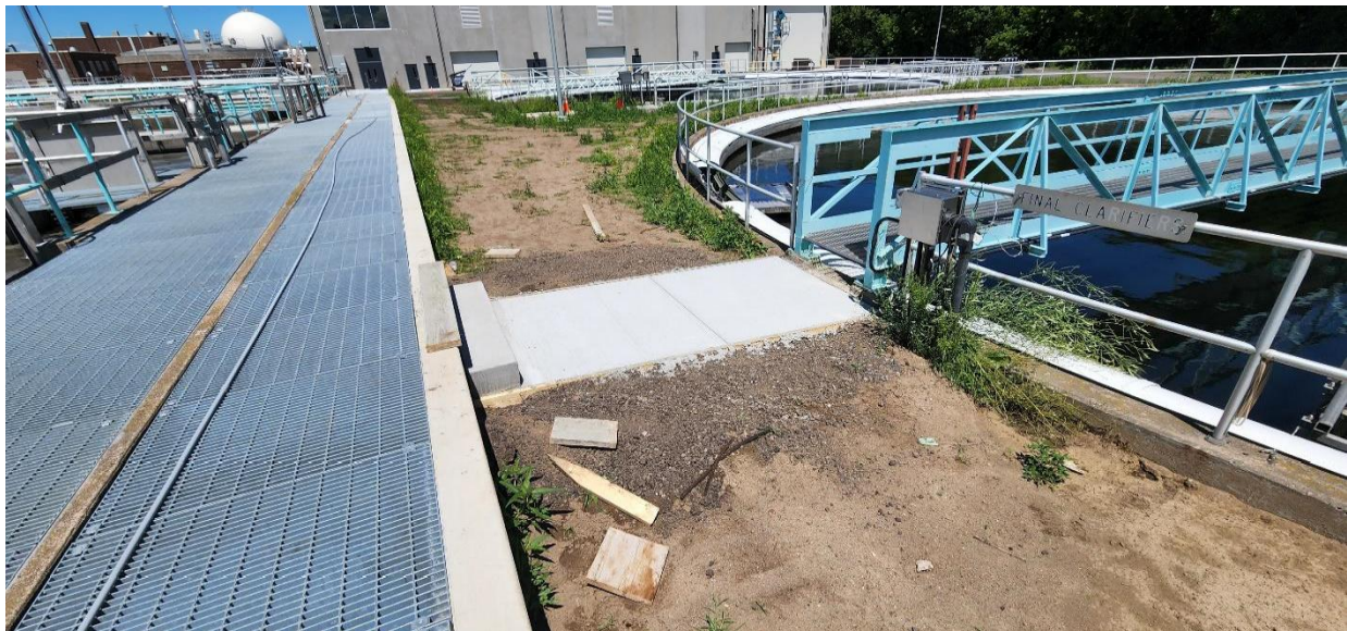
New concrete sidewalk between Structure 530 (Secondary Digester 2) and Structure 420 (Mixed Liquor Channel).
