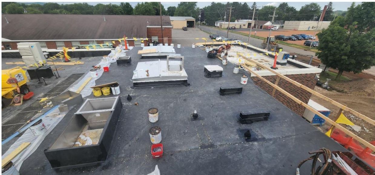
New roof membrane and topside view of new raw wastewater pump room access hatches of Structure 100 (Main Building).
