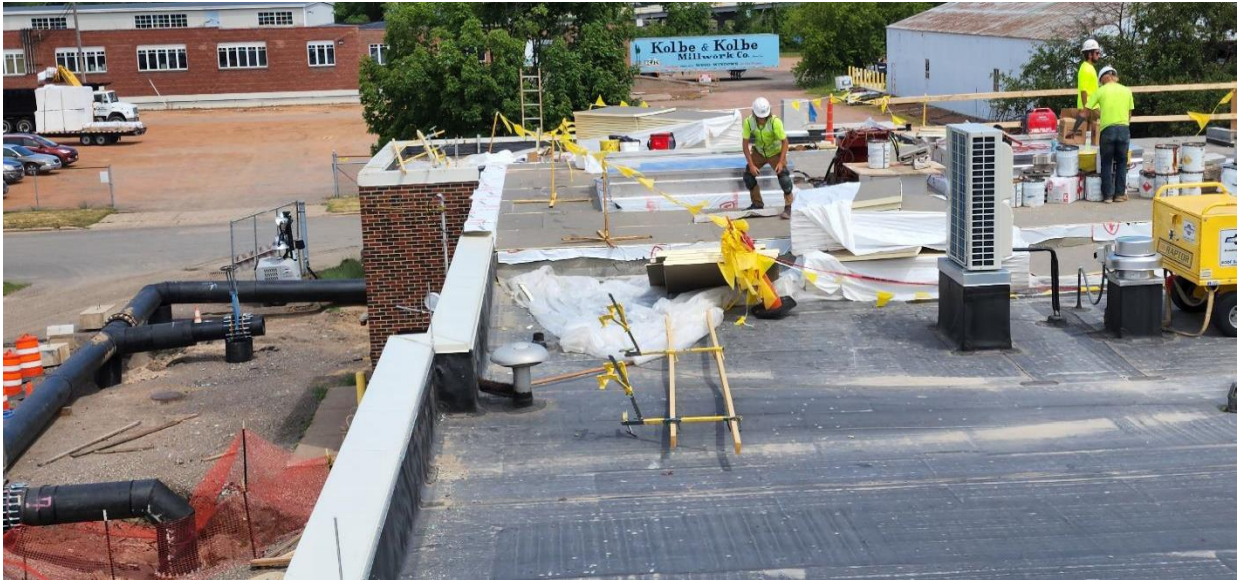
Quality Roofing installing insulation over new precast roof for the raw wastewater pump room of Structure 100 (Main Building).
