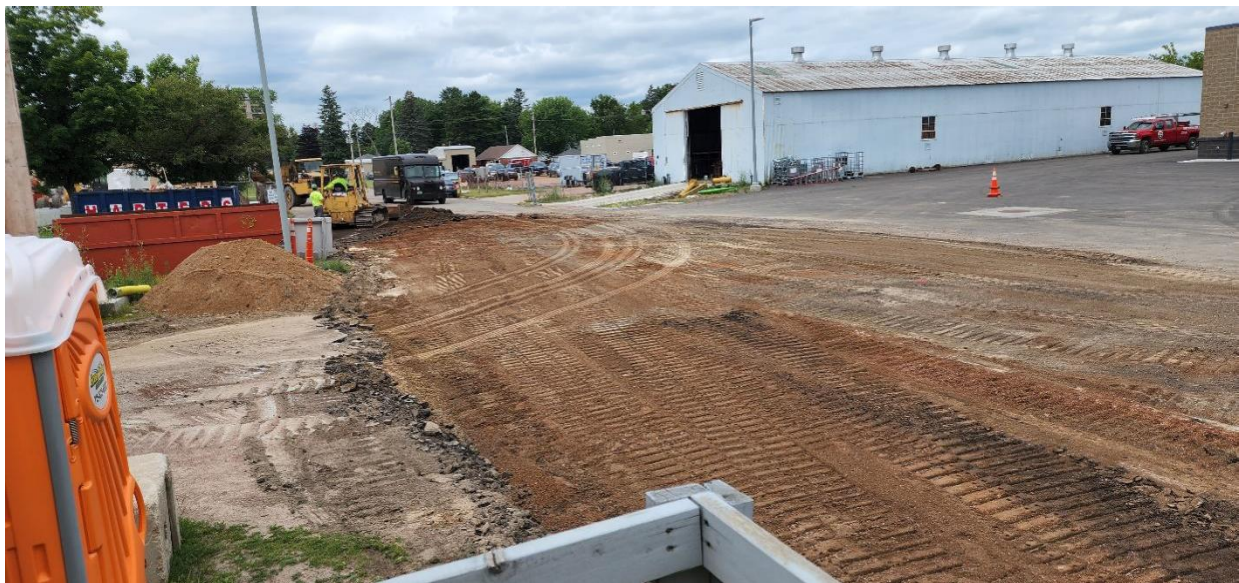
Asphalt removal completed along Adrian Street.
