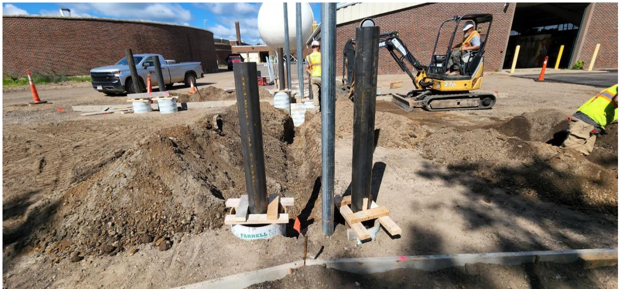
Van Ert Electric installing conduit and control wiring for new gate and access card reader.
