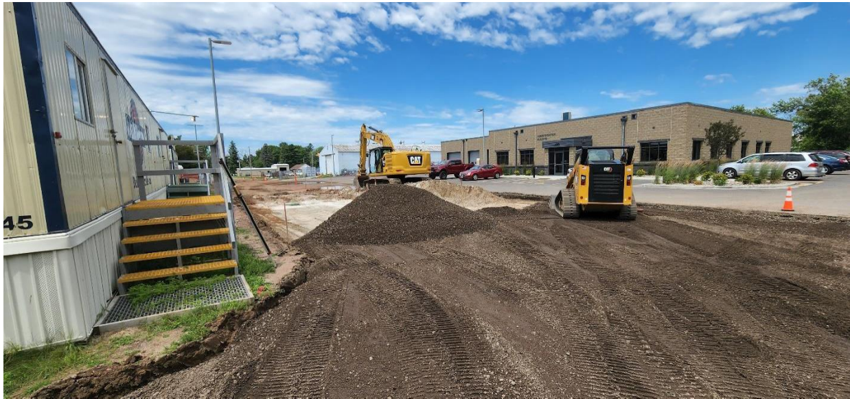
Preparing for asphalt on Adrian Street.
