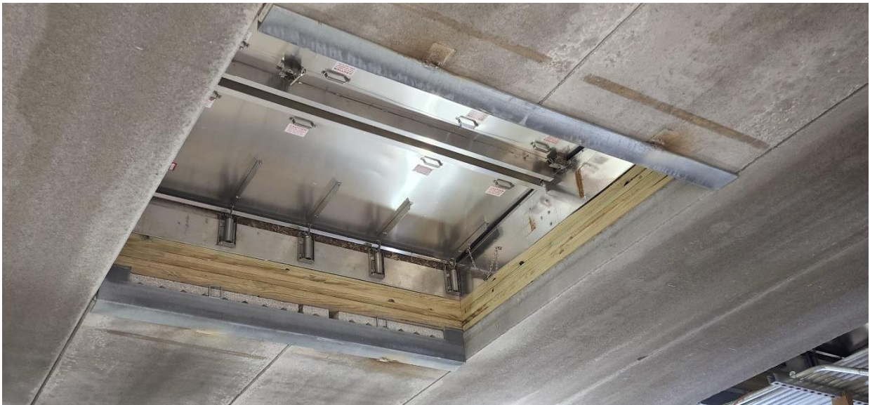
New roof hatches for raw wastewater pump room of Structure 100 (Main Building).
