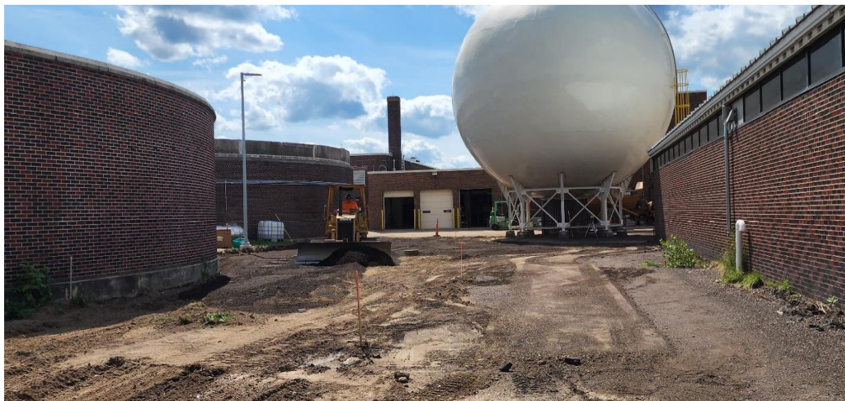
Final grading around Structure 750 (Gas Sphere).
