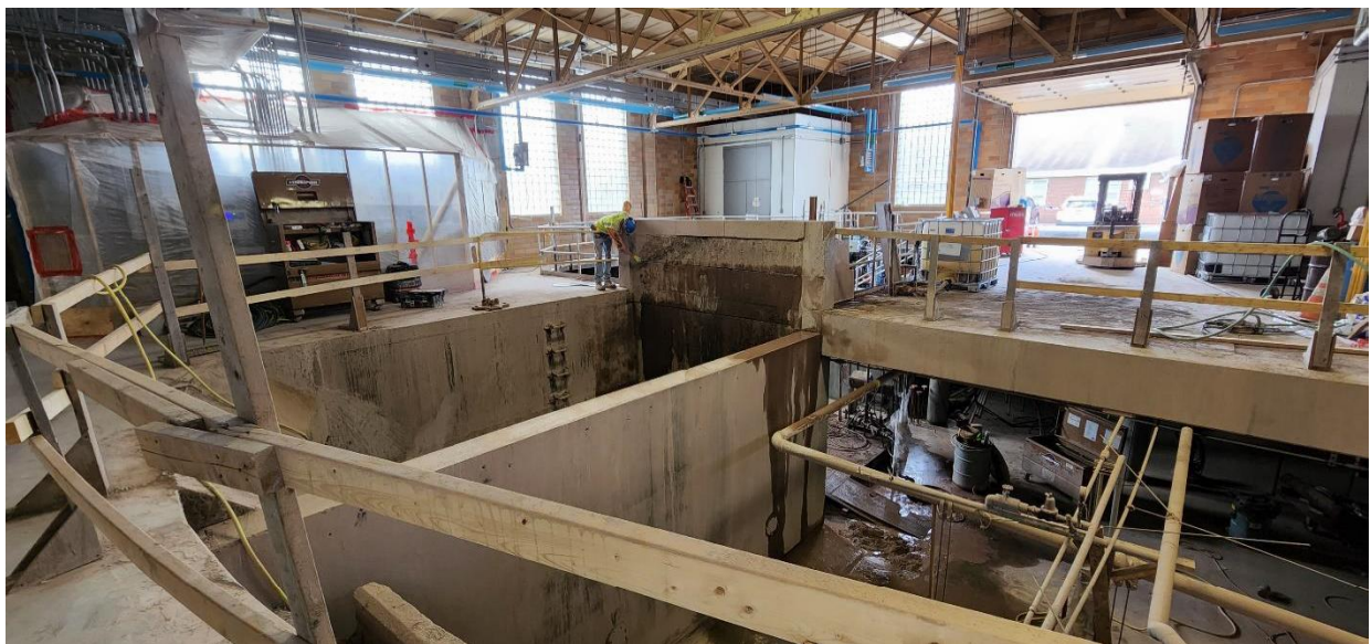
Concrete demolition continues in the new equipment maintenance/storage area of Structure 100 (Main Building).
