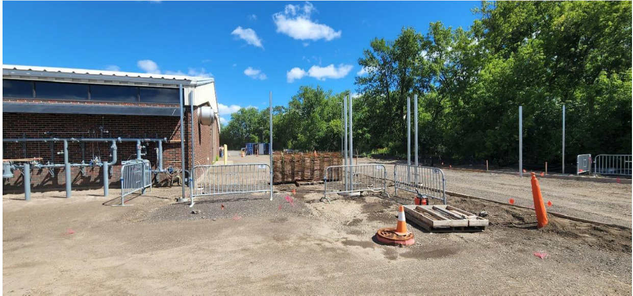
New fence posts set for new east access gate.
