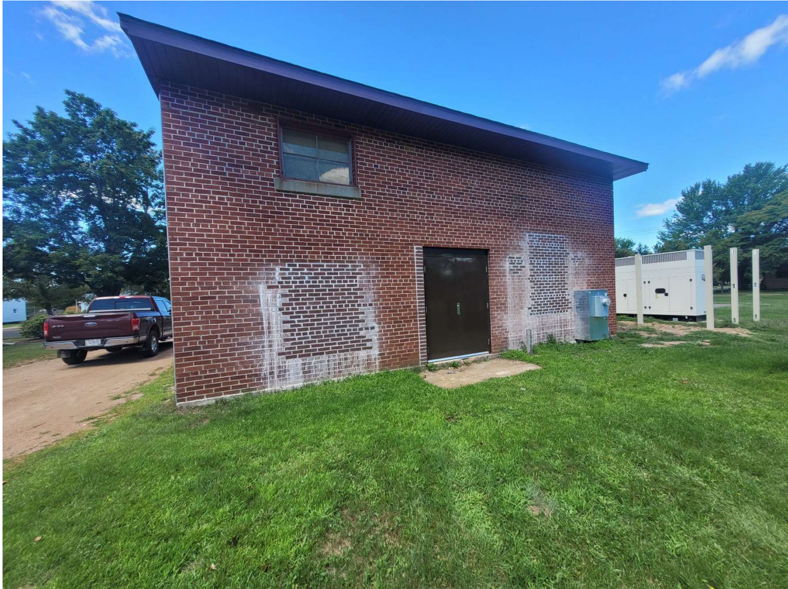
Well House Improvements – Elimination of Ground Level Windows & Generator Installation
