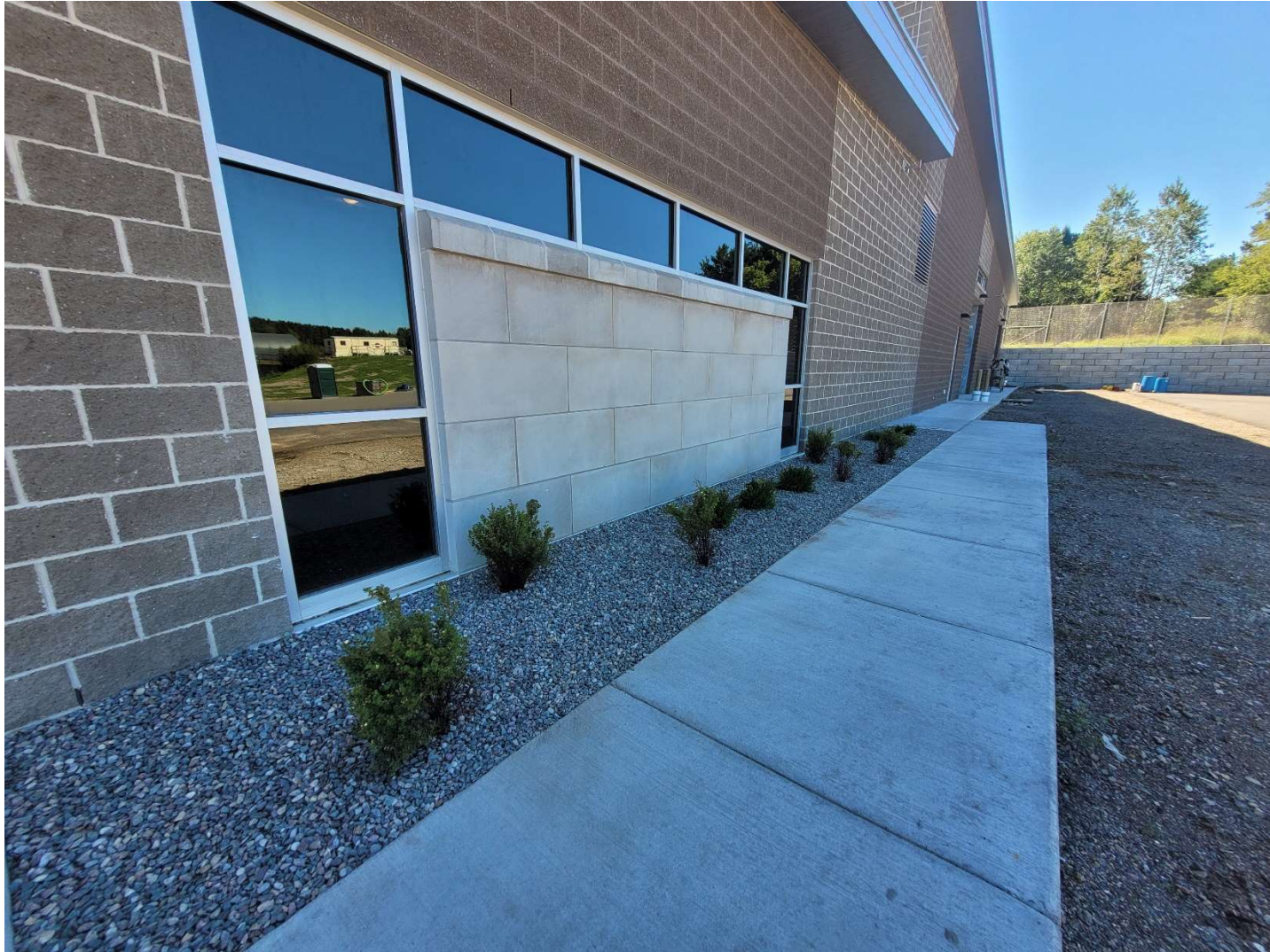
Landscaping installed along Administration Building
