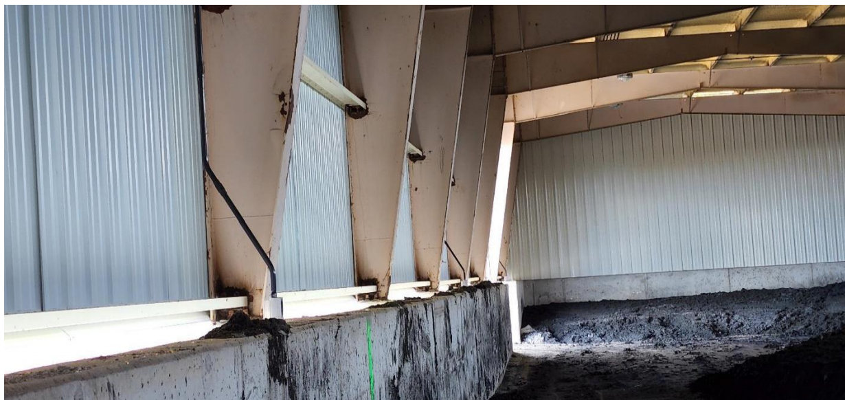
New outlets installed in center bay of Structure 760 (Biosolids Storage Building).
