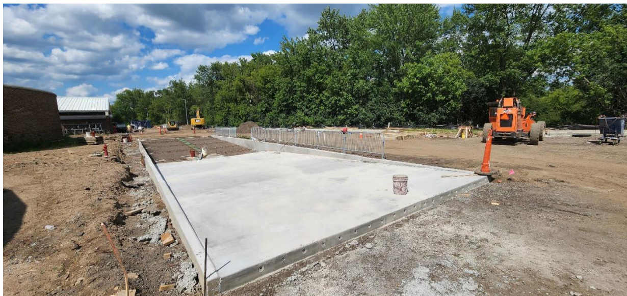
New concrete for modified septage receiving area.
