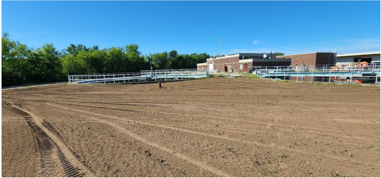
Grading of area between Structure 500 (Secondary Splitter) and the Structures 510 and 520 (Secondary Clarifiers 1 and 2) on the southeast side of the site.
