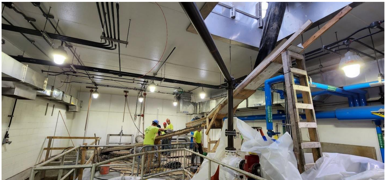
Concrete pour for new primary influent walls at Structure 200 (Grit Building).
