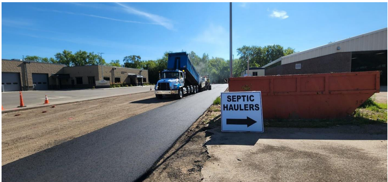
Binder course of asphalt being placed on Adrian Street.
