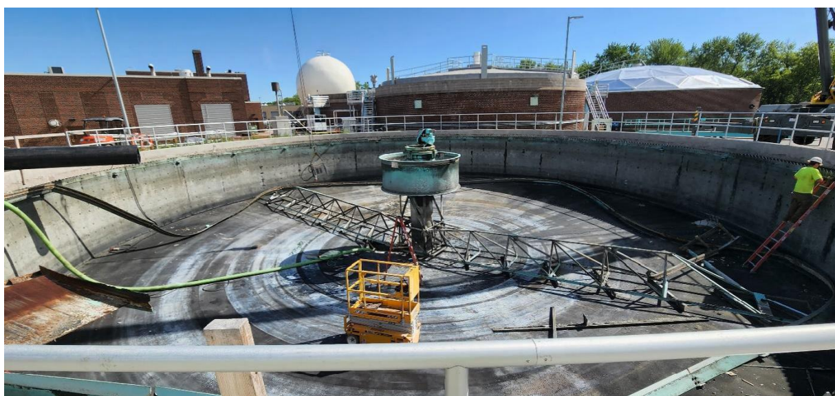
R-Industries removing the old mechanism and weirs of Structure 320 (Primary Clarifier 2).
