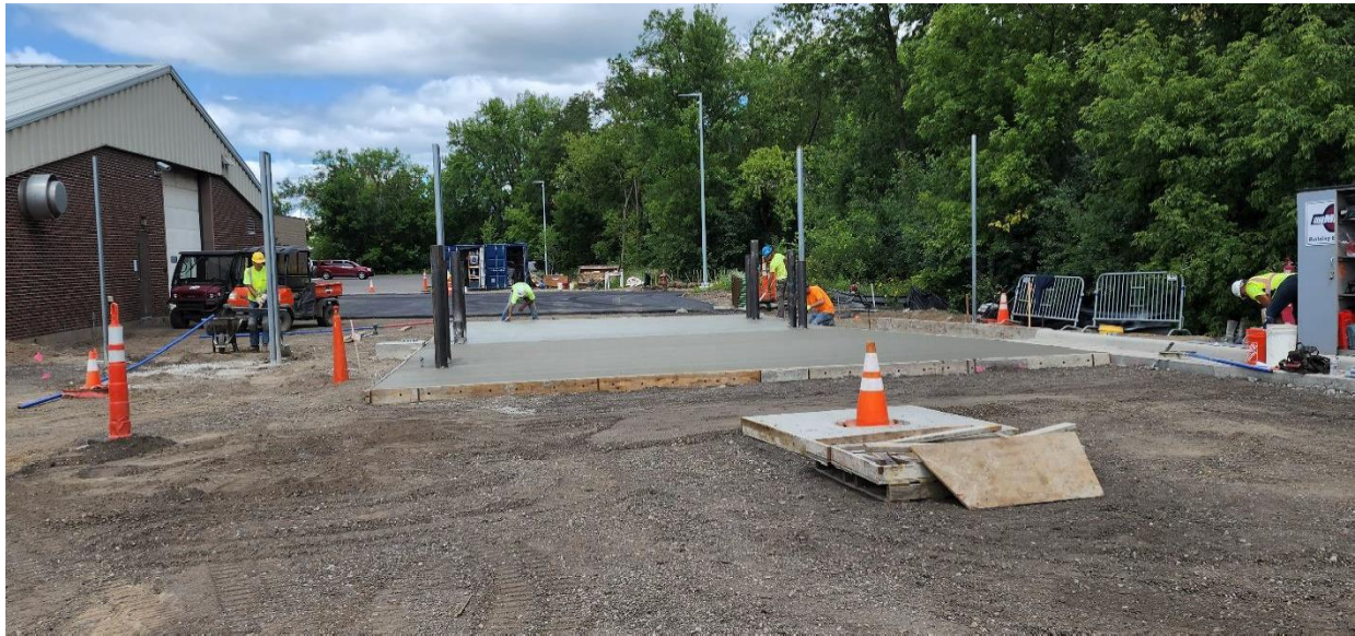
Concrete gate entrance mat installed.
