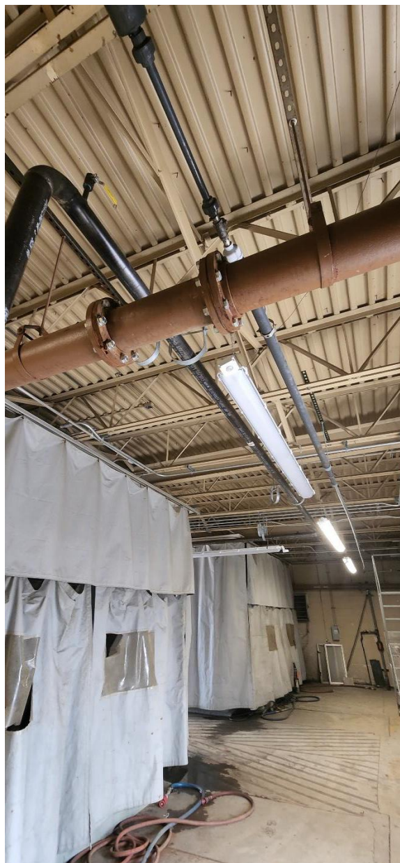
New lighting installed in existing belt filter press area of Structure 100 (Main Building).
