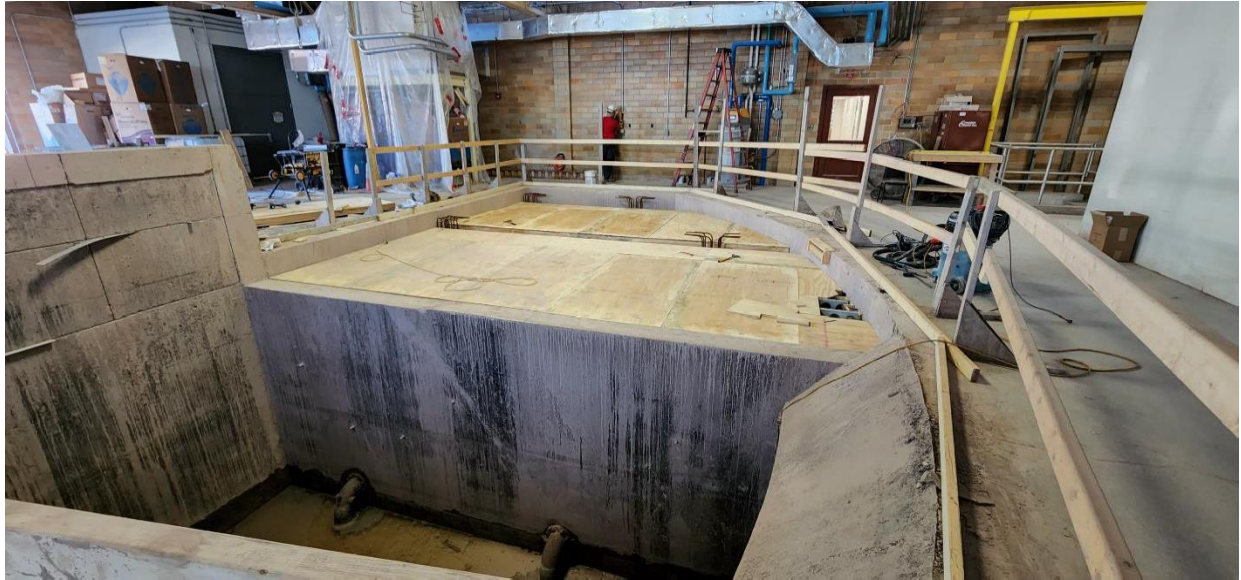
Structure 100 (Main Building): start of shoring and rebar for equipment/maintenance storage area floor.
