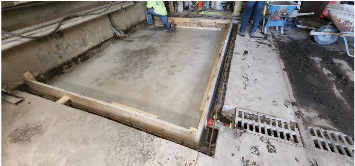
Finishing formwork for the new equipment wash down area in the north garage of Structure 100 (Main Building).
