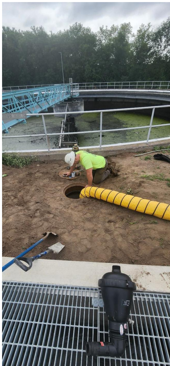
IGE installing the new RAS line air release valve.
