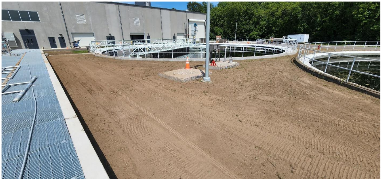
Site grading around Structures 530 and 540 (Secondary Clarifiers 3 and 4).
