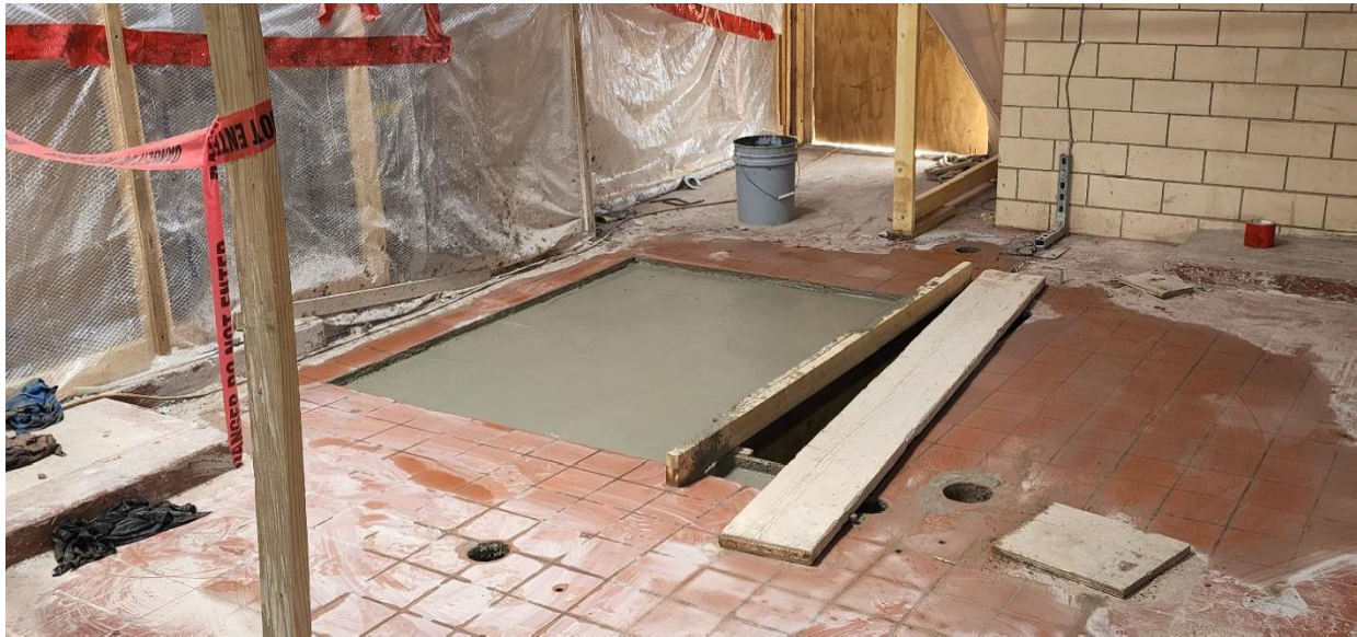
Concrete work to fill in old pump room access hatch of Structure 100 (Main Building).
