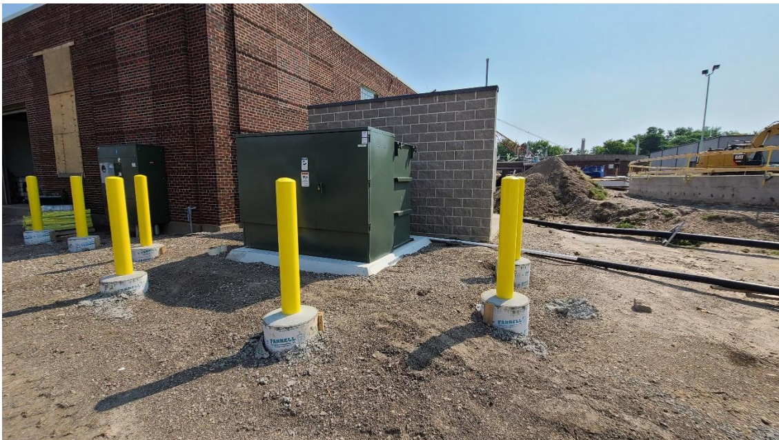
Pipe bollards placed for the protection of the new transformers to feed main plant power to Str. 100
