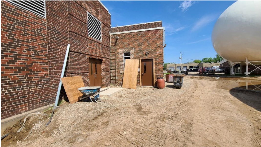
New doors, windows and exhaust louvers install at the east garage and gas compressor entrances of Structure 100 (Main Building).
