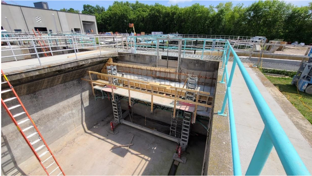
Form work set up for weir trough in Aeration Basin 6 (Basin 2C per plan).
