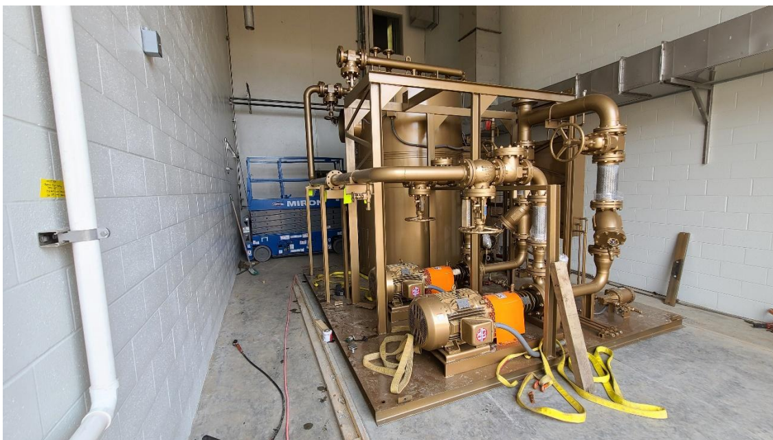
Thermal oil skid set on new pad at Structure 770 (Solids Building).
