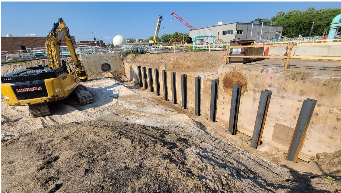
Michels placing H-piles for structural support at Structure 405 (Anoxic Selector Tank).
