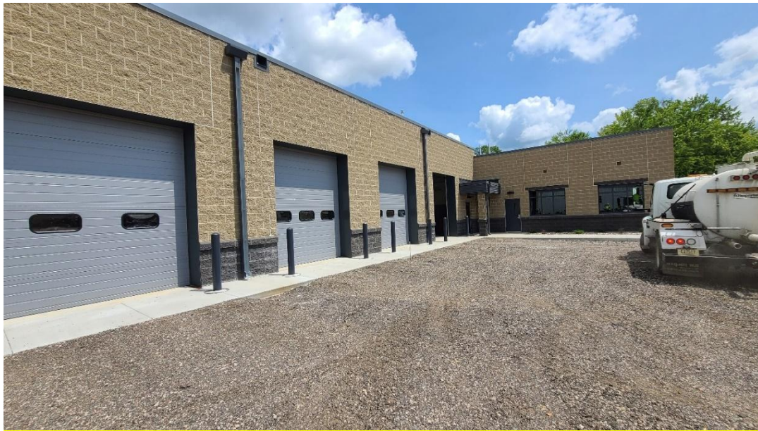
Structure 120 (Administration Building): landscape complete.
