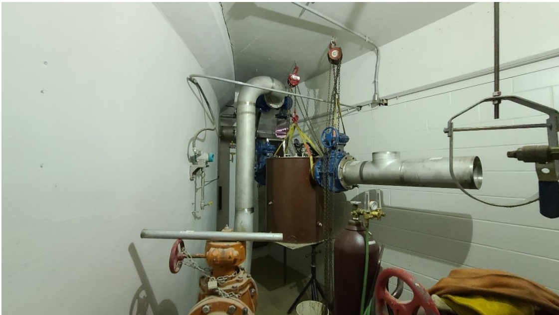
Gas handling room, piping being placed, room has been painted at Structure 700 (Digester Building).
