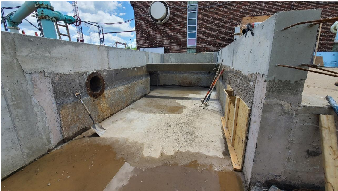
Miron form work to fill in hole from removed 48" pipe sleeve to 900 Tunnel.
