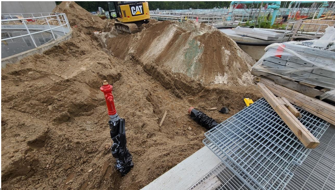
Placement of new yard hydrant east of tunnel 900 between Structure 340 and the 410 Aeration Basins
