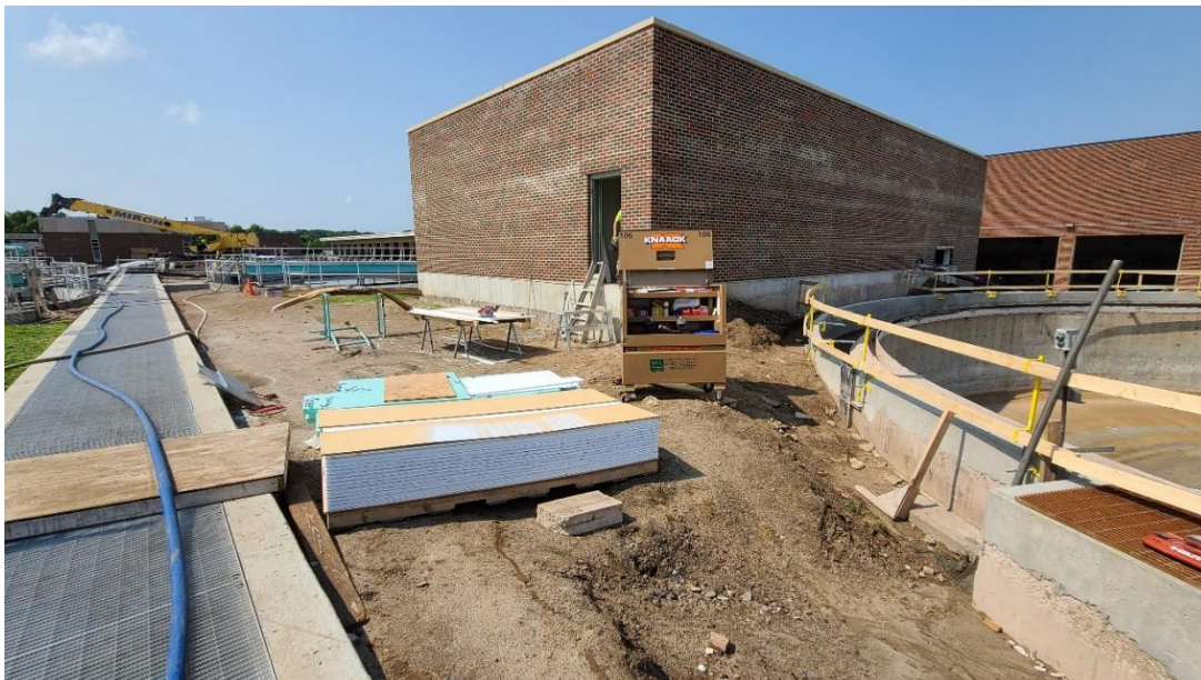
Exterior brickwork complete on Structure 200 (Grit Building).
