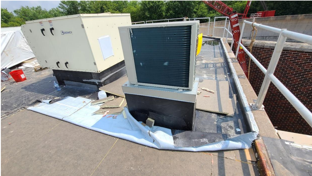
New roof membrane being place and HVAC equipment set at Stucture 700 (Digester Building).
