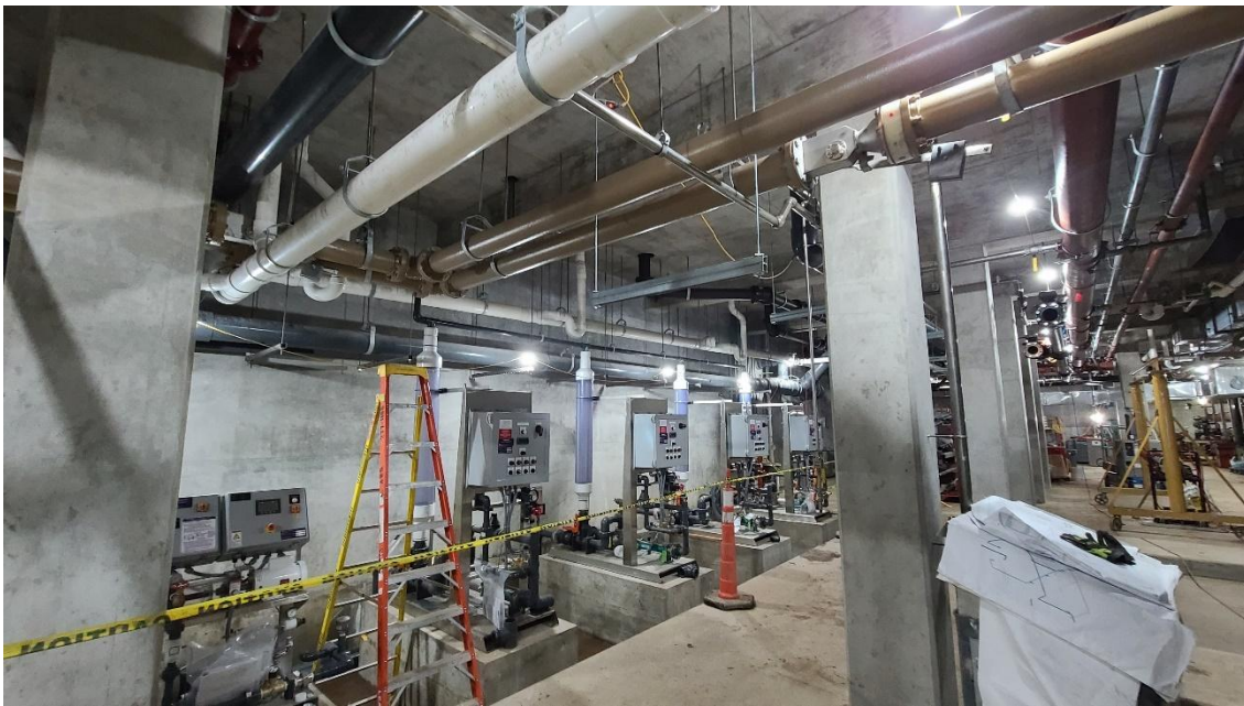
Lower level chemical feed pumps placed and piping to and from being installed at Structure 770 (Solids Building).
