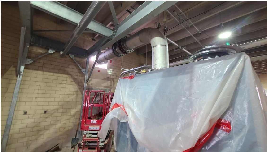
Aeration blower piping connected and run to the exterior of Structure 400 (Activated Sludge Building).
