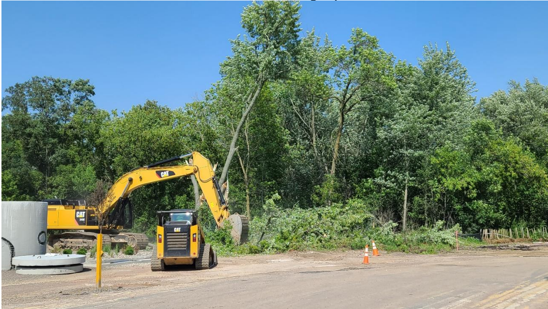
Precision removing trees for final stormwater tie-in at Structure 120 (Administration Building)
