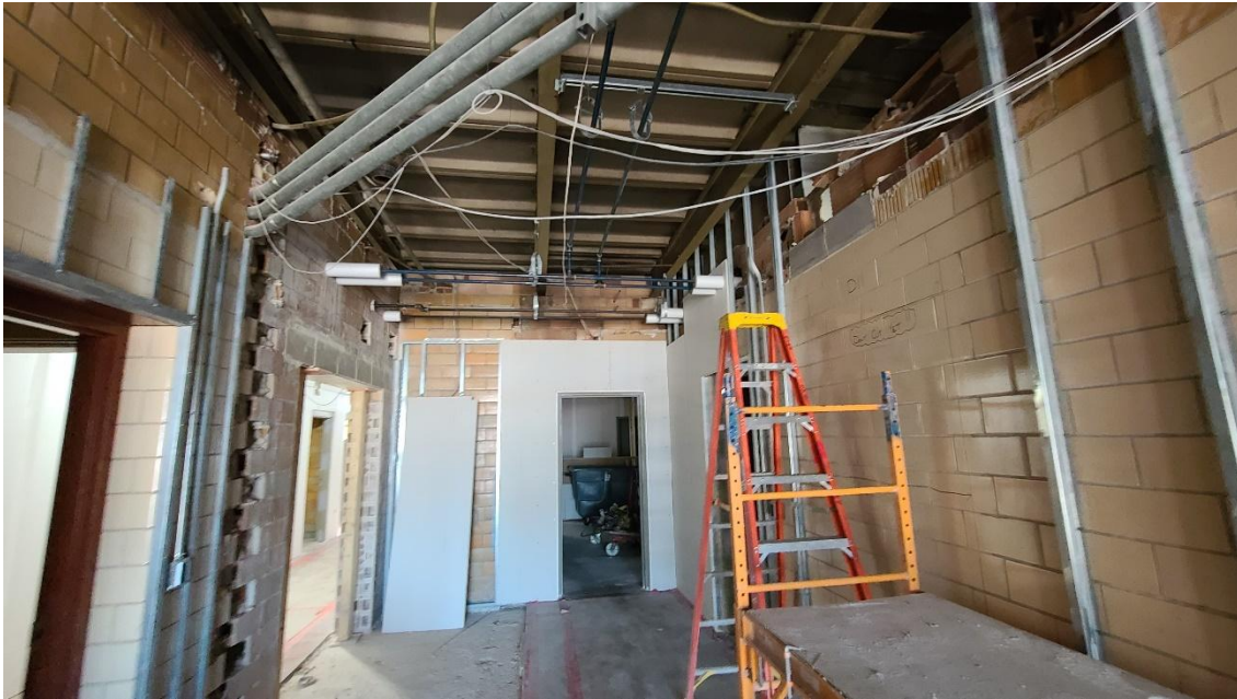
Structure 100 (Main Building): Demolition work in the main foyer area with new door way cut in to the left.
