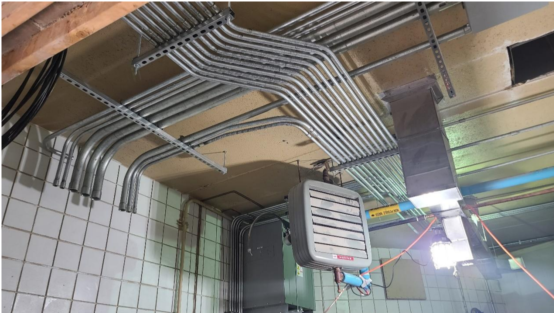
Conduit runs and placement in new electrical room of Structure 700 (Digester Building).
