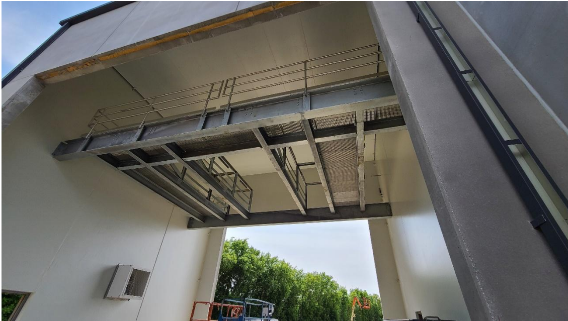
Structure 770 (Solids Building): biosolids handling area platform set.
