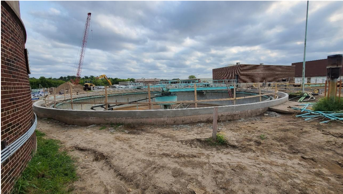
New top portion of basin wall on Structure. 320 (Primary Clarifier 2).
