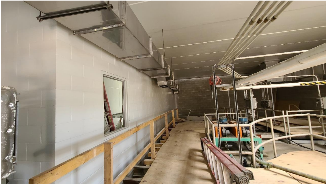
Interior painting and duct work has started in Structure 200 (Grit Building)
