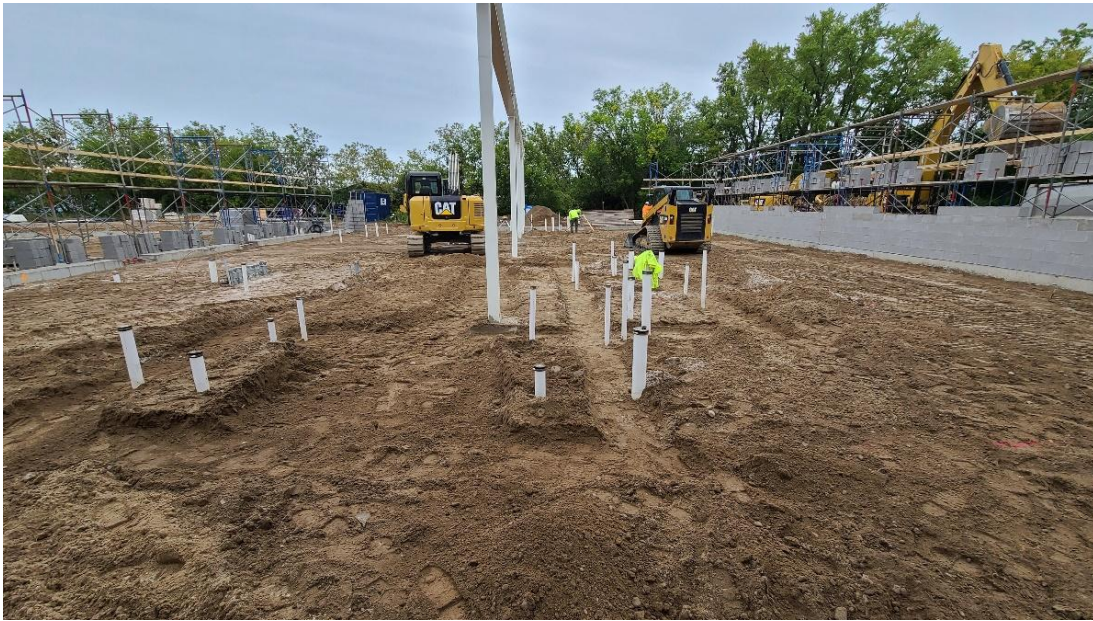
Structure 120 (Administration Building) below slab sanitary piping and electrical conduit.
