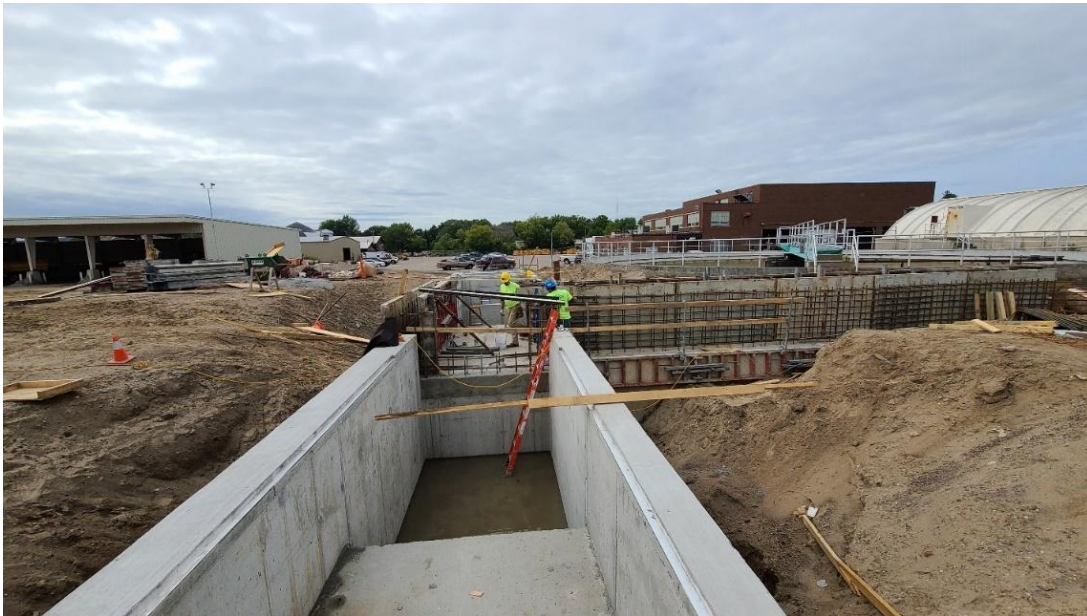
Structure 404 (Junction Structure) with Structure 350 (PE Channel) about to be tied into it.
