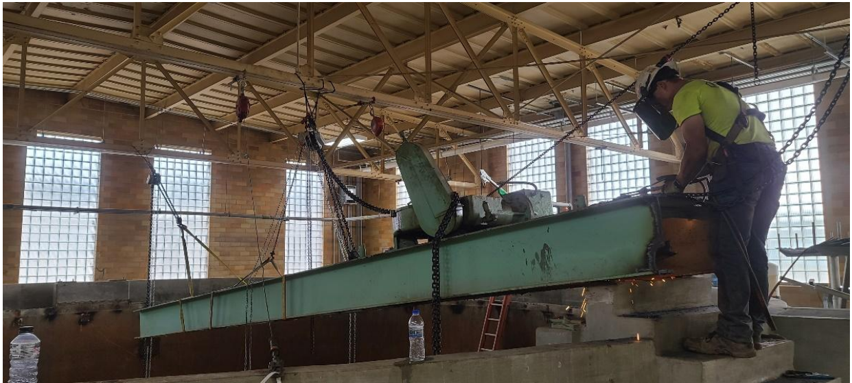
Demolition on center platform of existing gravity thickener.
