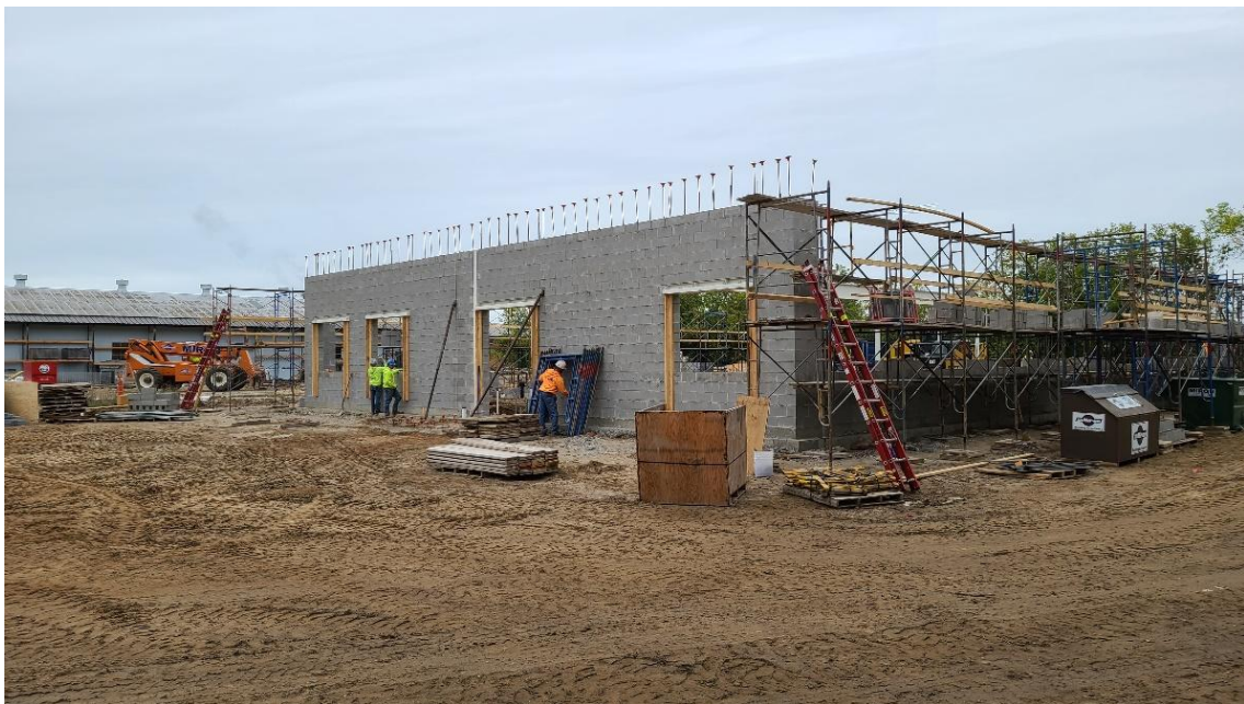
South concrete masonry unit wall of Structure 120 (Administration Building), with the start of the east wall.
