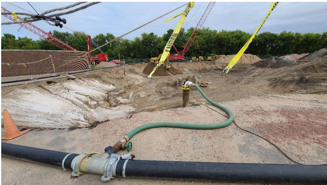
Structure 770 (Solids Building) excavation, existing dewatering well system and demolition of manhole structure.
