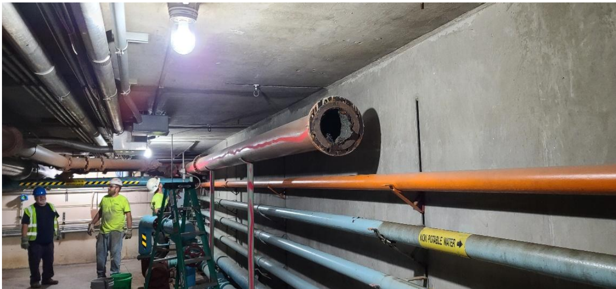
Removal of Gravity Thickener line in Tunnel that was tied into the 48" Effluent Line.
