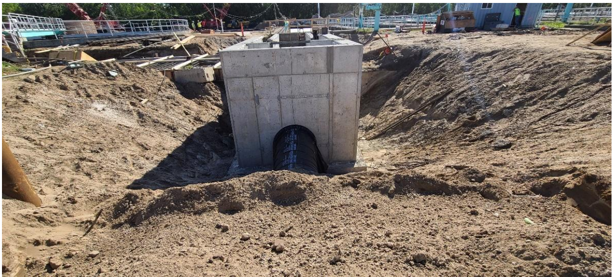
36" Bypass line exiting the west side of Structure 404 (Junction Structure).
