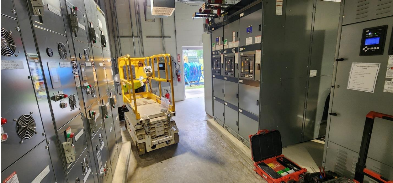
Work is taking place in Structure 100 (Process Building) electrical room.
