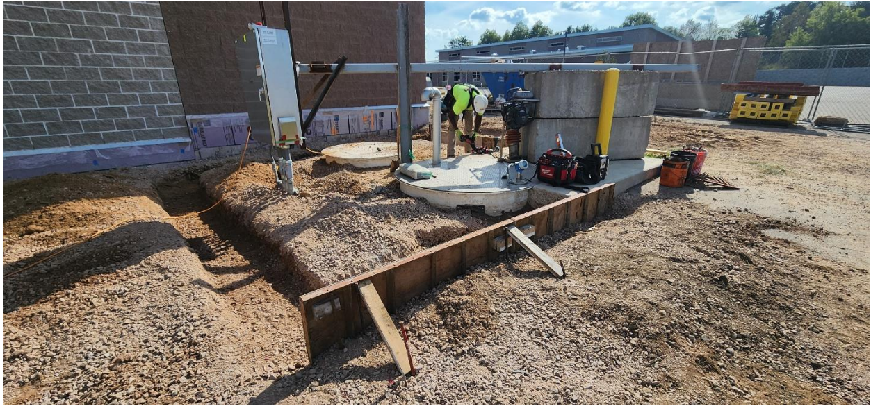
Prepping for new concrete slab around Structure 410 (Sanitary Lift Station).
