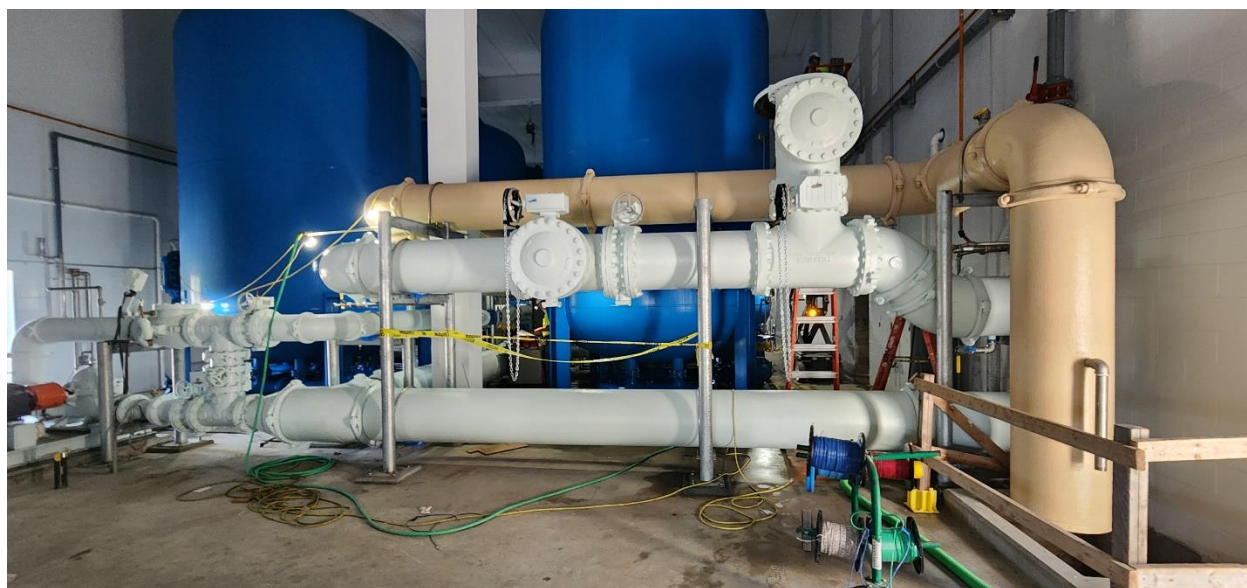
Structure 120 (PFAS Treatment Building) piping painted.
