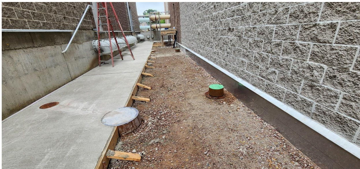
Half of concrete poured between Structure 100 (Process Building) and Structure 120 (PFAS Treatment Building).
