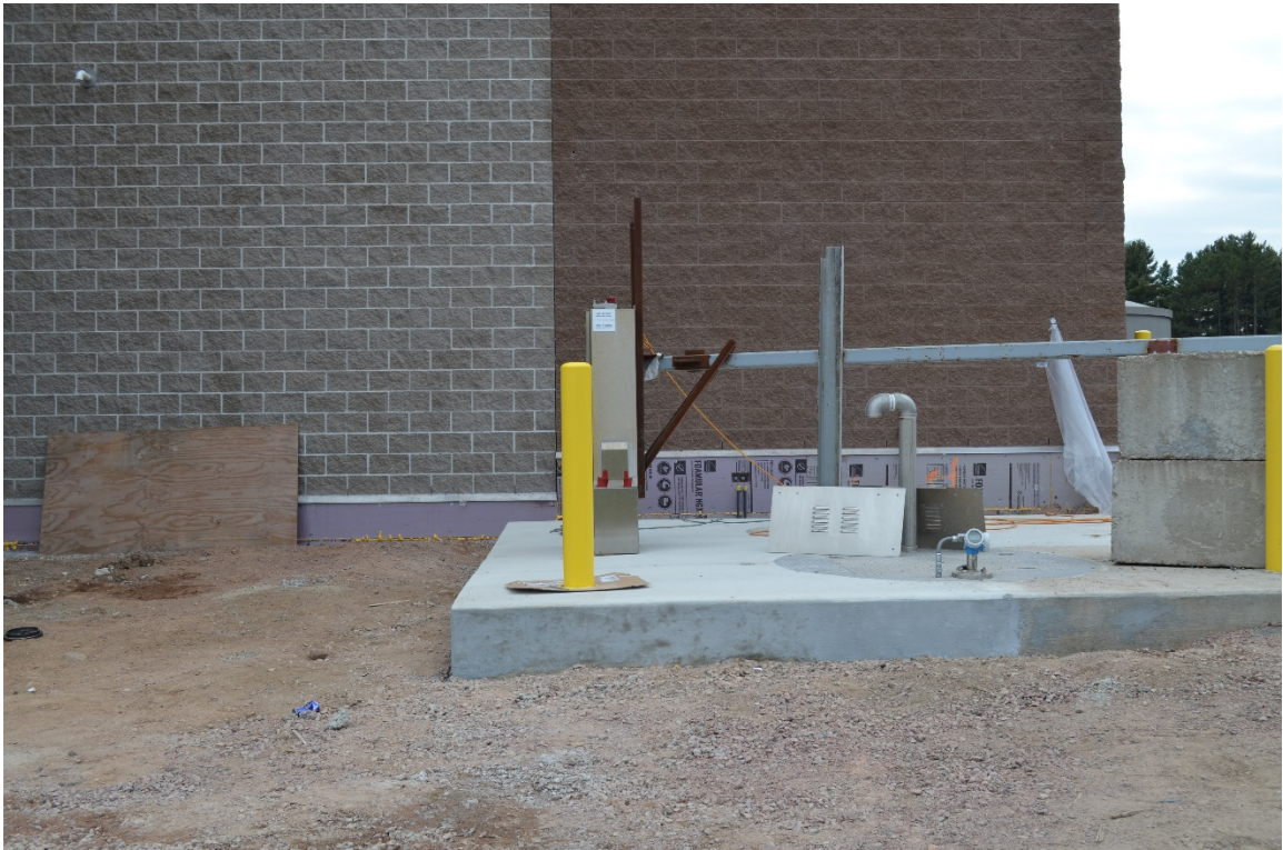
Structure 410 (Sanitary Lift Station) concrete slab complete and bollards painted.
