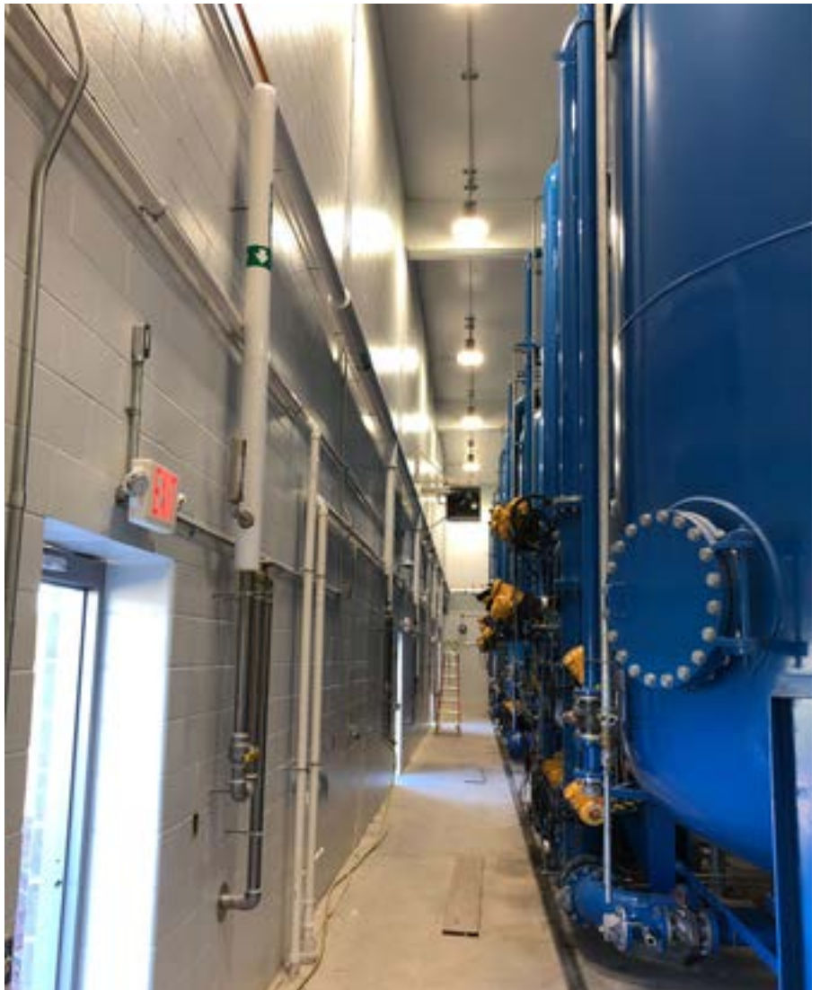
North side of PFAS Treatment Building (Structure 120): lighting in place, painting completed.
