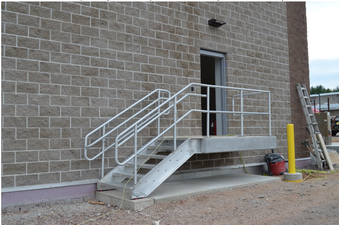
Steps installed on exterior door landings of PFAS Treatment Building.
