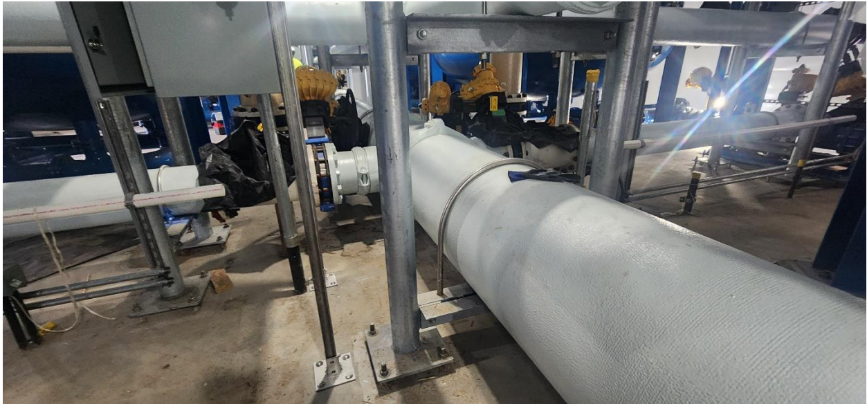
Work continues on PFAS treatment system piping in Structure 120 (PFAS Treatment Building)
