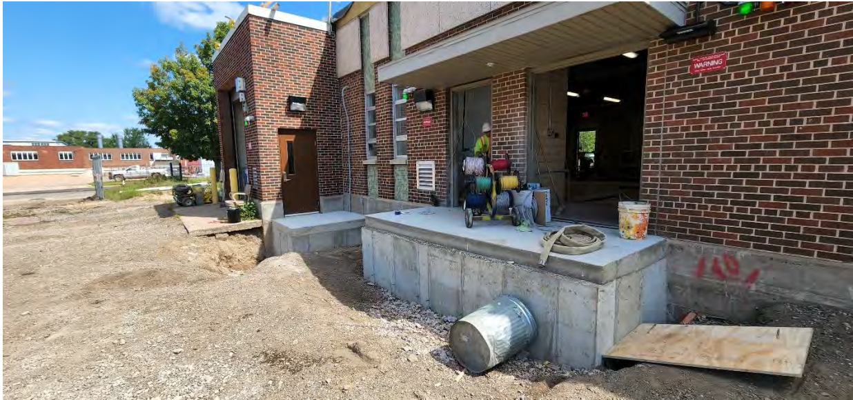
New foundations for stoops placed for screen and raw wastewater pumping rooms of Structure 100.
