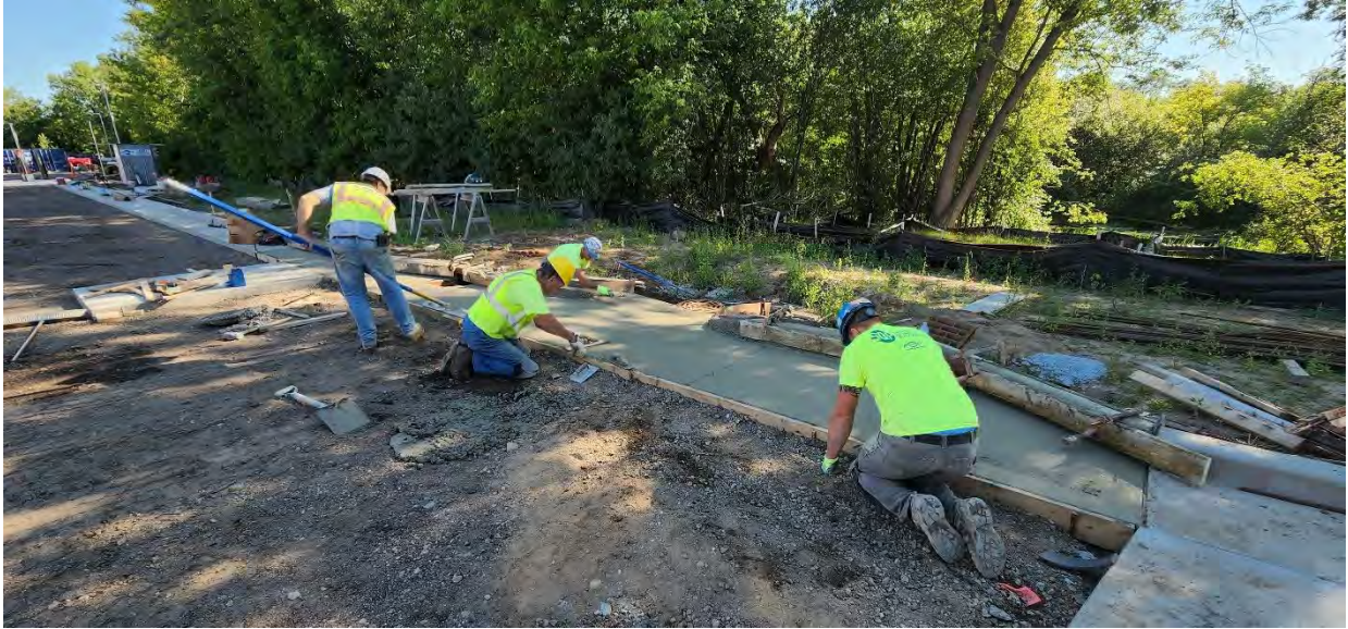
Last section of curb and gutter being placed north of Structure 770 (Solids Building) and east of Structure 700 (Digester Building).
