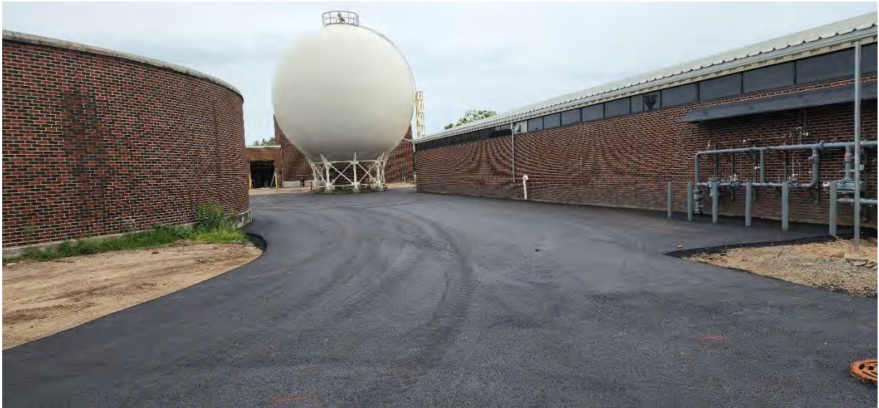
Asphalt binder course placed around gas ball and between Structure 110 (Vehicle Storage Building) and Structure 700 (Digester Building).
