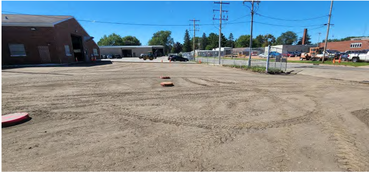
Ready for asphalt between Department of Public Works and WWTF near Adrian Street.
