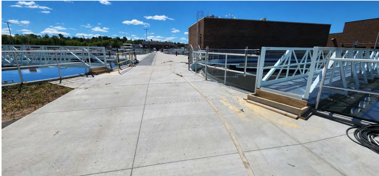
Prepping for concrete step pours for Structures 310 and 320 (Primary Clarifiers 1 and 2).
