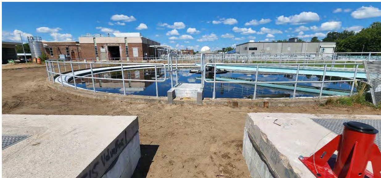
New scum beach platform at Structure 510 (Secondary Clarifier 1).
