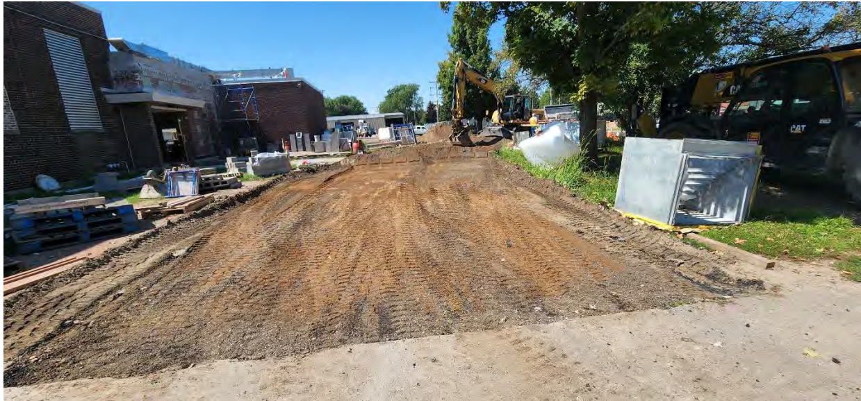
Temporary septic receiving driveway removed, new septic receiving area up and running.
