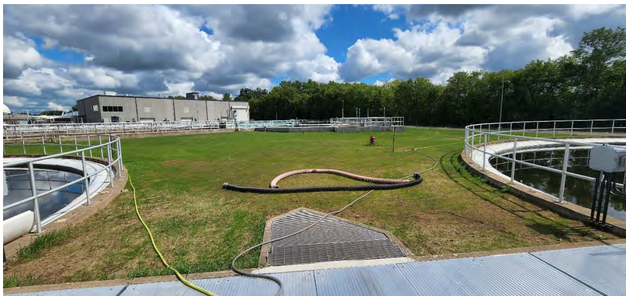
New grass between Structures 510 and 520 (Secondary Clarifiers 1 and 2) looking north to the Structure 500 (Splitter Basin).
