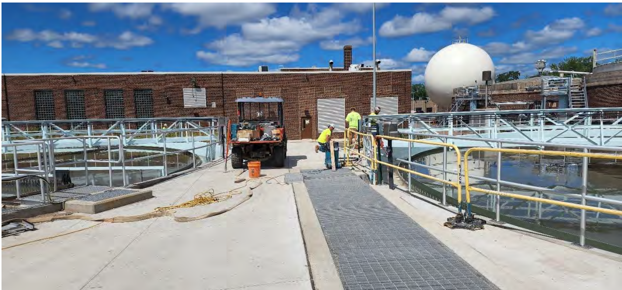
New handrail being completed around Structures 310 and 320 (Primary Clarifiers 1 and 2).
