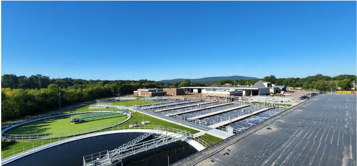
Looking south from the roof of Structure 770 (Solids Building).
