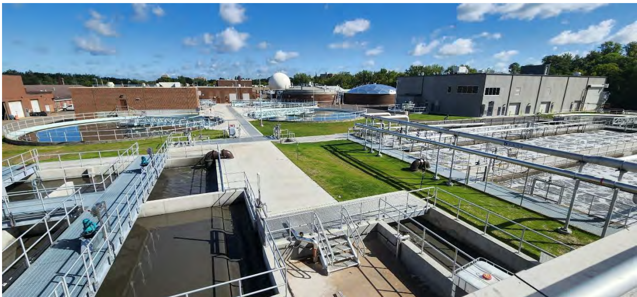
Looking north from the roof of Structure 400 (Activated Sludge Building).
