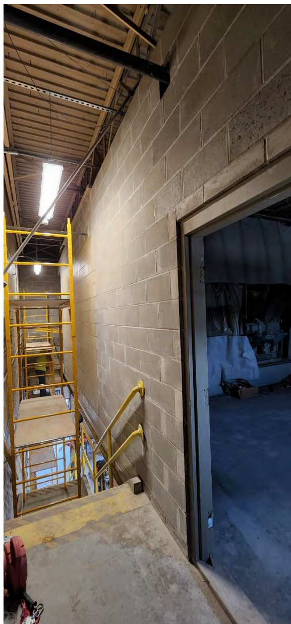
New concrete masonry unit wall at old belt filter press stairway with new lighting.
