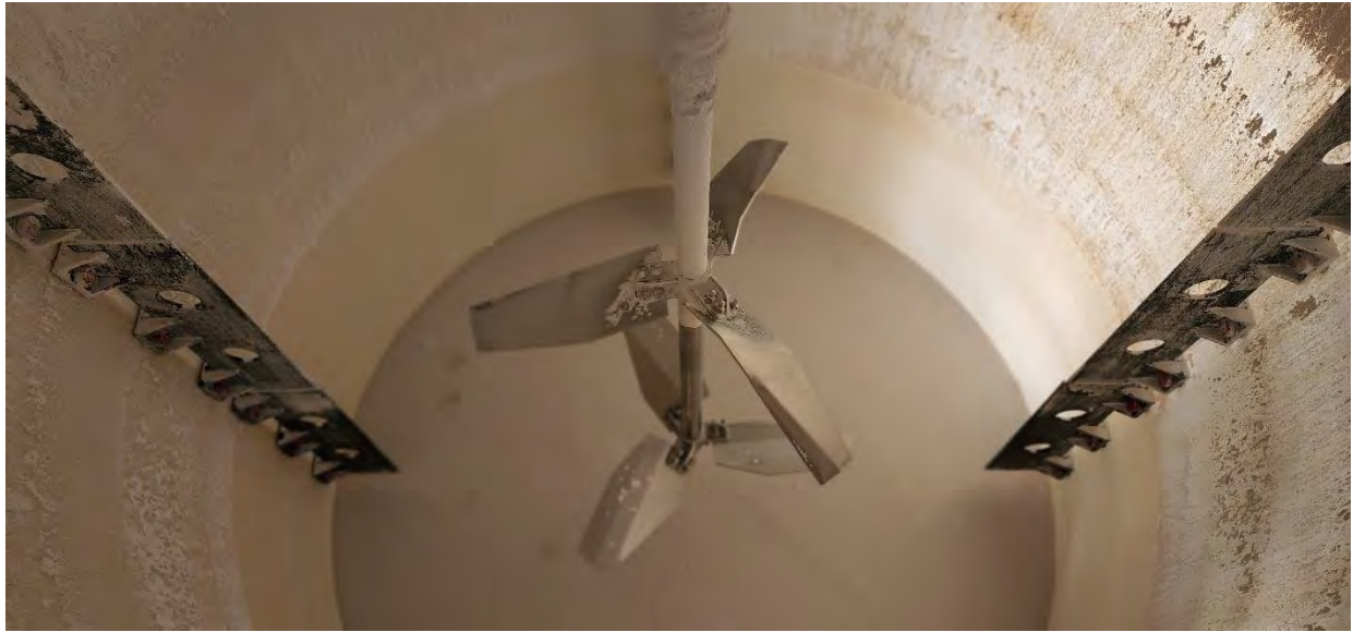
Look inside a Structure 610 (Chemical Building) storage tank at tank baffles and mixing blades.
