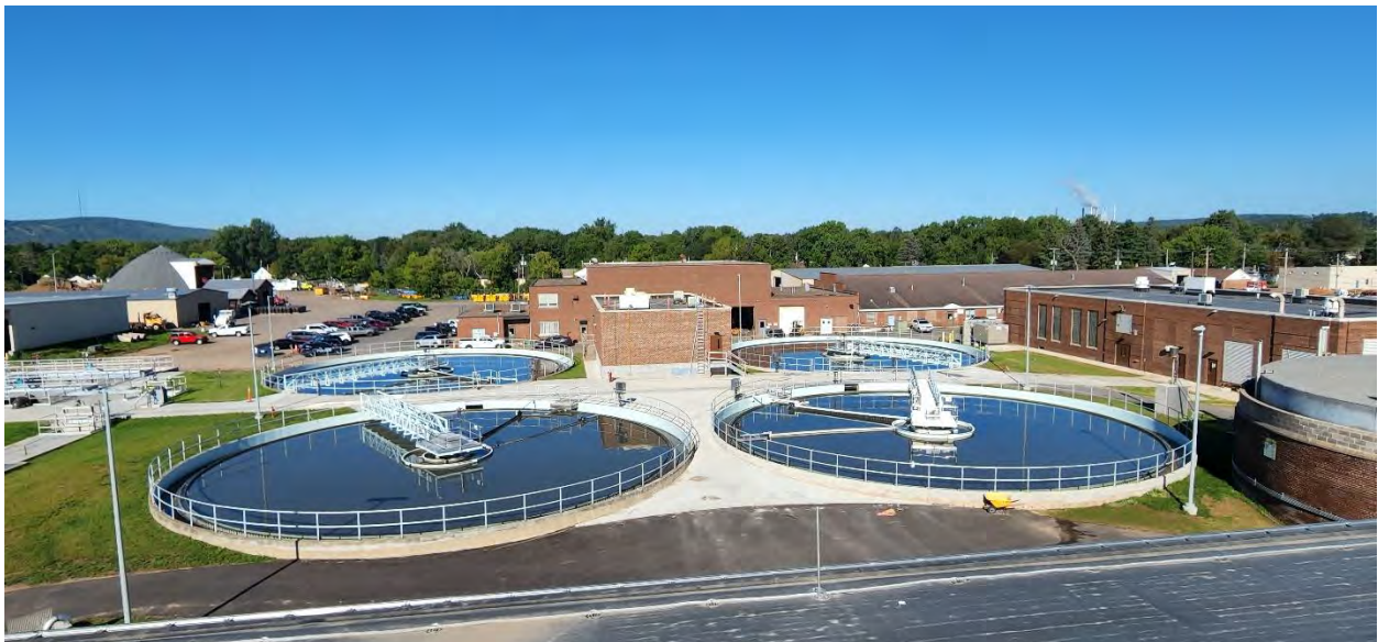
Looking west from the roof of Structure 770 (Solids Building).
