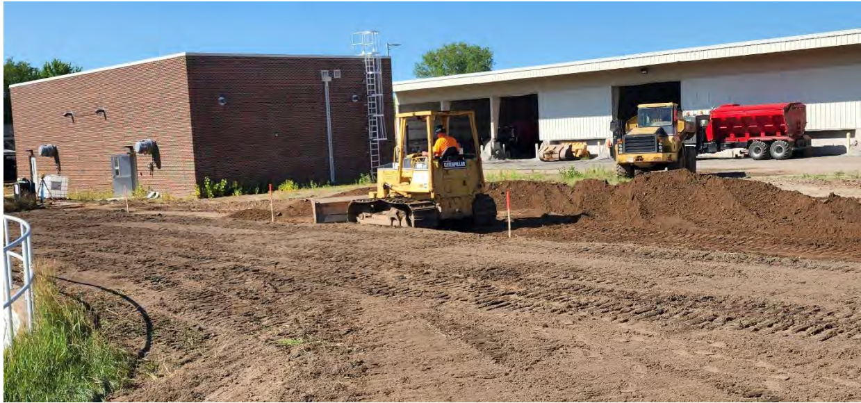
Grading for landscaping and sidewalk between Structure 400 (Activated Sludge Building) and Structure 600 (Effluent Building).
