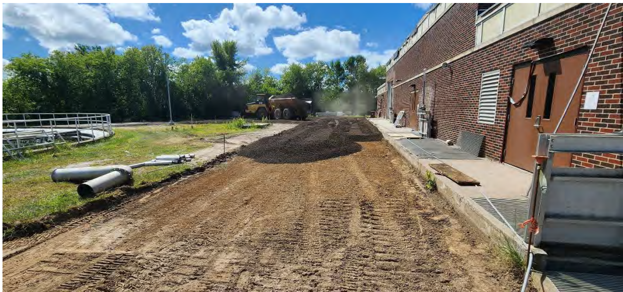
Road base being placed along the east side of Structure 600 (Effluent Building).
