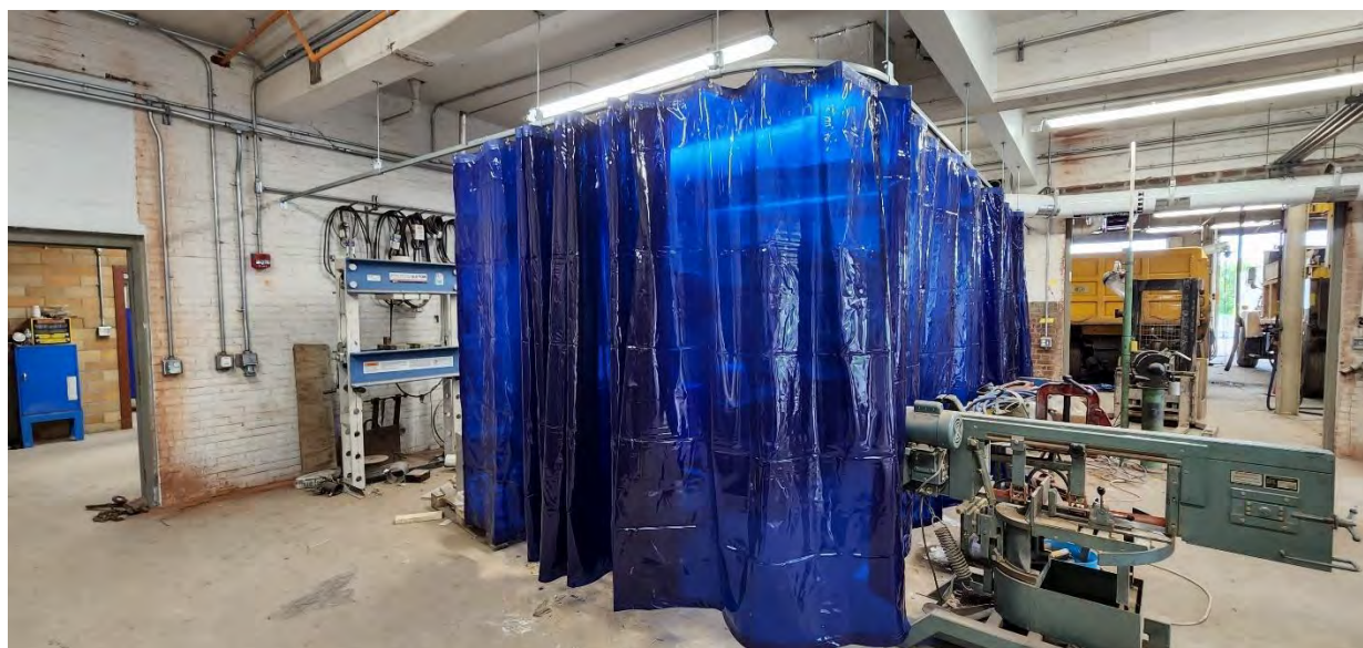
New welding curtain hung at Structure 100 (Main Building).
