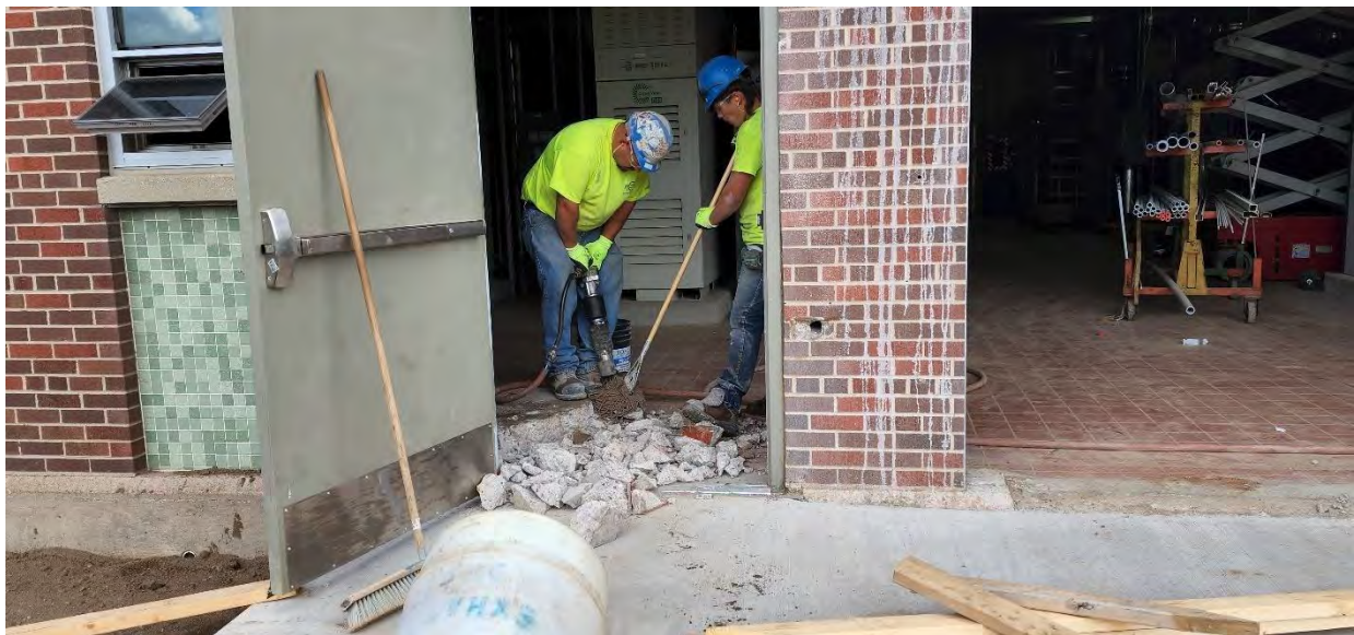
Demolition of the old air compressor pad in Structure 400 (Activated Sludge Building), using a wet mop for dust control
