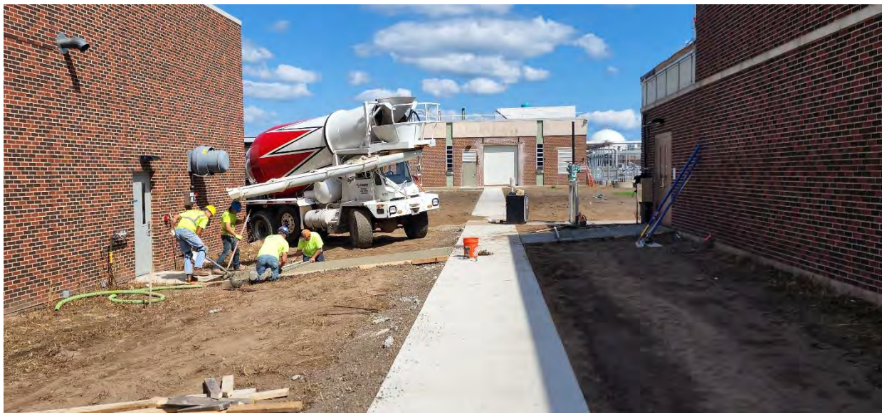
Concrete sidewalk installed between Structures 600 and 610 (Effluent Building and Chemical Building), heading north to Structure 400 (Activated Sludge Building).
