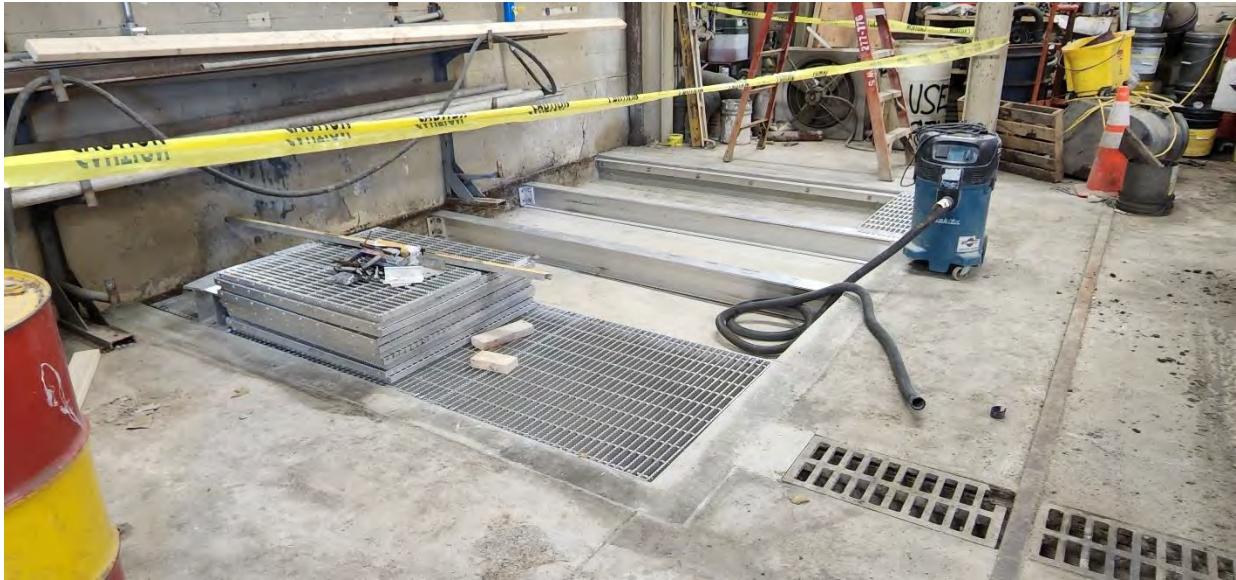
Structure 100 (Main Building) new equipment wash down area in north garage.
