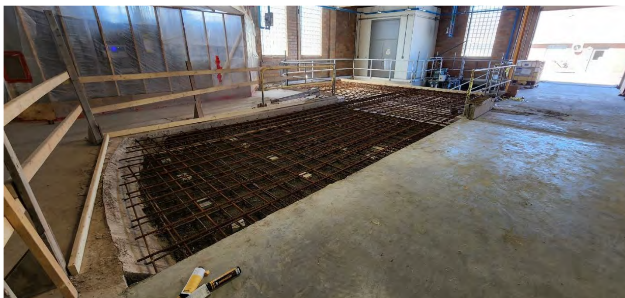
Final area of floor in new storage area of Structure 100 ready for concrete, filled in old gravity belt thickener basin with structural fill and rebar.
