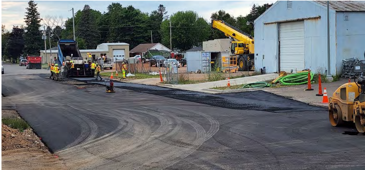
Asphalt being placed along Adrian Street.
