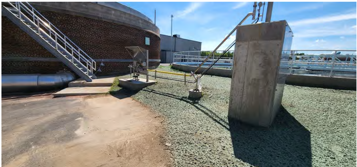
Landscaping mulch and grass placed around new flare of Structure 755 (Waste Gas Burner).
