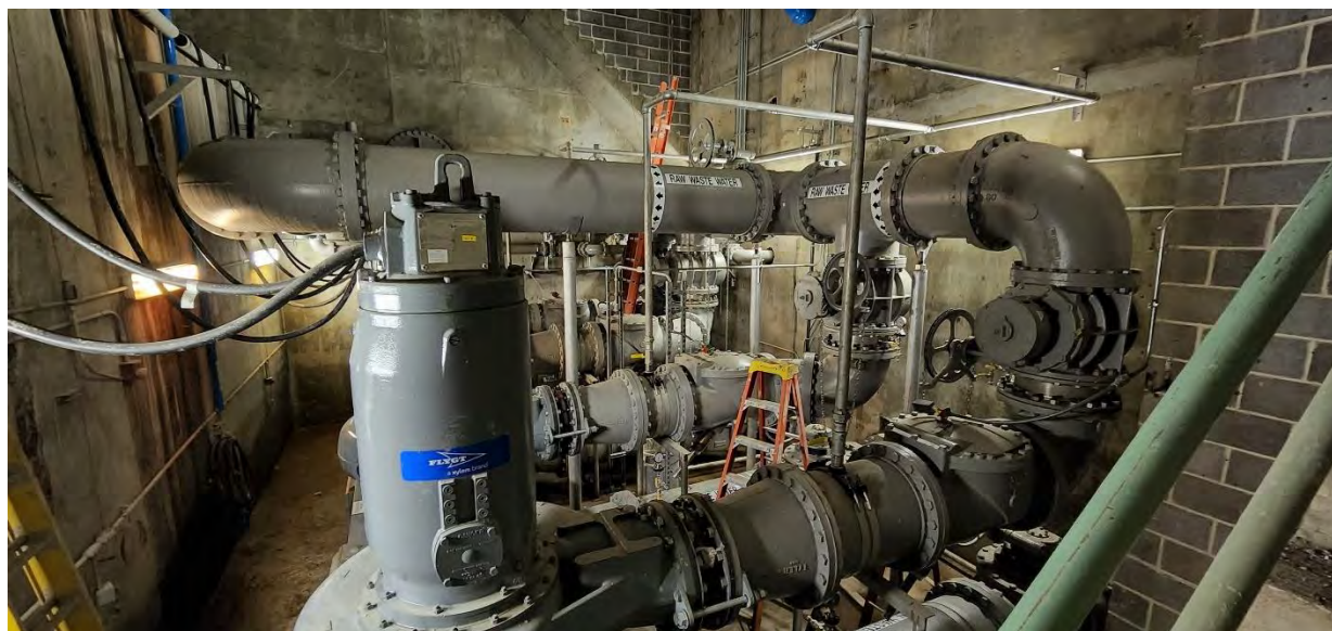
Structure 100 raw wastewater pump room piping and pumps painted.
