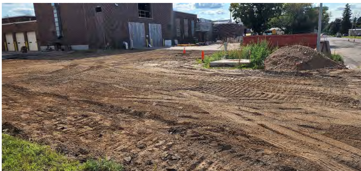
Removal of old parking area on north side of Structure 100 (Main Building) completed to prepare for new asphalt.
