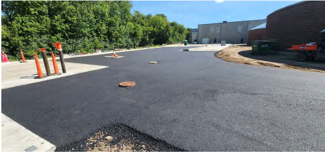
New asphalt binder course placed around new septage receiving area, east of Structure 700 (Digester Building), picture looking south at Structure 770 (Solids Building).
