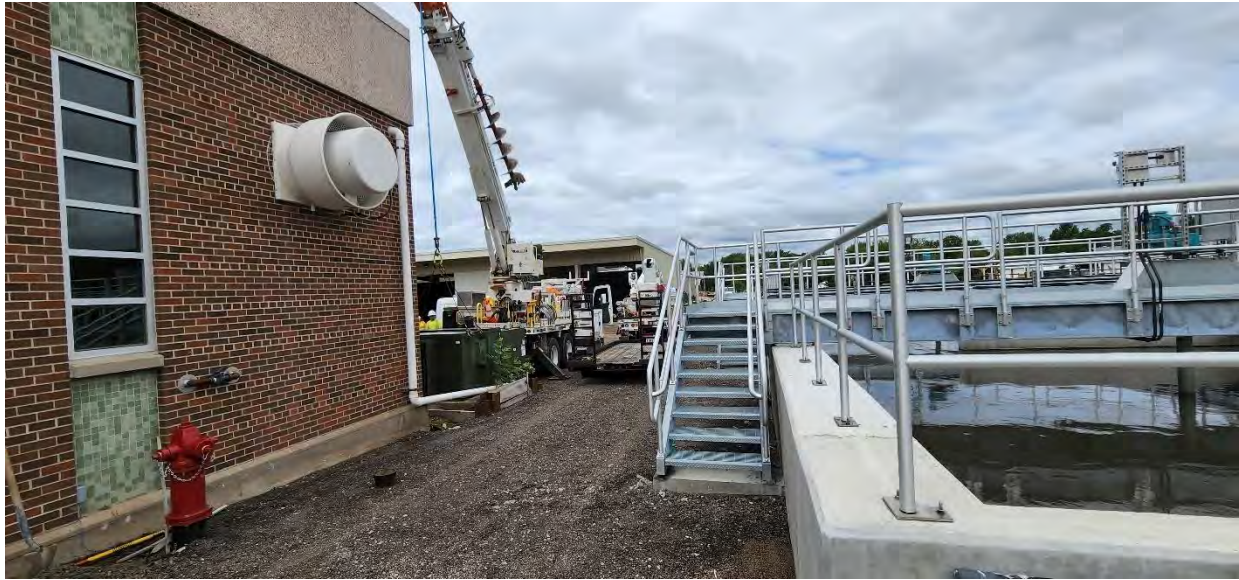
WPS removing old transformer at the northwest corner of Structure 400 (Activated Sludge Building).
