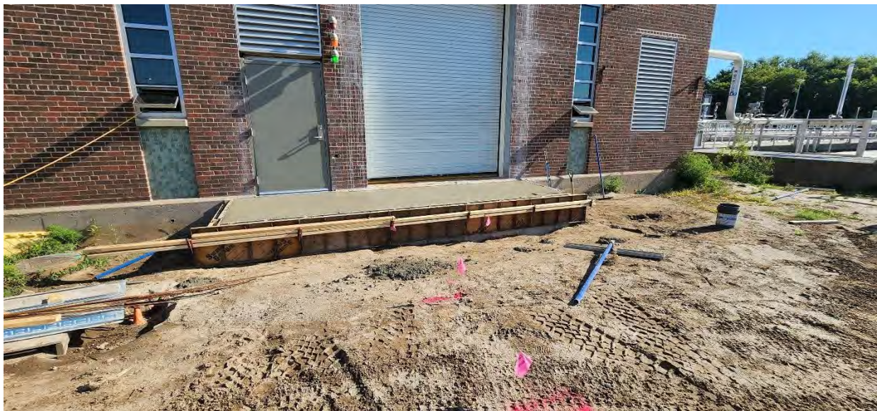
New concrete stoops for doors at Structure 400 (Activated Sludge Building).
