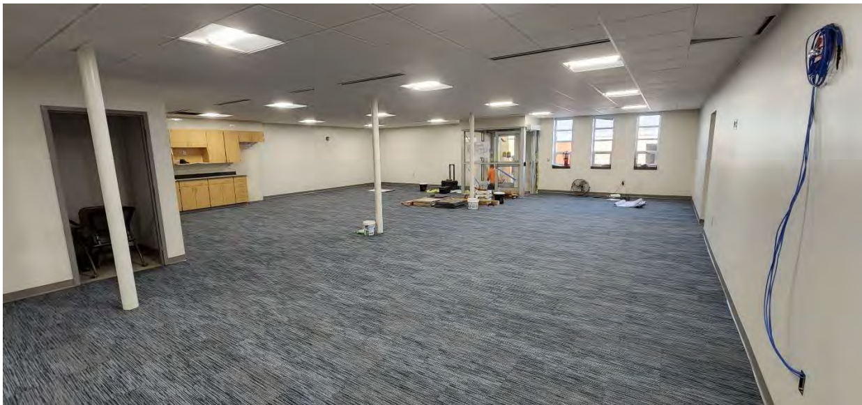
Flooring being placed in new training room of Structure 100.
