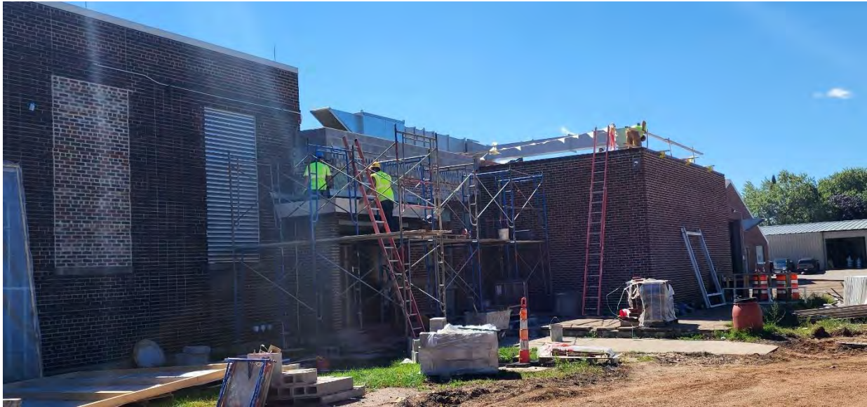
Mason starting brick inlay of demolished area from placement of new precast roof for raw wastewater pump room of Structure 100.
