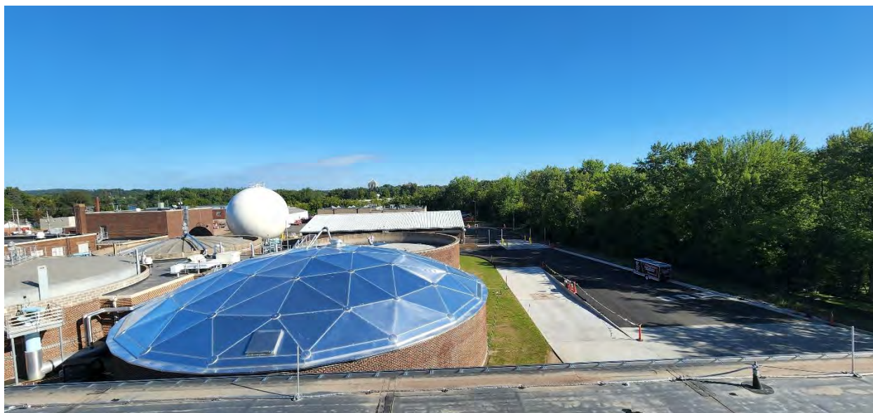
Looking north from the roof of Structure 770 (Solids Building).
