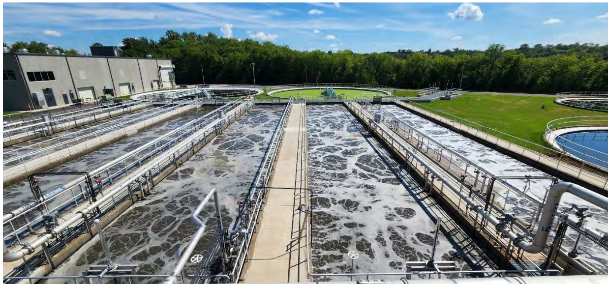
New handrail complete for Structure 410 (Activated Sludge Basins) and grass growing.
