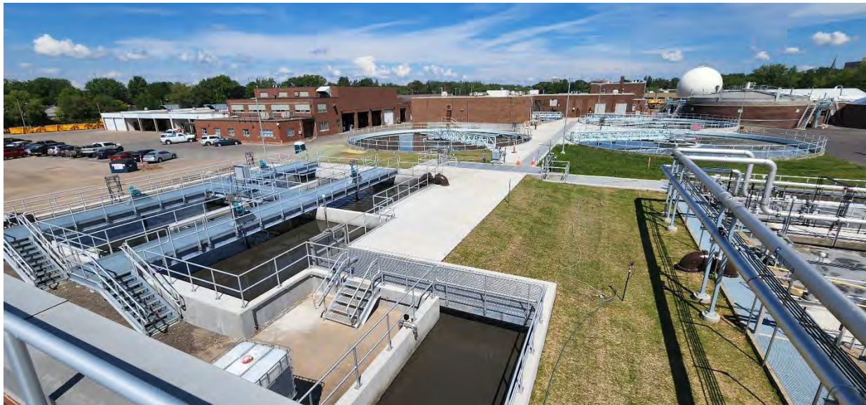
New grass planted between Structure 404, 405 and Primary Clarifiers
