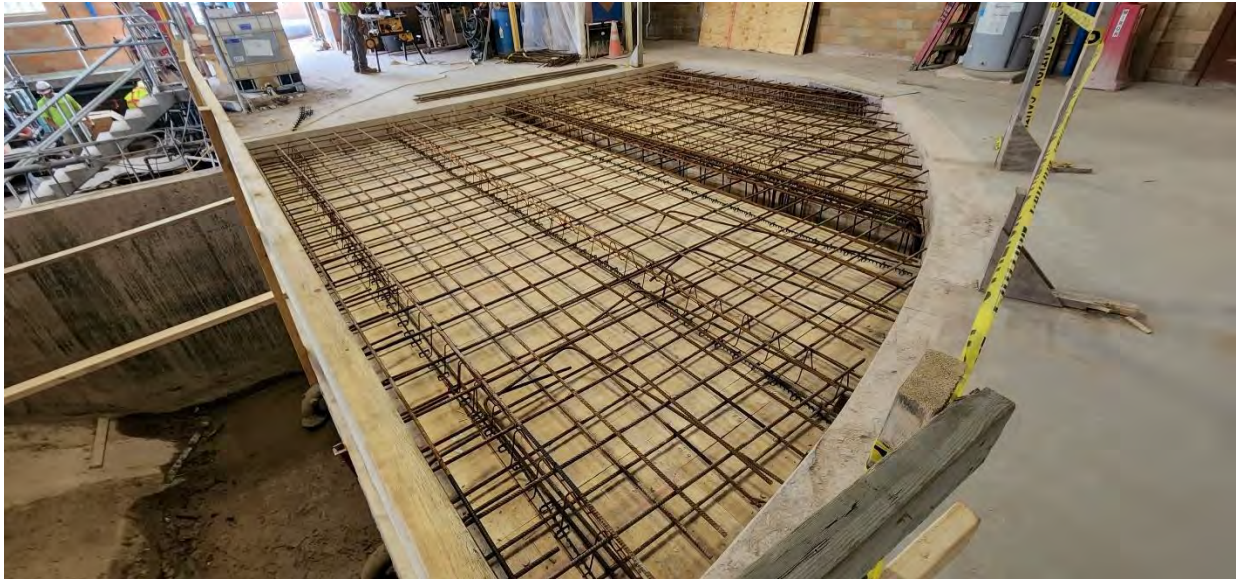
Rebar completed for one half of the new floor in the storage/shop area of Structure 100 (Main Building).
