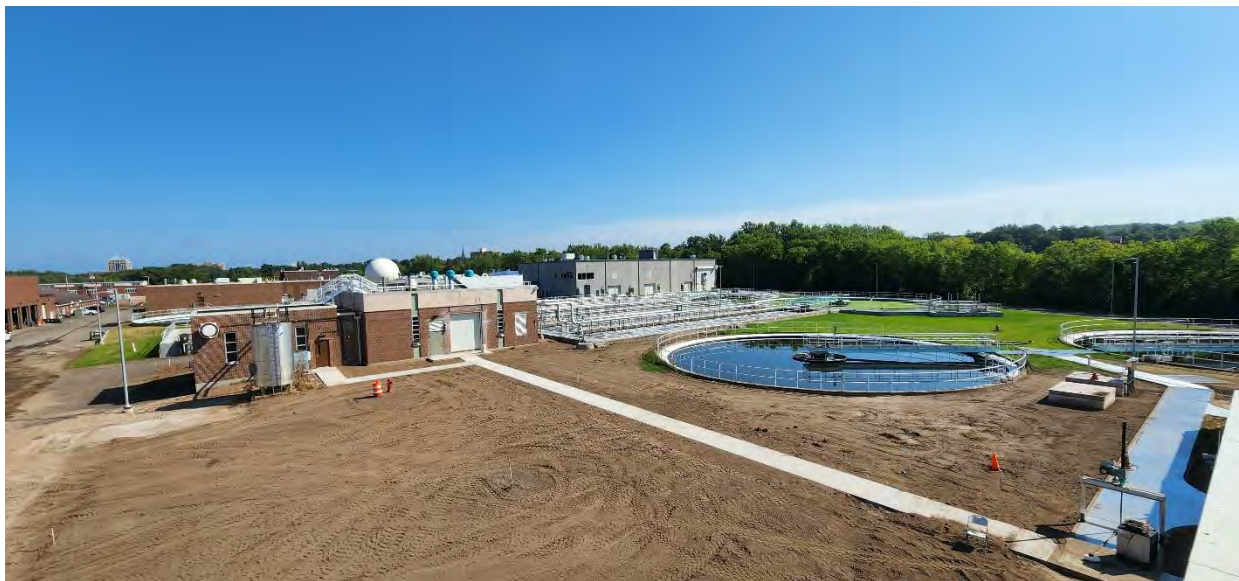
Topsoil placed and getting ready for mulch and seed between Structures 400 and 610 (Activated Sludge Building and Chemical Building).
