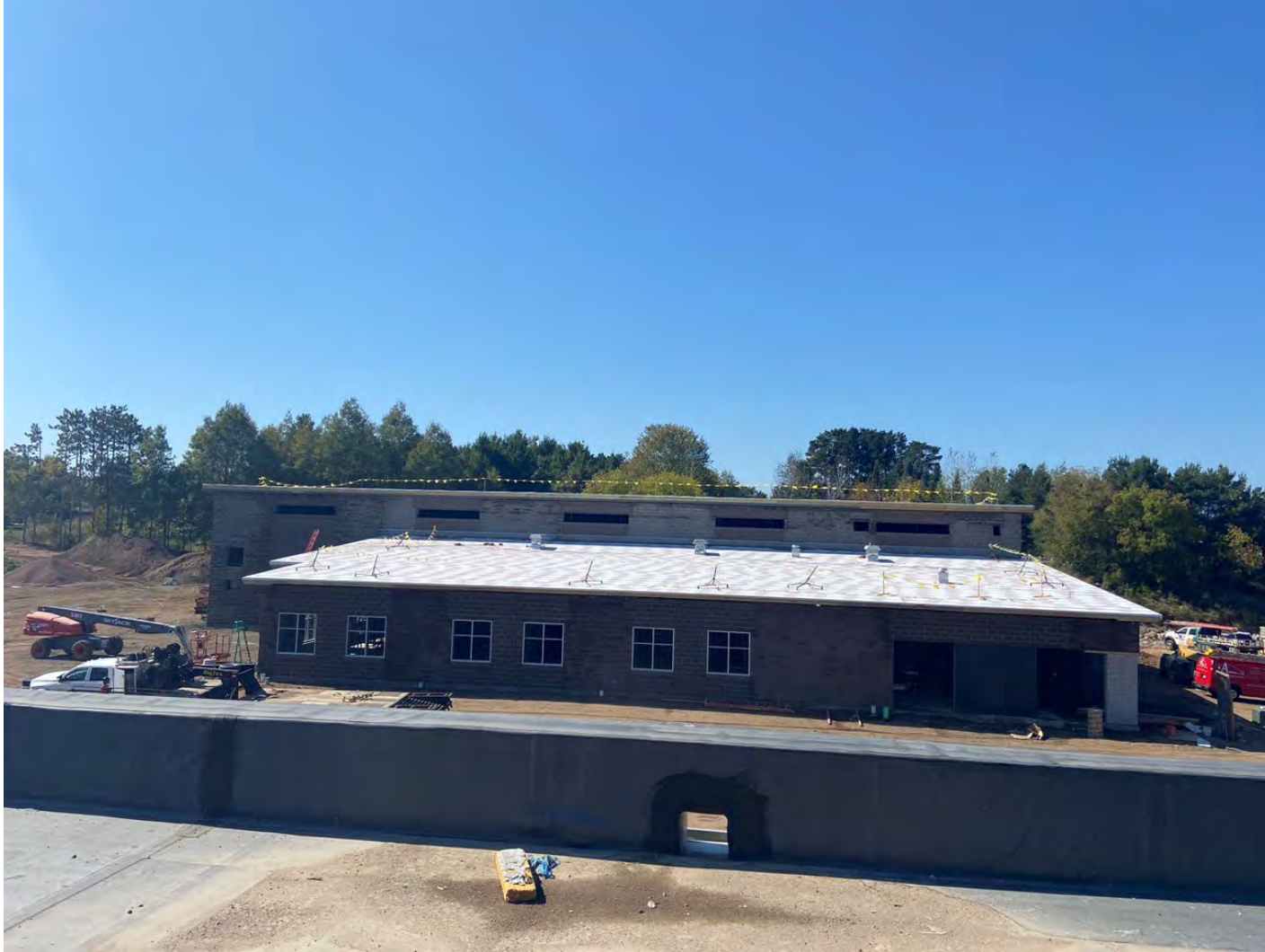
Administration Building from Roof of DWTF, looking West
