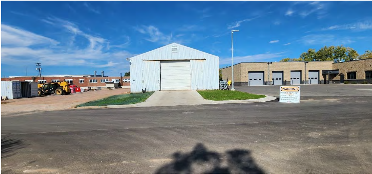
Final asphalt on Adrian Street and grass growing in front of Structure 115 (Equipment Storage Building).
