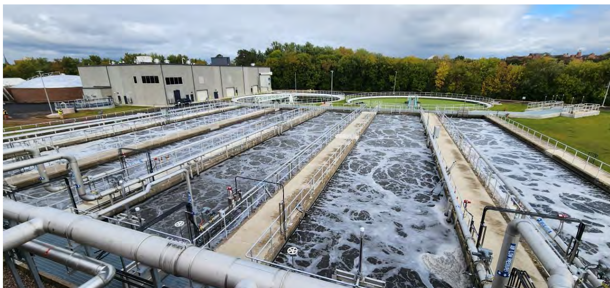
View from top of Structure 400 (Activated Sludge Building) looking east at aeration basins, new secondary effluent clarifier and Structure 770 (Solids Building).
