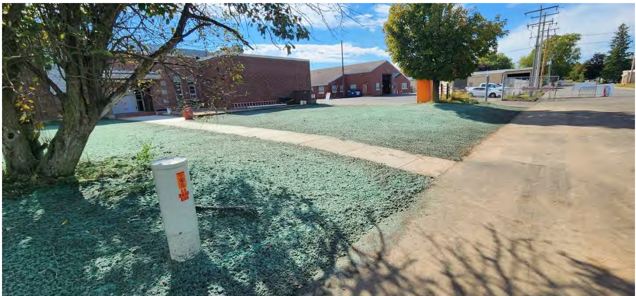
Mulch and seed, as well as new sidewalk in front of Structure 100 (Main Building).
