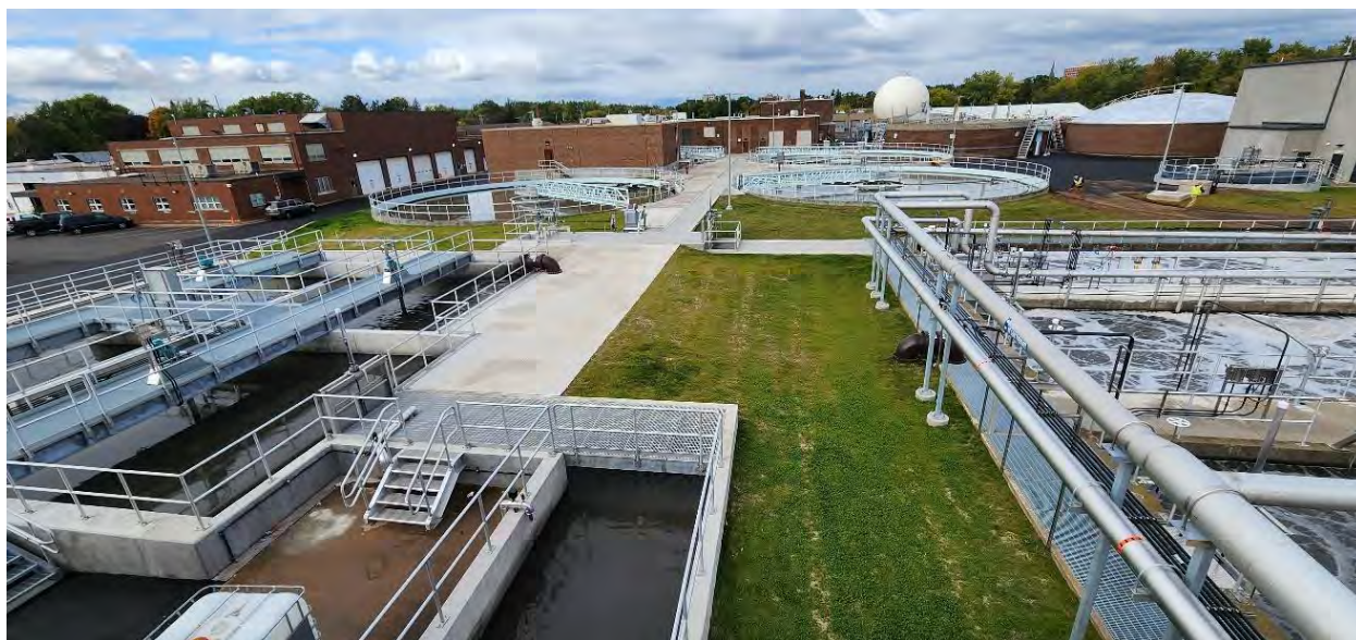
View from the top of Structure 400 (Activated Sludge Building) looking north
