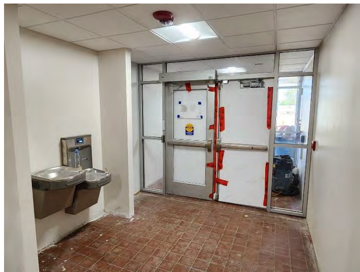
New main entrance foyer of Structure 100 (Main Building).
