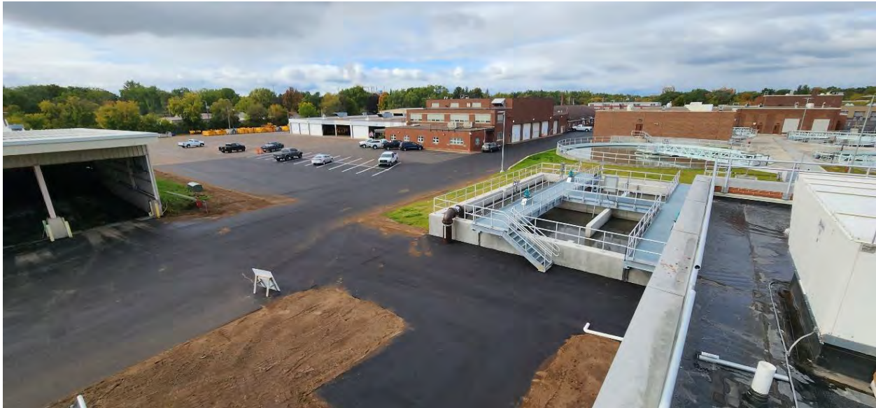
Final view from top of Structure 400 (Activated Sludge Building) looking northwest at Department of Public Works and Structure 405 (Anoxic Selector Tank).
