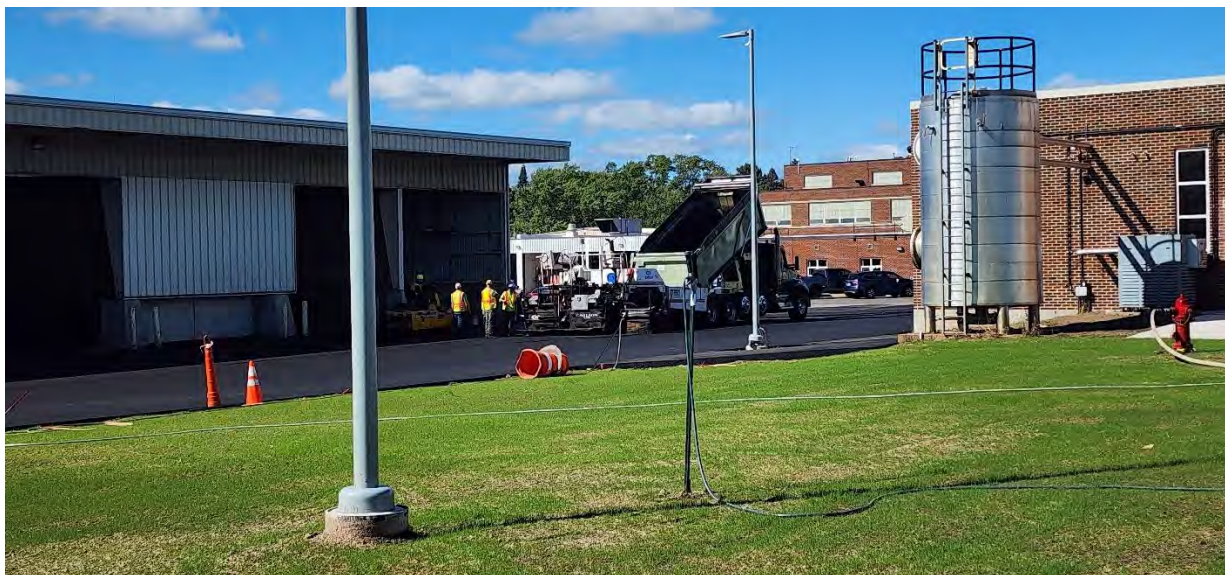
New asphalt east of Structure 760 (Biosolids Storage Building).
