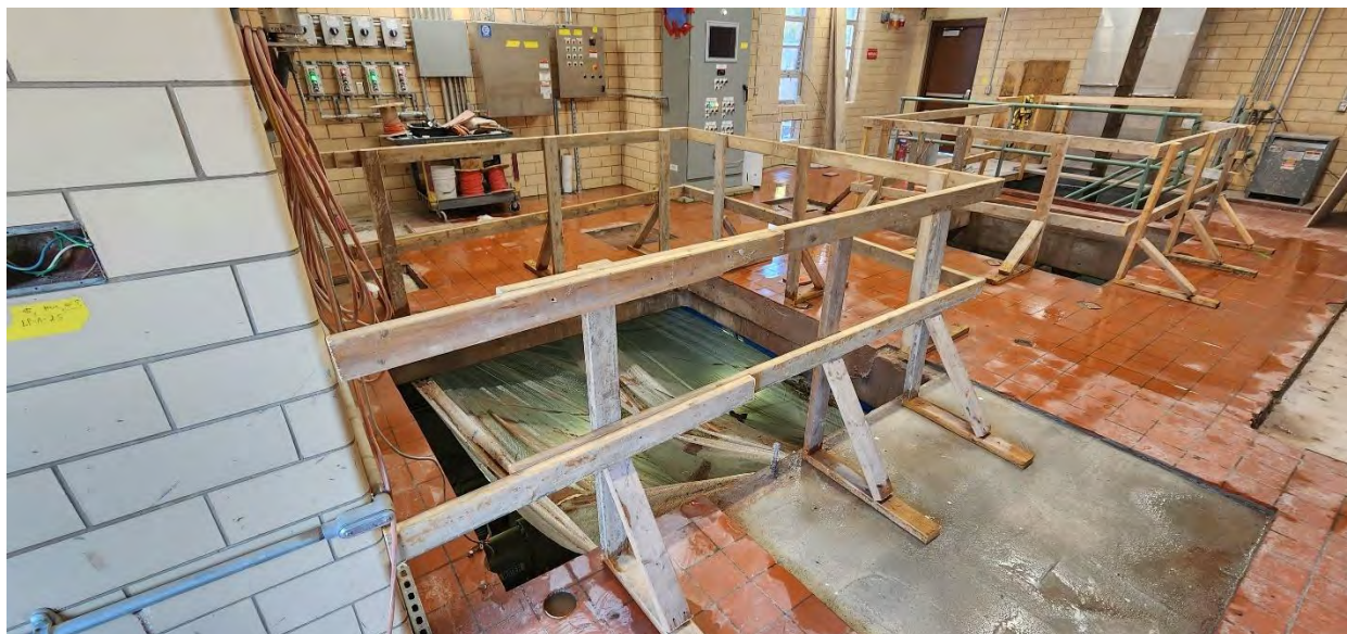
New raw wastewater (RWW) pump hatch openings in RWW pump electrical room of Structure 100 (Main Building).
