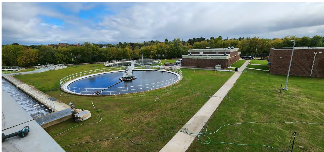
View from top of Structure 400 (Activated Sludge Building) looking southeast looking at Structures 510 and 520 (Secondary Clarifiers 1 and 2) and Structure (Effluent Building).
