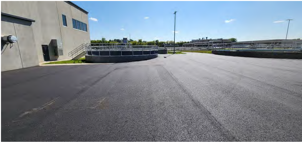
New asphalt on west side of Structure 770 (Solids Building) and around Structure 775 (PSD Thickener).
