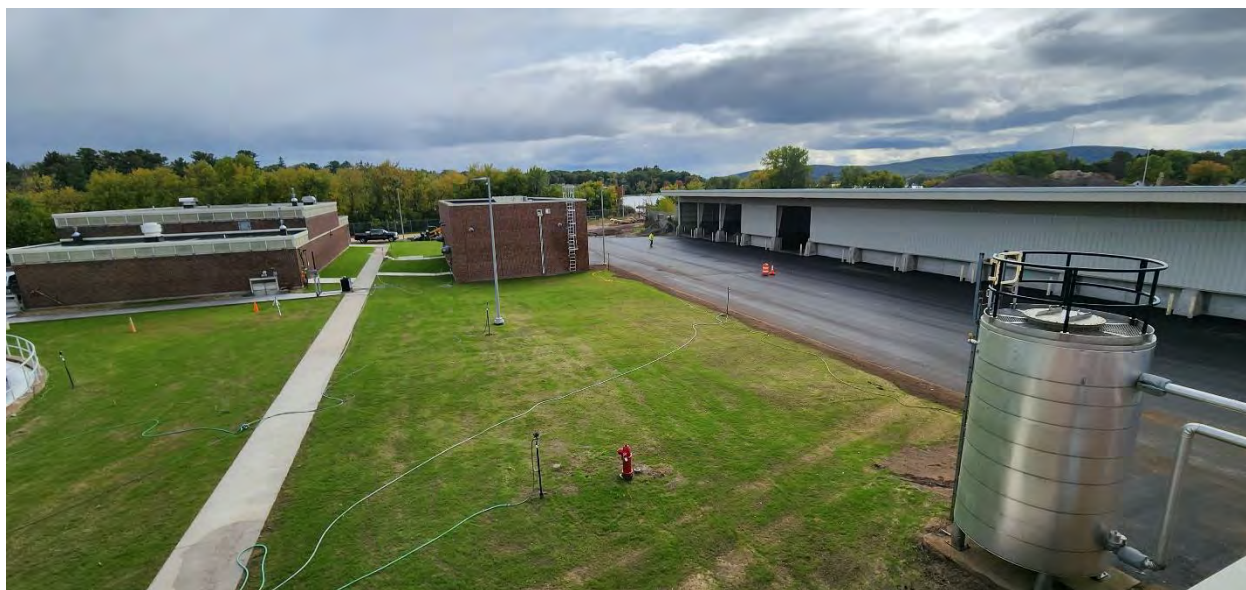
Looking south at Structure 600 (Effluent Building), Structure 610 (Chemical Building) and Structure 760 (Biosolids Storage Building), new grass and asphalt
