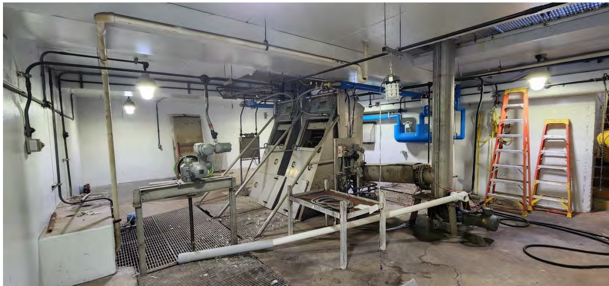
New paint in headworks screen room of Structure 100 (Main Building).
