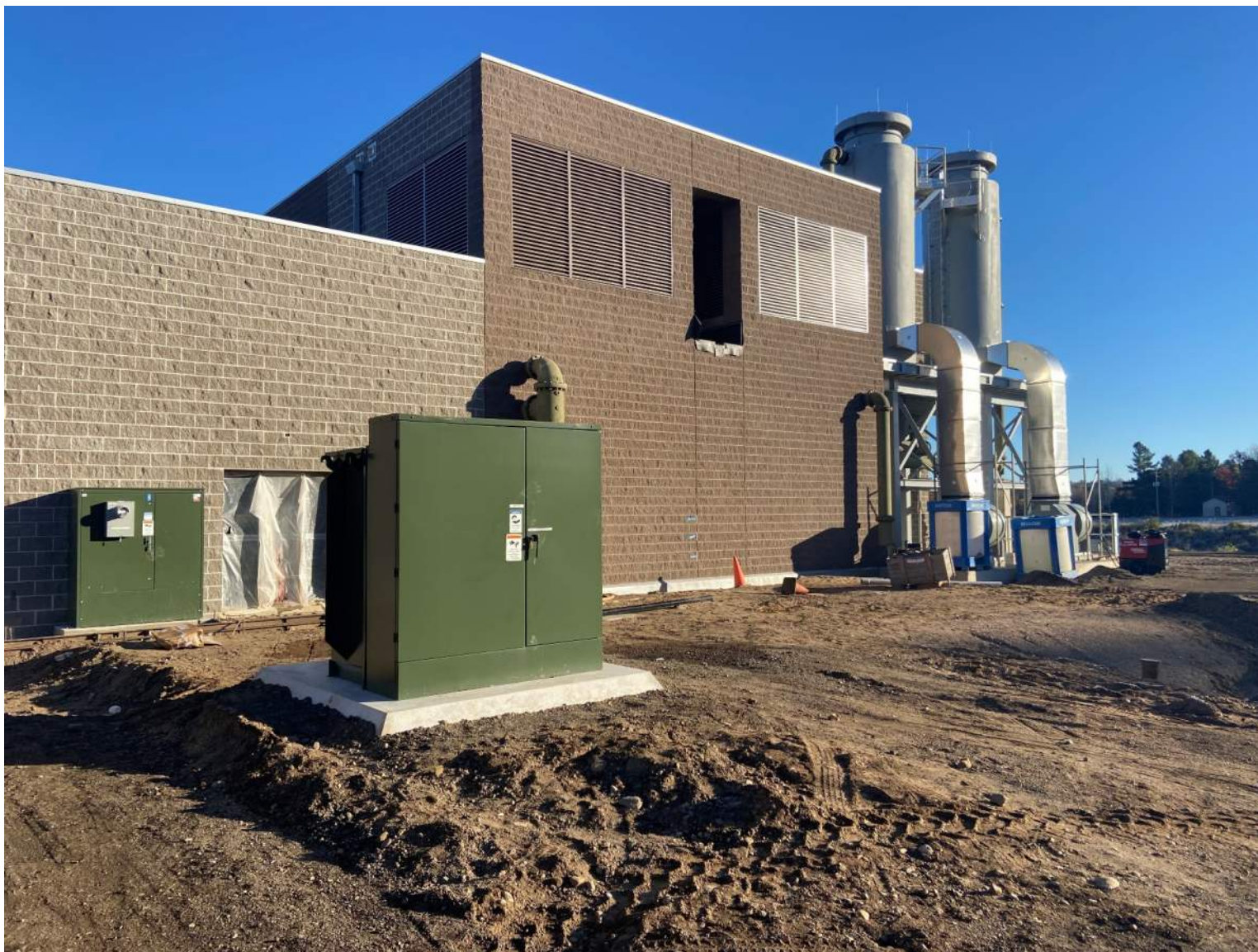
WPS installed regulator and power supply to site
