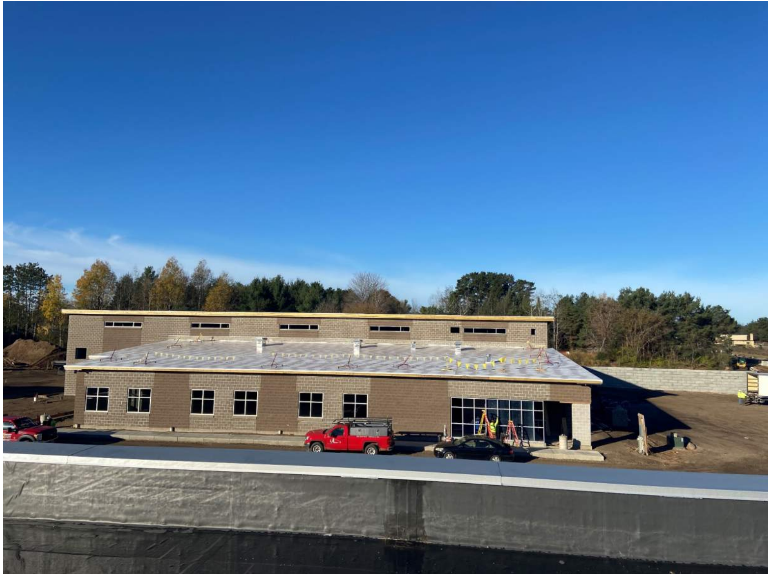
Concrete walks along vehicle storage / administration building
