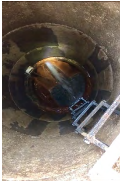
Joints, Steps, Service Connections in Manholes
