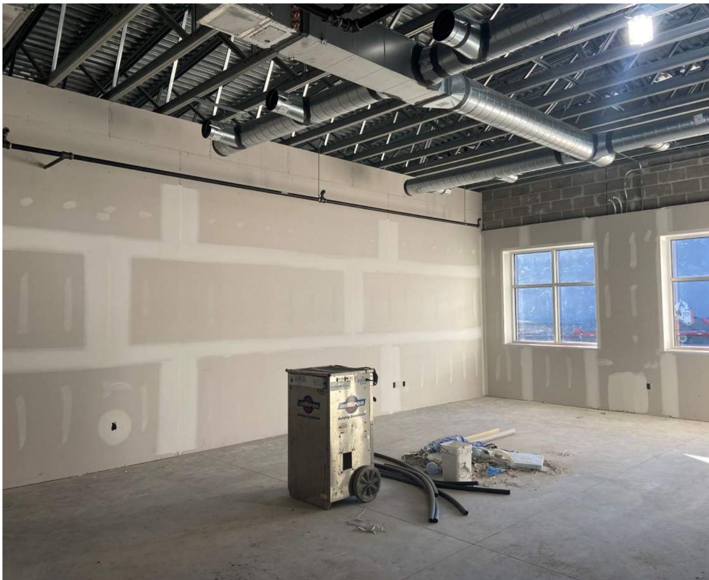
Drywall in conference room at vehicle storage / administration building
