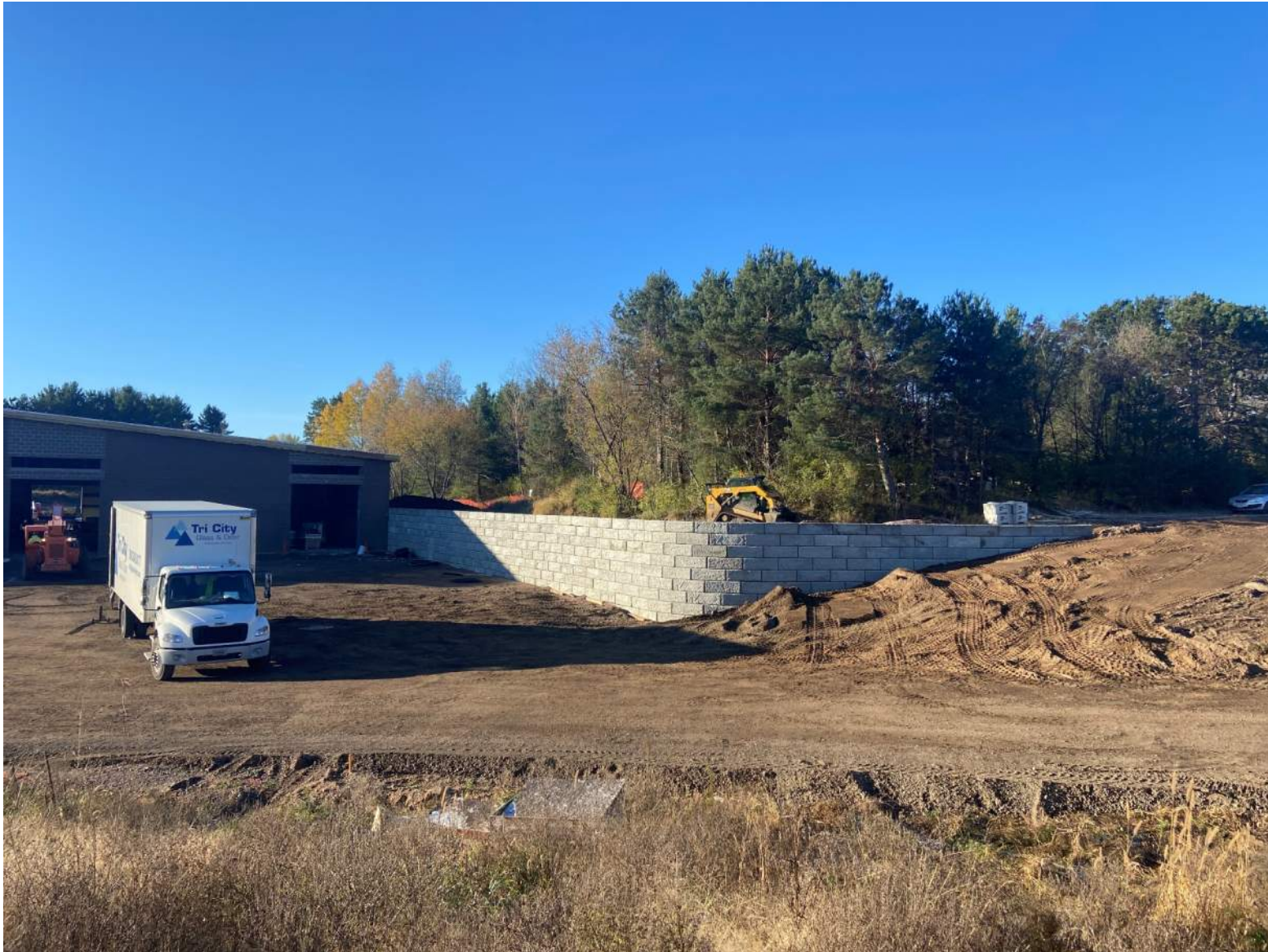
Retaining wall adjacent to vehicle storage / administration building
